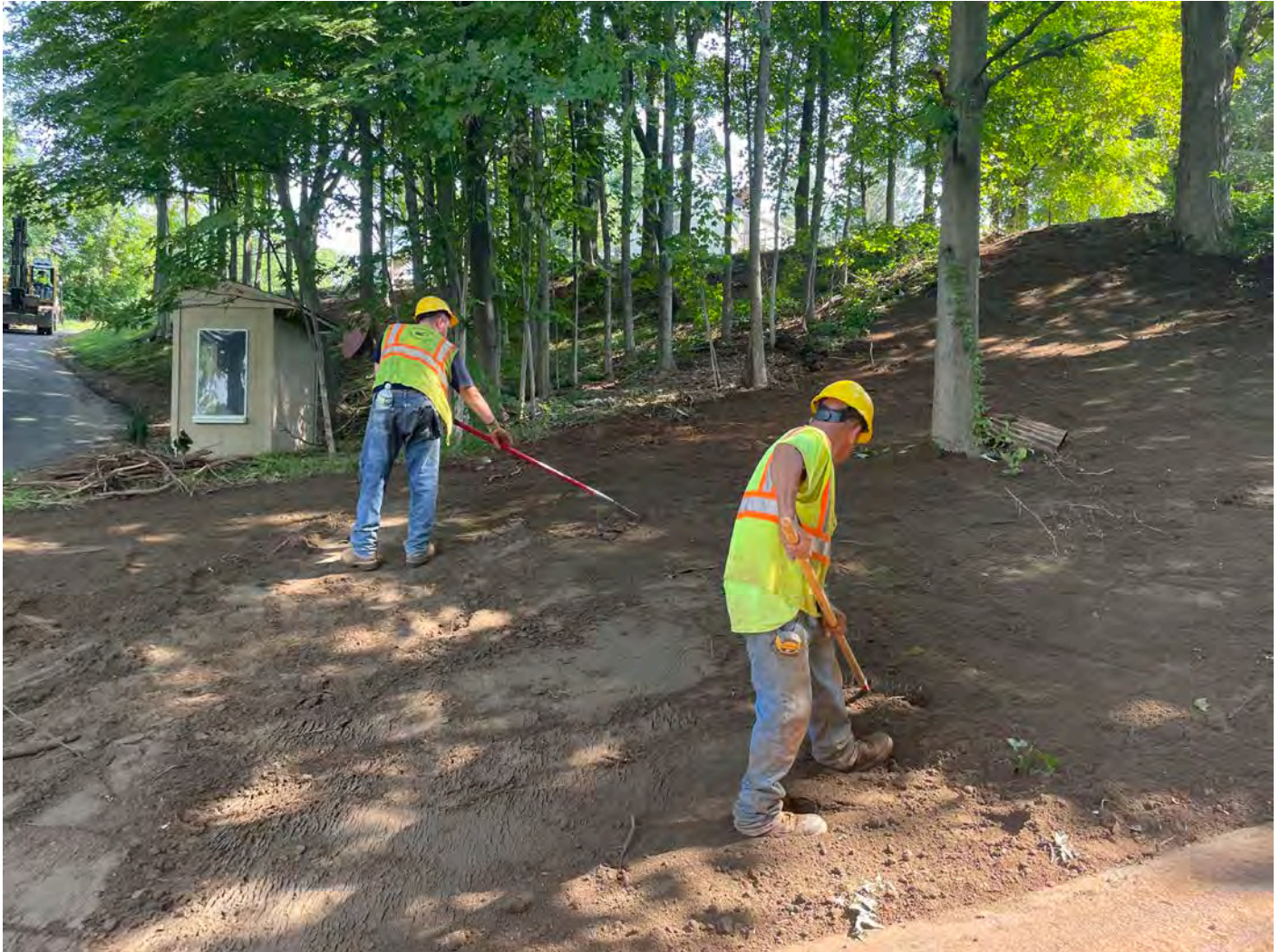
Picture 9: Ludlow grading loam on a portion of the 95R Maple Avenue property that was disturbed during the installation of a 2" copper water service line. View to northeast.
