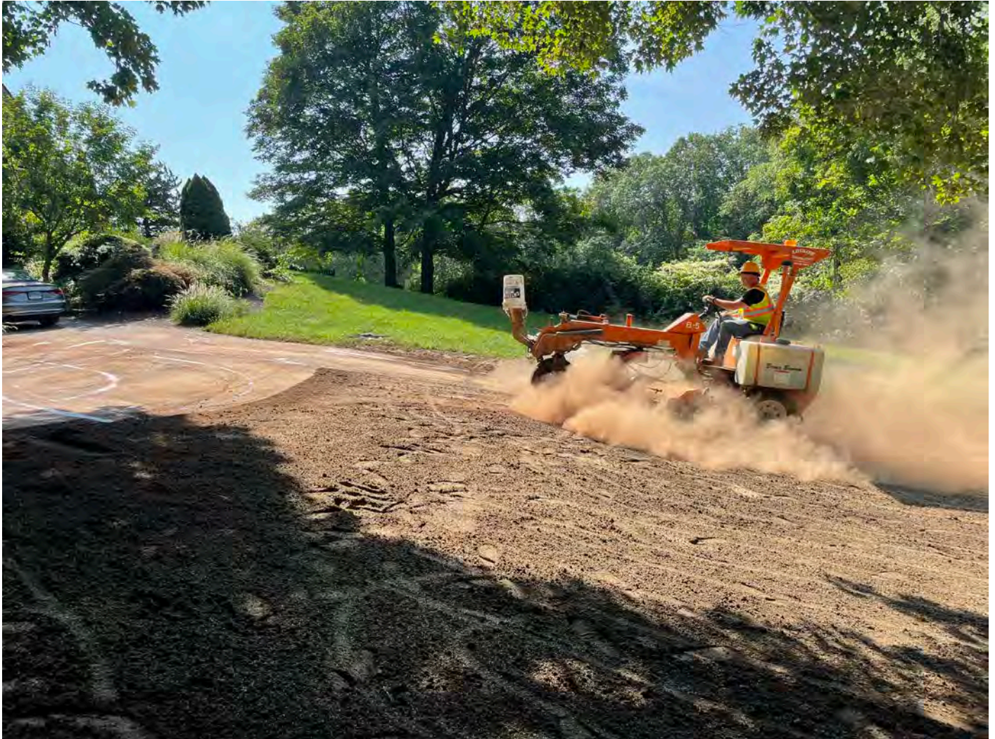
Picture 8: Ludlow using a Broce Broom to clean the driveway of the 95R Maple Avenue property. View to south.
