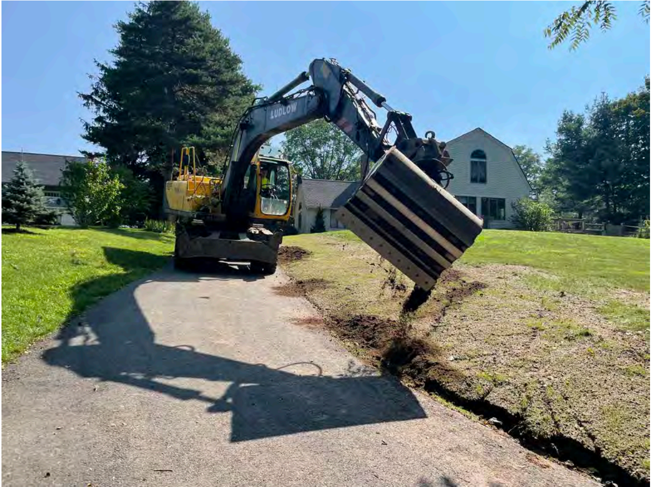
Picture 7: Ludlow placing loam on the south side of the 97 Maple Avenue property to fix some recent erosion damage to the loam and grass seed they placed recently.
