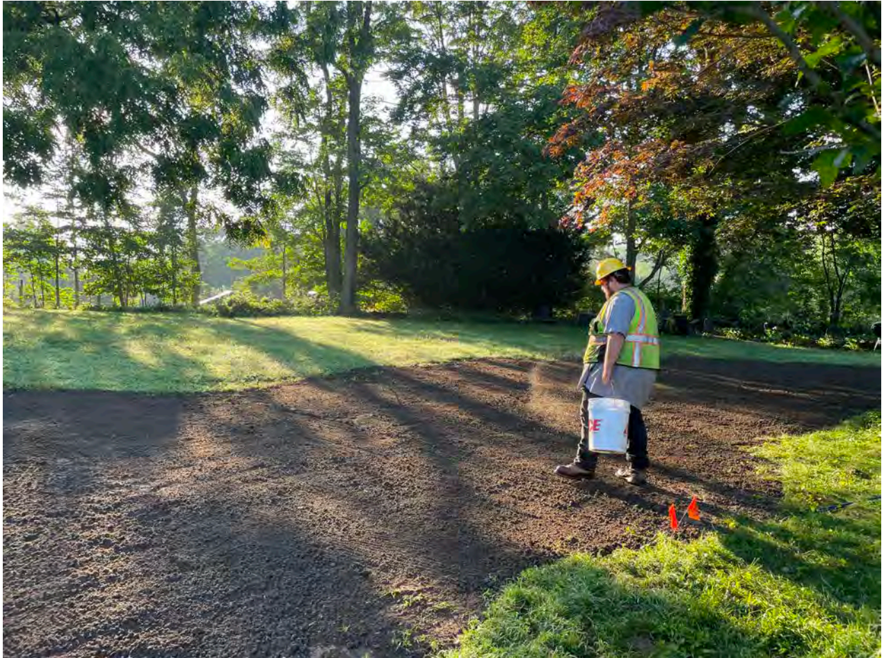
Picture 3: Ludlow placing grass seed over freshly placed loam on the east side of the 95R Maple Avenue residence. View to the southeast.
