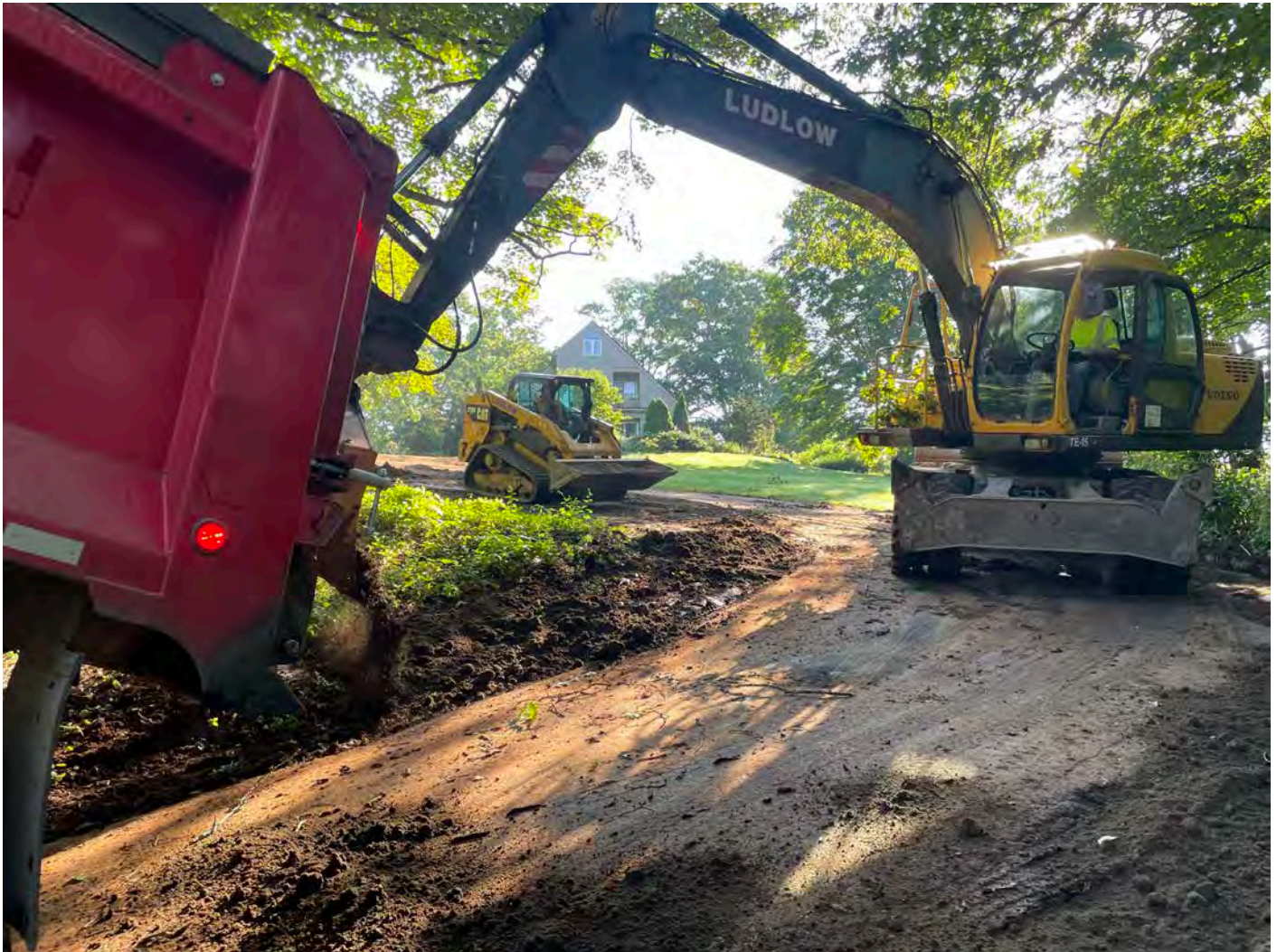
Picture 5: Ludlow placing loam on the north side of the driveway for the 95R Maple Avenue residence. View to the southeast.
