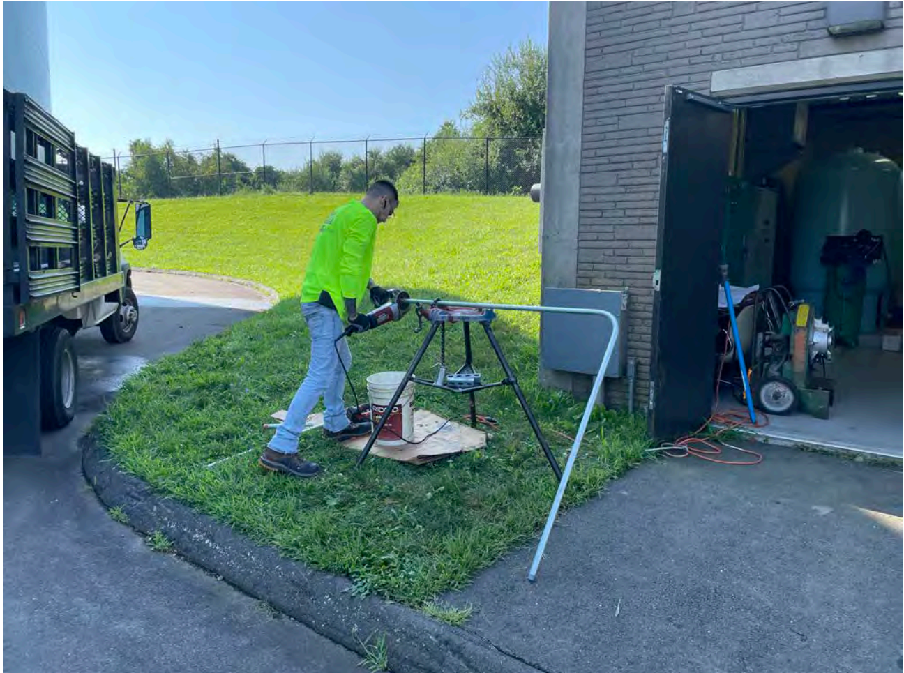
Picture 2: A&R Electrical threading the end of a steel conduit that will be installed inside of the Long Hill pump station in Middletown. View to the southeast.
