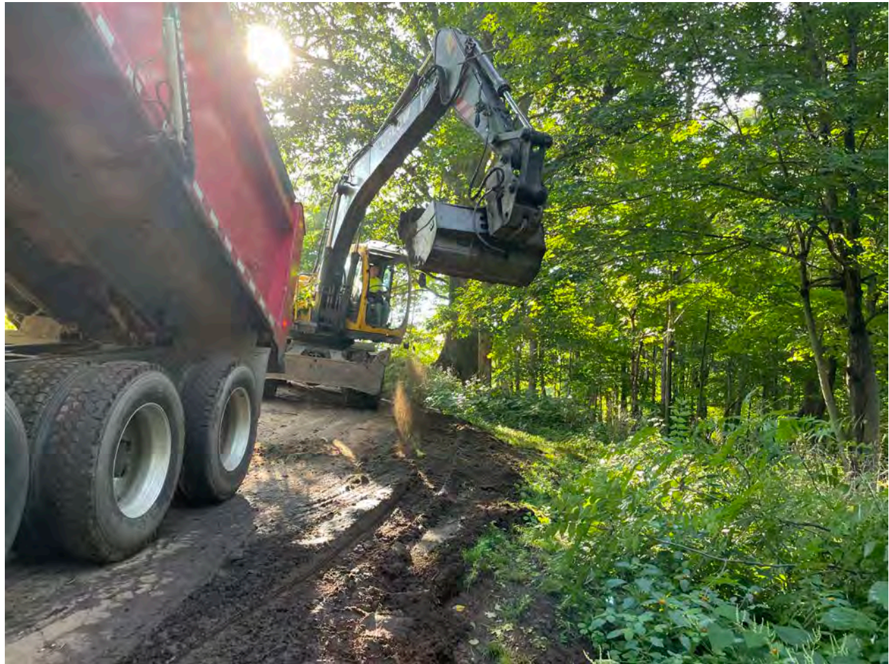
Picture 4: Ludlow placing loam on the south side of the driveway for the 95R Maple Avenue residence. View to the southeast.
