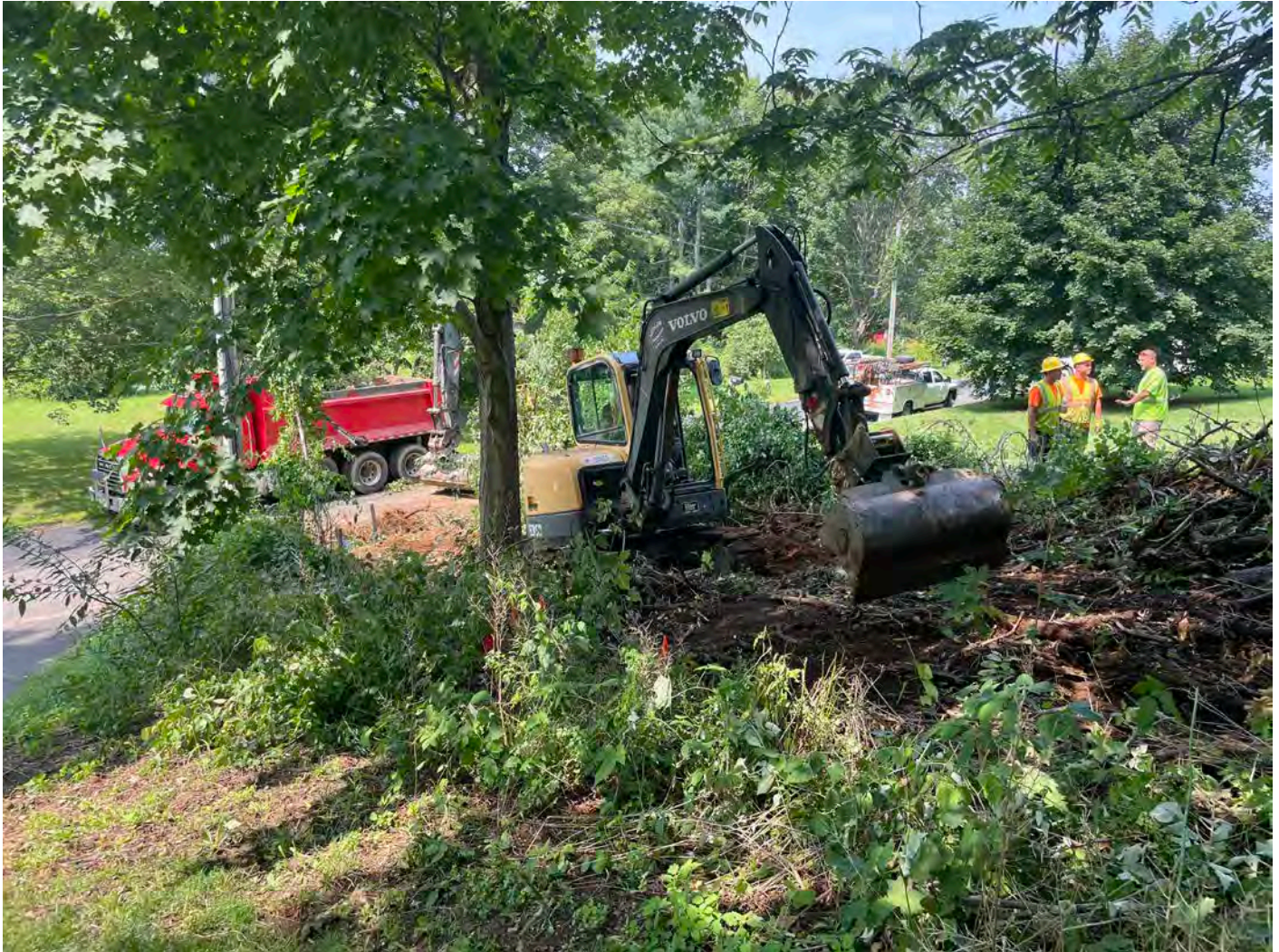
Picture 10: Ludlow grubbing brush on the northern property line of the 109 Maple Avenue property. View to northwest.
