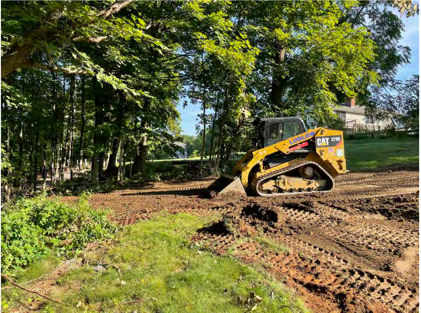
Picture 6: Ludlow grading loam on the 95R Maple Avenue property. View to the north.
