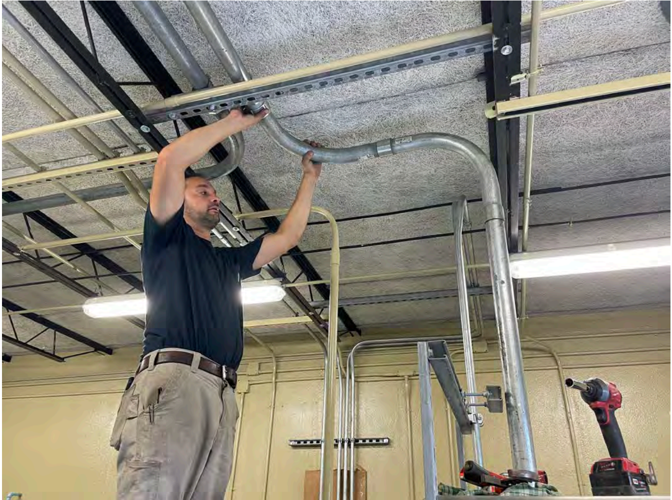
Picture 1: A&R Electrical installing a 2" steel conduit at the Long Hill pump station in Middletown.
