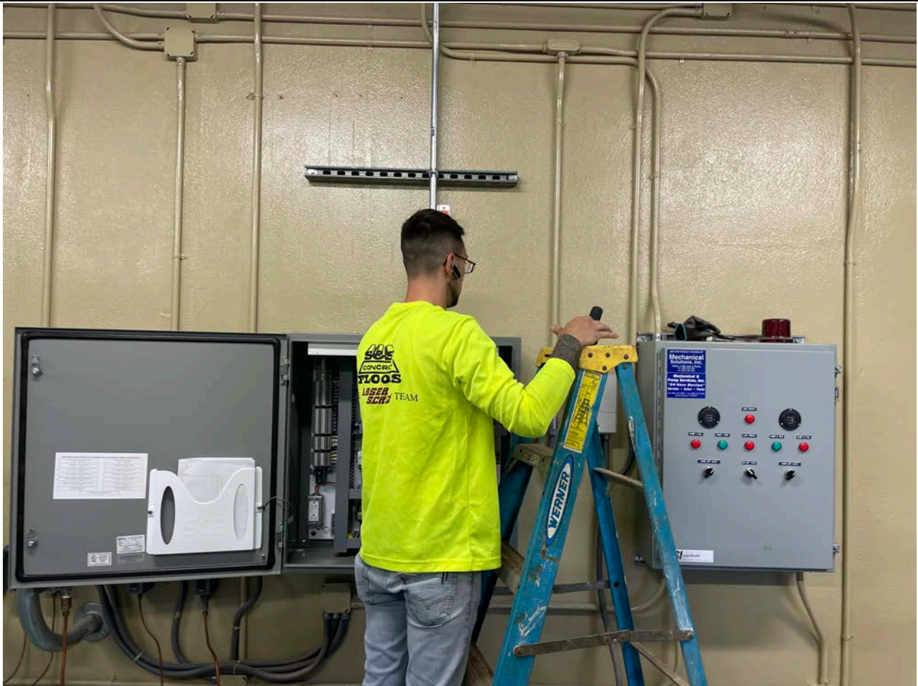
Picture 2: -A&R Electrical working on an instrumentation panel at the Long Hill pump station. View to the west.
