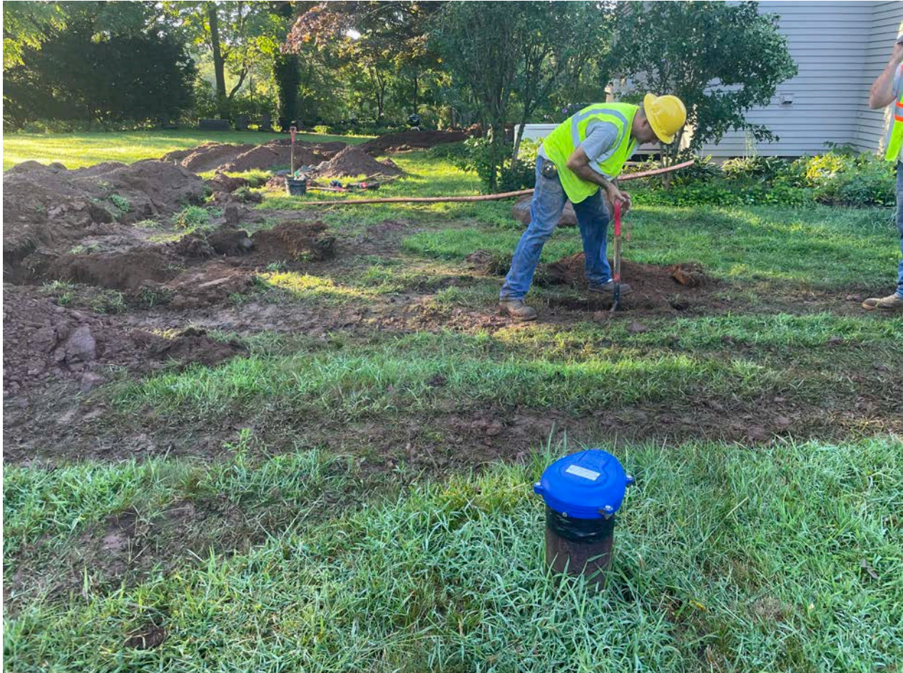
Picture 3: Ludlow hand digging to locate the water line between the 95R Maple Avenue residence and it's drinking well. View to the south.
