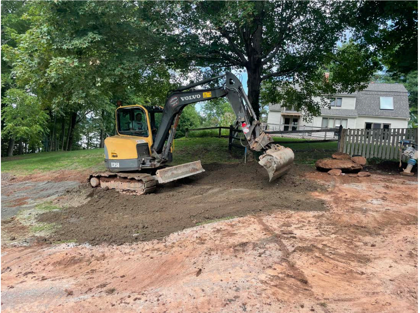
Picture 8: Ludlow grading loam over the backfilled trench at the 95R Maple Avenue property. View to north.
