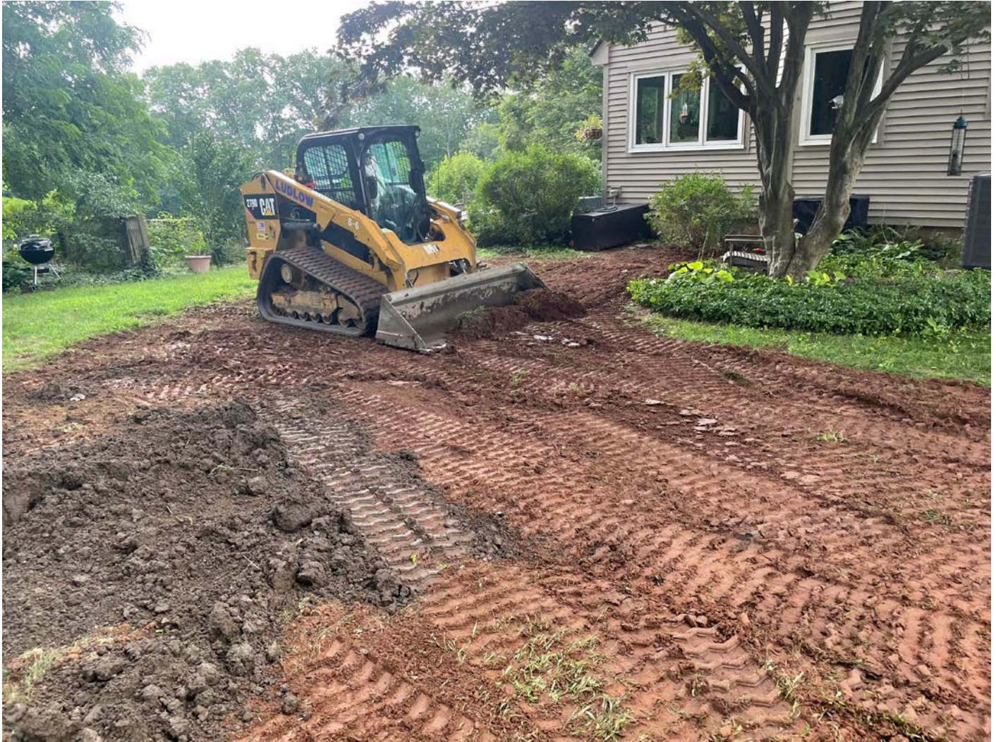
Picture 9: Ludlow grading loam over the backfilled trench at the 95R Maple Avenue property. View to southwest.
