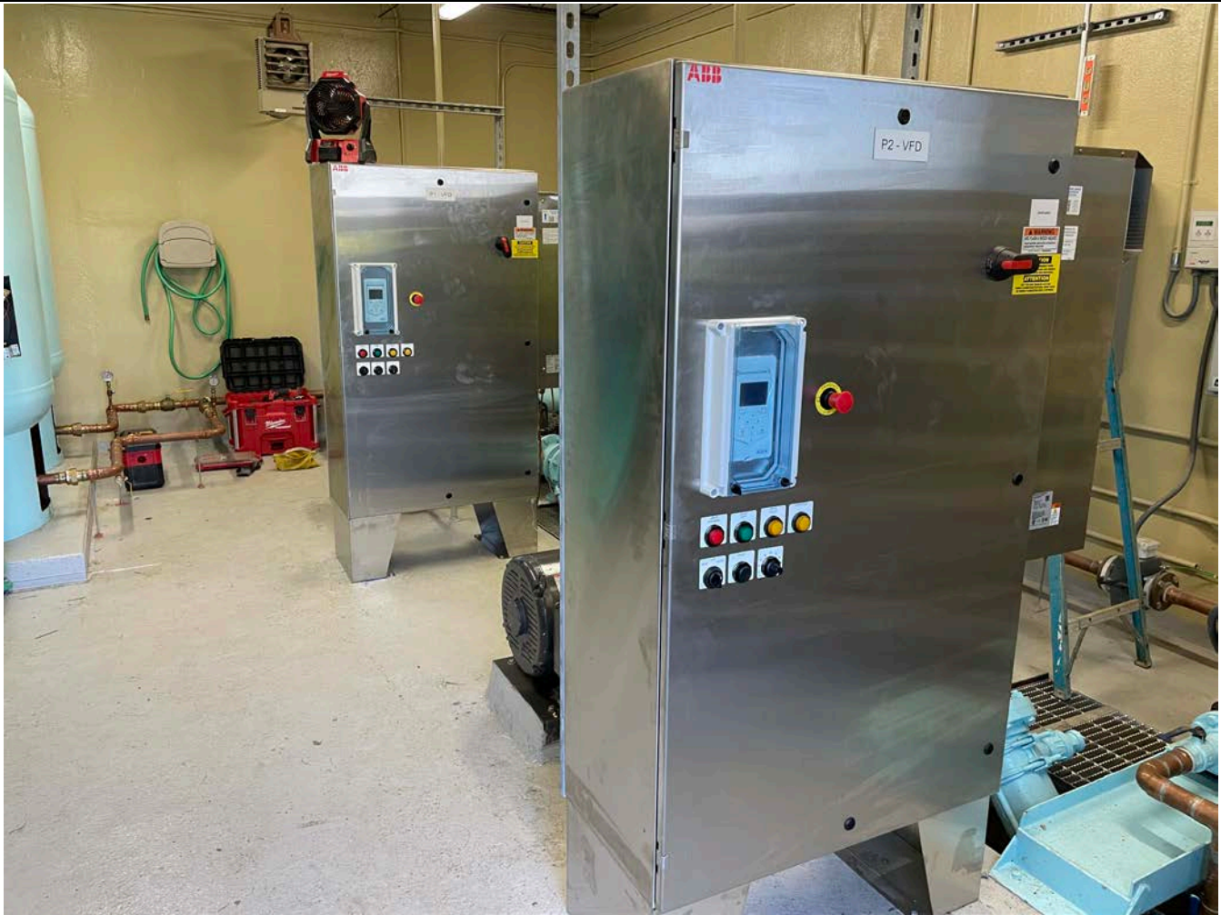
Picture 1: Long Hill pump station where A&R Electrical has installed two VFD cabinets. View to the south.
