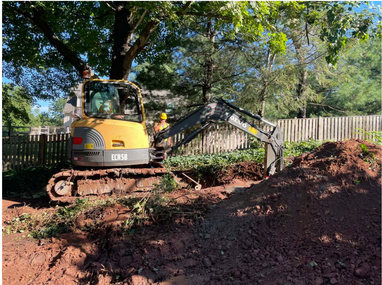
Picture 4: Ludlow excavating for the installation of a 2" copper water line at the 95R Maple Avenue residence. View to the north.
