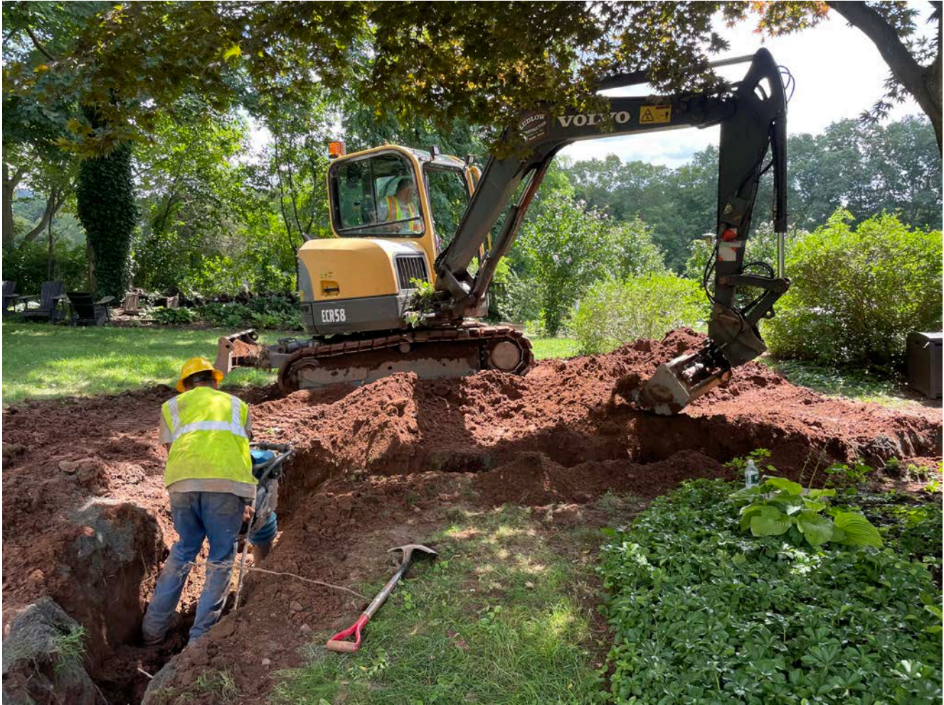
Picture 7: Ludlow placing sand over placed 2" copper water service on the east side of the 95R Maple Avenue residence. View to south.
