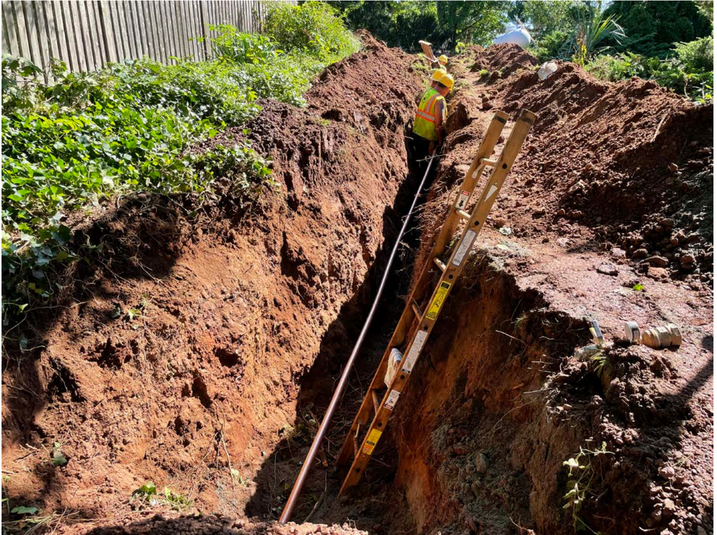
Picture 5: Ludlow placing 2" copper water service line at the 95R Maple Avenue property. View to the east.
