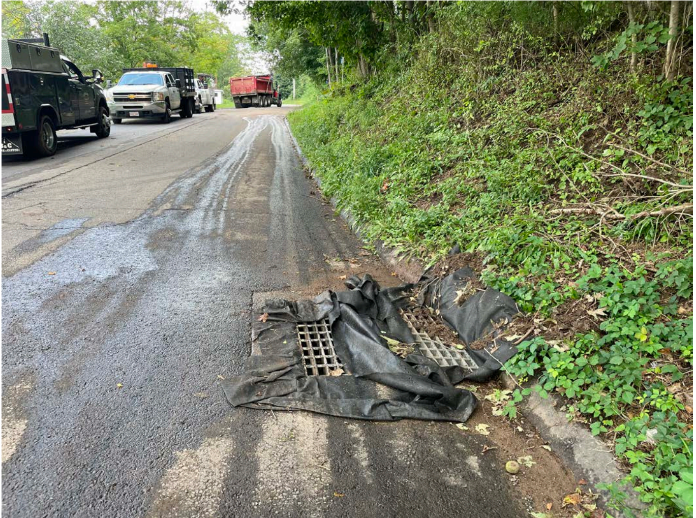
Picture 6: Filter fabric placed at a catch basin on the east side of Maple Avenue; south and downgradient of 95R Maple Avenue. View to the north.
