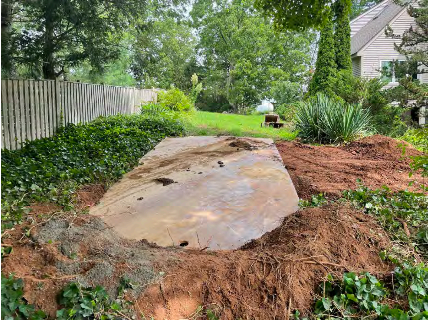
Picture 6: Steel plate that Ludlow placed over a portion of the excavation at the 95R Maple Avenue property. View to the east.
