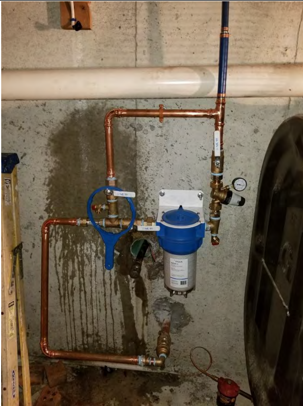
Picture 2: -Final water service components that Fazzino Plumbing installed at the 10 Johns Way residence in Durham.
