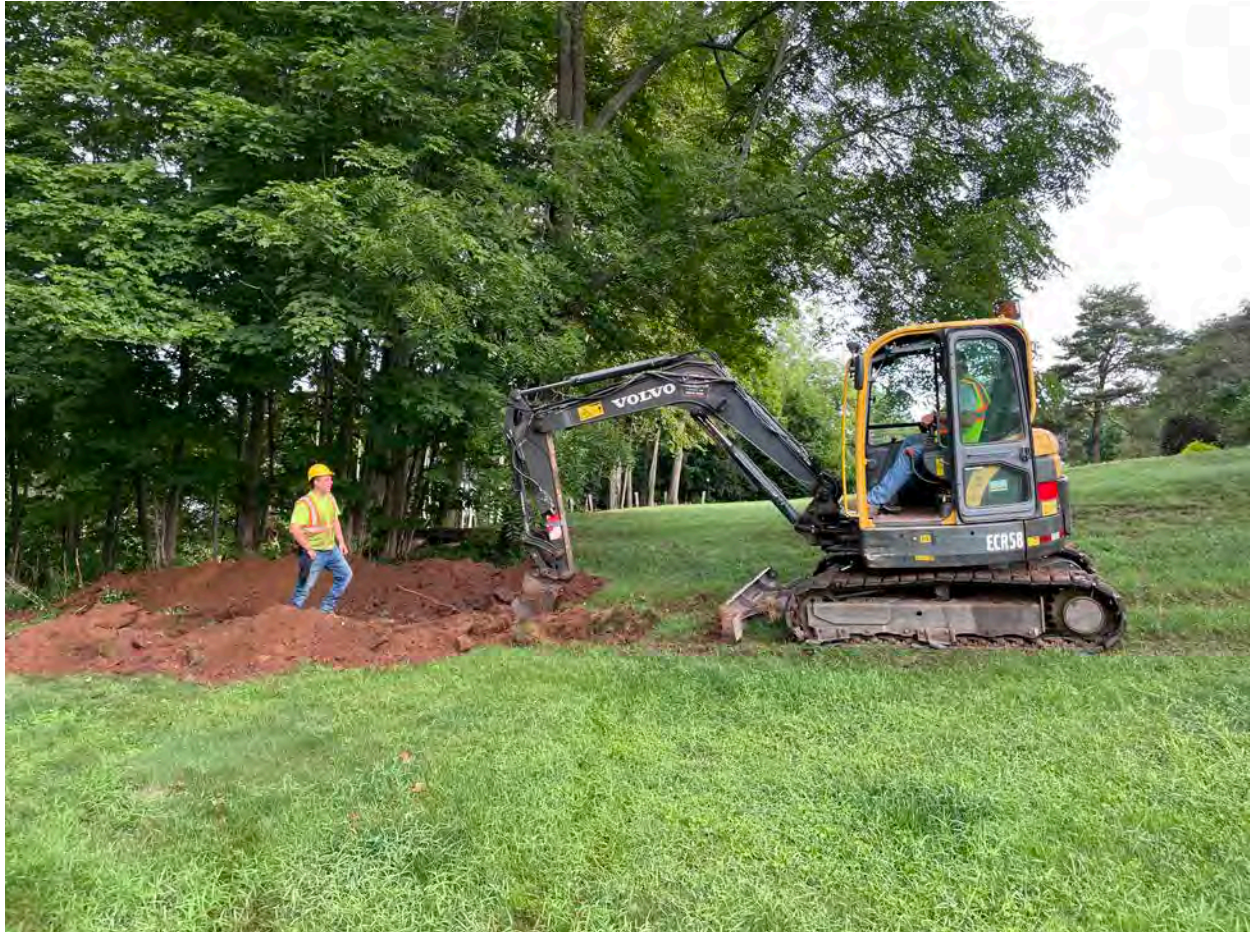
Picture 1: Ludlow excavating at the 95R Maple Avenue property for the installation for 2" copper water service line. View to the north.
