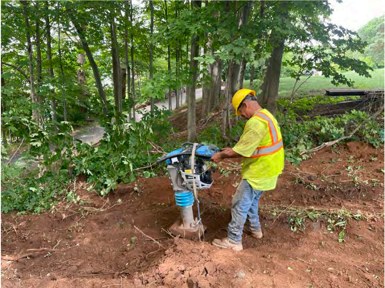
Picture 7: Ludlow compacting native fill that was placed back in the trench with a jumping jack. View to north.
