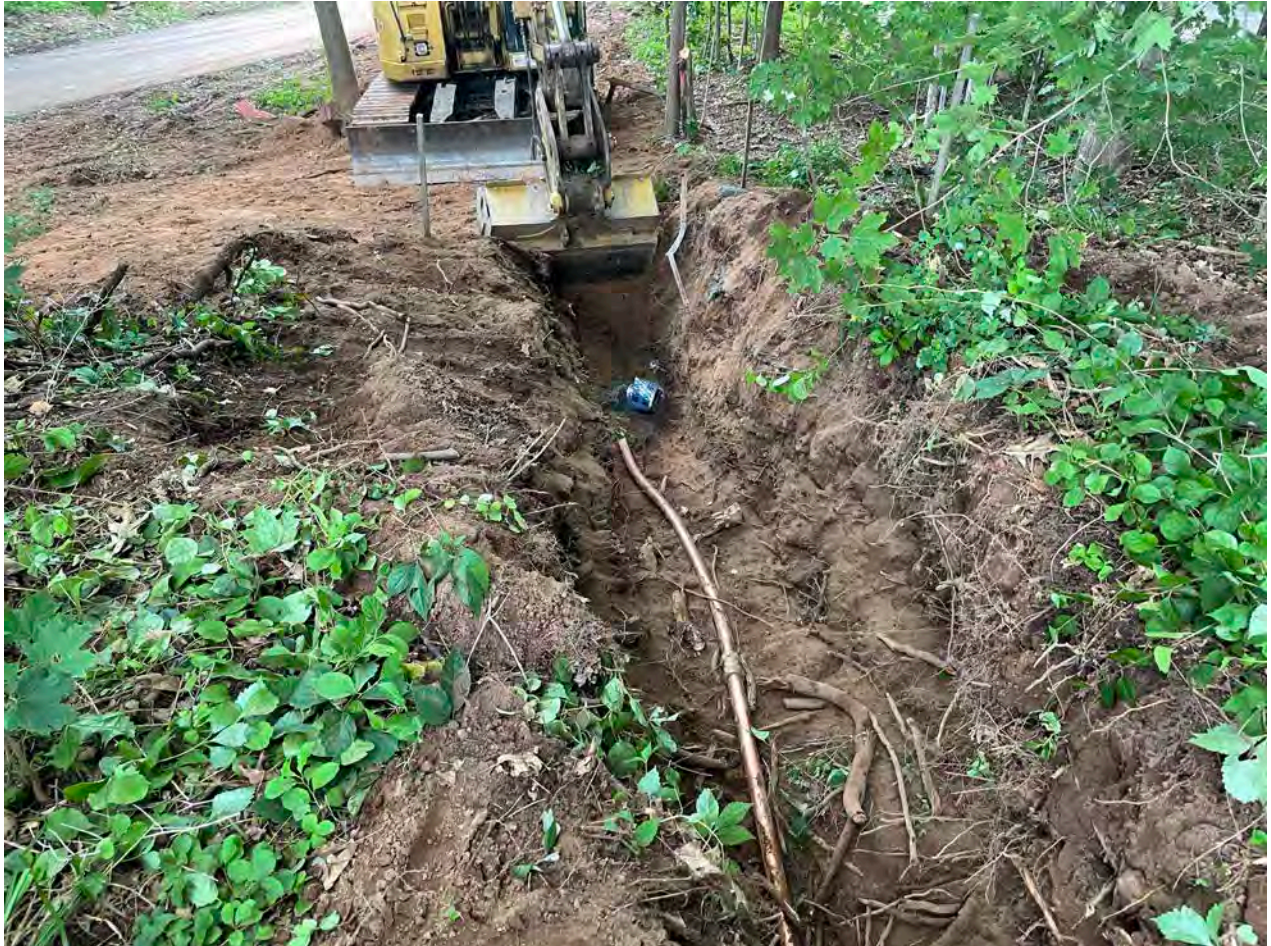
Picture 3: Ludlow installing 2" copper water service line next to Maple Avenue at 95R Maple Avenue in Durham. View to the west.
