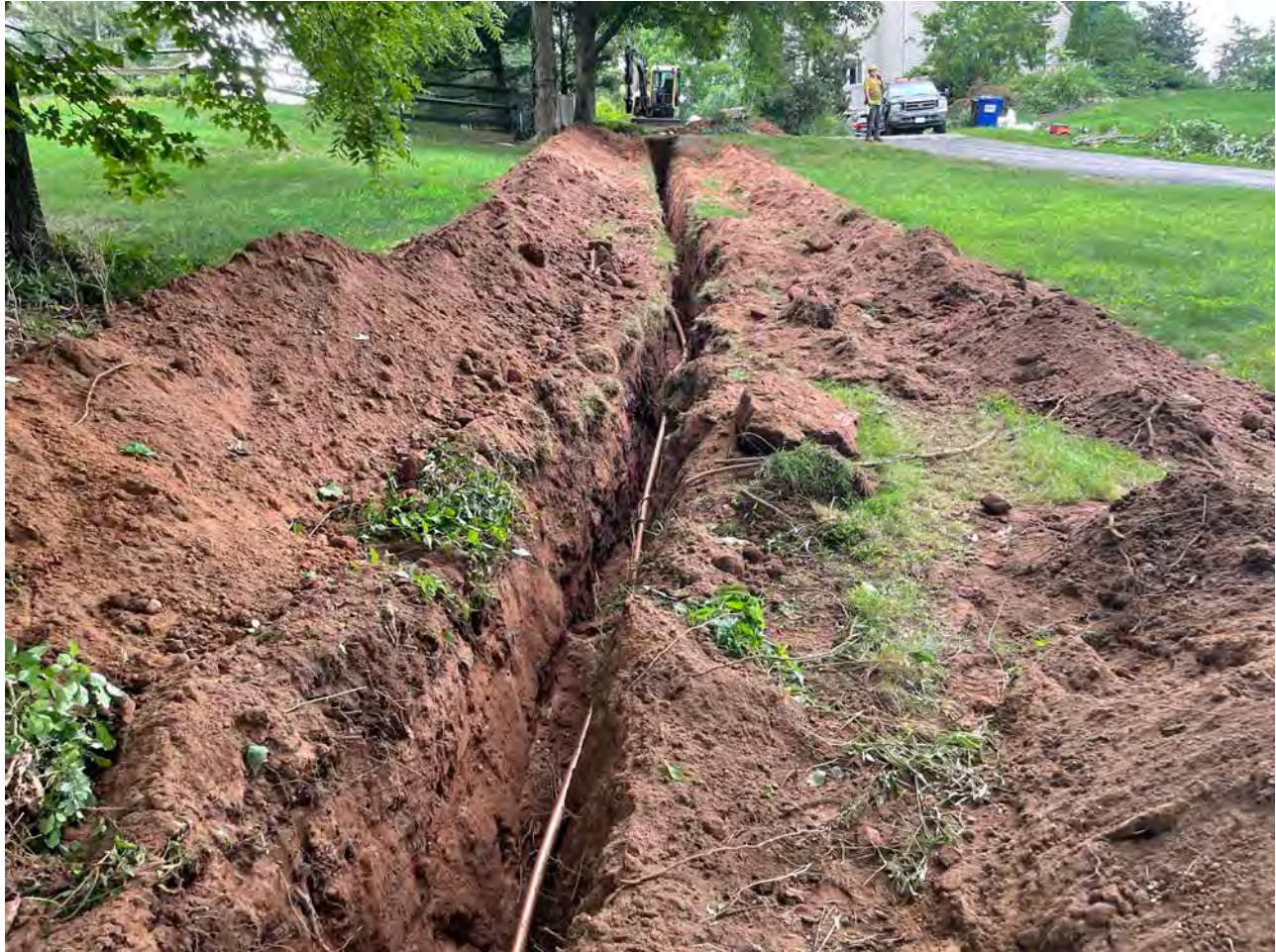
Picture 4: 2" copper pipe that Ludlow has placed in the trench they excavated at the 95R Maple Avenue property. View to the east.
