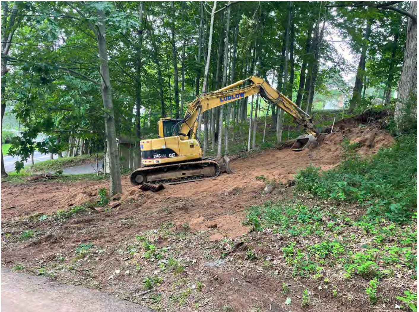
Picture 5: Ludlow placing native fill over the 2" copper water service they installed line next to Maple Avenue at 95R Maple Avenue in Durham. View to the west.
