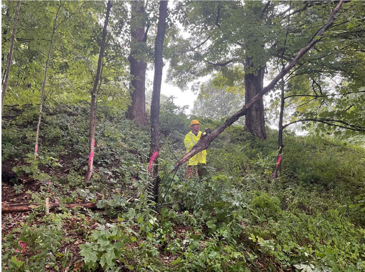
Picture 1: Ludlow clearing a path at the 95 Maple Avenue property for the installation for 2" copper water service line. View to the southeast.
