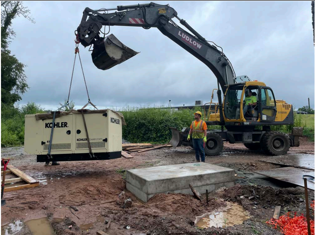
Picture 2: Ludlow lifting the booster station generator onto its concrete pad, which is located next to the station's southwest corner. View to the northwest.
