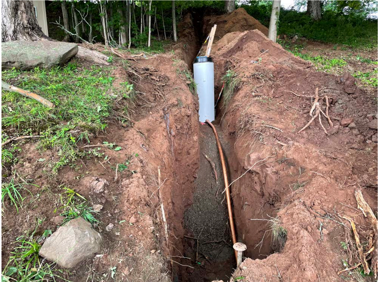
Picture 4: Meter pit with 2" copper pipe connecting it to the curb stop for the 95 Maple Avenue property. View to the east.
