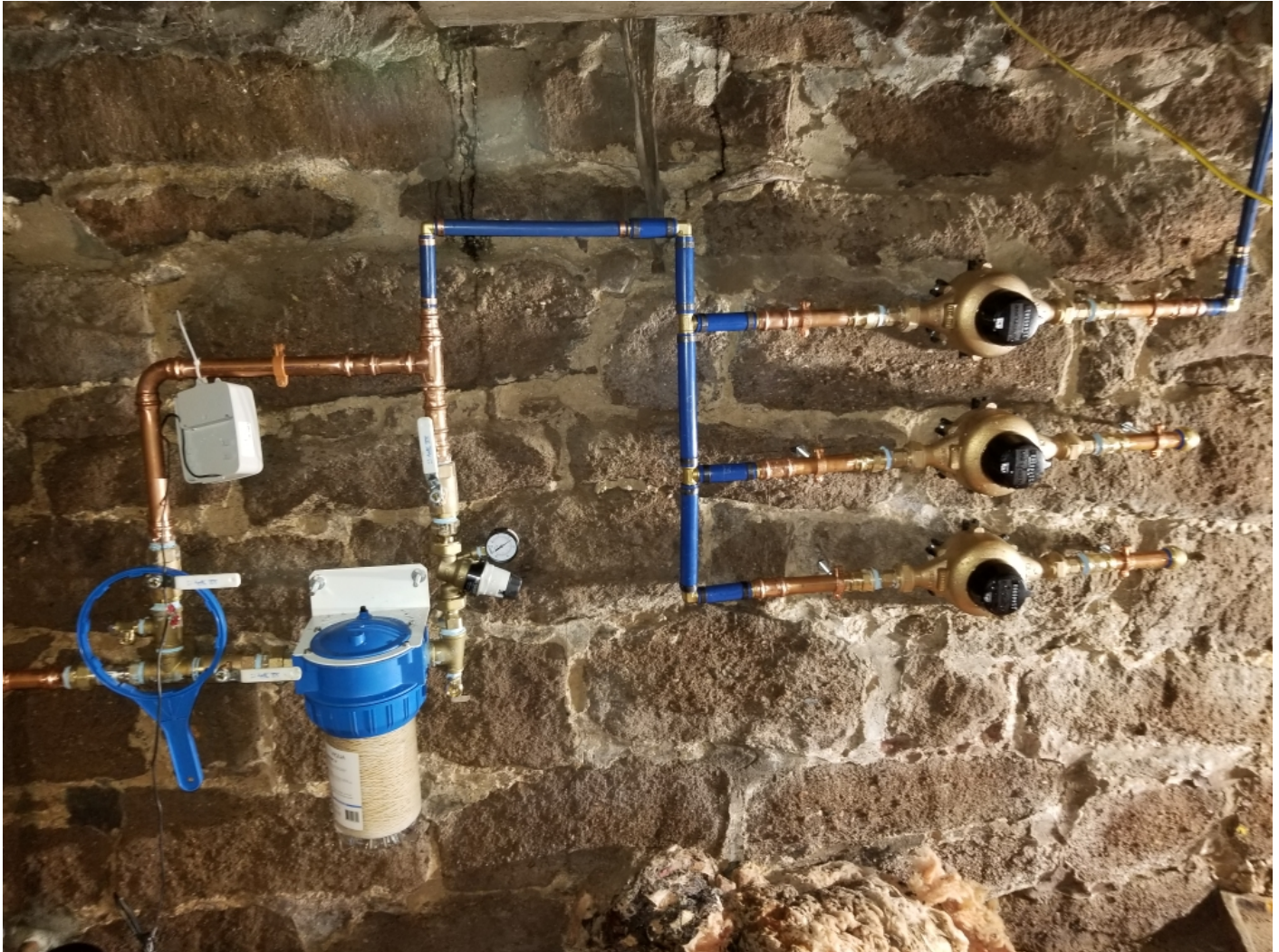
Picture 9: Sub-meters and final water service components installed at 235 Main Street residence.
