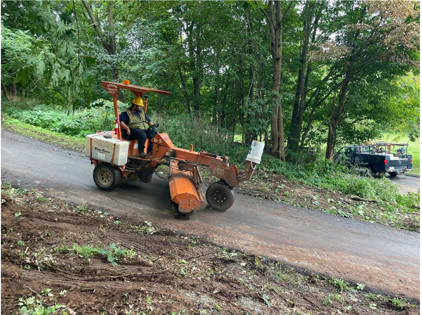
Picture 8: Ludlow using a Broce Broom to clean the driveway at 95 Maple Avenue. View to the south.
