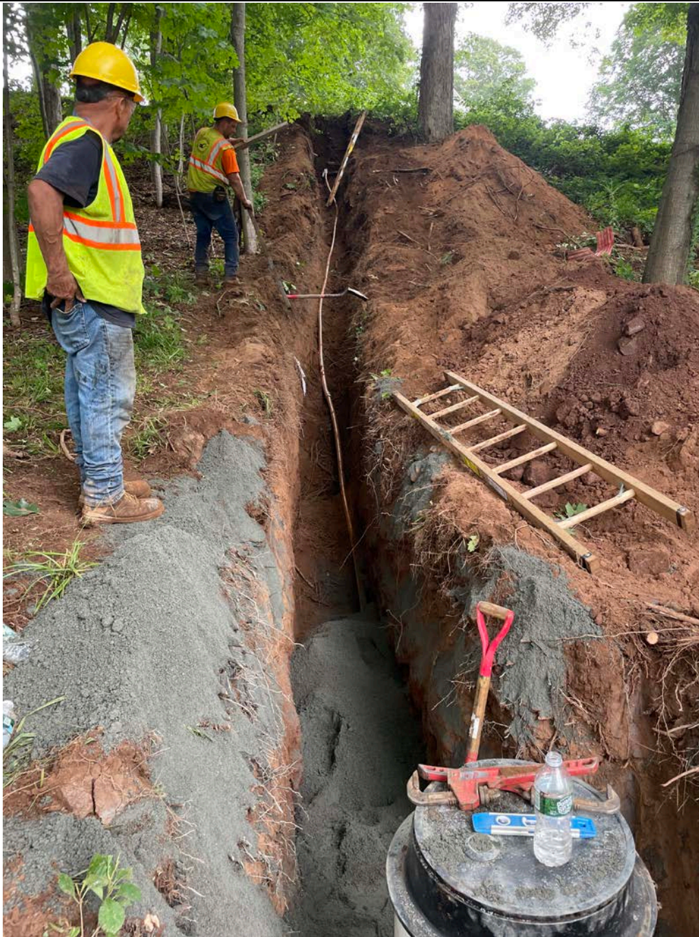
Picture 6: 2" copper water service pipe that Ludlow has connected to the meter pit at the 95 Maple Avenue property. View to the east.
