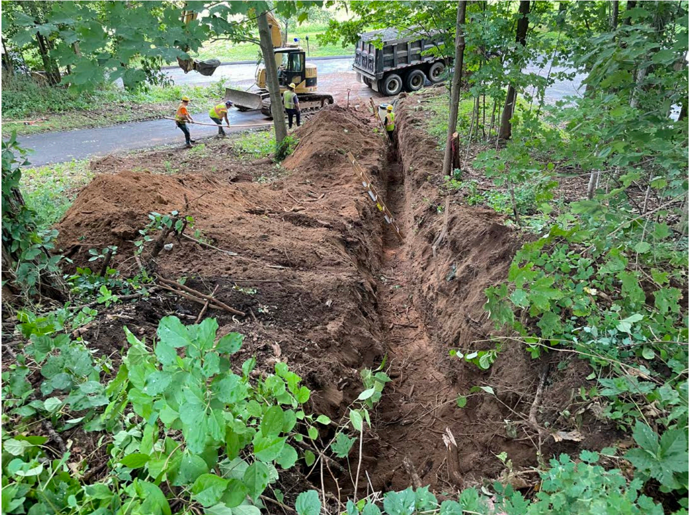
Picture 5: Trench that Ludlow has excavated at the 95 Maple Avenue property for the installation of a 2" copper water service line. View to the west.
