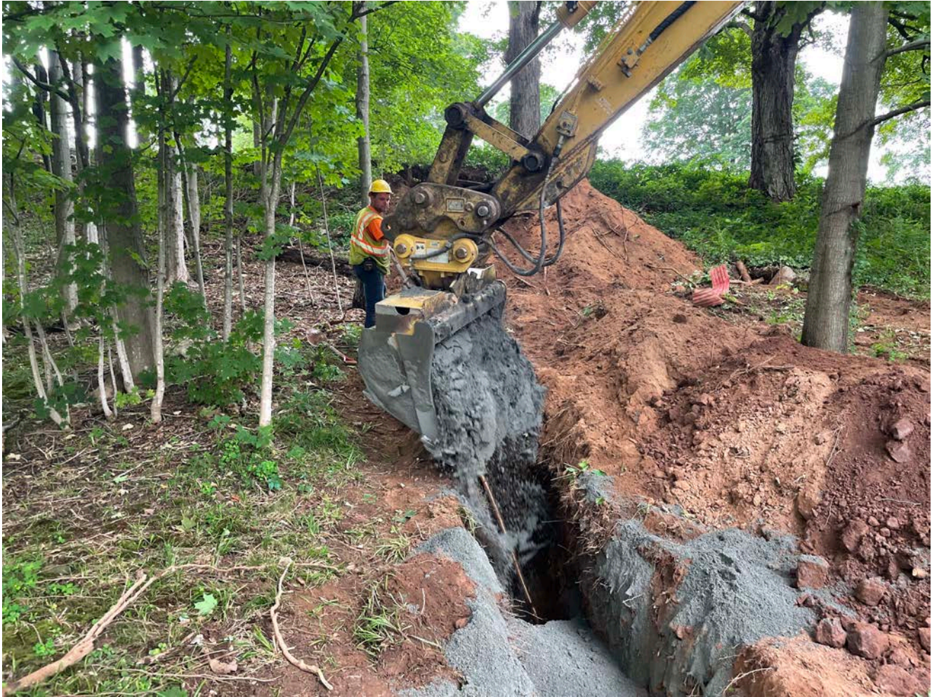
Picture 7: Ludlow placing sand over 2" copper water service line that they installed today at the 95 Maple Avenue, Durham, residence. View to east.
