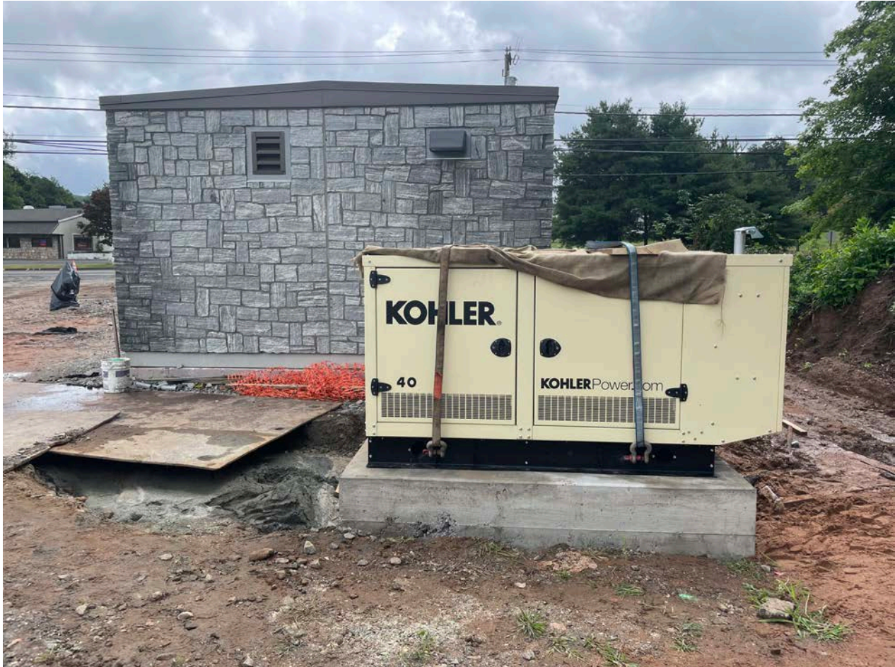
Picture 3: Generator situated on its concrete pad on the southwest corner of the booster station located at Station 750+63 in Middletown. View to the east.
