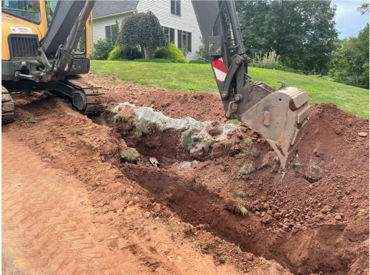
Picture 6: Ludlow excavating soil around a 4" PVC drain pipe they broke yesterday at the 97 Maple Avenue property as they prepare to repair the pipe. View to the southeast.
