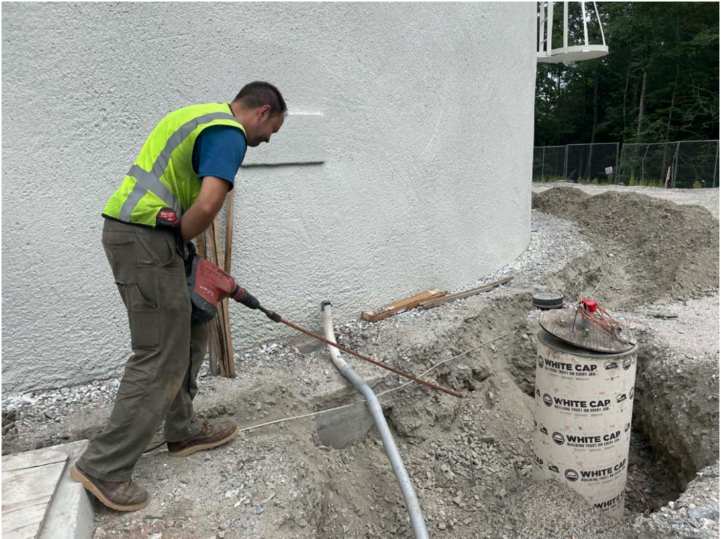
Picture 10: A&R Electrical installing a grounding rod on the west side of the water tank located east of the Shared Access Driveway. View to the southeast.
