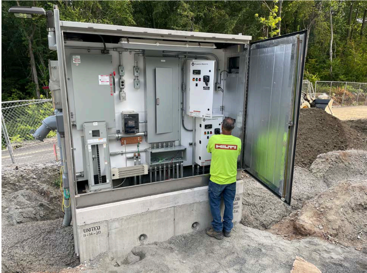
Picture 1: United Concrete working on the wiring located between the altitude valve vault and the electrical enclosure located north of the vault. View to the north.
