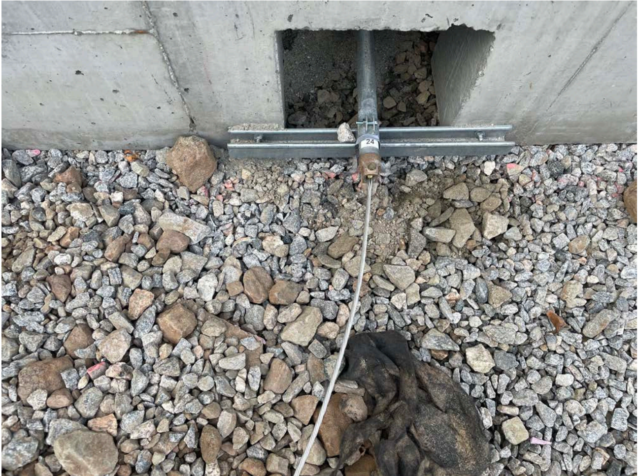
Picture 2: Ground wire attached to the north side of the electrical enclosure located at the water tank work zone in Middletown.
