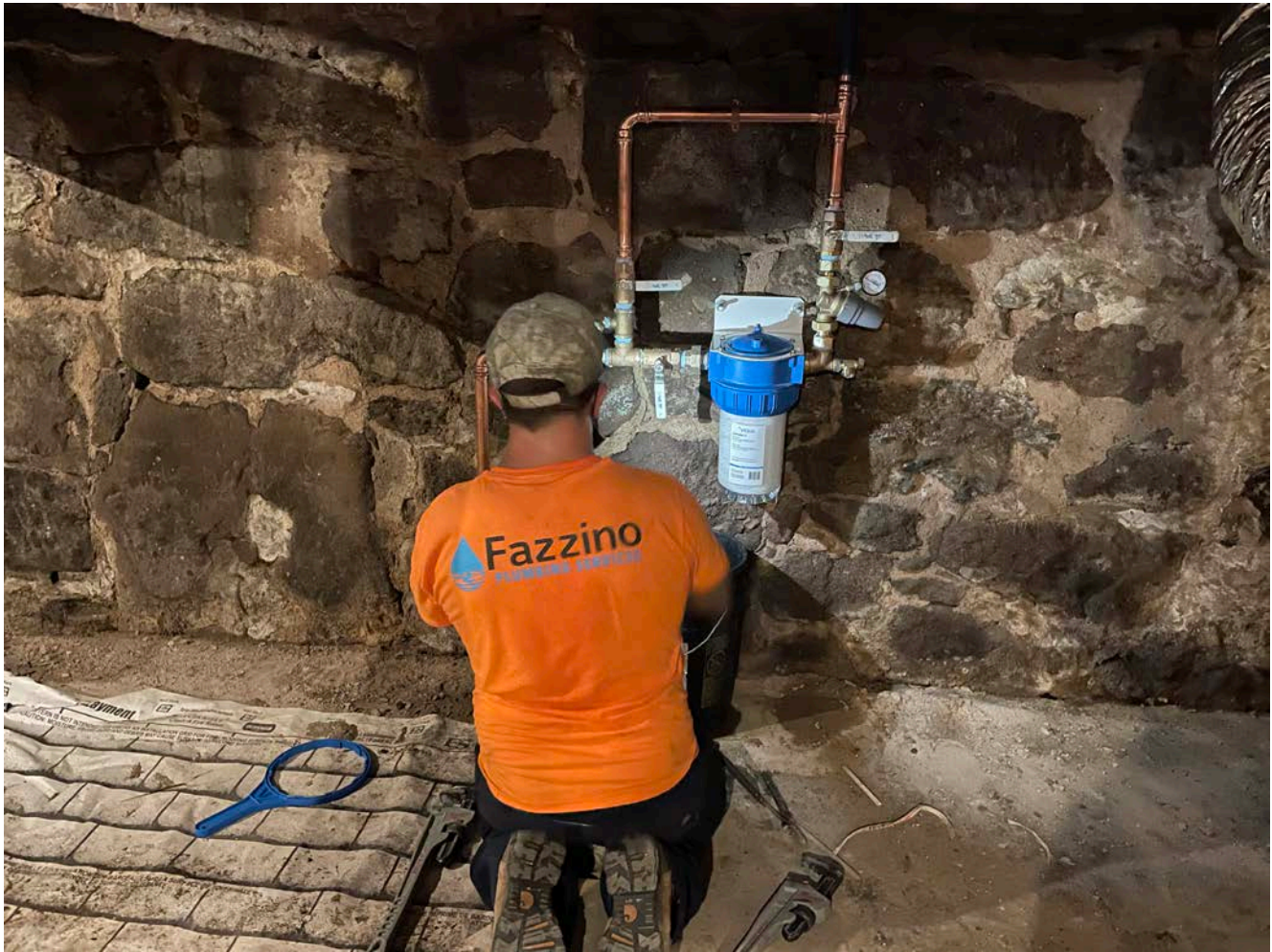
Picture 7: Fazzino Plumbing installing final water service components at the residence located at 293 Main Street, Durham. View to the west.
