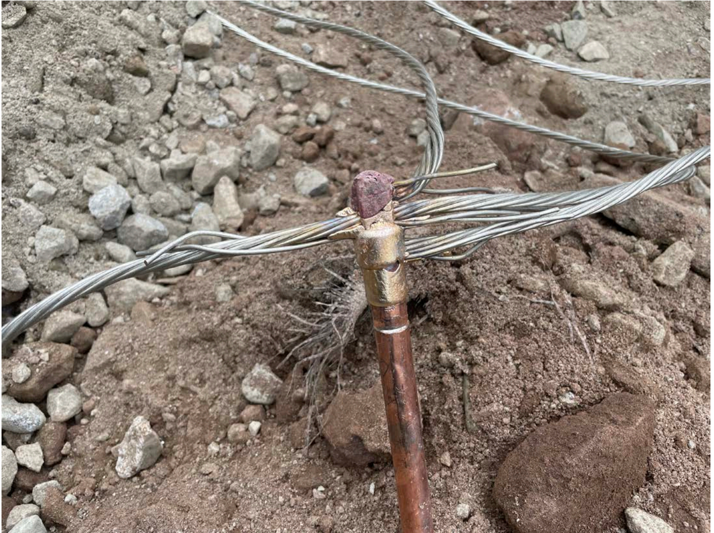
Picture 8: Ground wires welded to a grounding rod after A&R Electrical cad welded them together at the water tank work zone.
