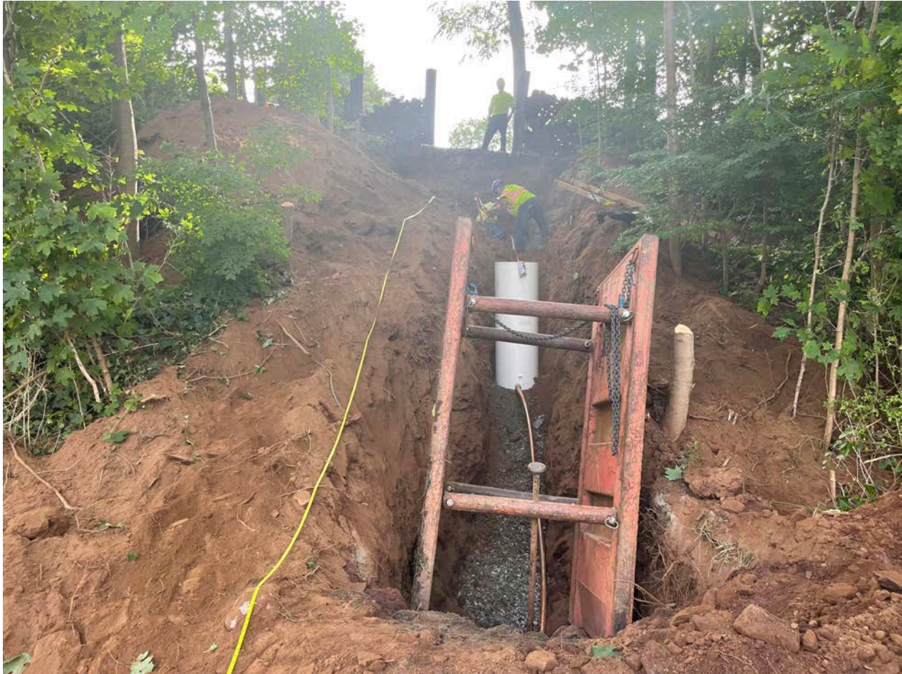
Picture 3: Ludlow installing 1.5" copper water service line from the meter pit eastwards to the driveway for the 97 Maple Avenue property. View to the east.
