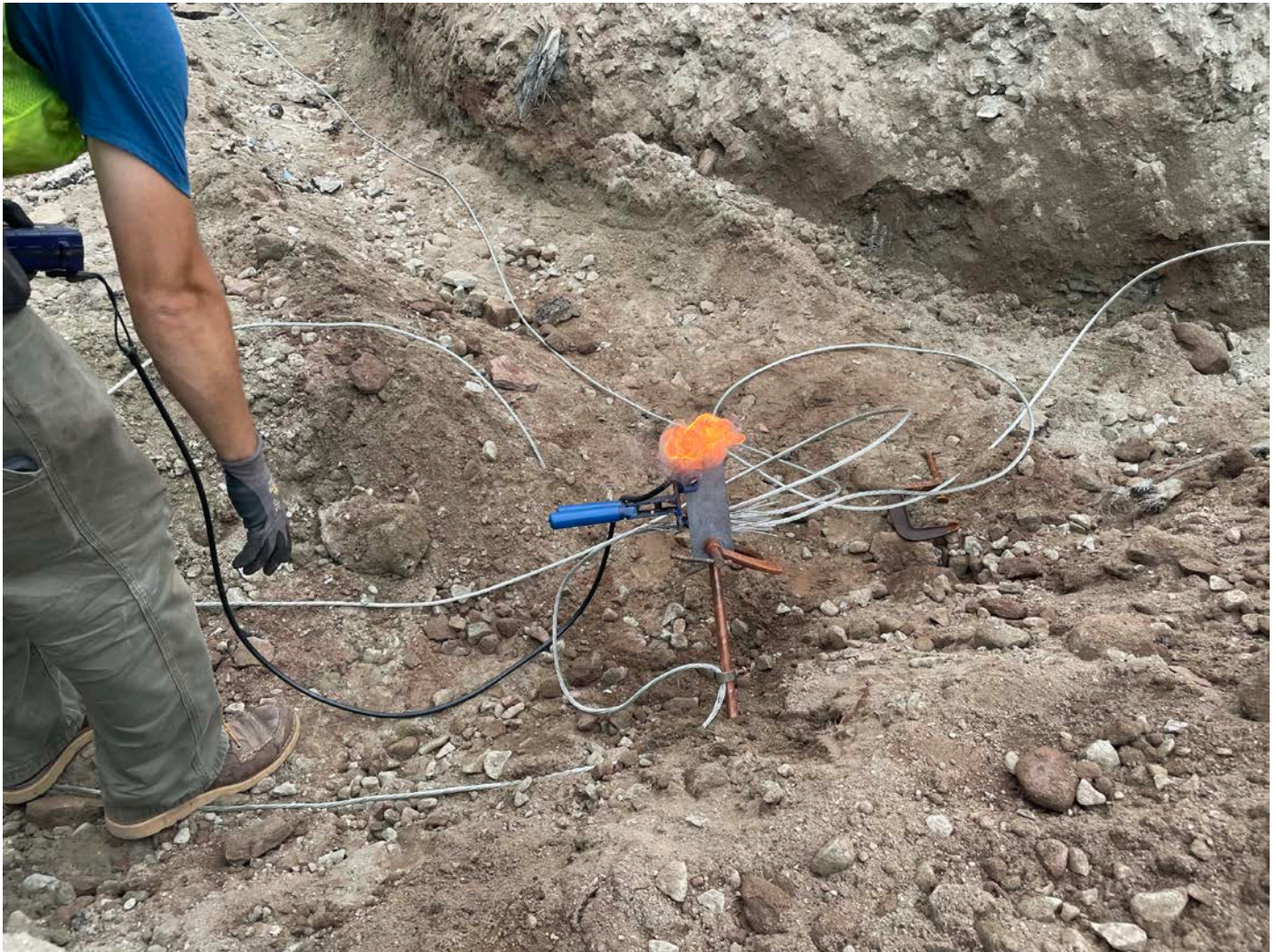
Picture 5: A&R Electrical cad welding ground wires to a grounding rod at the water tank work zone.
