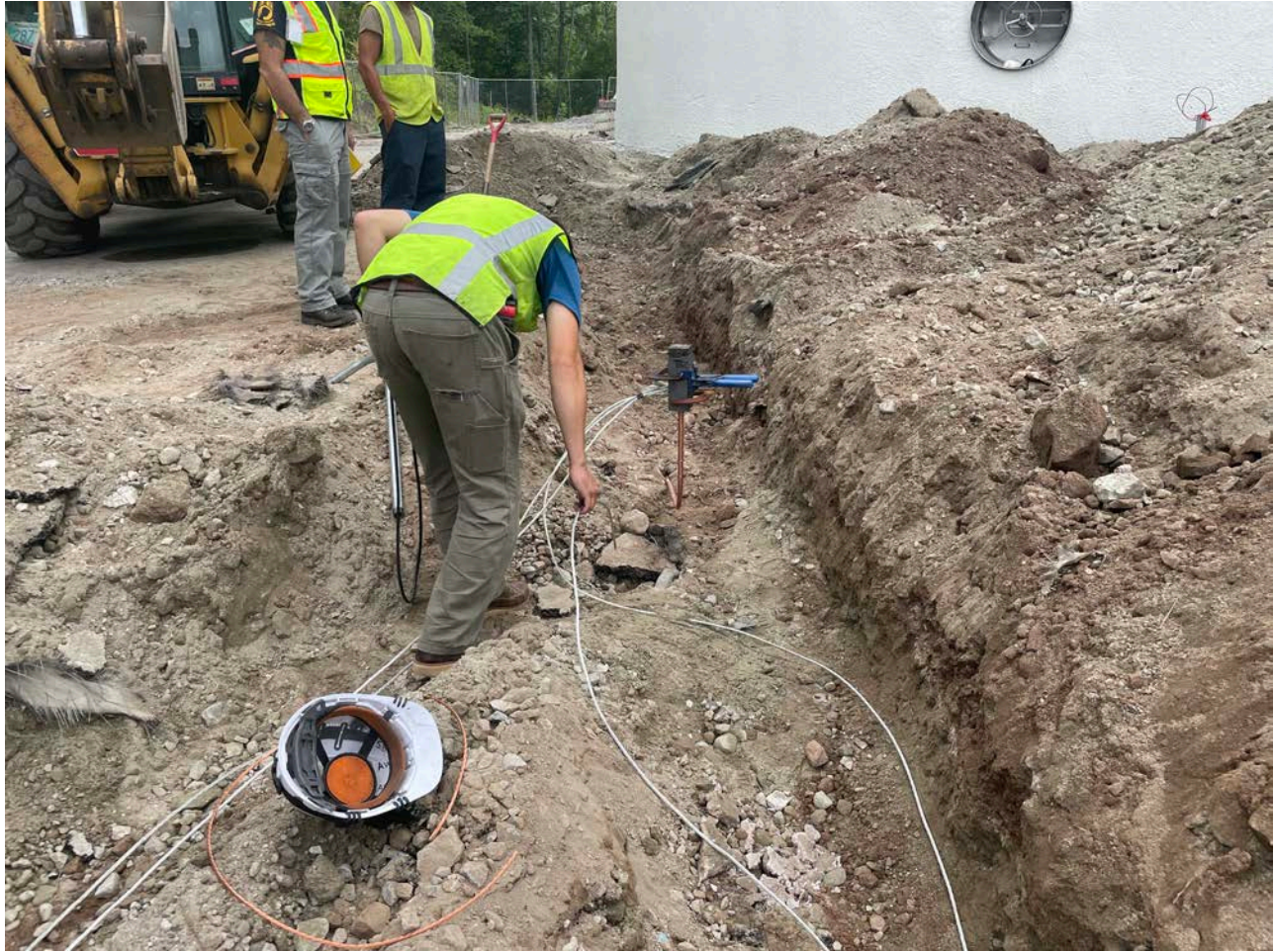
Picture 4: A&R Electrical setting up to connect ground wires to a grounding rod using cad welding. View to the east.
