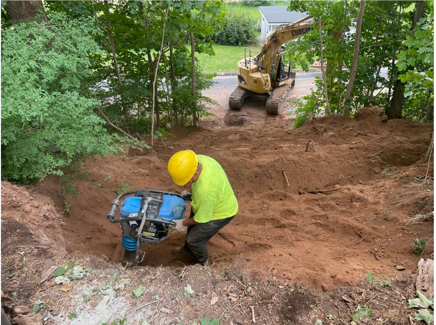
Picture 9: Ludlow compacting native backfill with a jumping jack at the 97 Maple Avenue property. View to the west.
