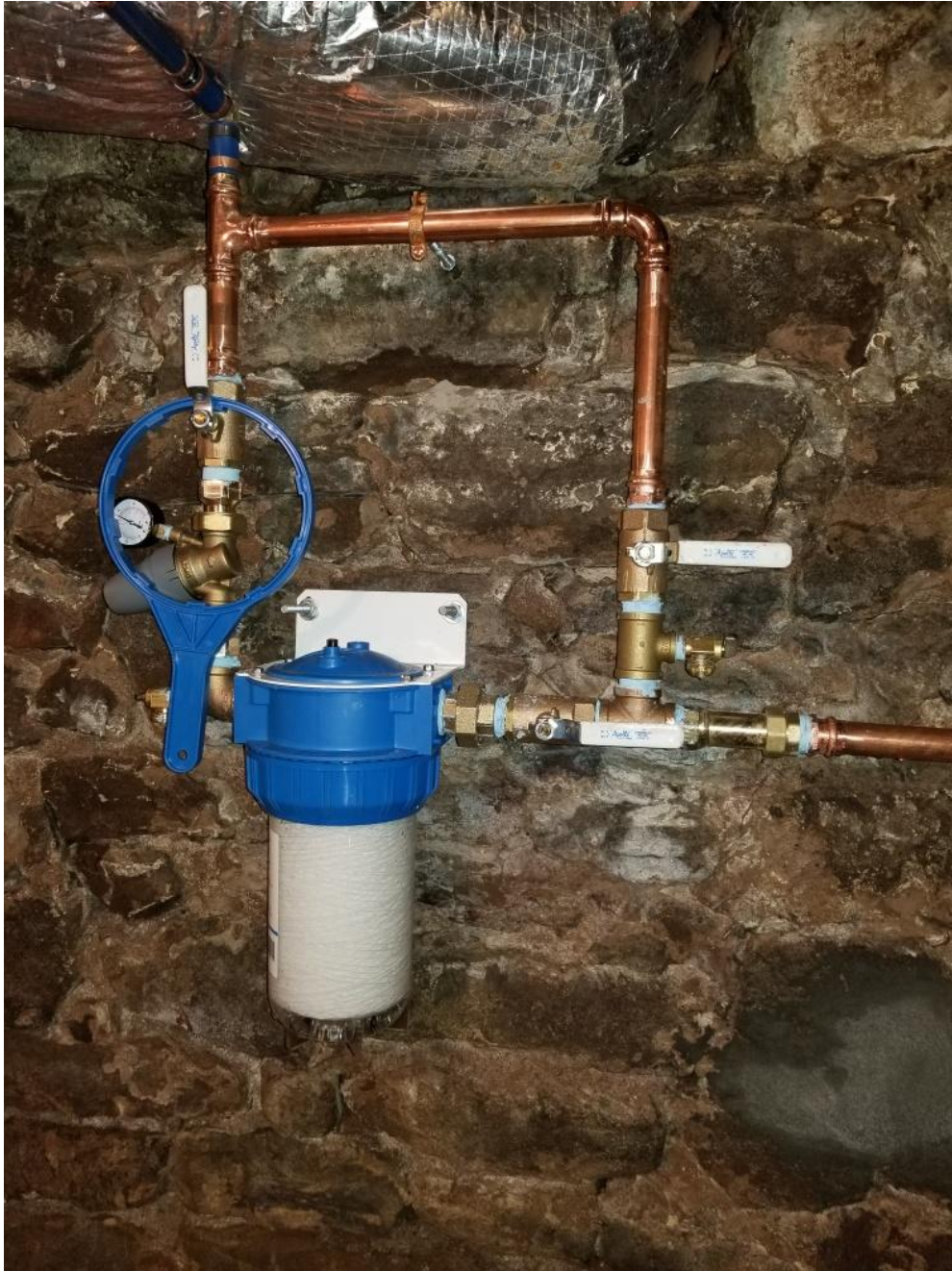
Picture 13: Final water service components that Fazzino Plumbing installed today at the residence located at 262 Main Street, Durham. View to the south.
