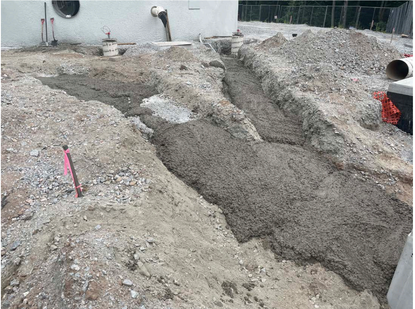
Picture 10: 4000 PSI concrete that was placed over a section of the utility duct bank on the west side of the water tank located east of the Shared Access Driveway in Middletown. View to the southeast.
