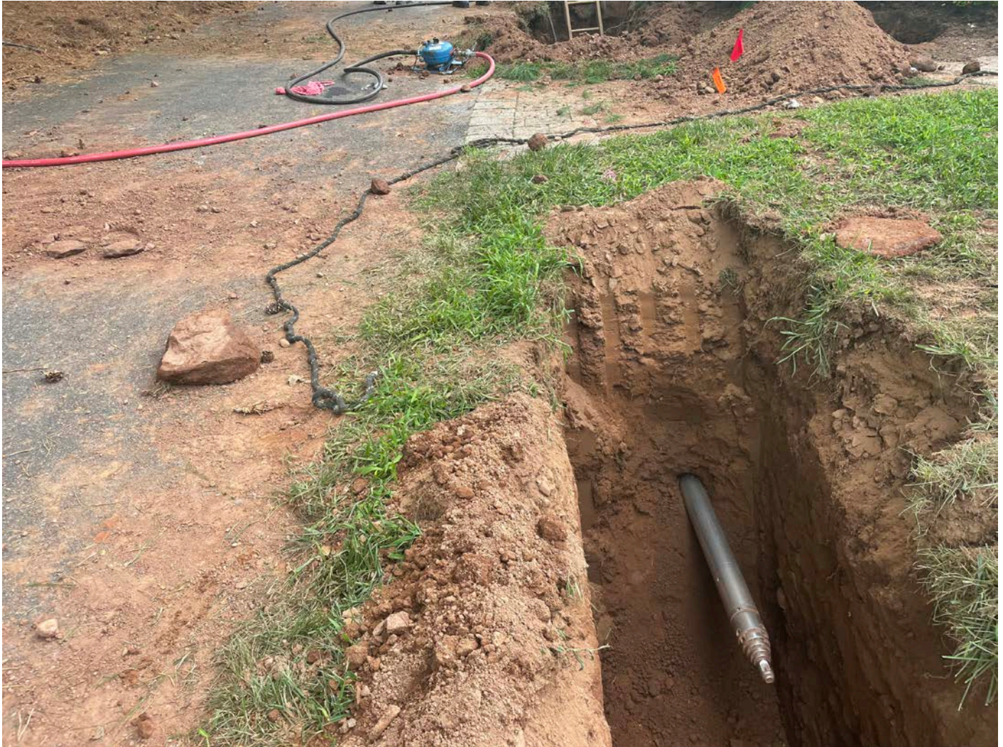
Picture 5: Ludlow using a pneumatic mole to create a hole beneath a brick walkway for the placement of 1.5” copper line. View to the east.
