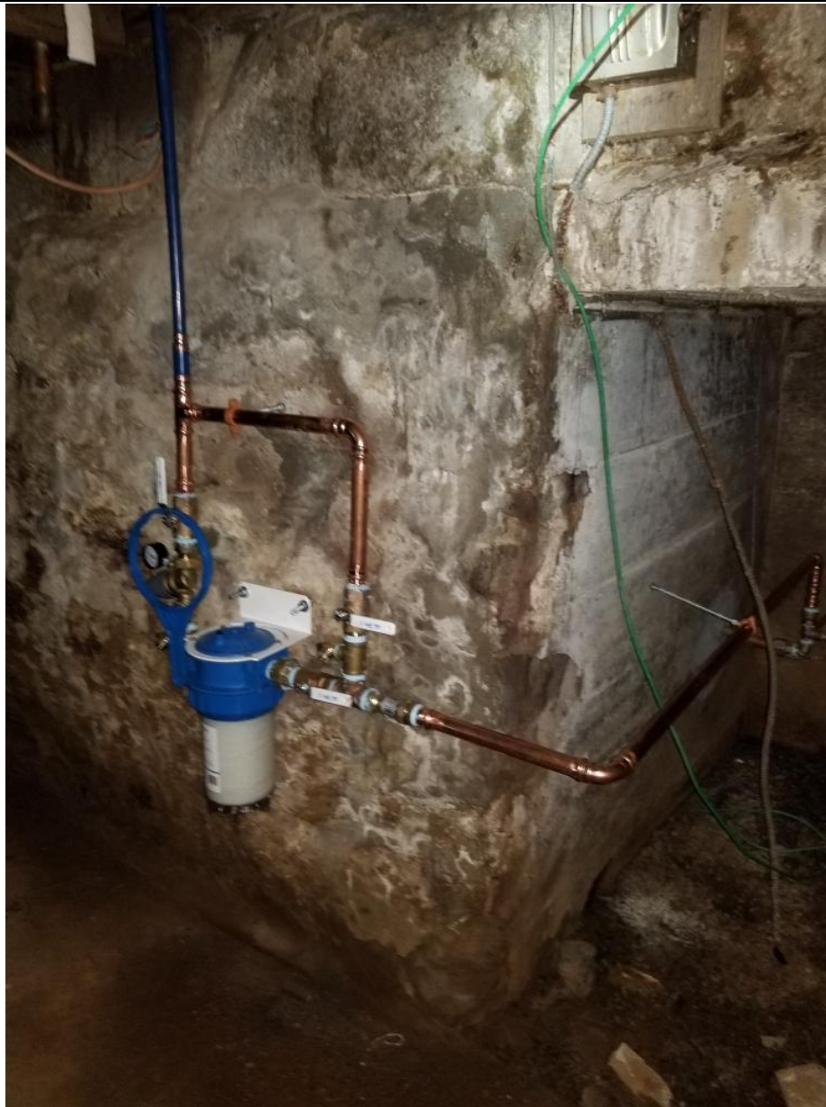
Picture 12: Final water service components that Fazzino Plumbing installed today at the residence located at 252 Main Street, Durham. View to the south.
