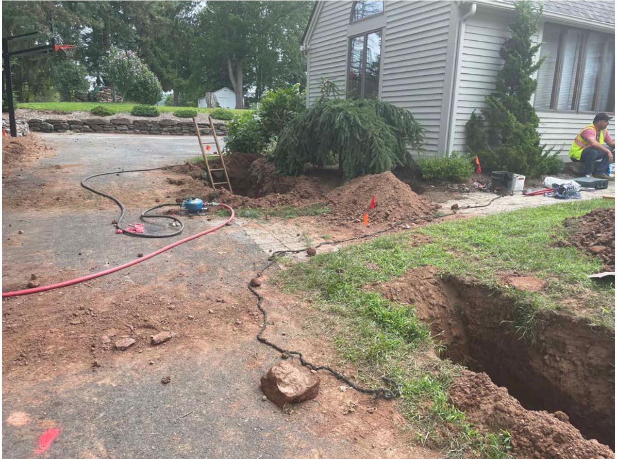
Picture 3: View of the excavation that Ludlow has made at the 97 Maple Avenue property for the installation of a 1.5" copper water service line. Ludlow used a pneumatic mole to punch a hole under the brick sidewalk for the copper pipe to be placed. View to the southeast.
