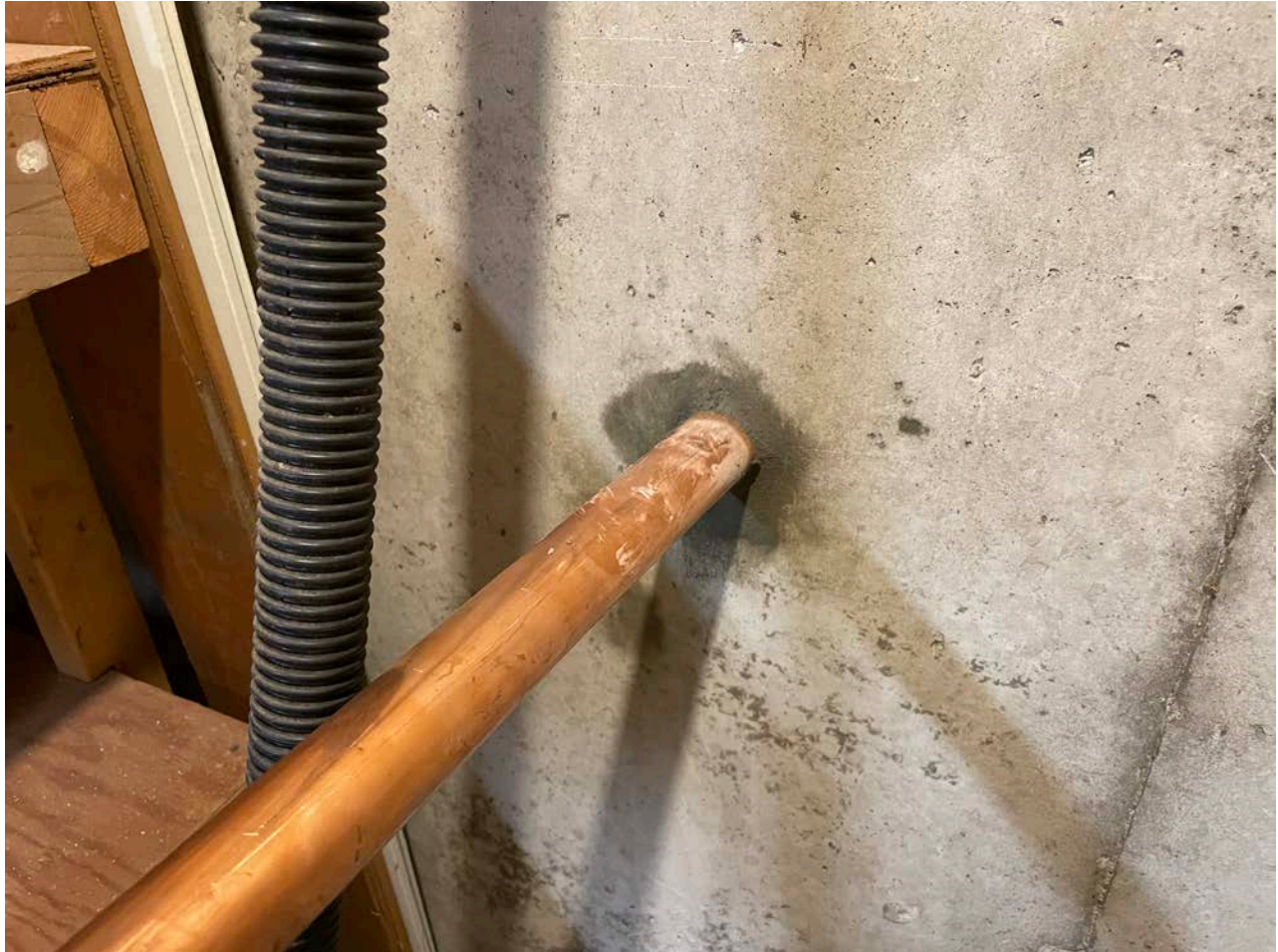
Picture 6: 1.5" copper pipe that was inserted through the northern foundation of the 97 Maple Avenue residence and secured in place with non-shrink grout. View to the northwest.
