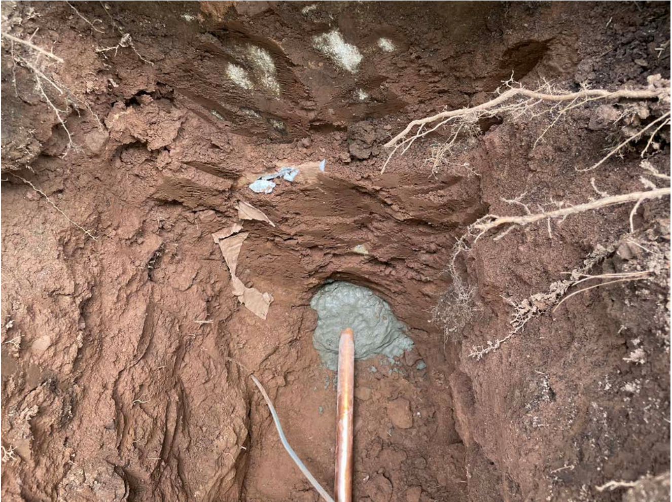
Picture 7: 1.5" copper pipe that was inserted through the northern foundation of the 97 Maple Avenue residence and secured in place with non-shrink grout. View to the south.
