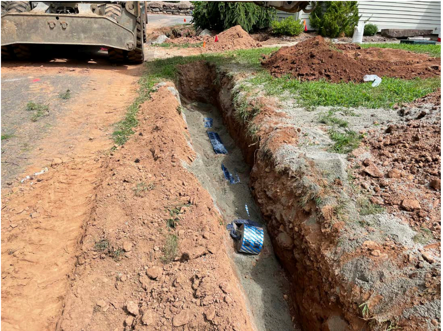
Picture 8: Ludlow in the process of placing sand followed by caution tape over installed 1.5" copper water service line at the 97 Maple Avenue property. View to the east.
