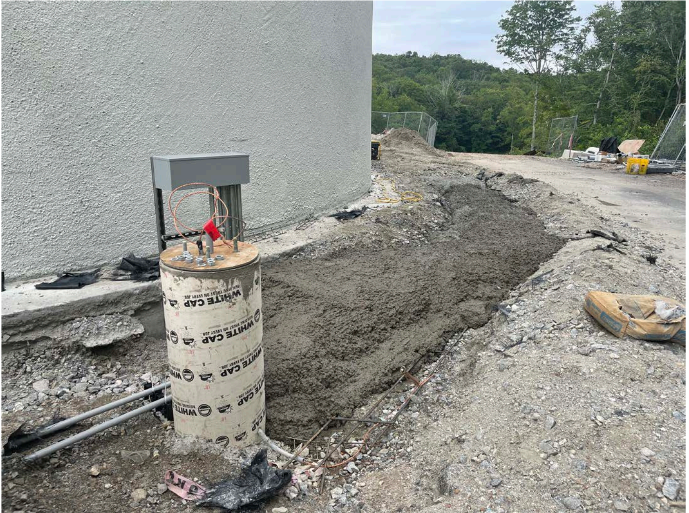
Picture 9: 4000 PSI concrete that was placed over a section of the utility duct bank on the north side of the water tank located east of the Shared Access Driveway in Middletown. View to the west.
