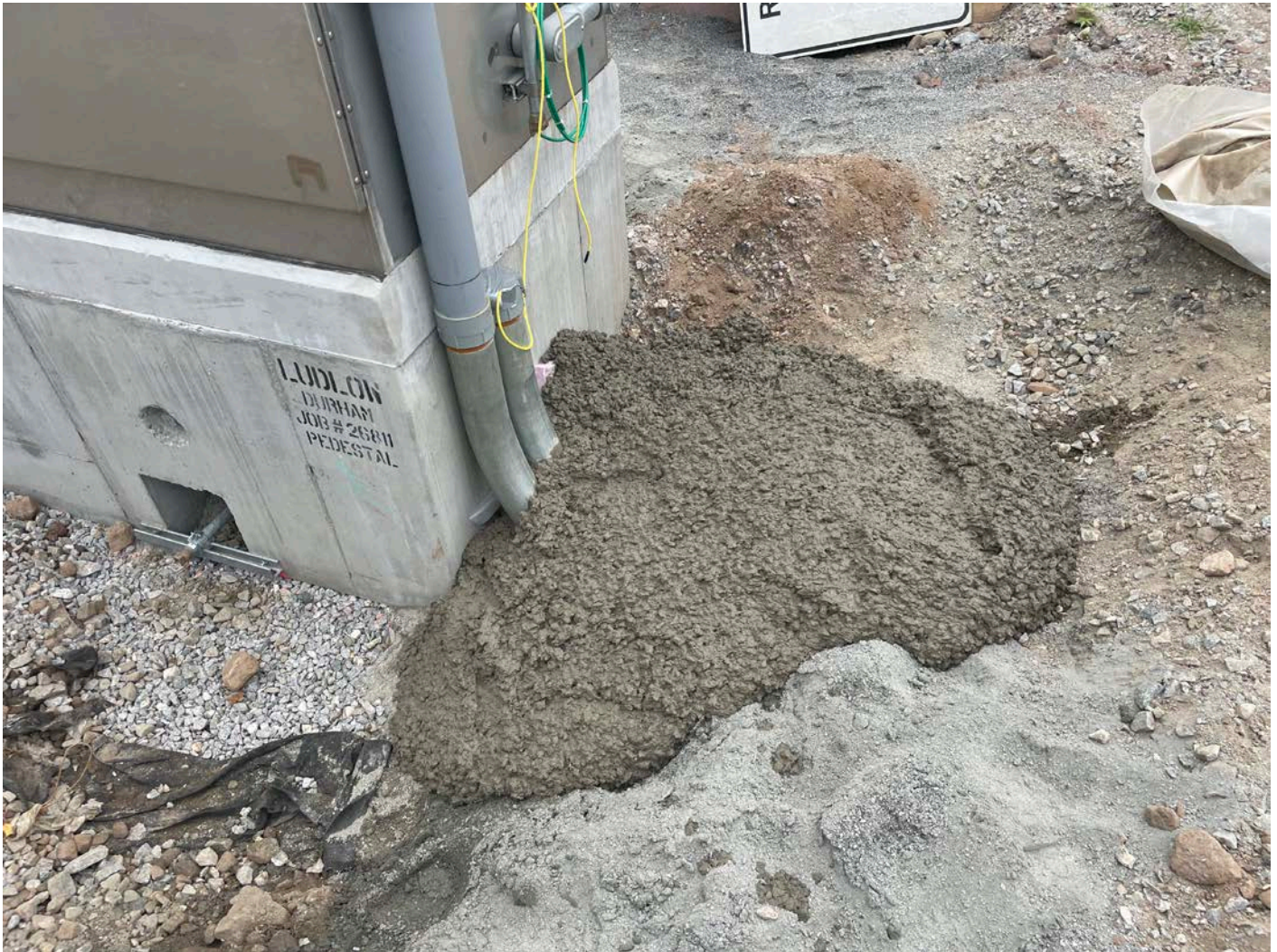
Picture 11: 4000 PSI concrete that was placed over a section of the utility conduits on the west side of the electrical enclosure located north of the altitude valve vault at the water tank work zone in Middletown. View to the southeast.
