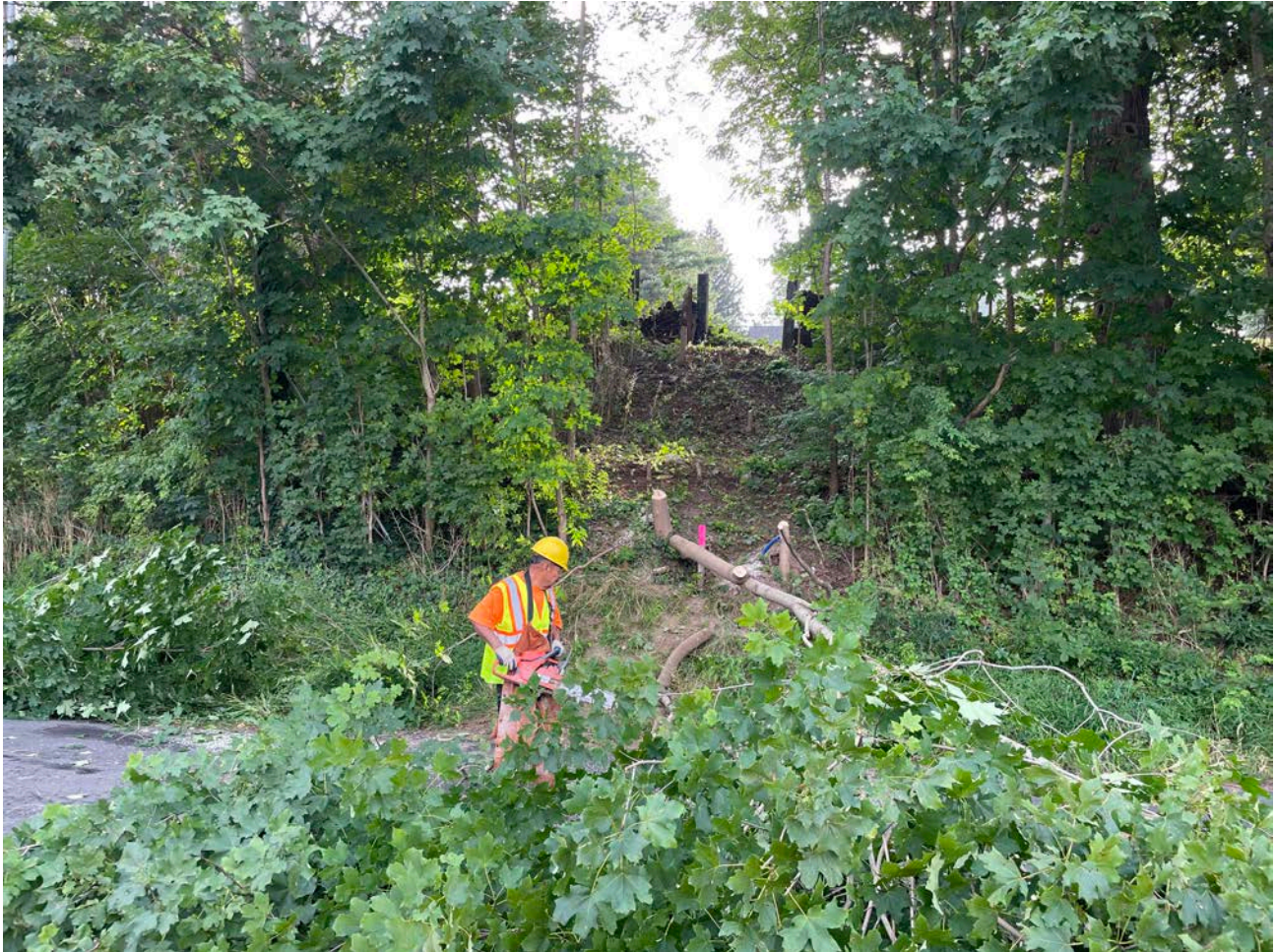
Picture 2: Ludlow removing trees at the 97 Maple Avenue property to install a 1.5" copper water service line to the residence. View to the east.
