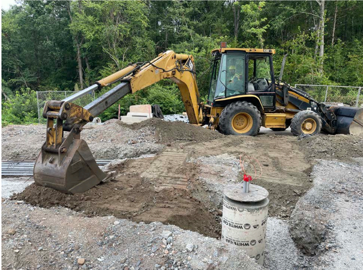
Picture 1: Ludlow backfilling over portions of the utility duct banks located west and north of the water tank located east of the Shared Access Driveway in Middletown. View to the north.
