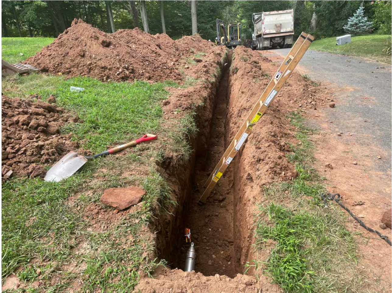
Picture 4: Ludlow excavating on the 97 Maple Avenue property. Note pneumatic mole in trench. View to the west.
