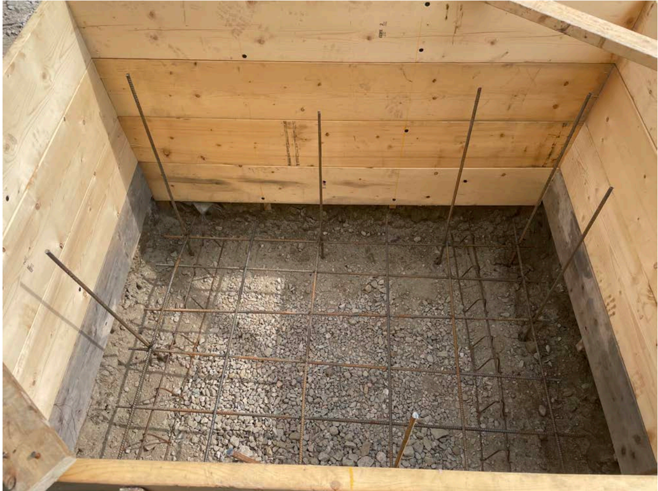
Picture 4: Rebar that Ludlow is placing inside of the concrete form for the blower enclosure pad on the northeast side of the water tank.
