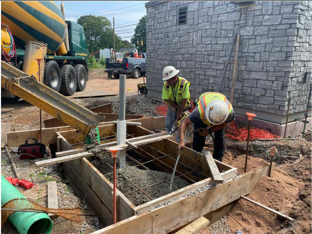
Picture 7: Ludlow vibrating concrete as it is being placed in the concrete form for the generator pad located on the southwest corner of the booster station. View to the northeast.
