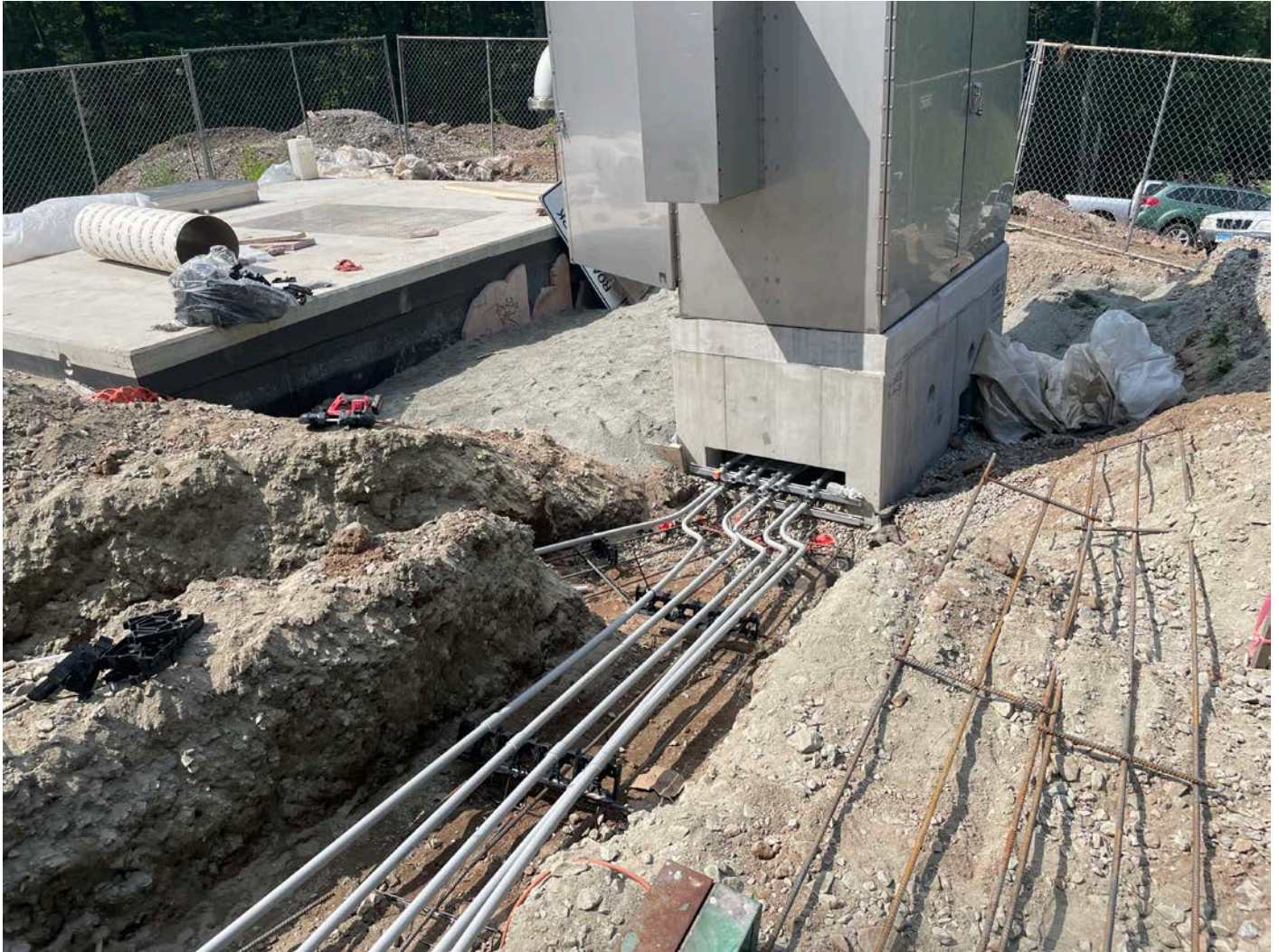
Picture 5: 1" Schedule 40 PVC conduit that A&R Electrical installed coming off the east side of the electrical enclosure located on the north side of the altitude vault. View to the east.
