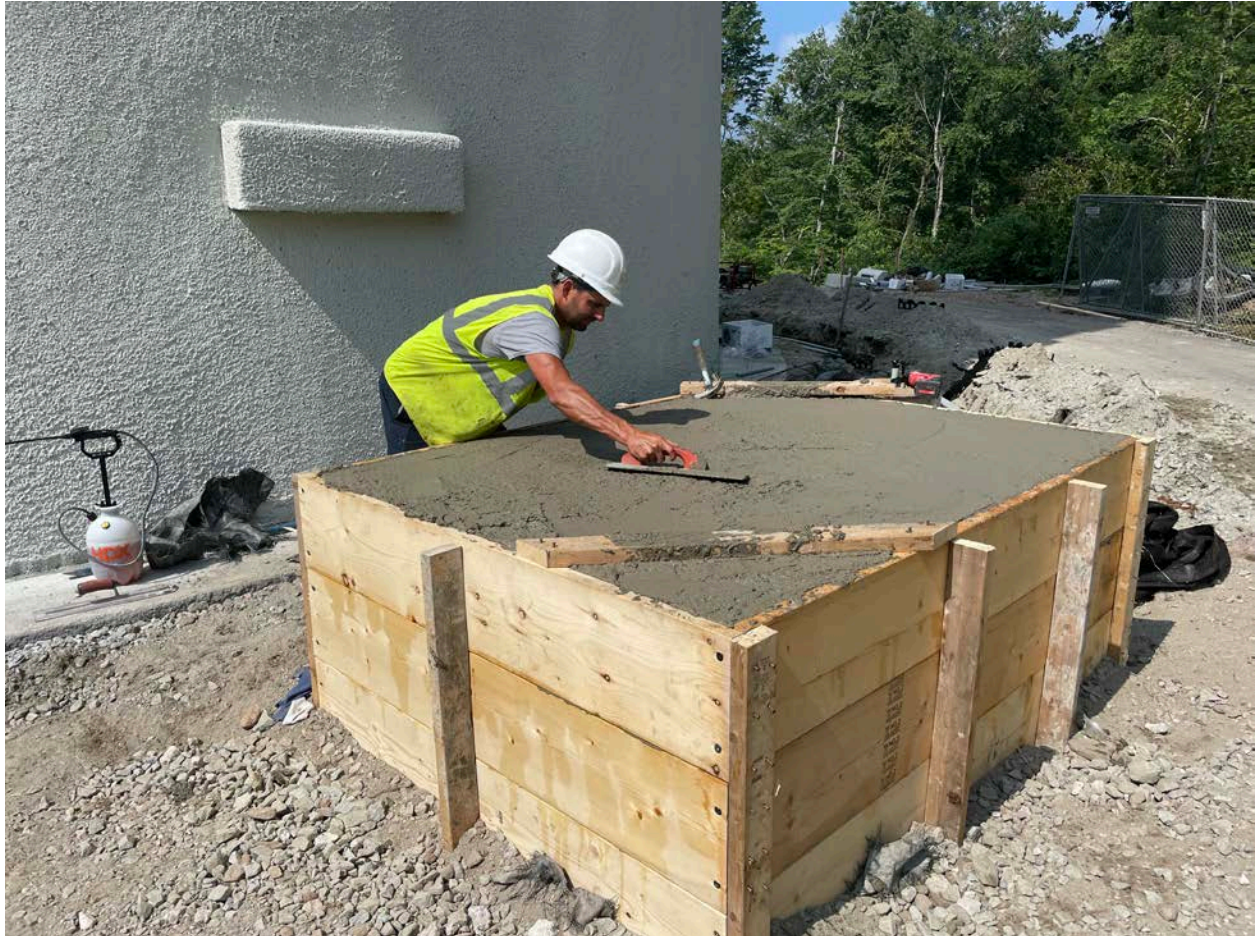
Picture 6: Ludlow troweling the concrete that was just poured into the concrete form for the blower enclosure pad located on the northeast side of the water tank located east of the Shared Access Driveway. View to the west.
