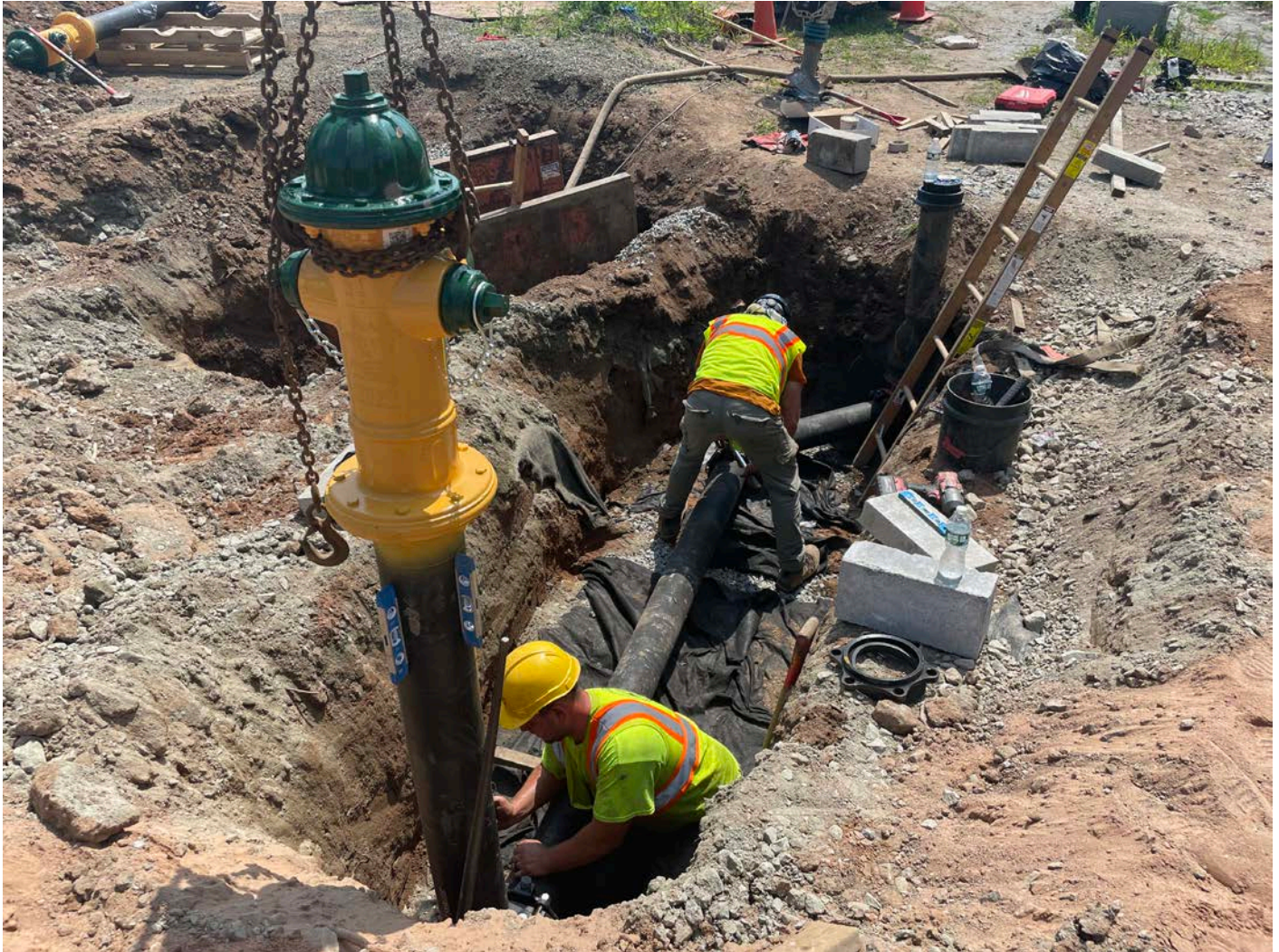
Picture 8: Ludlow installing one of two hydrants that they installed today near the northeast corner of the booster station. View to the south.
