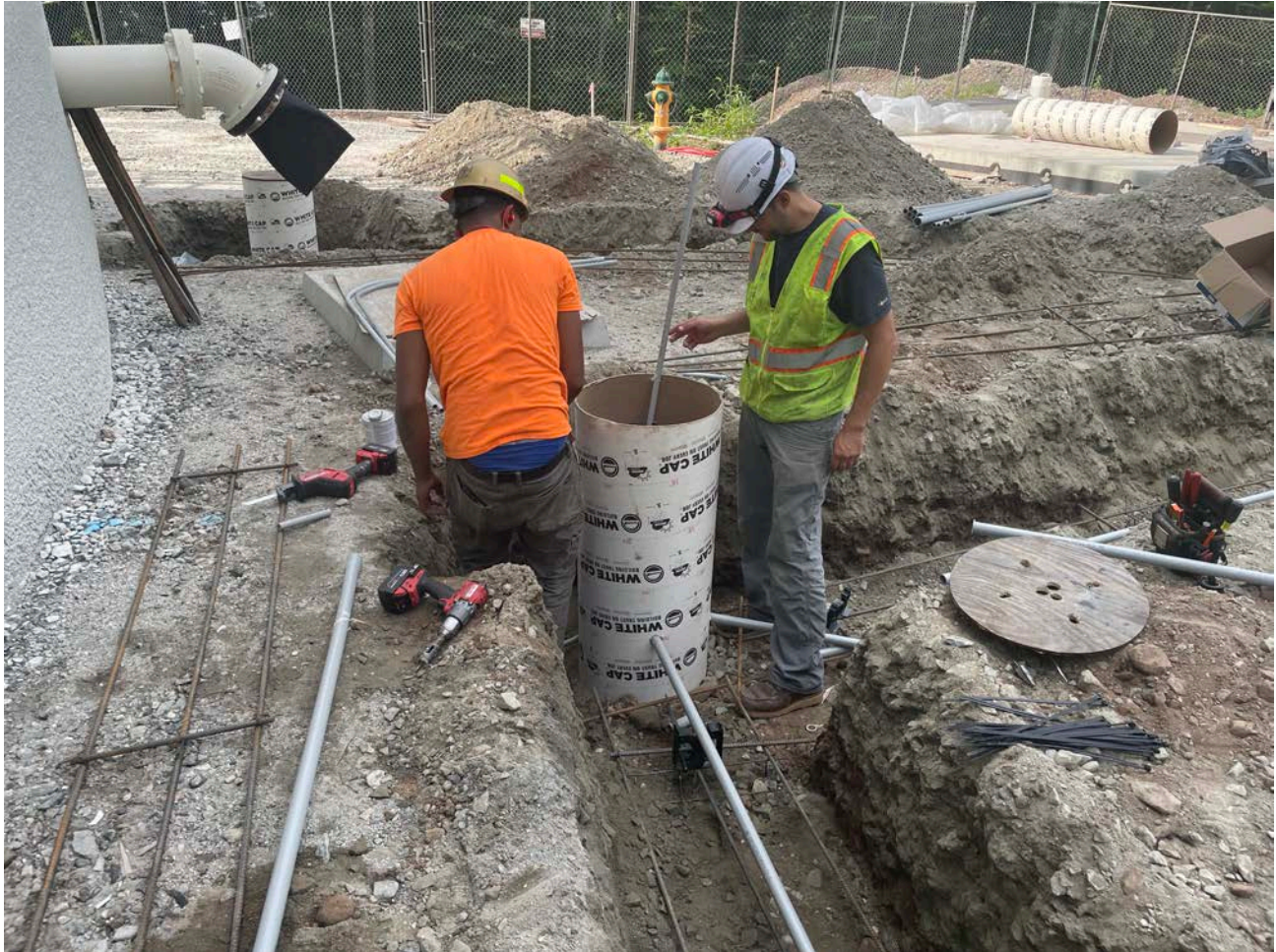
Picture 2: A&R Electrical installing 1" schedule 40 PVC conduits for the light pole standards on the west side of the water tank located east of the Shared Access Driveway in Middletown. View to the south.
