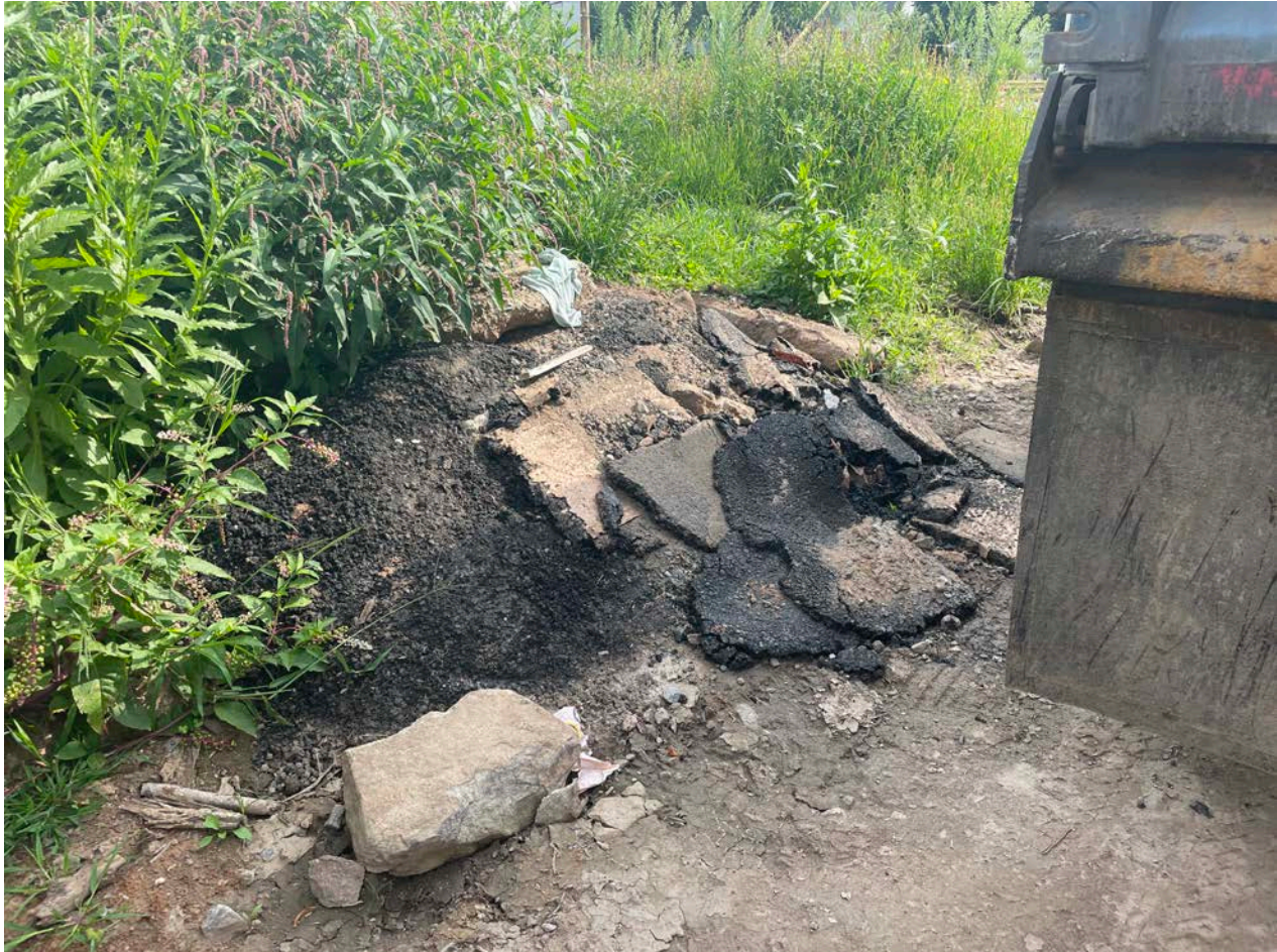
Picture 3: Waste asphalt that was recently placed at the booster station work zone. Ludlow confirmed that this material was not placed by them. View to the northeast.
