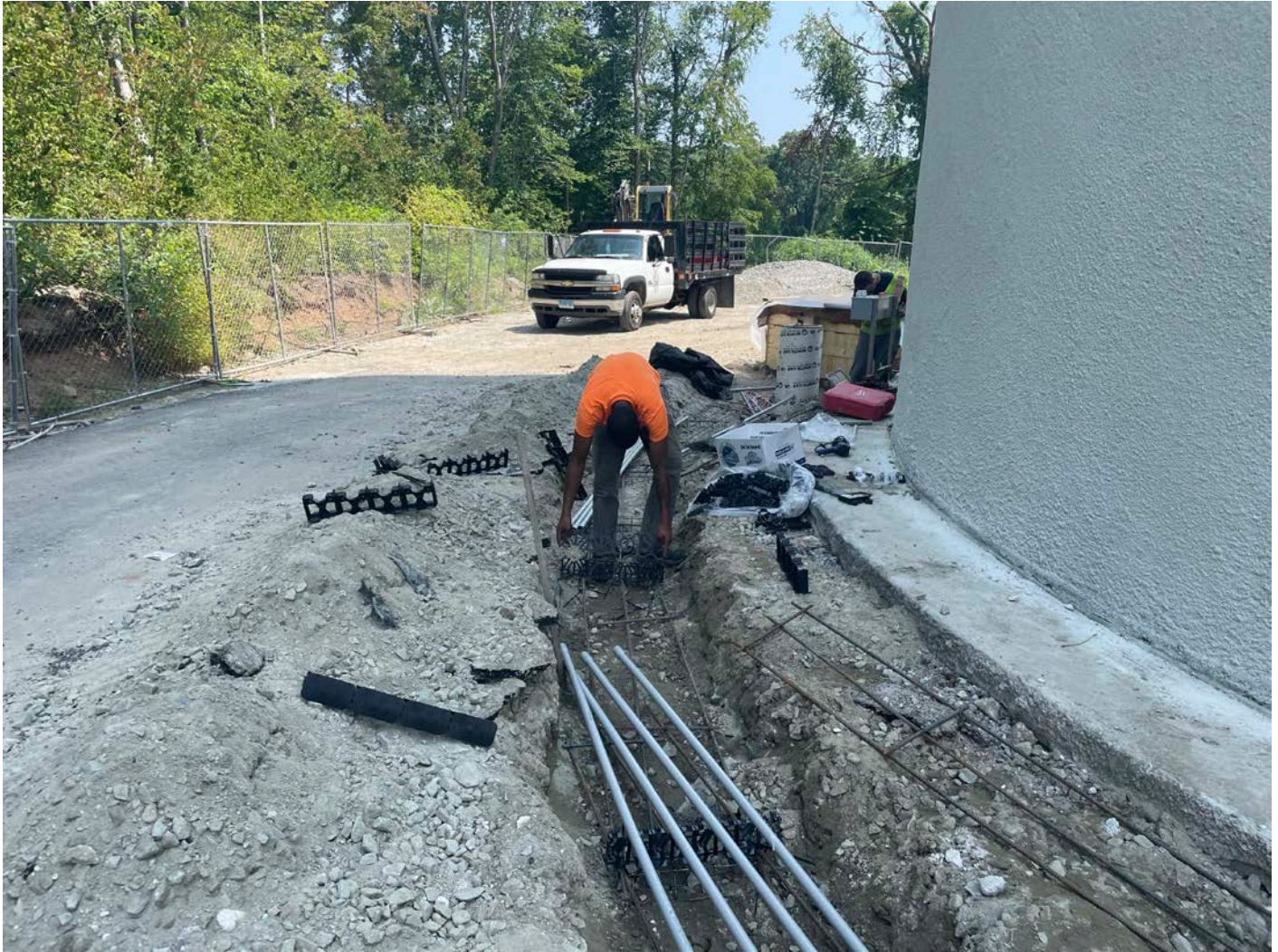
Picture 9: A&R Electrical placing 3” plastic chairs in the utility duct bank trench located on the north side of the water tank. View to east.
