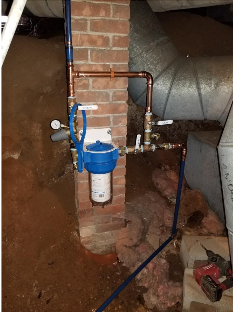
Picture 6: Final water service components installed at the church located at 236 Main Street, Durham.
