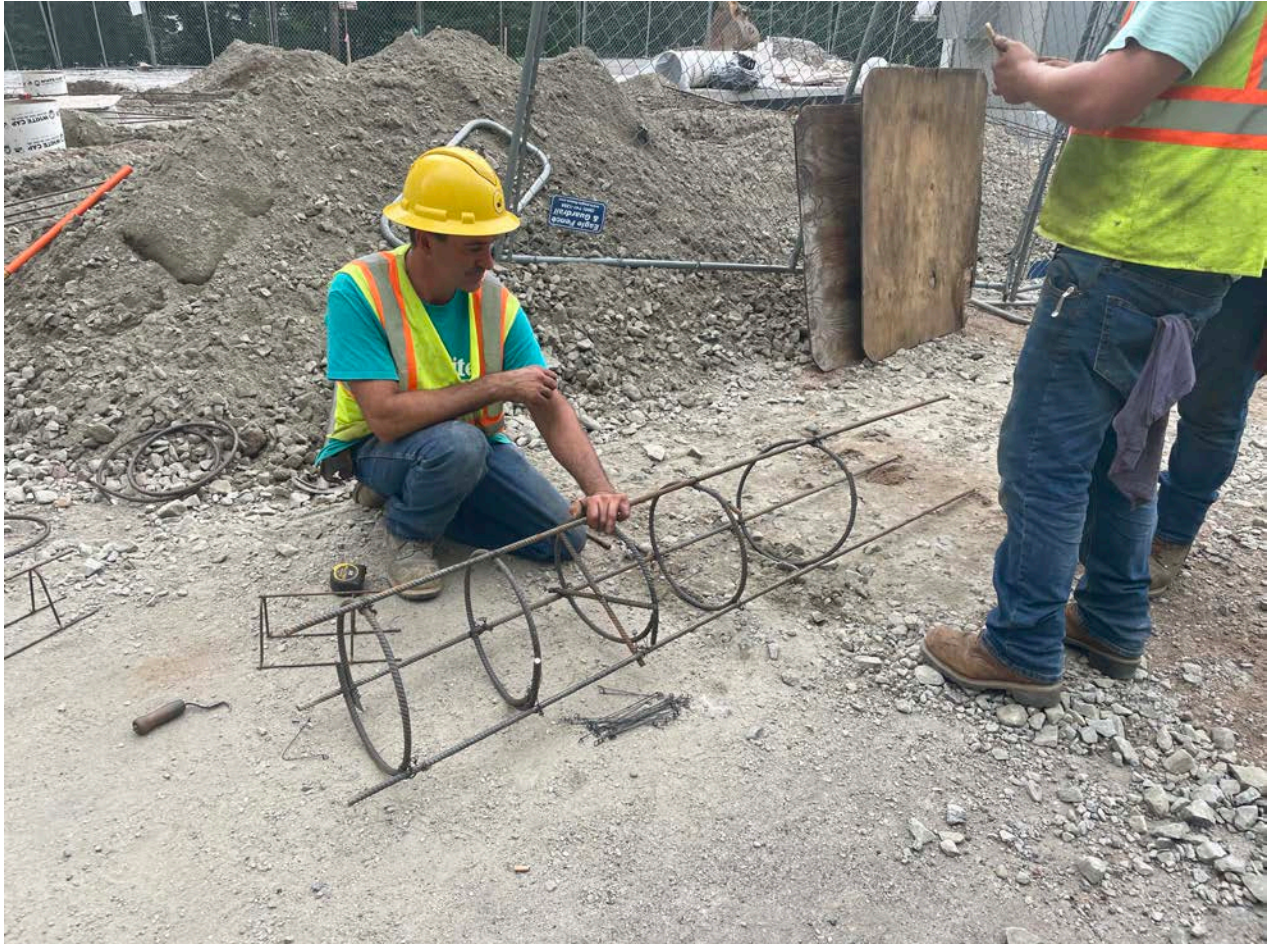
Picture 3: Ludlow securing sections of rebar together for placement in sonotubes for light pole bases at the water tank work zone located east of the Shared Access Driveway in Middletown.
