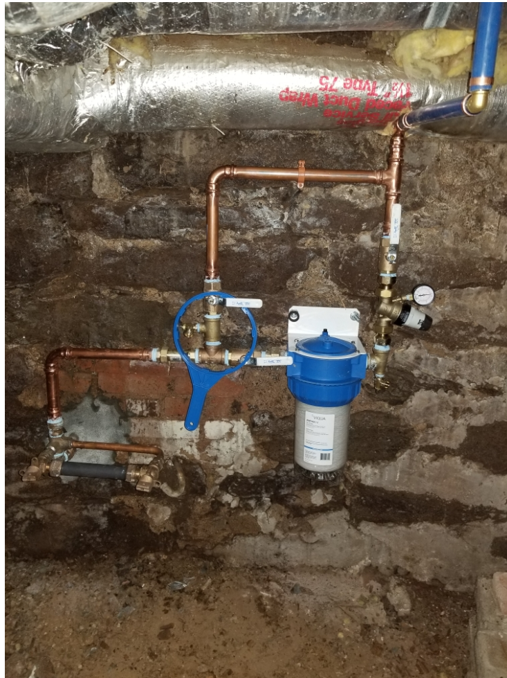
Picture 7: Final water service components installed at the residence located at 256 Main Street, Durham.
