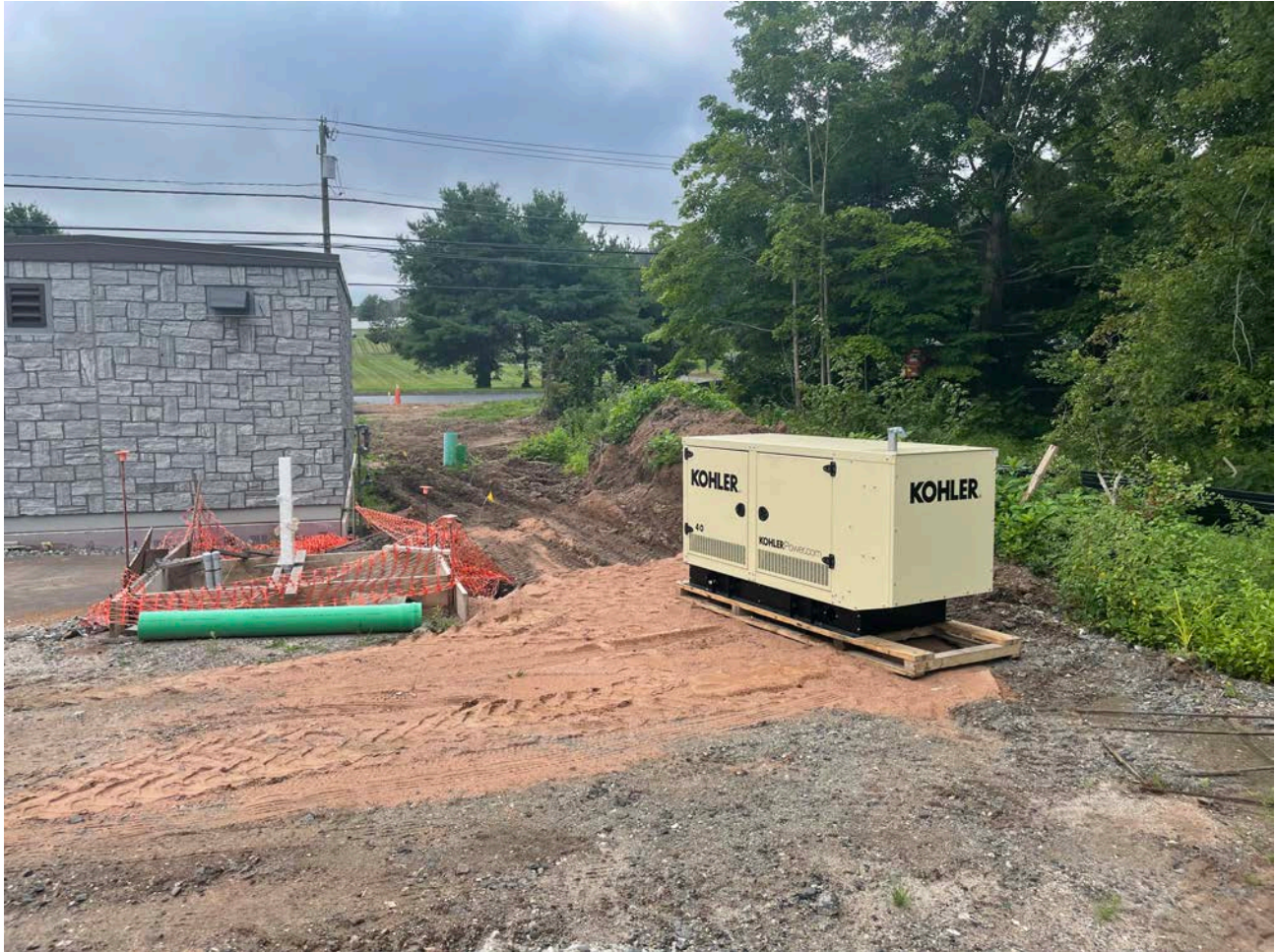
Picture 2: Generator that Ludlow staged on the west side of the booster station located at Station 750+63 in Middletown. View to the east.
