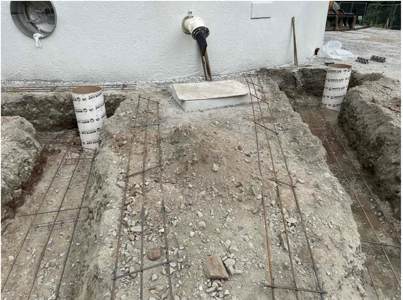
Picture 5: View of utility duct trenches, associated rebar, and sonotubes located on the west side of the water tank located to the east of the Shared Access Driveway in Middletown. View to the east.
