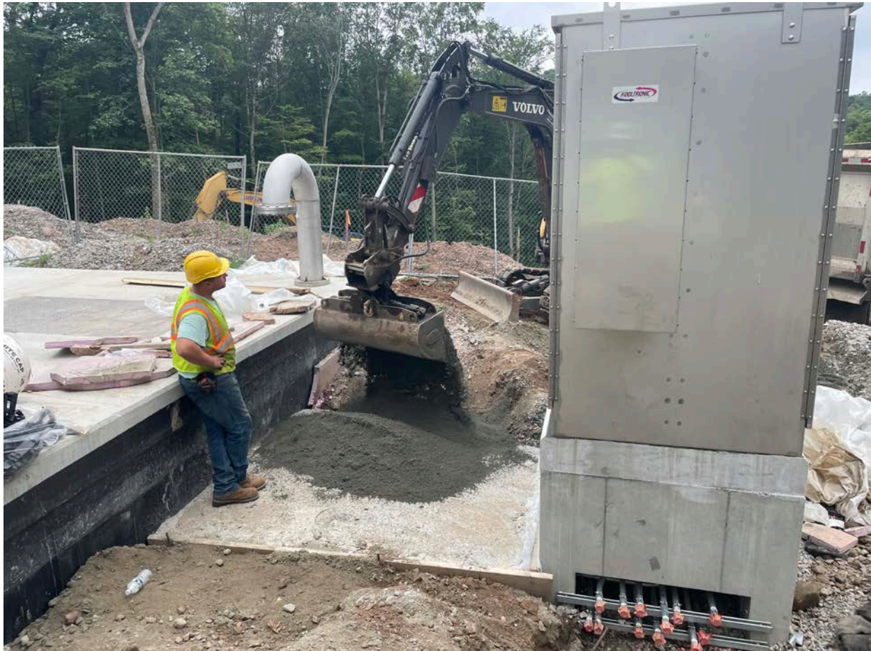
Picture 1: Ludlow placing sand over the concrete-encased utility conduits located between the altitude valve vault and the electrical cabinet located several feet to the north of the vault. View to the west.
