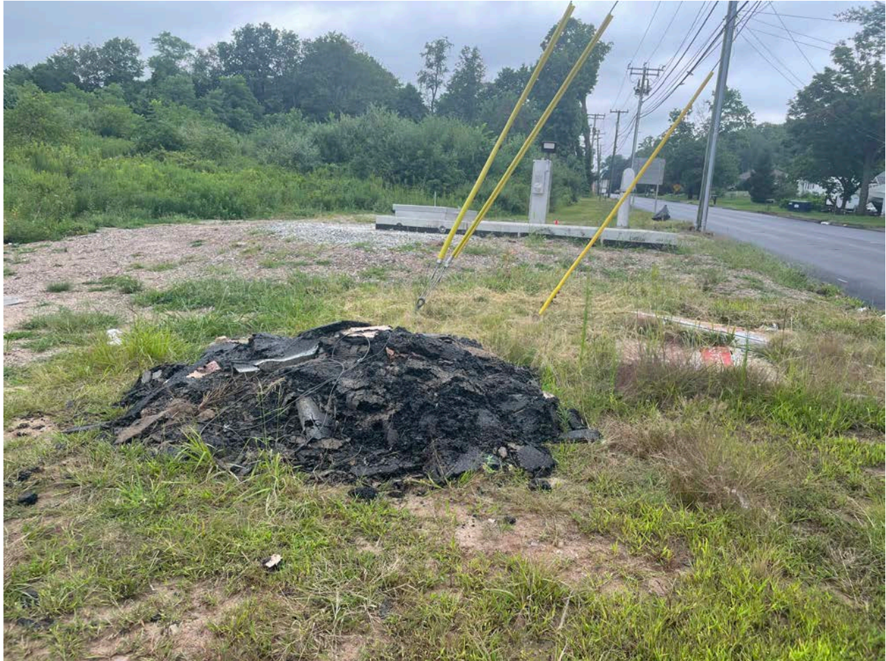
Picture 4: Waste asphalt that was recently placed just south of the pressure PRV vault. Ludlow confirmed that this material was not placed by them. View to the north.
