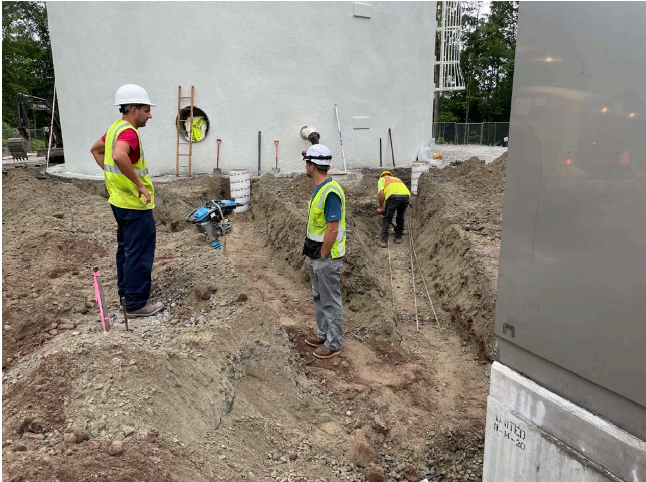
Picture 4: Ludlow placing rebar and chairs in the trenches that Ludlow placed excavated west of the water tank located east of the Shared Access Driveway in Middletown. View to the east.
