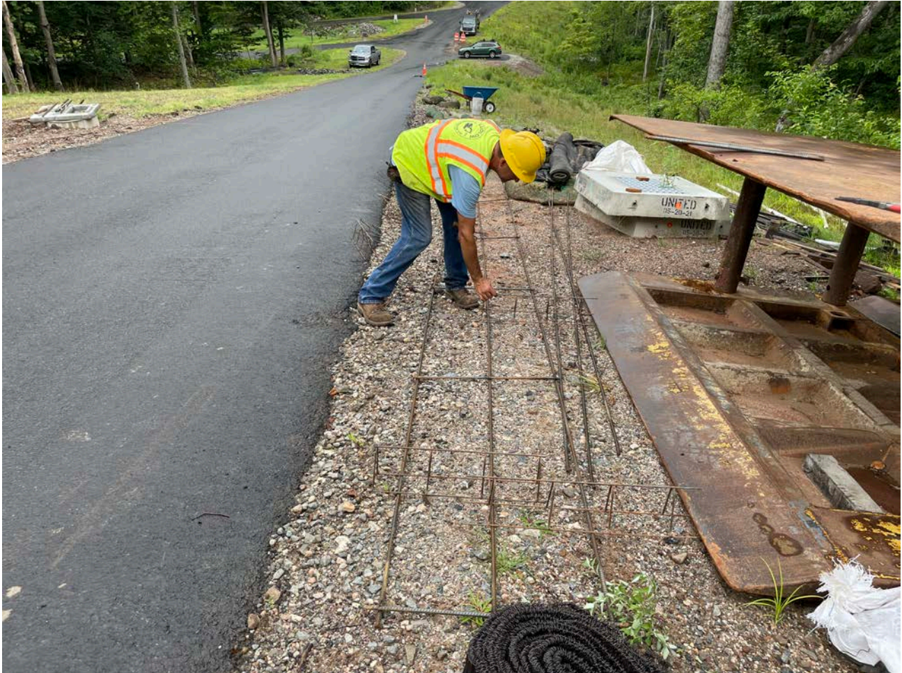
Picture 3: Ludlow staging rebar and chairs that will be wired together and placed in the bottom of the trenches Ludlow is excavating for the installation of duct banks on the west and north side of the water tank located east of the Shared Access Driveway in Middletown. View to the west.
