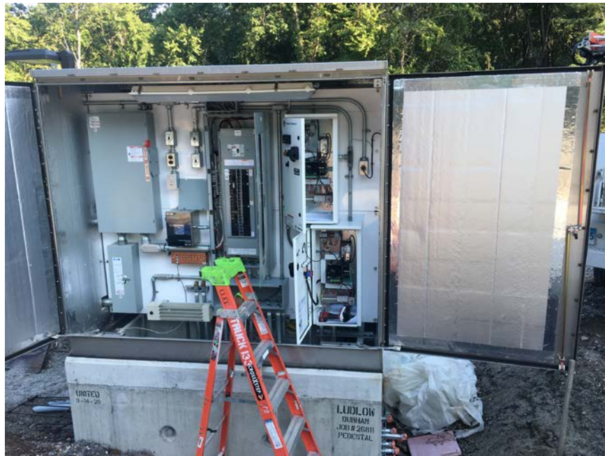
Picture 4: Facing north. Completed control panel up at the Tank. Electrical just needs to run conduits and wire.
