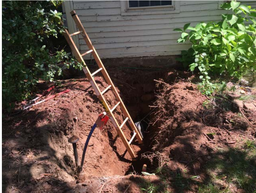
Picture 13: Facing east, 297 Main Street curb stop and trench. Foundation thicker than most other homes. Possible leaking in house causing well to run dry. Location put on priority list.
