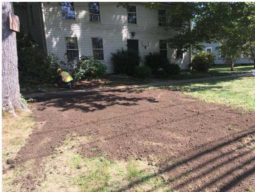
Picture 14: Facing southeasterly at 297 Main Street. Final grading and replacing brick trim.
