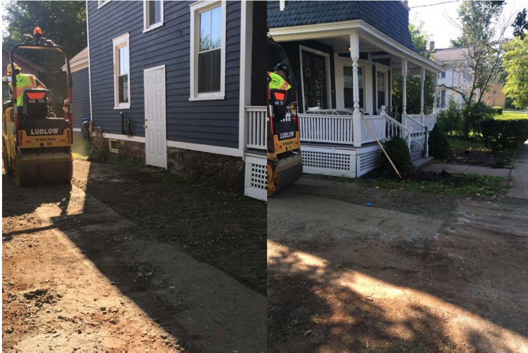
Picture 9: Facing west (L) and south (R). Left is compacting gravel drive, 1" copper enters just base basement window. Right the blue dot is the curb stop.
