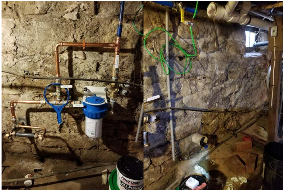
Picture 2: Fazzino installation at 257 Main Street. Left picture is the north wall installation. Right shows inlet.
