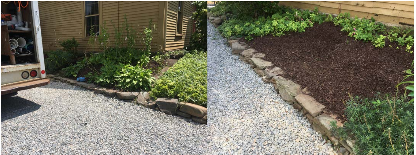
Picture 16: Facing southerly, after shots of stone wall at 257 Main Street after Ludlow made effort to repair. Homeowner seemed pleased with the effort.
