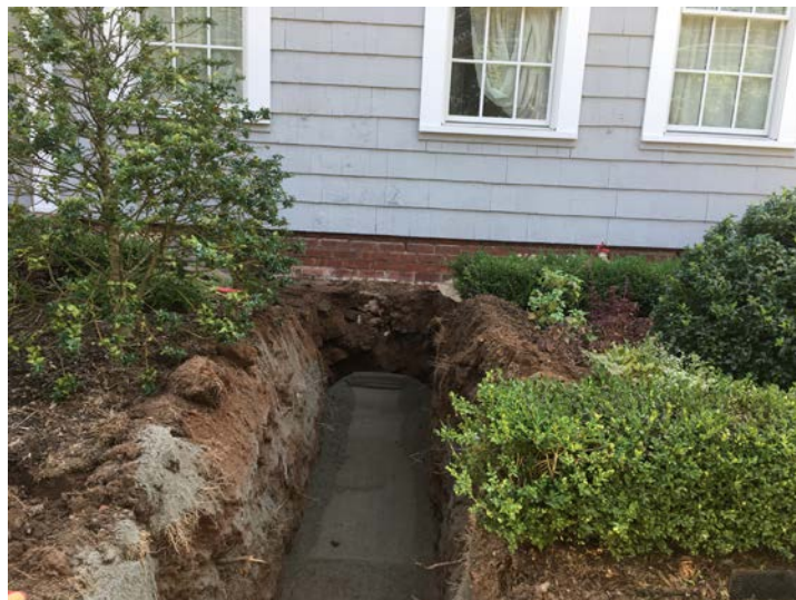
Picture 10: Facing east, 293 Main Street. Resident helped with removing and replacing shrubs. Sanded in 1" copper line.
