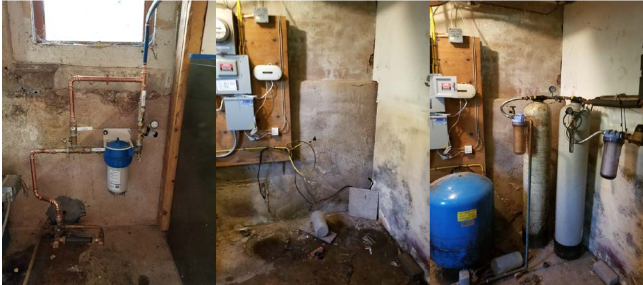
Picture 3: Fazzino installation at 253 Main Street. Left picture is the north wall installation. Center and right are pre-installation.
