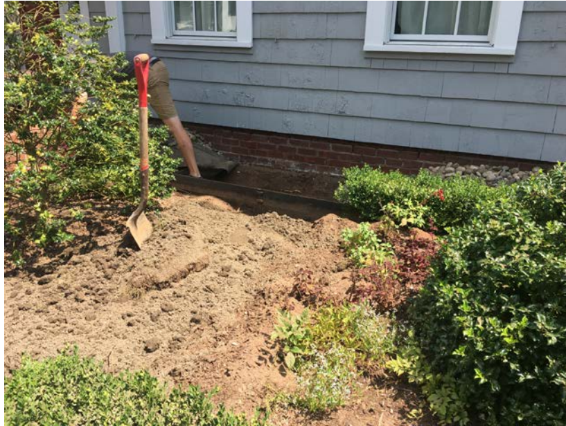
Picture 11: Facing easterly. Finish grade at 293 Main Street.
