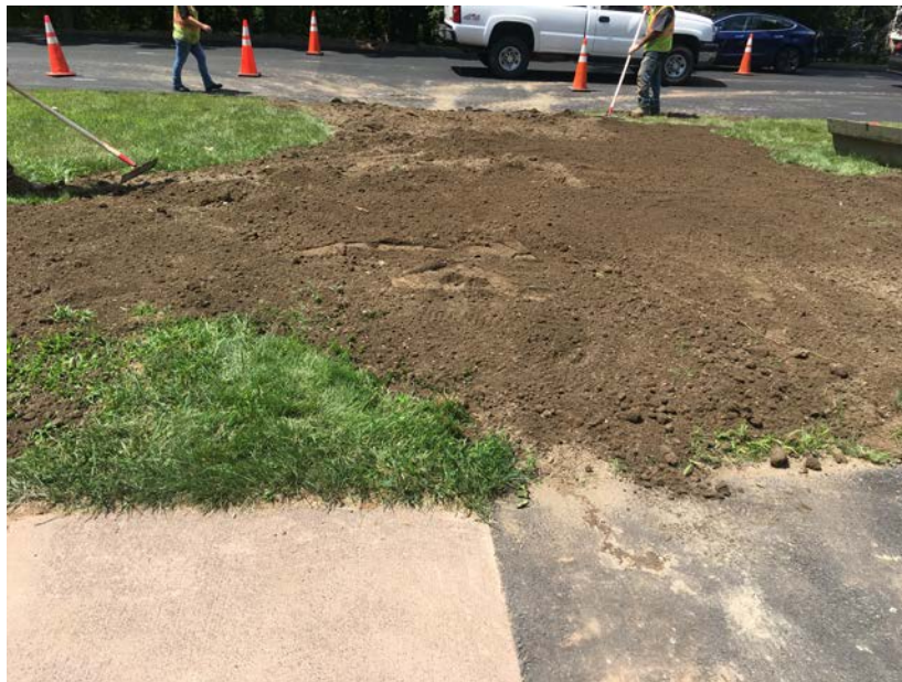
Picture 12: Facing west. Entrance re-grading/seeding at 293 Main Street.
