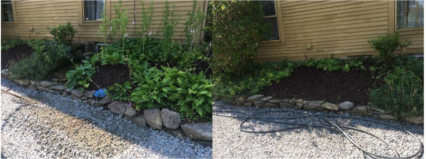
Picture 15: Facing southerly, before shots of stone wall at 257 Main Street, subject of complaint about replacement of wall.
