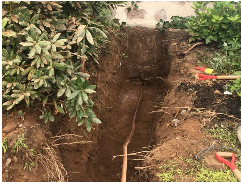
Picture 10: Facing north, 1" copper service into 289 Main Street.
