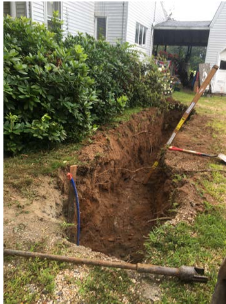
Picture 7: Facing east. View of trench at 289 Main Street.
