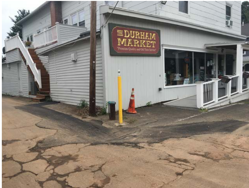
Picture 16: Facing northwest. Durham Market. Patched last night.
