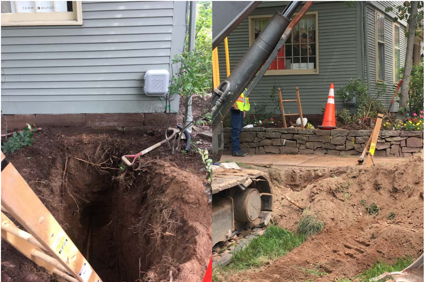
Picture 8: Facing east. Durham Eye Care 243 Main Street. Left is 1" copper line into house, 43 inches from corner and 5 feet below top of sill. Right view from further back. Note curb stop adjacent to sidewalk by crack.
