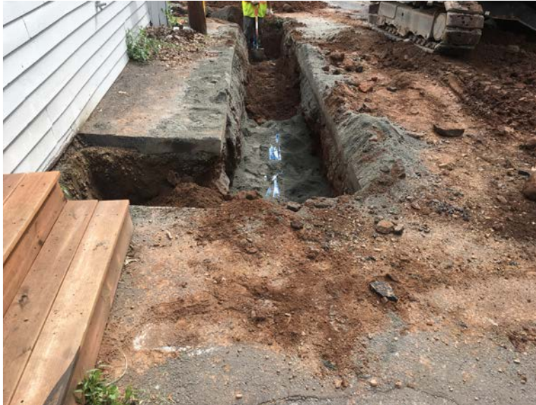
Picture 4: Facing east. Water line trench on south side of Durham Market, 5 feet out.
