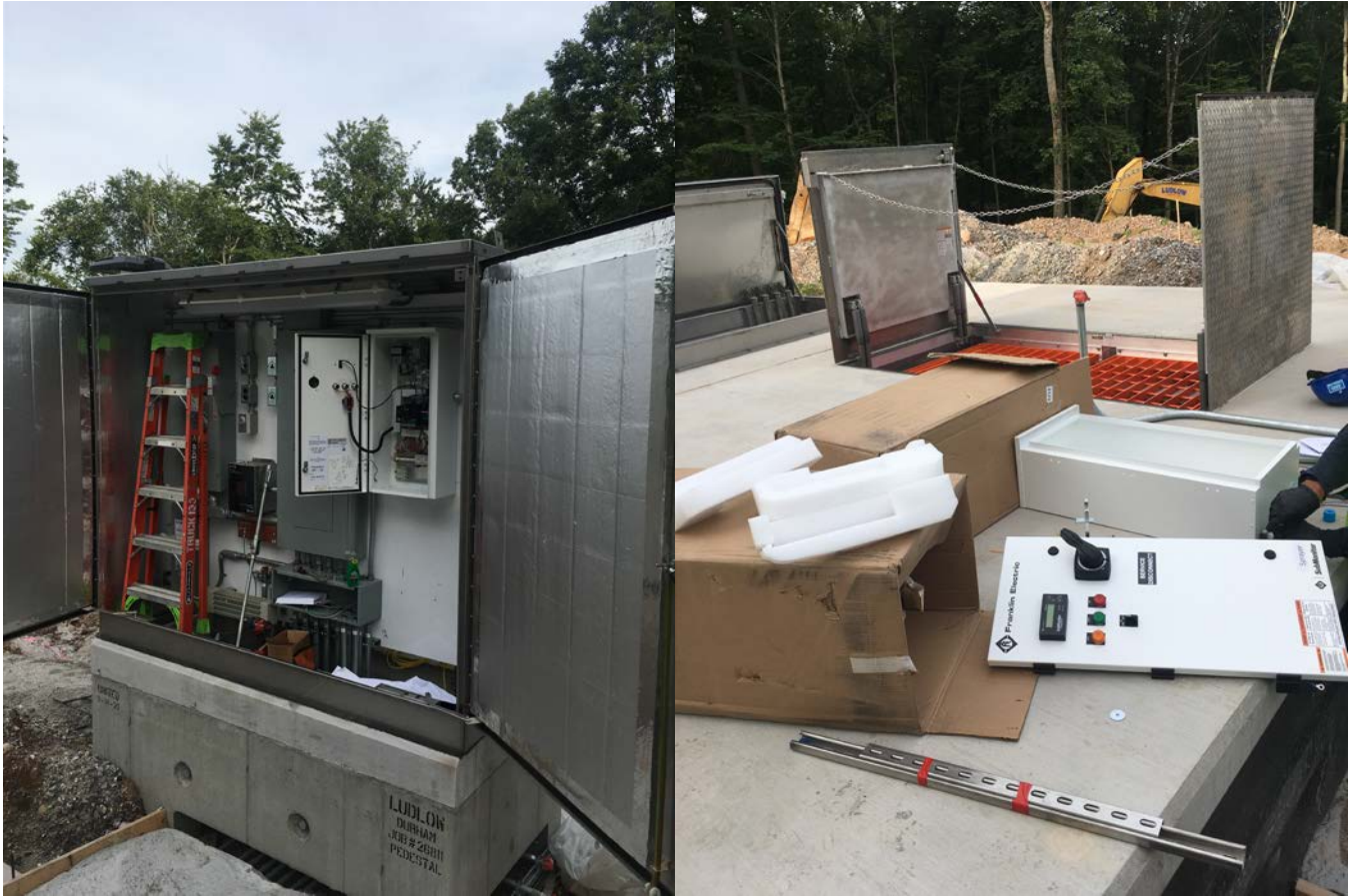
Picture 1: United Concrete electrician working on Control Box up at the Tank. Electrician had to reconfigure the box because the control panels being installed were larger than expected.
