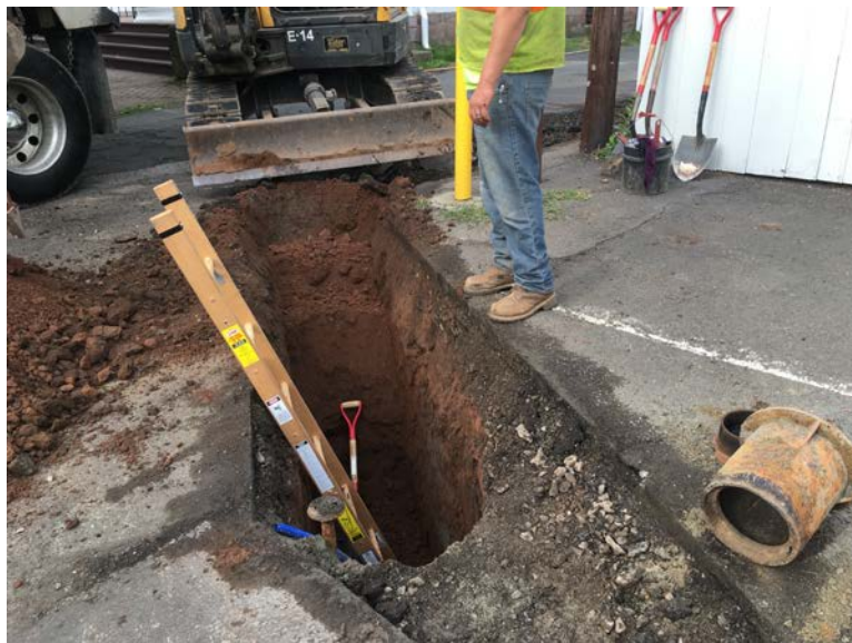
Picture 3: Facing southwest Curb stop in front of ladder.
