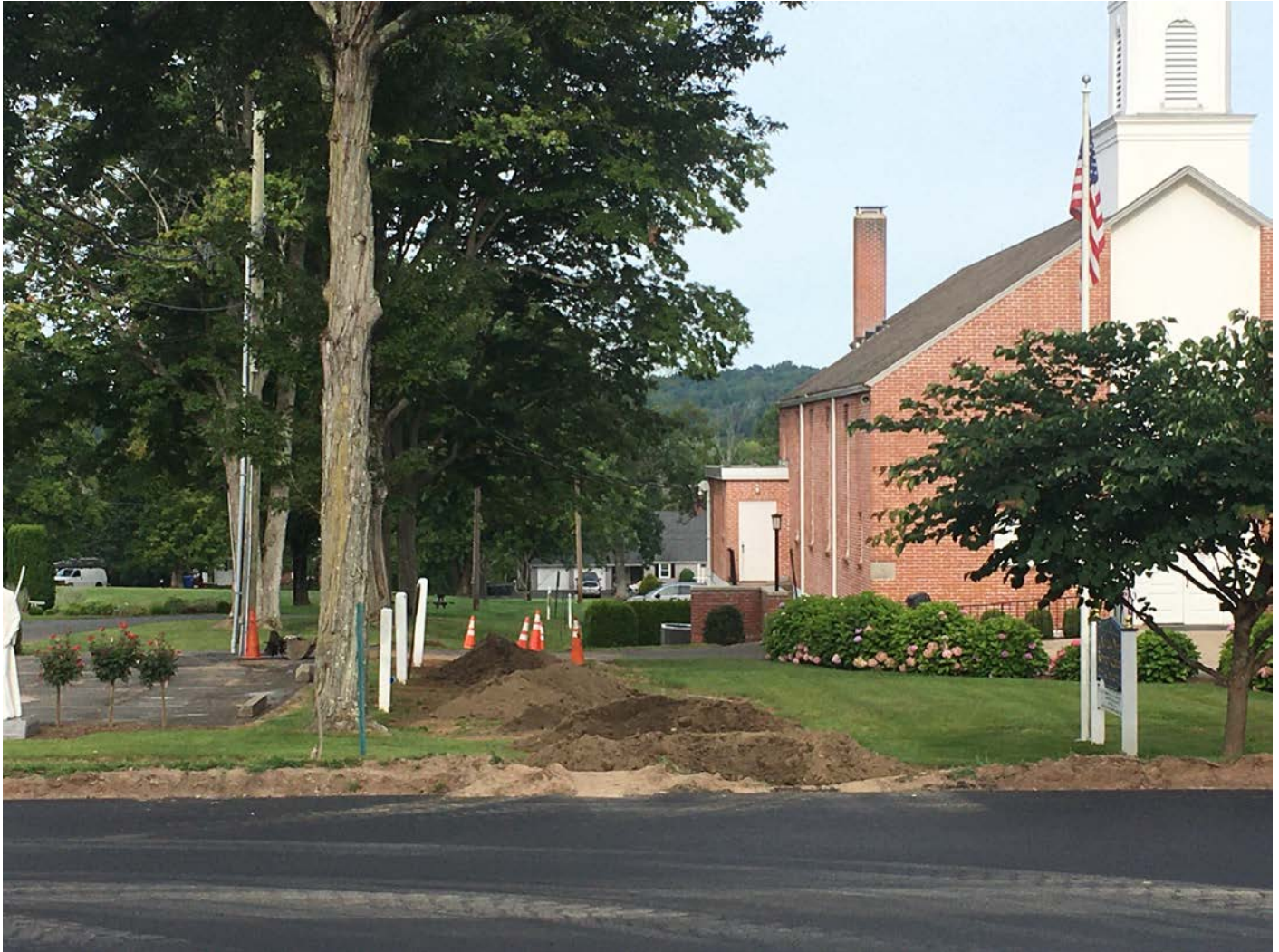
Picture 11: Facing west. 280 Main Street. Notre Dame Church. To be completed this week.
