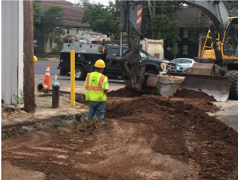
Picture 6: Facing northeast. Backfilling water line trench. The telephone pole existing well, and bollard line roughly up with the curb stop (located behind the worker).
