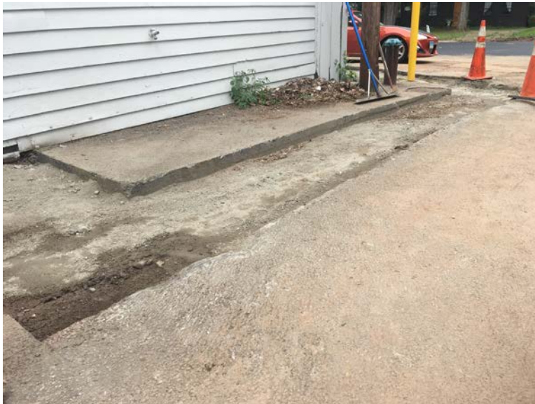
Picture 5: Facing east. Same view as above. Finished fill, waiting for asphalt.
