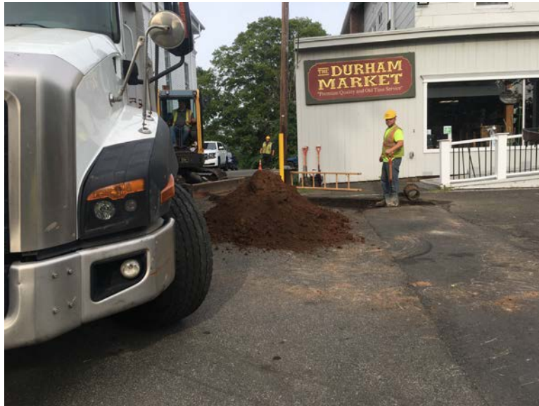
Picture 2: Facing west. Durham Market water line installation 1 inch copper line..
