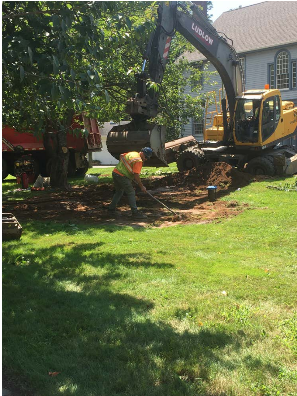
Picture 9: Ludlow regrading and cleaning up at 272 Main Street. Note water supply well location.
