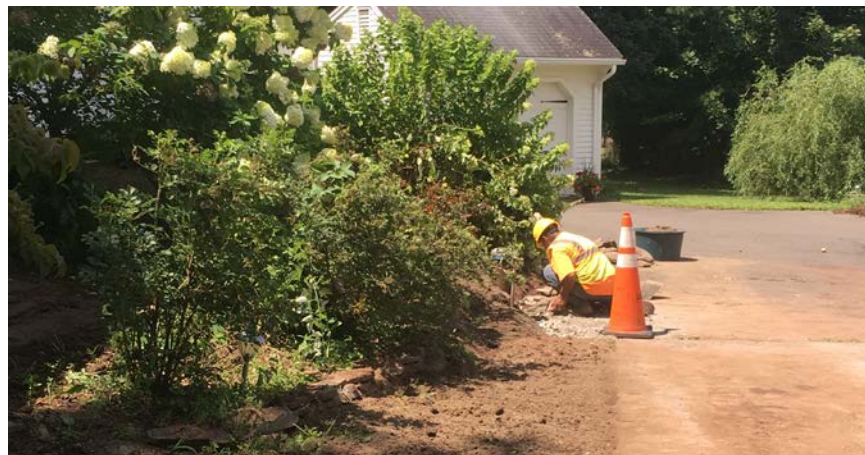
Picture 6: Facing west. Re-setting flagstone wall along drive. Small wall maybe 10 feet long.
