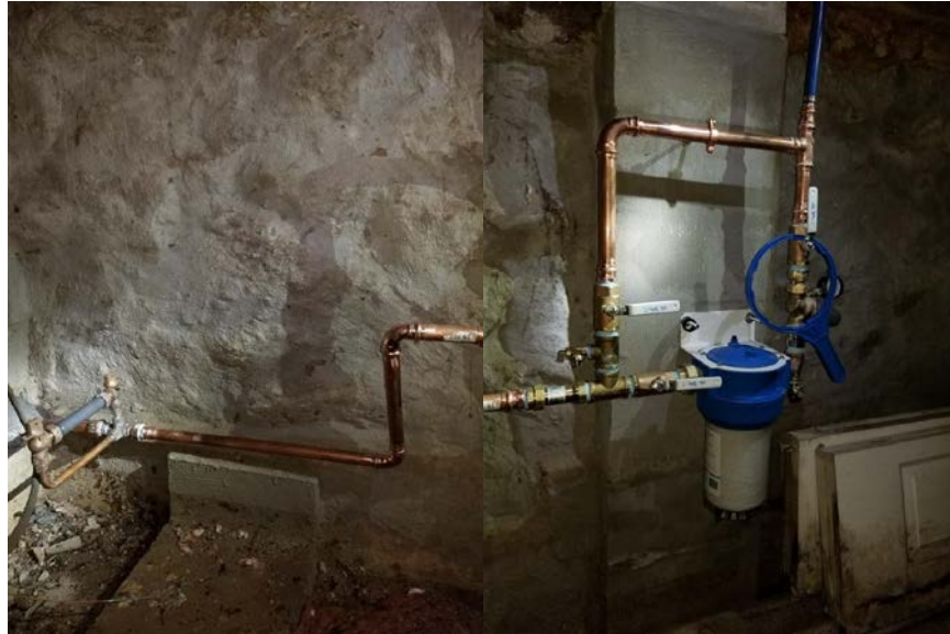
Picture 3: Fazzino installation at 233 Main Street, complete.
