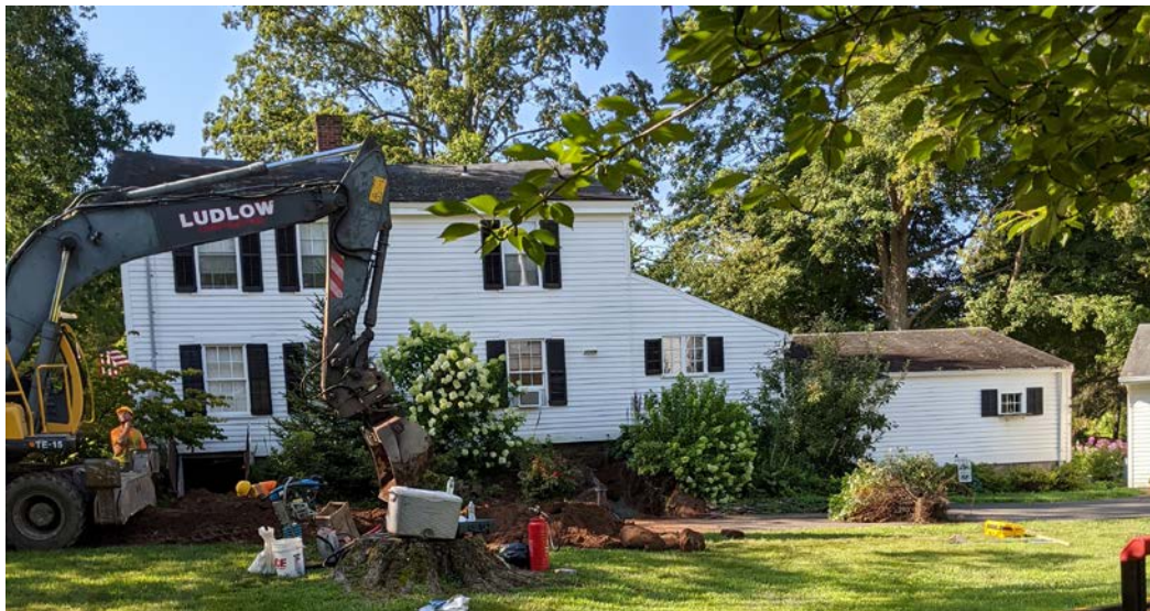
Picture 4: Facing south. Ludlow backfilling 1" copper service line at 268 Main St. Line installed along edge of drive.
