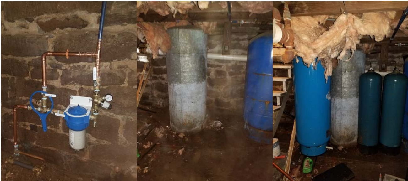
Picture 2: Fazzino installation at 235 Main Street. Need to install three smaller water meters on landlords' side but otherwise complete. Fazzino did not state when they would get to doing the additional meters.
