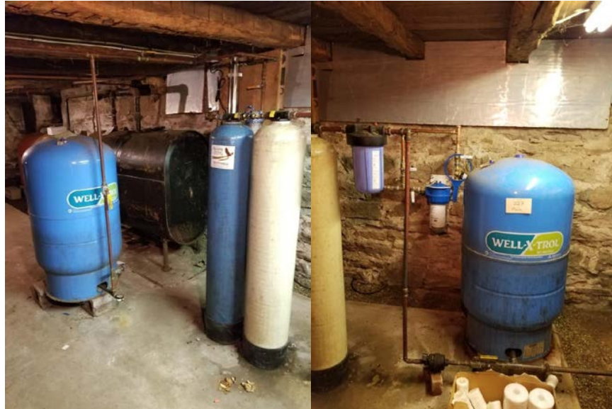
Picture 1: Fazzino installation at 227 Main Street. Completed pre-water line to allow smooth transition of service.
