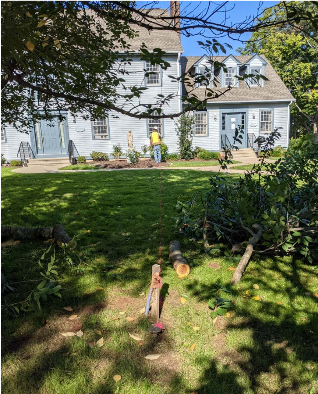
Picture 7: Facing west. Laying out the line at 272 Main St (church rectory). Line enters where person is standing; 5.5 feet to nearest corner of building to the right of person in photo Note tree limbs cut to provide access. Existing well is to right of new water line.
