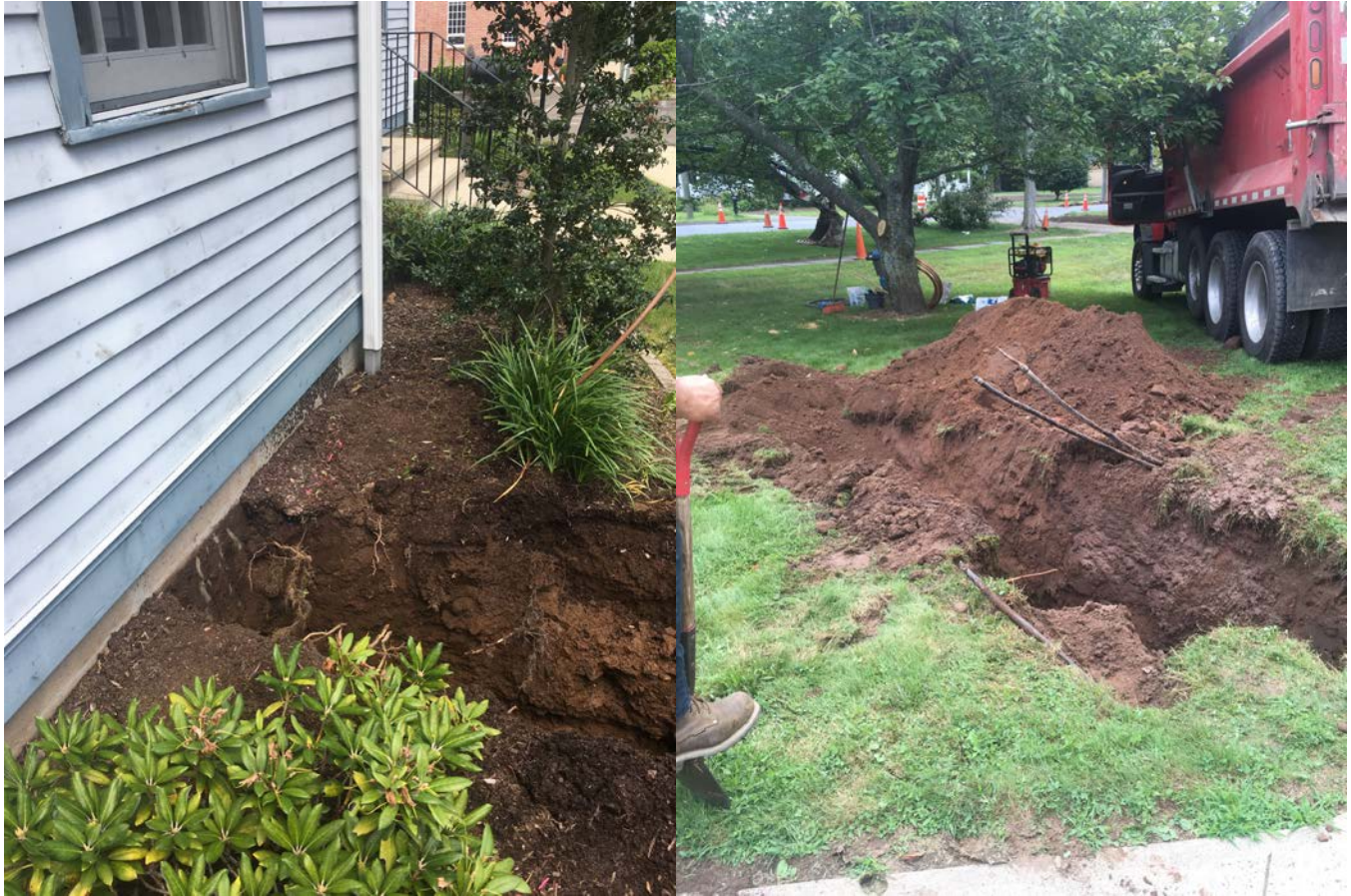
Picture 8: Ludlow excavating at 272 Main Street property. Left faces north. Installation trench for 1" copper service line; 6 feet deep from top of sill. Right faces east. Trench extending out to curb stop. Note tubes sticking up are part of a drip irrigation lines that seems to be randomly buried. Ludlow is looking for parts to repair.
