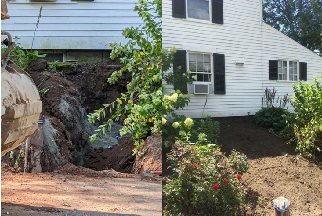
Picture 5: Facing south – 268 Main St. Left is service line buried in sand with water tape on top. Right is finish grade. Line is 14 feet from back sloped roof section of building.
