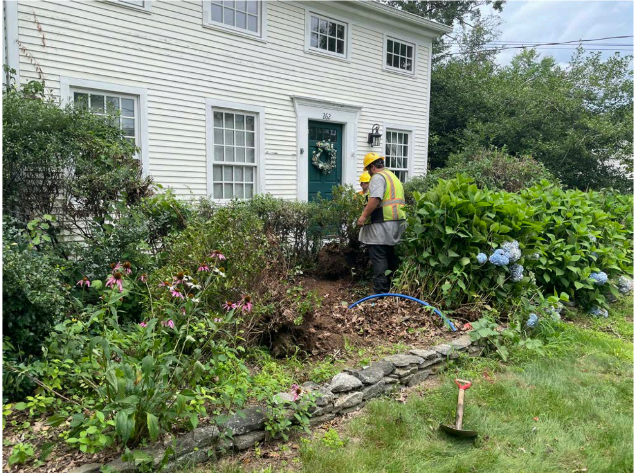
Picture 5: Ludlow moving shrubs from the path they will excavate at the 262 Main Street property for the installation of a 1" copper water service line. View to the northwest.
