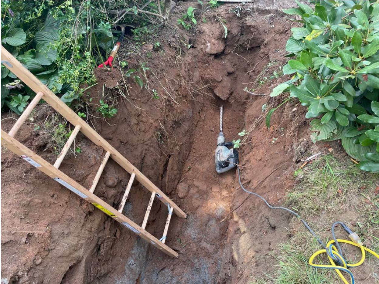
Picture 2: Ludlow in the process of penetrating the foundation on the east side of the 267 Main Street, Durham, residence for the installation of a 1" copper water service line. View to the east.
