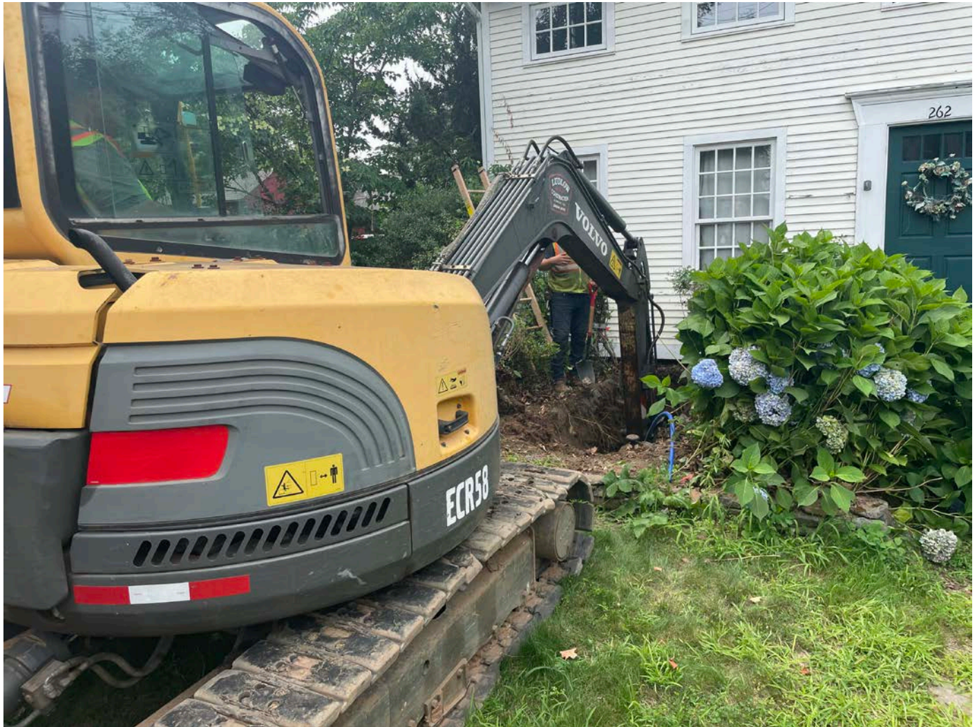
Picture 6: Ludlow excavating at the 262 Main Street property for the installation of a 1" copper water service line. View to the west.
