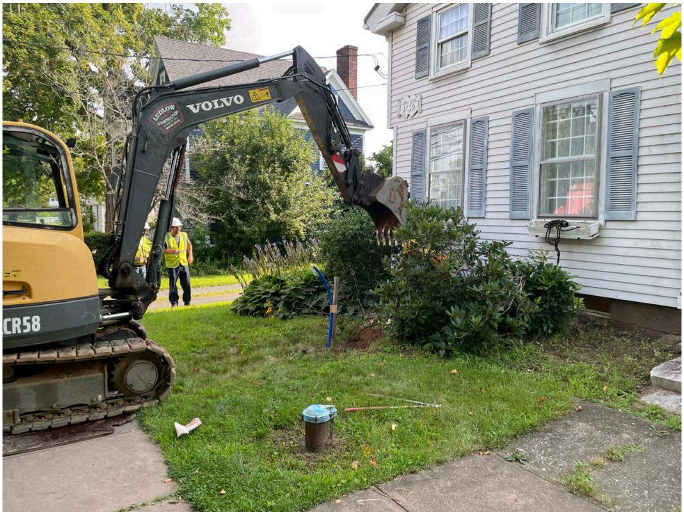
Picture 1: Ludlow excavating on the west side of the 267 Main Street, Durham, residence for the installation of a 1" copper water service line. View to the southwest.
