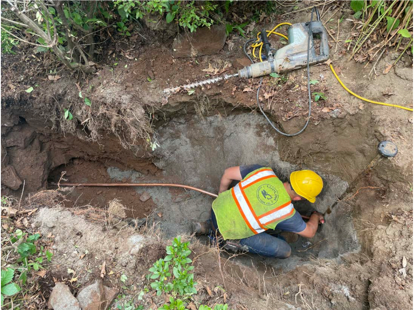
Picture 7: Ludlow installing a 1" copper water service line through the foundation of the 267 Main Street, Durham.
