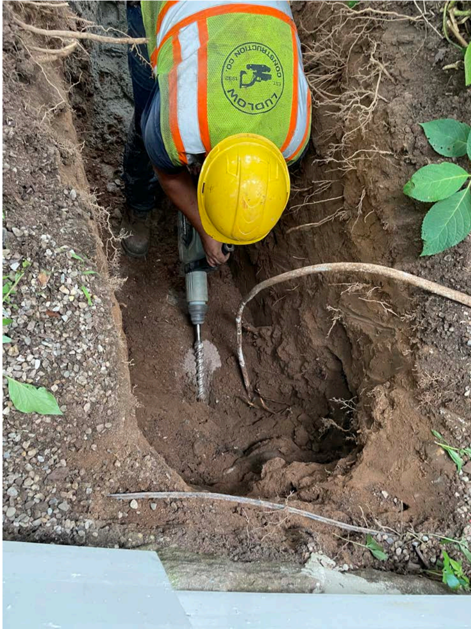
Picture 4: Ludlow in the process of penetrating the foundation on the east side of the 256 Main Street, Durham, residence for the installation of a 1" copper water service line.
