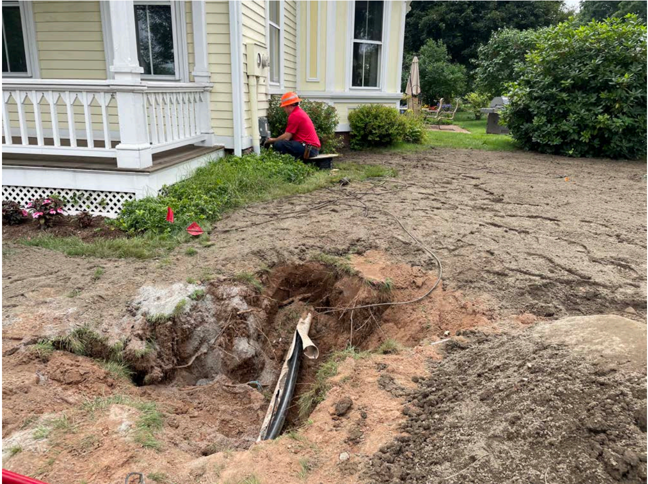
Picture 3: Frontier working at the 265 Main Street residence repairing the communications cable that was severed yesterday by Ludlow during the installation of a 1" copper water service line.
