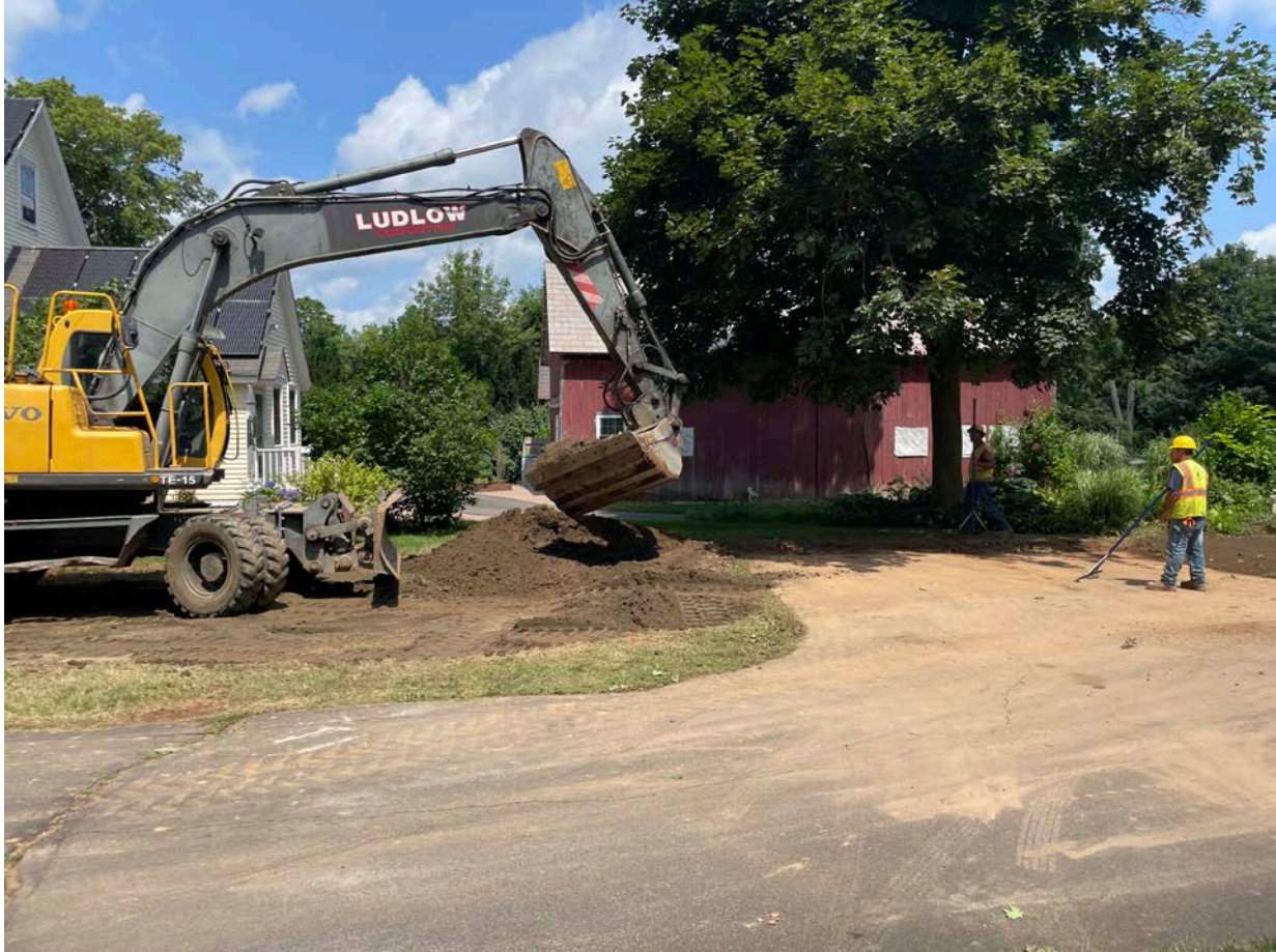
Picture 4: Ludlow placing loam on portions of the lawn at the 261 Main Street property that were disturbed during the installation of a 1.5" copper water service line. View to the east.
