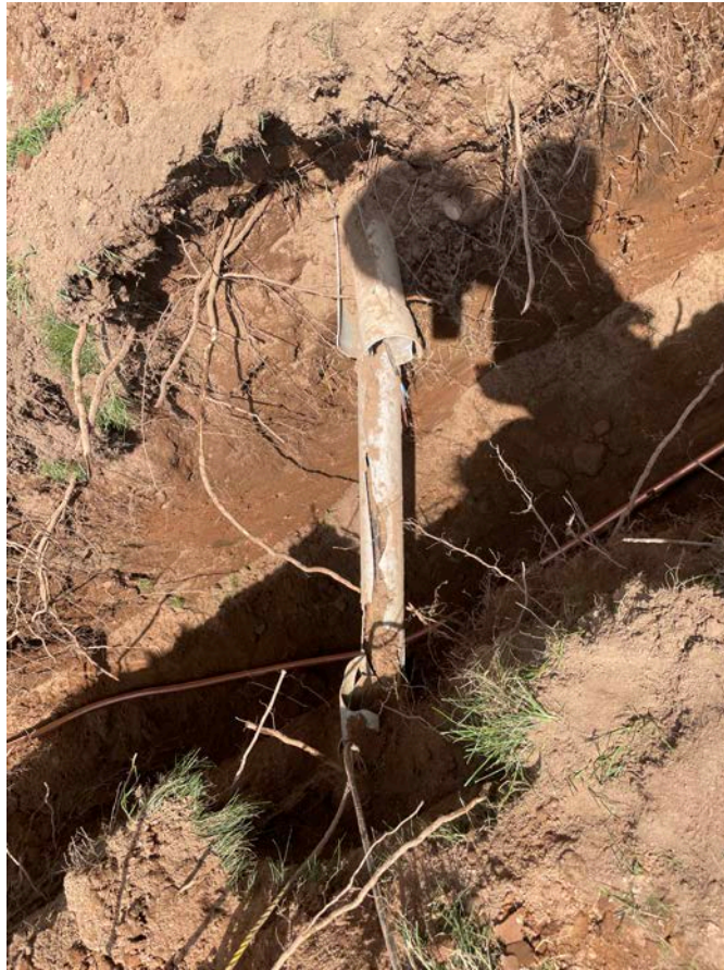
Picture 8: Communications line that was severed during the installation of a 1" copper water service line at the 257 Main Street residence. View to the east.
