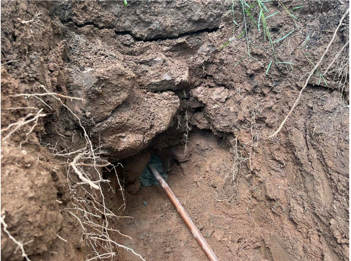
Picture 7: 1" copper water service line that was installed through the field stone foundation of the residence located at 257 Main Street, Durham. View to the north.
