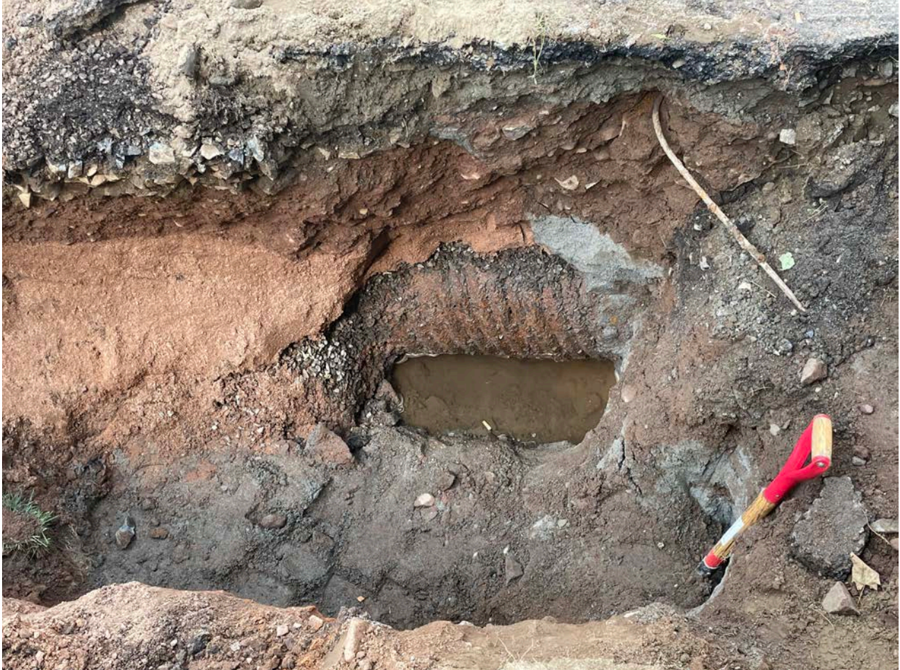
Picture 3: 16" metal storm drain that Ludlow daylighted when they investigated a sink hole on Main Street next to the 397 Main Street, Durham, residence. Note the holes that are visible on the side of the pipe. View to the west.
