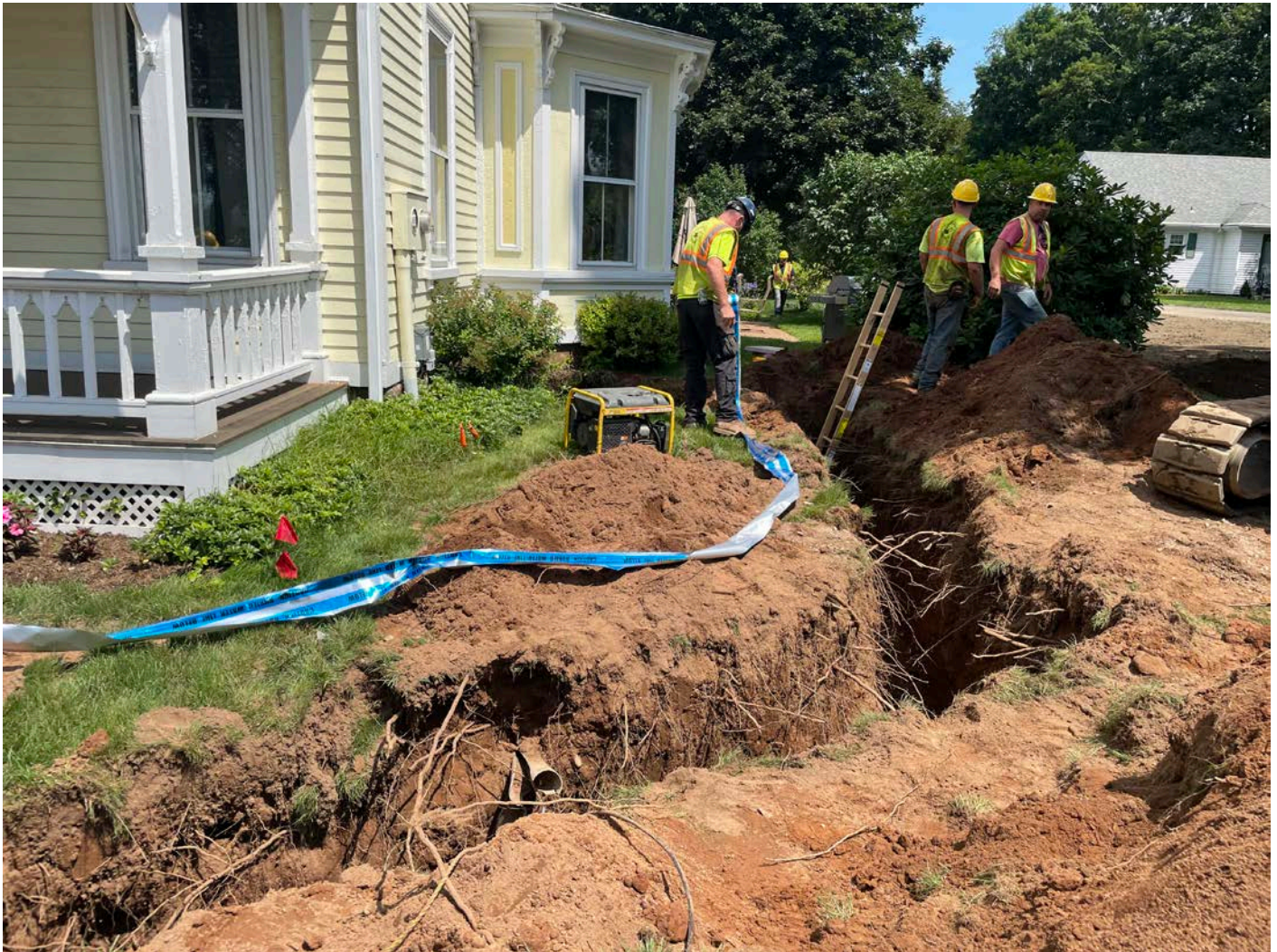
Picture 6: Ludlow about to place caution tape into the excavation at the 257 Main Street property for the installation of a 1" copper water service line. View to the east.
