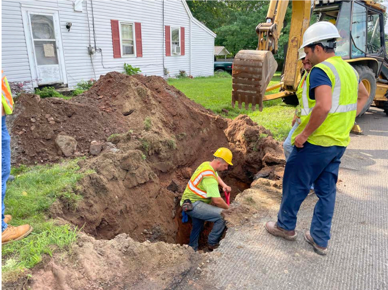
Picture 2: Ludlow excavating a sink hole on Main Street next to the 397 Main Street, Durham, residence. View to the south.
