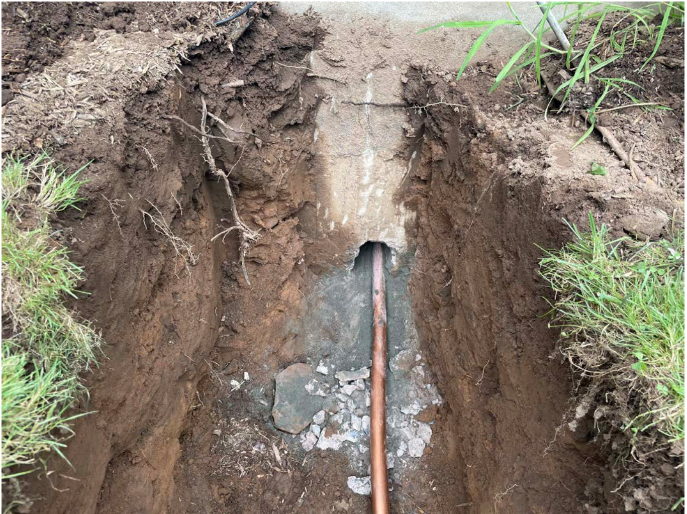
Picture 1: 1.5" copper water service line that was inserted through the east side of the foundation at 261 Main Street, Durham. View to the west.
