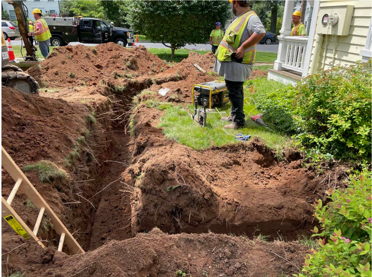
Picture 5: Ludlow excavating at the 257 Main Street property for the installation of a 1" copper water service line. View to the west.
