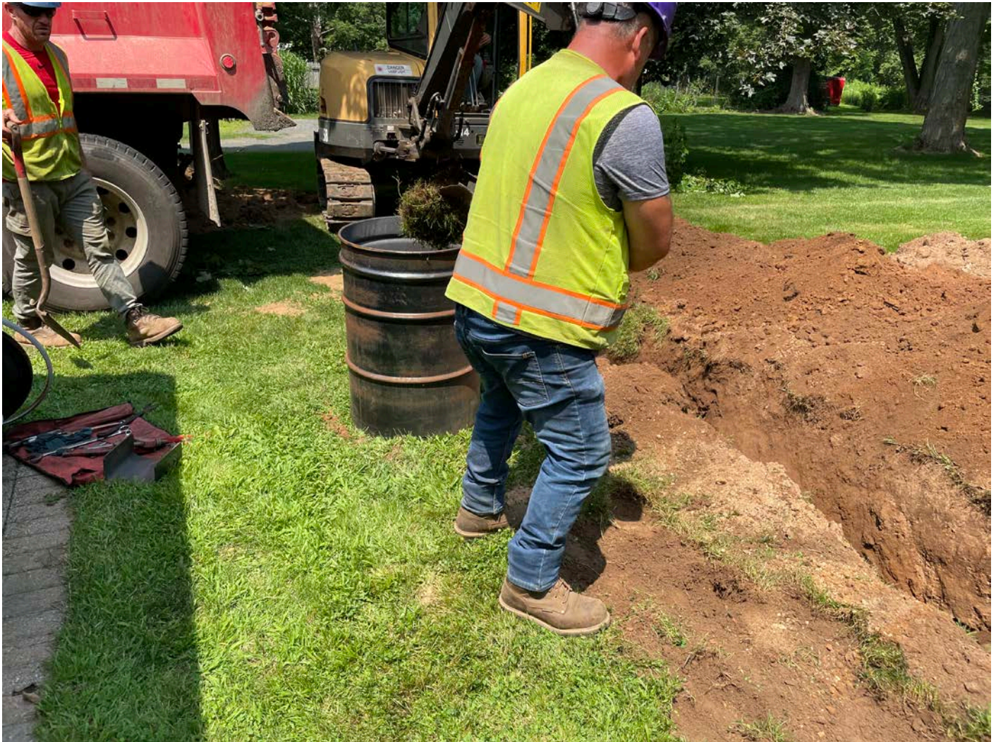
Picture 9: Ludlow containerizing a small amount of soil that was impacted during the release of hydraulic fluid at the 261 Main Street, Durham, property. View to the north.
