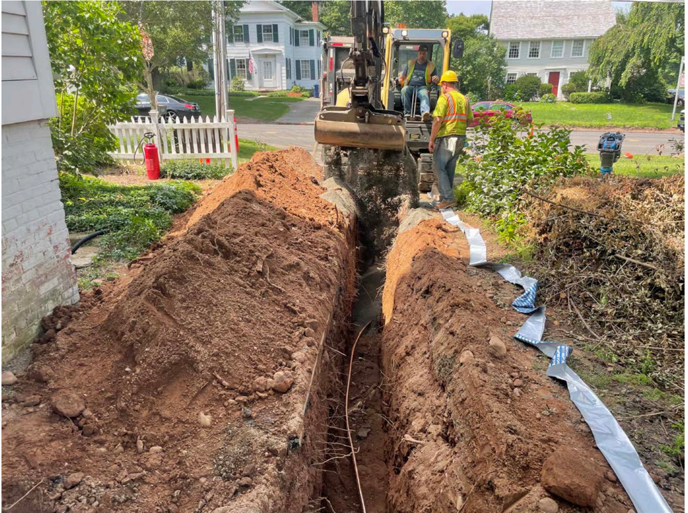
Picture 6: Ludlow backfilling over 1" copper water service line on the north side of the 253 Main Street residence. View to the west.
