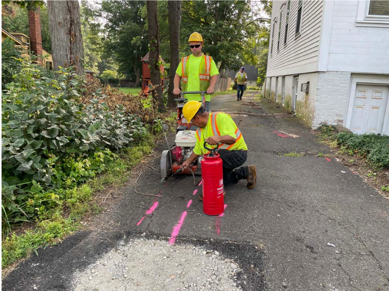
Picture 2: Ludlow saw cutting the outline of a trench before excavating on the driveway for 253 Main Street, Durham. View to the west.
