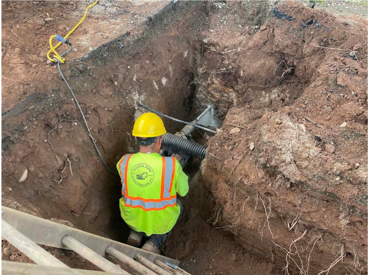
Picture 5: Ludlow using a rotary hammer to penetrate the southern foundation of the 253 Main Street residence. View to the northwest.
