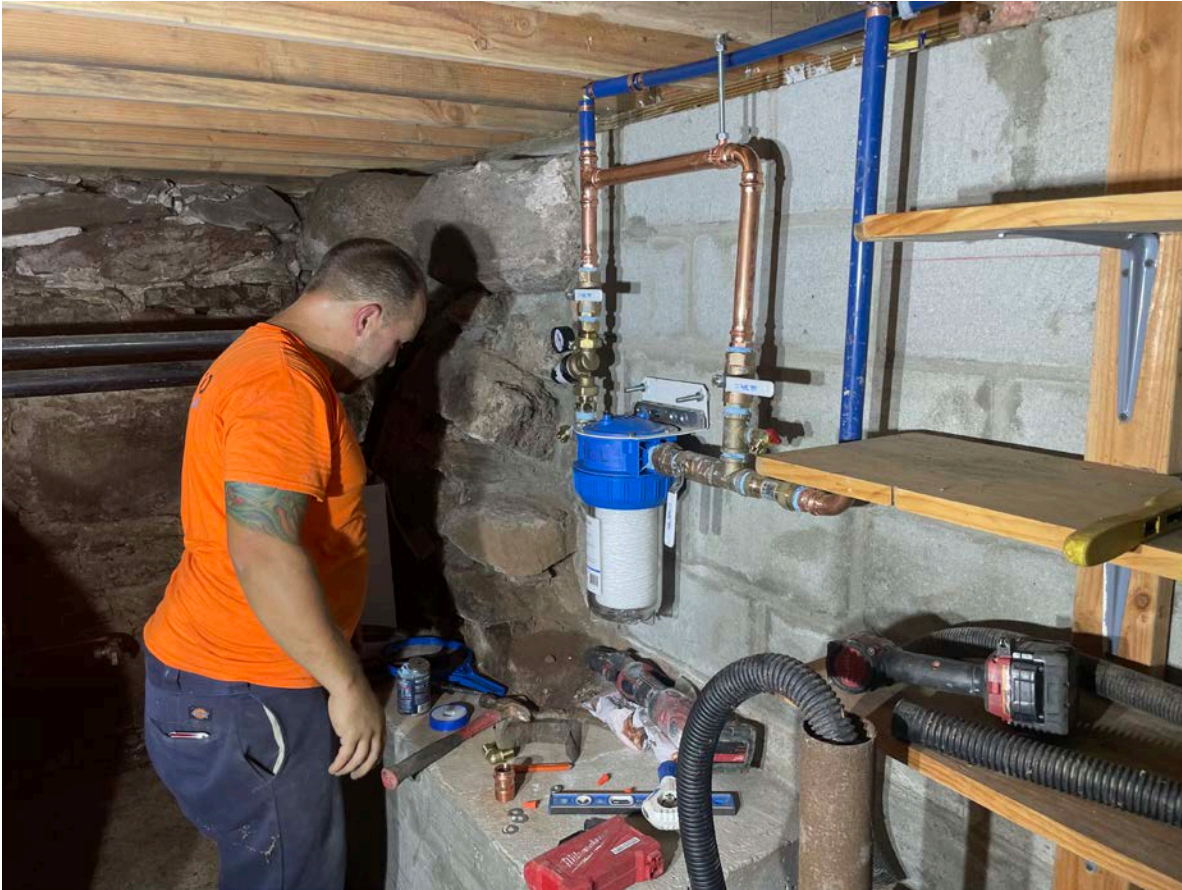
Picture 8: Fazzino installing final water service components the 196 Main Street, Durham, residence.
