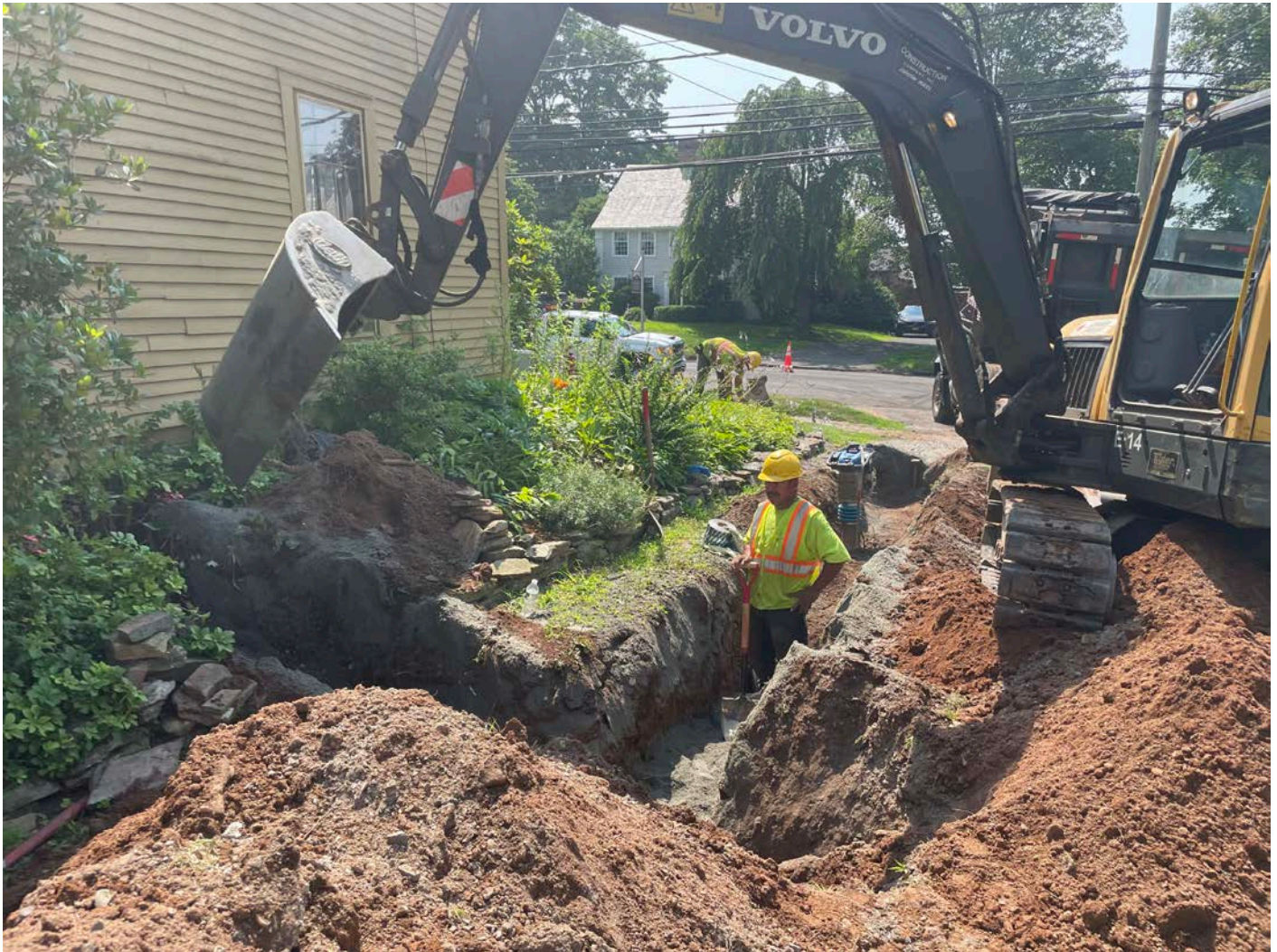
Picture 7: Ludlow backfilling over 1" copper water service line on the north side of the 257 Main Street residence. View to the southwest.
