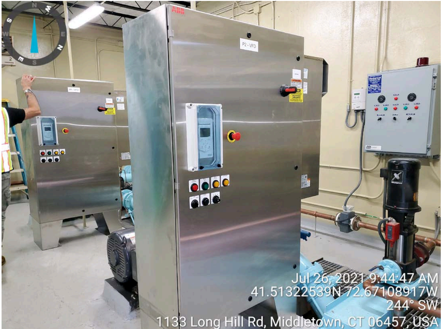
Picture 9: VFD panels that Ludlow installed at the Long Hill pump station today.
