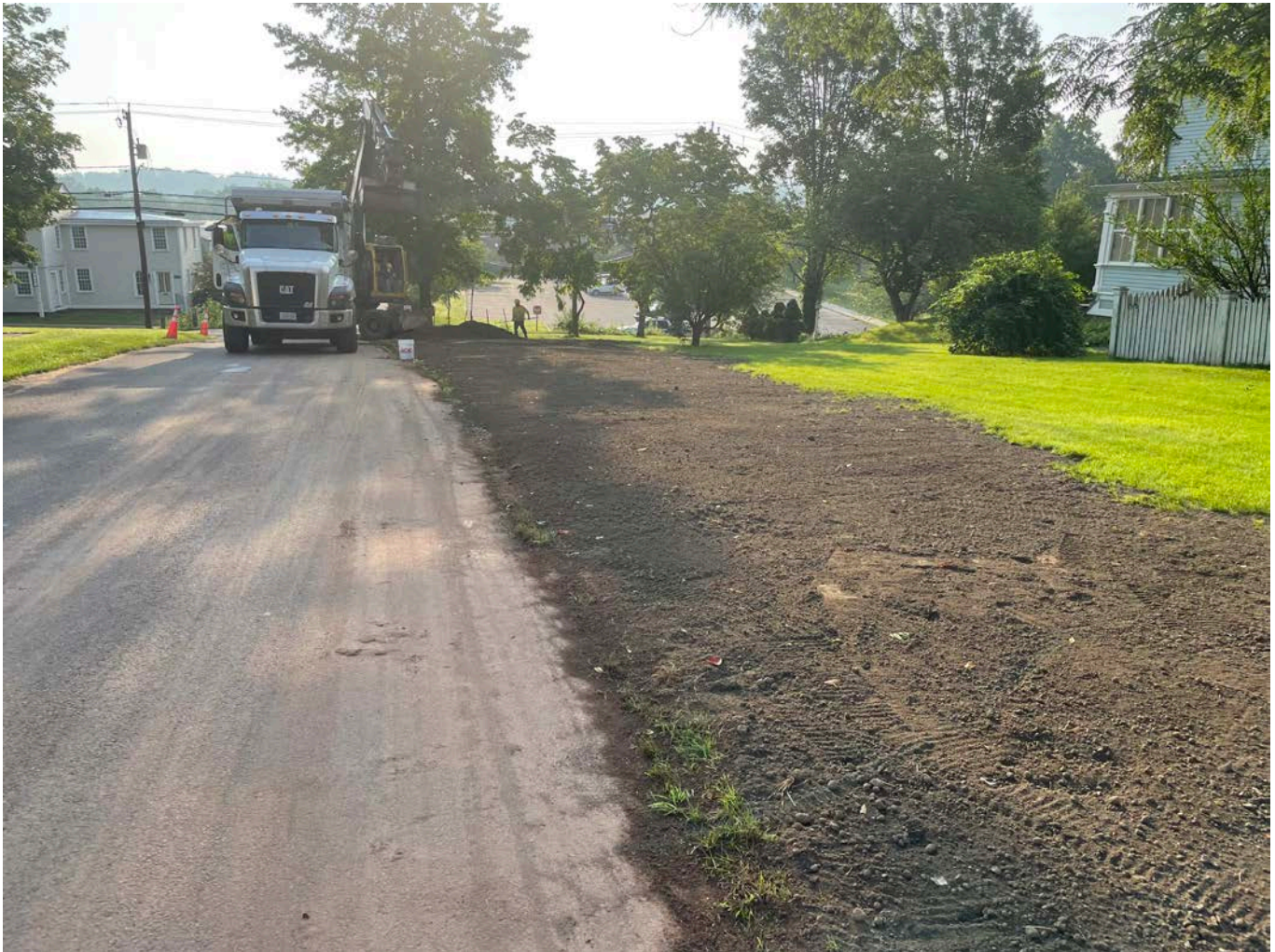
Picture 1: Ludlow finishing the placement of loam and seed at 196 Main Street, Durham. View to the east.
