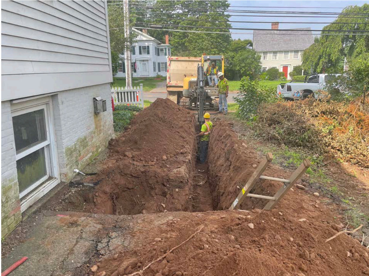
Picture 4: Ludlow excavating on the driveway of the 253 Main Street residence as they prepare to install 1" copper water service line to the home. View to the west.
