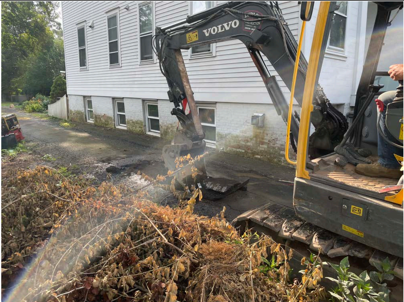
Picture 3: Ludlow excavating on the driveway of the 253 Main Street residence as they prepare to install 1” copper water service line to the home. View to the northwest.
