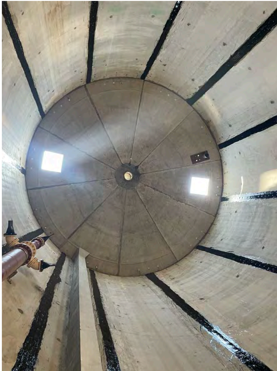
Picture 6: Top of the water tank after DN Tanks filled holes for the lift lines with non-shrink grout (Tamms Structural Mortar).
