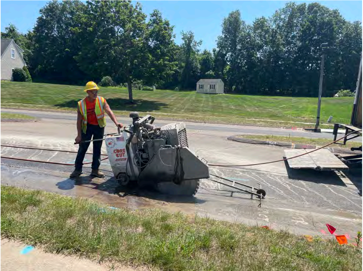
Picture 7: Ludlow saw cutting pavement on the westbound lane of Talcott Ridge Drive. View to the south.
