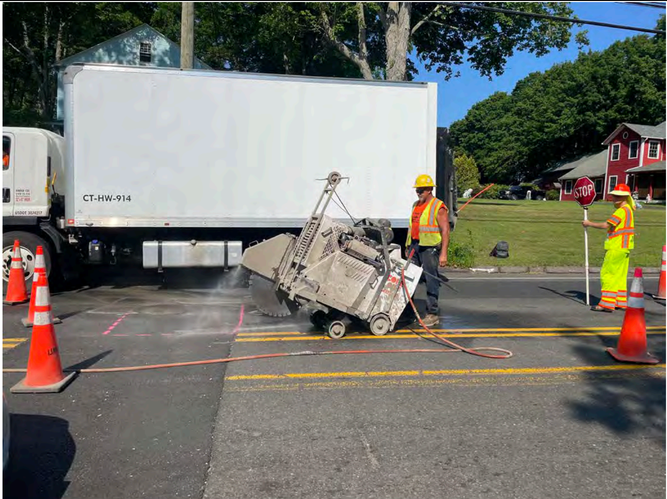
Picture 2: Ludlow saw cutting pavement on the southbound lane of Main Street due east of 208 Main Street (~Station 197+90). View to the west.
