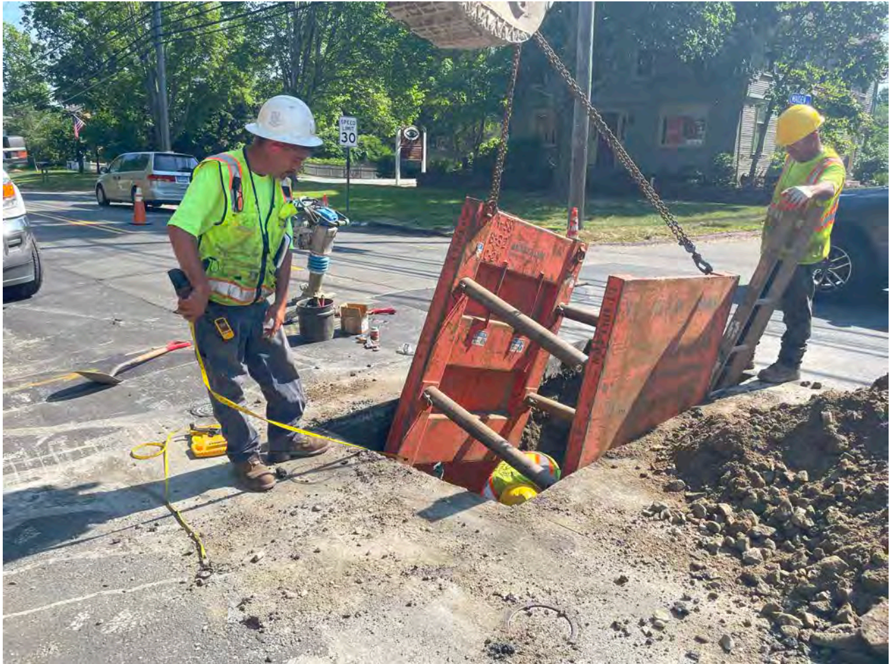
Picture 3: Ludlow removing 1" copper blowoff line from the intersection of Maiden Lane and the southbound lane of Main Street, Durham. View to the northeast.
