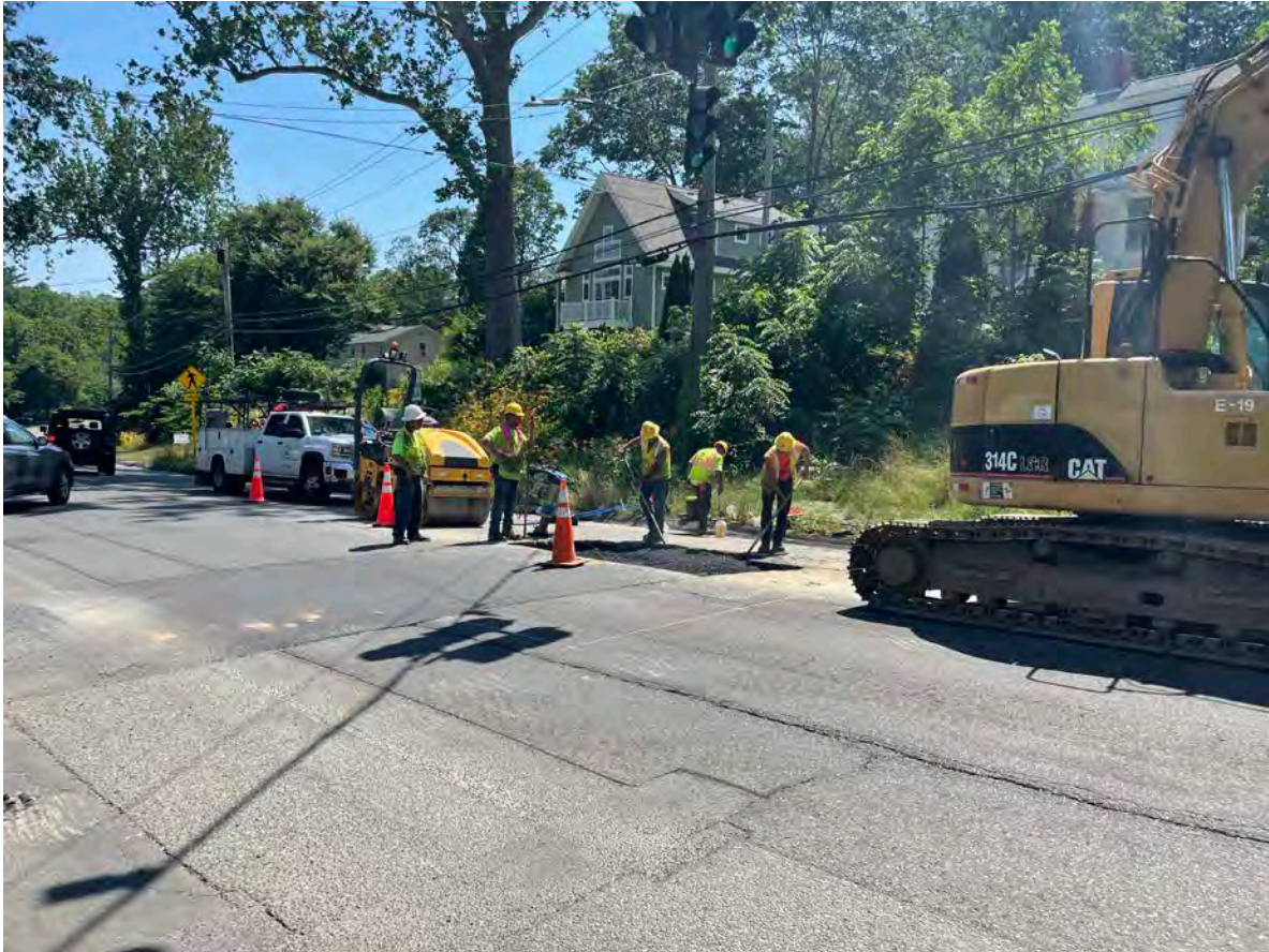
Picture 9: Ludlow placing the first lift of asphalt on the patch where they removed a 1" copper blowoff line on the southbound lane of Main Street, Durham where it intersects with Pickett Lane. View to the southwest.
