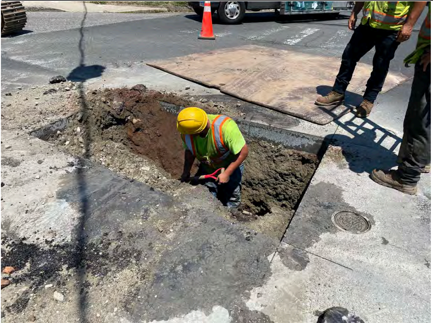
Picture 5: Ludlow removing 1" copper blowoff line from the intersection of Wallingford Road and the southbound lane of Main Street, Durham. View to the southwest.
