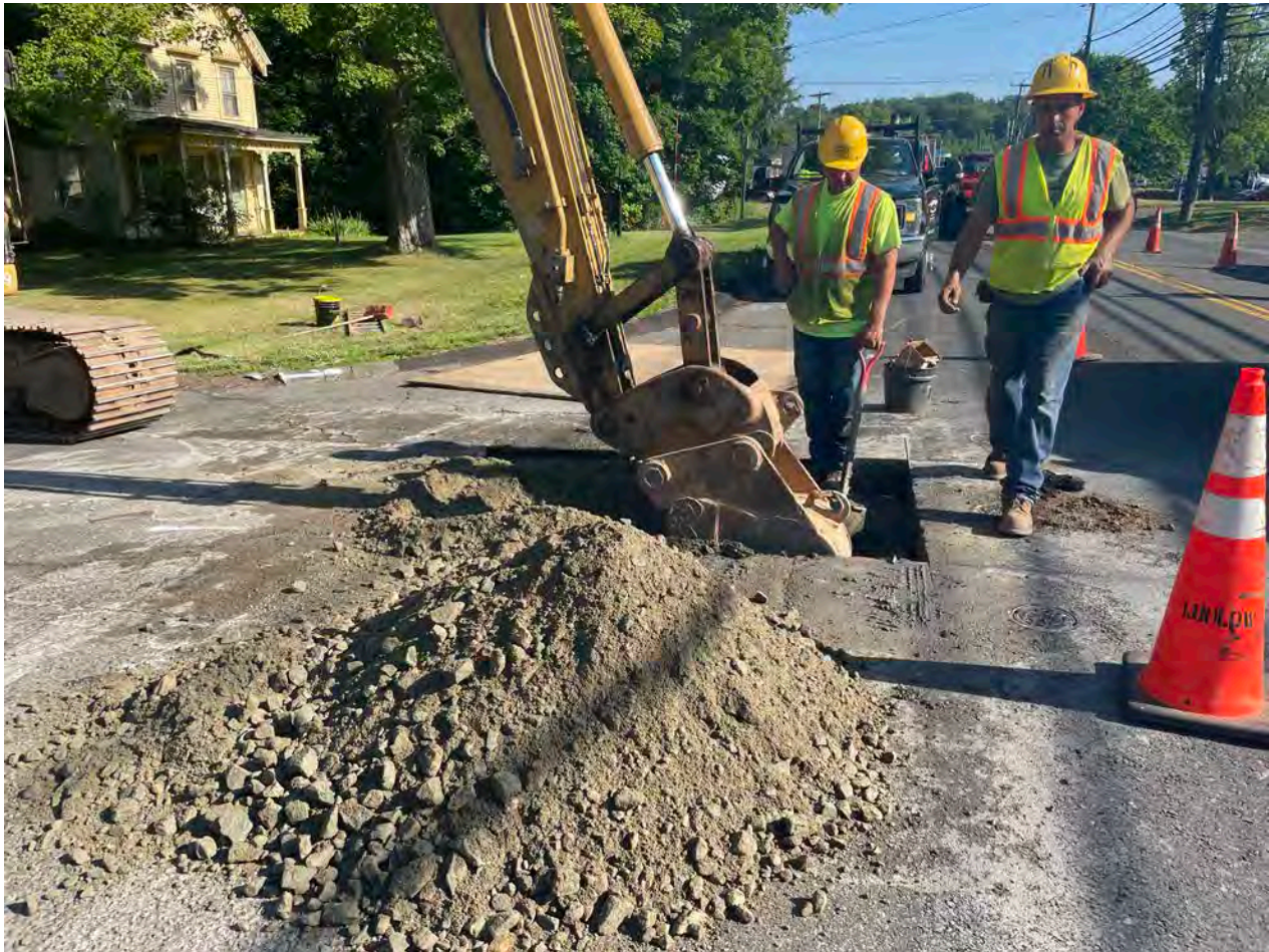
Picture 1: Ludlow excavating at the intersection of Talcott Lane and the southbound lane of Main Street, Durham as they prepare to remove a 1" copper blowoff line. View to the north.
