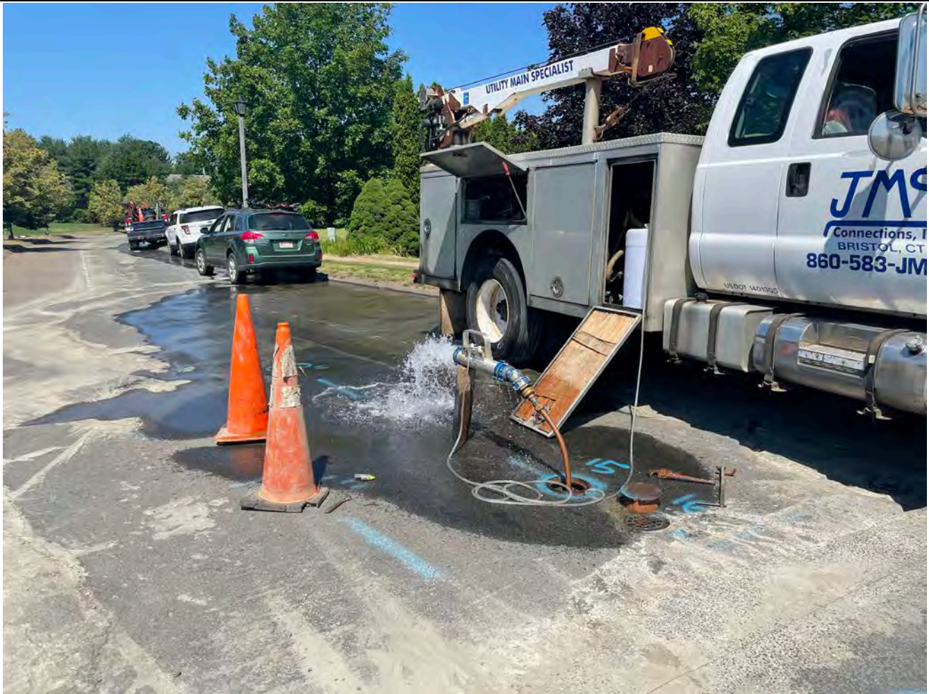
Picture 4: Ludlow purging 8" DIP line that runs between the booster Station and the intersection of Talcott Ridge Drive and Watch Hill Drive, Middletown as part of dechlorination activities. View to the west.
