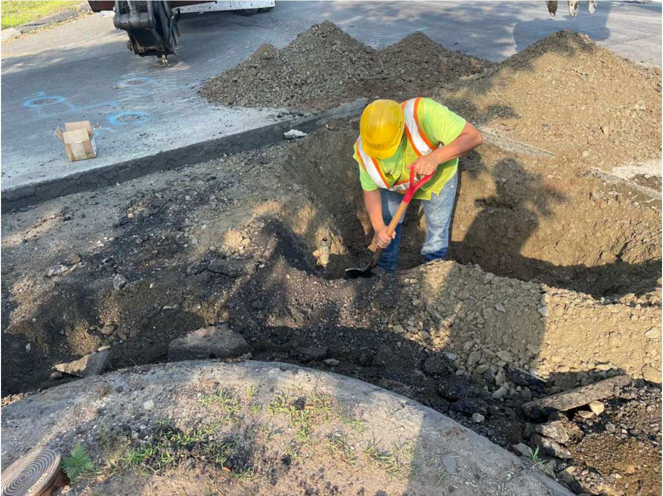
Picture 2: Ludlow hand digging around a 1" copper blow off pipe that they plan to remove today. View to the southwest.
