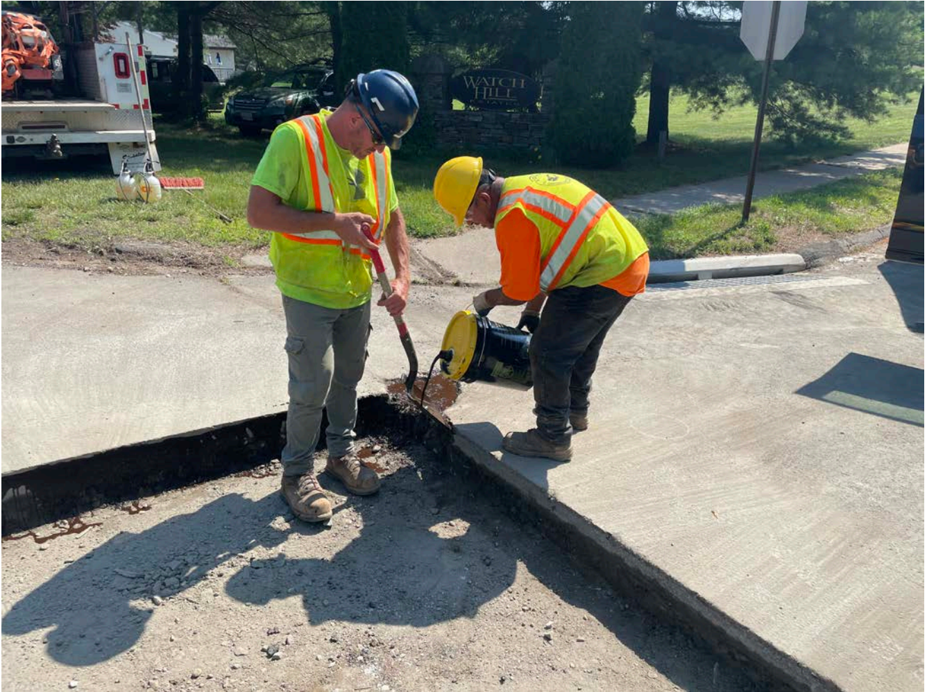
Picture 4: Ludlow placing tack coat on the edges of cut pavement as part of permanent paving activities at the intersection of Talcott Ridge Drive and S. Main Street, Middletown. View to the southwest.
