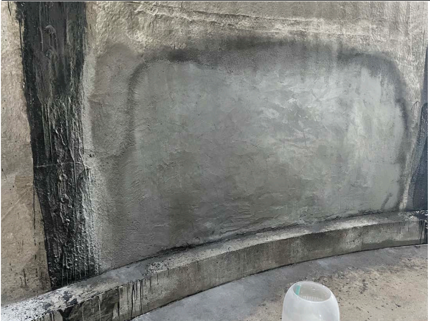
Picture 5: Non-shrink grout that DN Tanks mortared over the repaired portion of the water tank where a temporary access was once located. View to the east.
