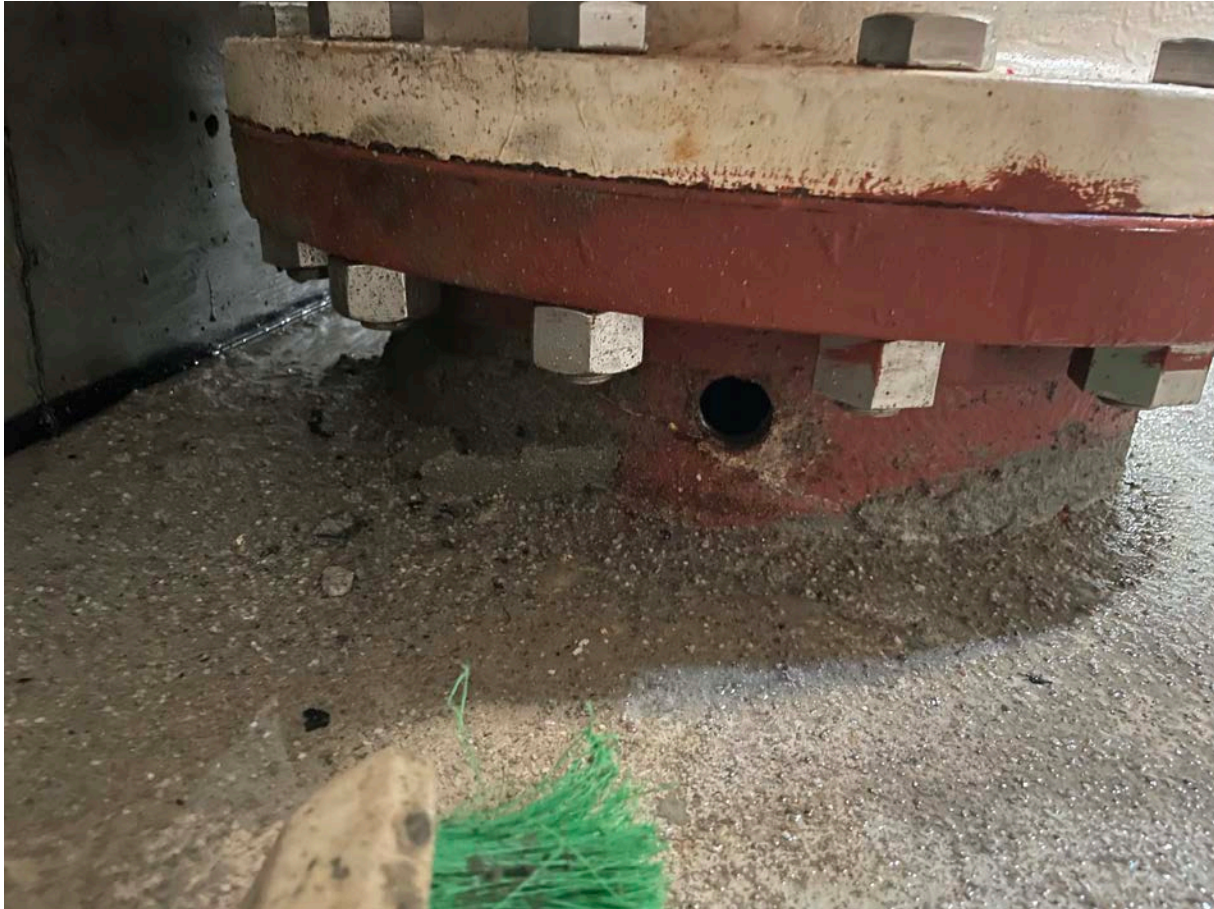
Picture 6: Hole left in the base of the inlet of the water tank where Ludlow removed a 1" stub used for pressure testing. DN Tanks stated that this hole will not be capped. View to the west.
