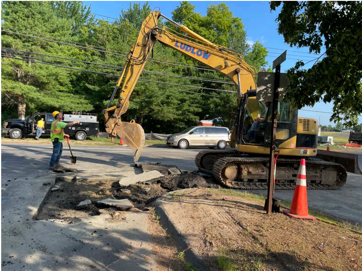
Picture 1: Ludlow removing asphalt from a trench cut overcut at the intersection of Talcott Ridge Drive and S. Main Street, Middletown. View to the west.
