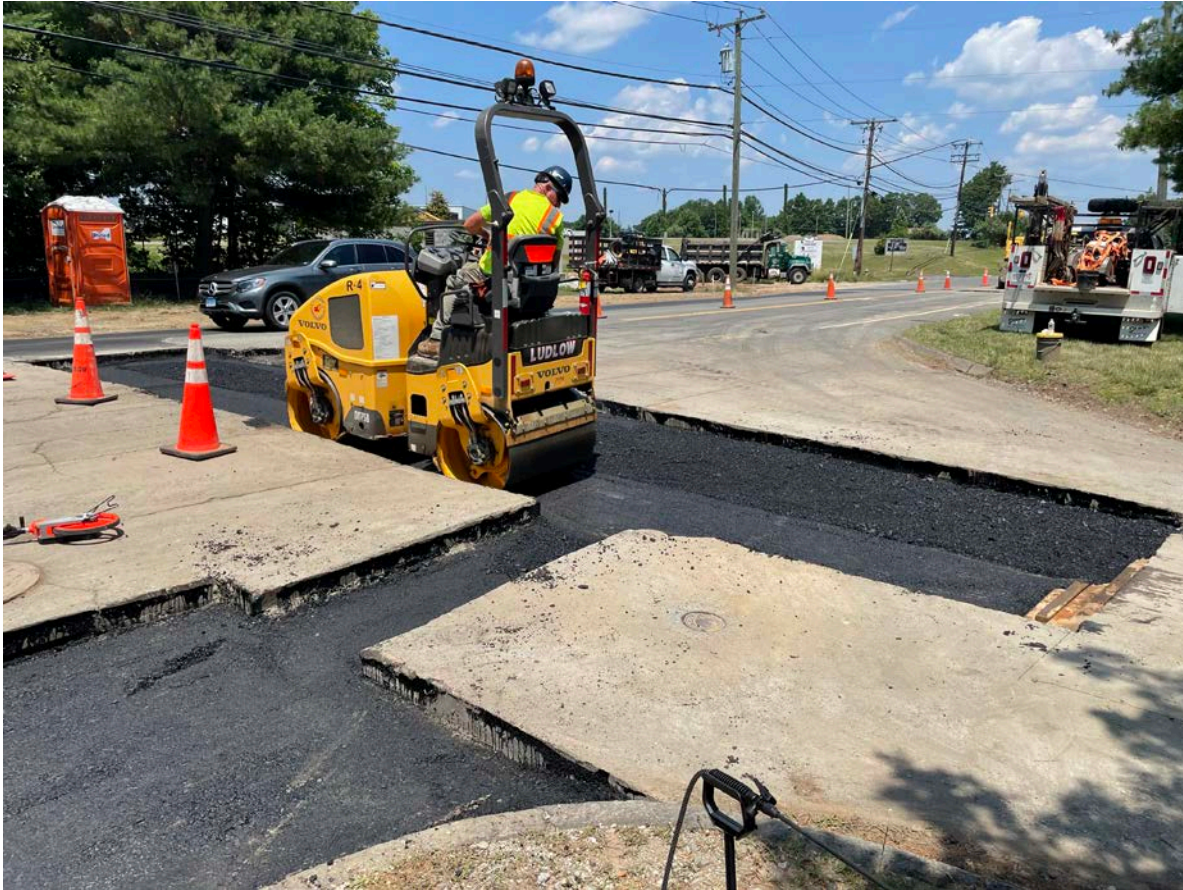
Picture 9: Ludlow rolling the first lift of asphalt on trench overcuts on the northbound lane of S. Main Street, Middletown. View to the north.
