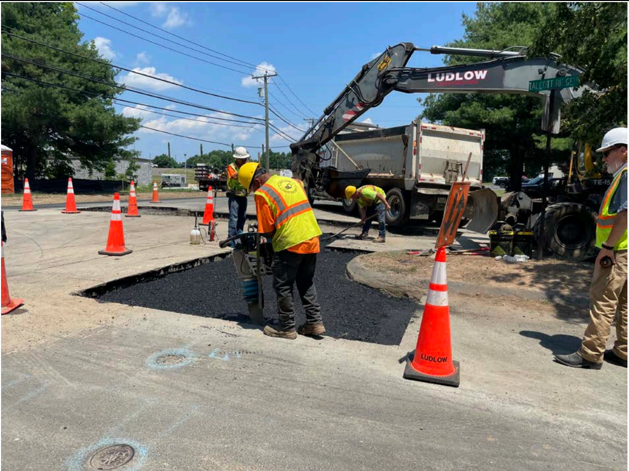
Picture 7: Ludlow using a jumping jack to compact asphalt along the edge of a trench overcut on S. Main Street as part of permanent paving activities. View to the north.
