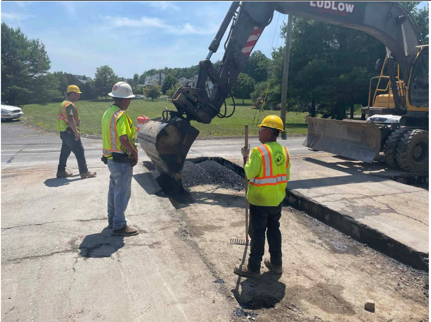
Picture 5: Ludlow placing the first lift of asphalt on trench overcuts on S. Main Street near Station ~700+00 in Middletown. View to the east.
