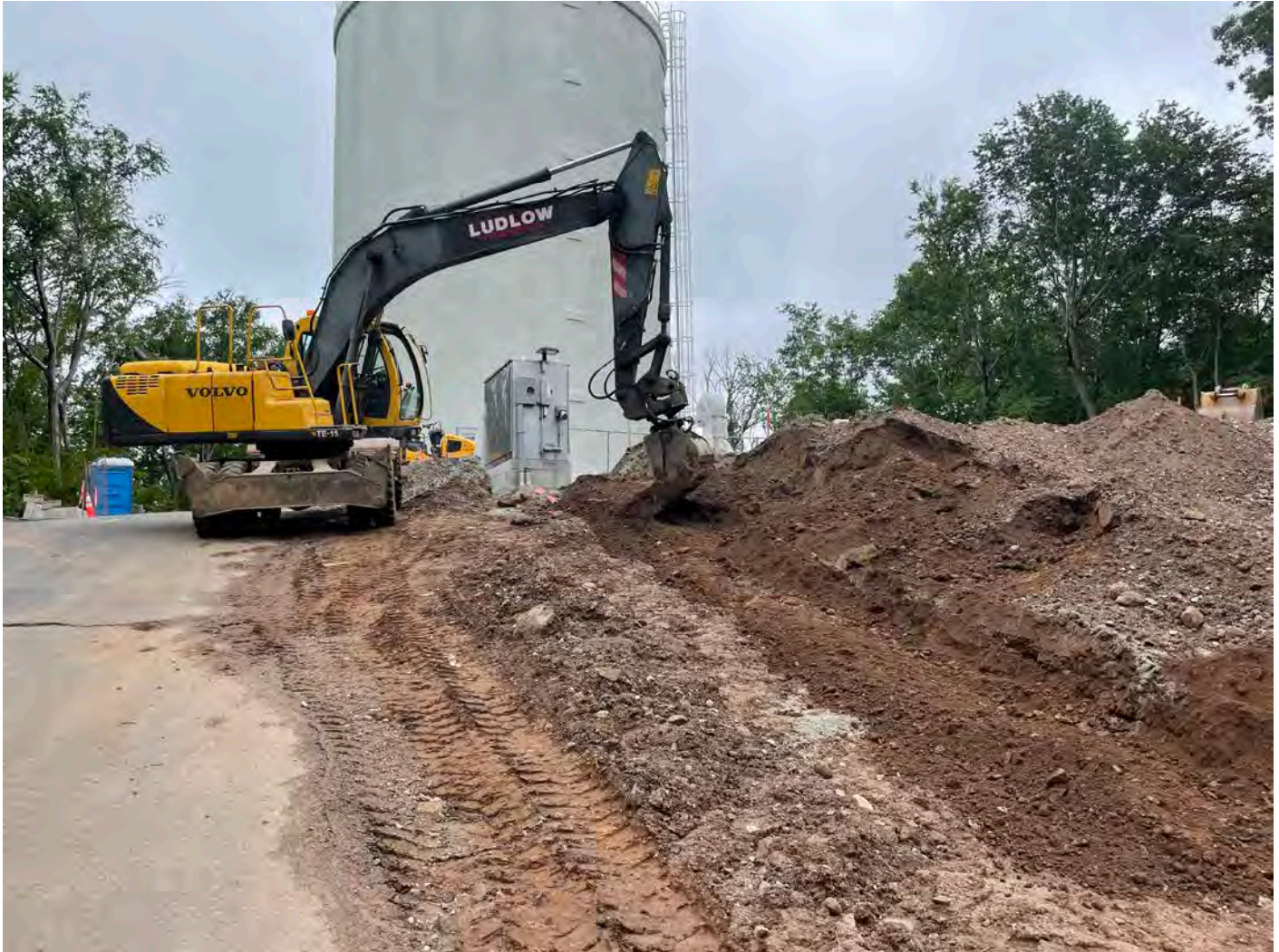
Picture 8: Ludlow placing backfill over electrical and communications conduits in the utility trench located south of the Shared Access Driveway in Middletown. View to the east.
