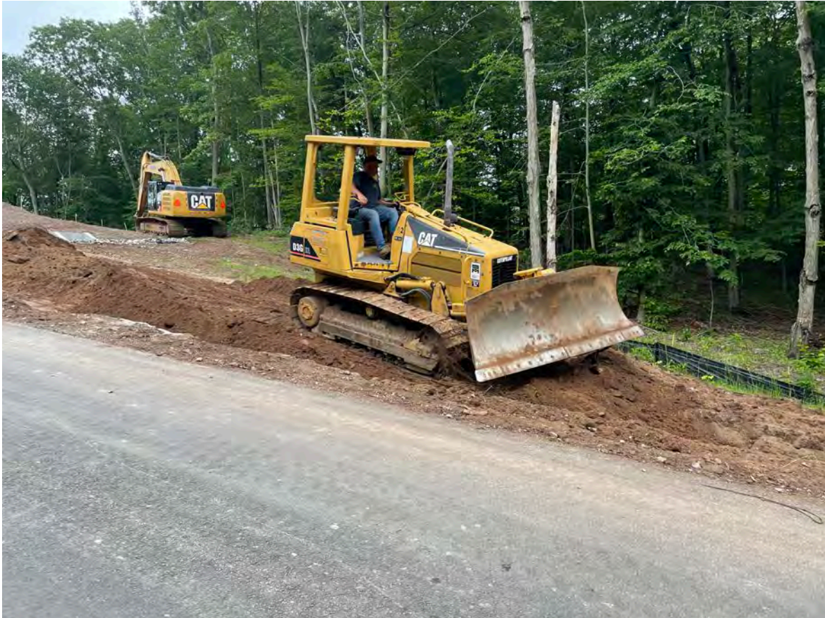
Picture 9: Ludlow grading backfill that they placed over electrical and communications conduits in the utility trench located south of the Shared Access Driveway in Middletown. View to the southeast.
