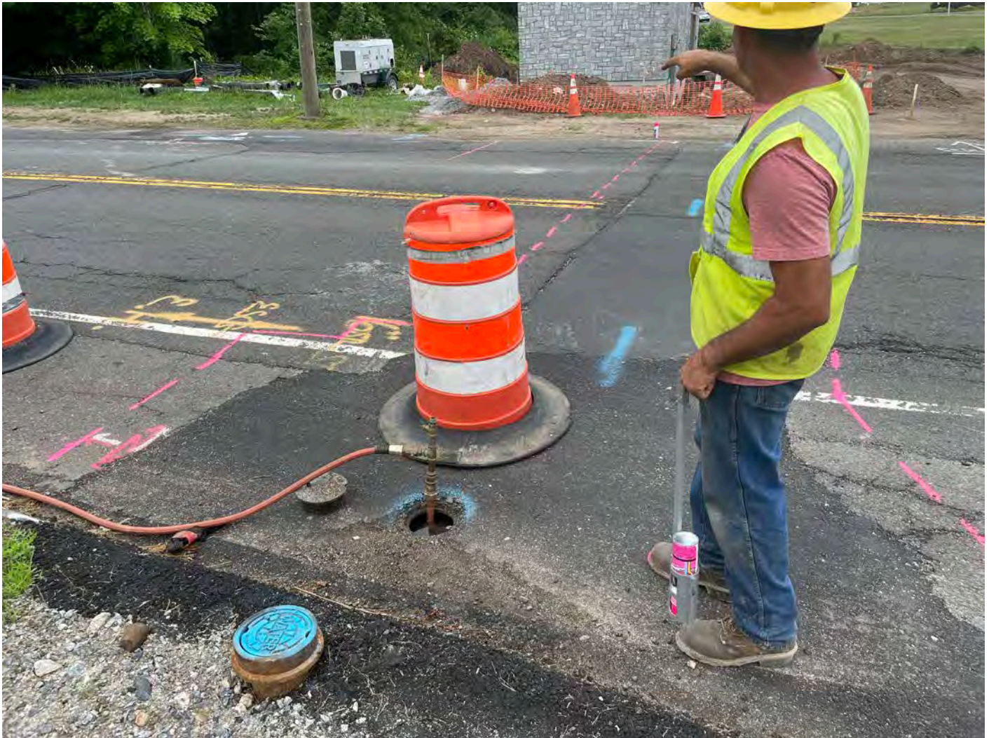
Picture 11: Ludlow flushing an 8" water line that is located on a portion of Talcott Ridge Drive and on the booster station property. View to the west.
