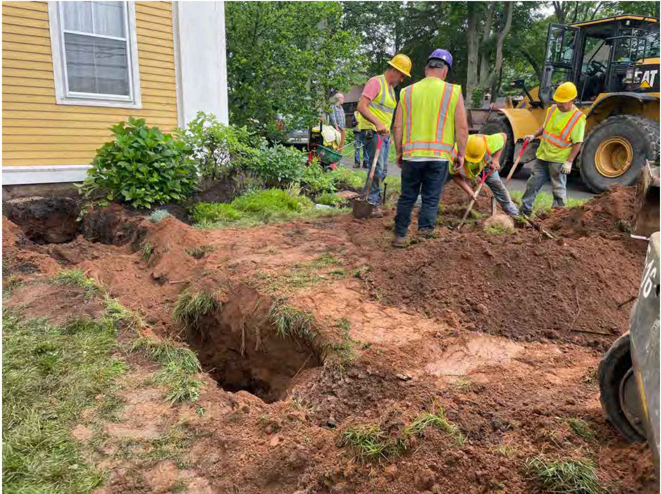
Picture 3: Ludlow hand digging on the northeast corner of the 202 Main Street residence to daylight a 4" PVC line that runs from the home's septic tank to its leach field. The trench that Ludlow started to excavate to place a 1" copper water service line through the east side of the home's foundation is visible on the left. View to the northwest.
