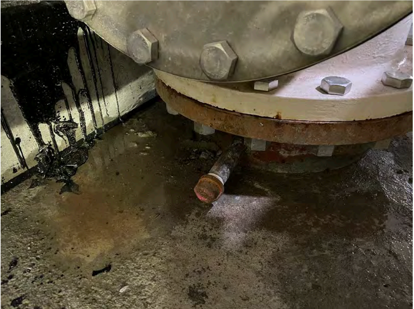
Picture 4: Short pipe nipple located at the base of the inlet pipe of the water tank that Ludlow installed to assist in pressure testing the pipes associated with the water tank. The removal of this nipple and cap is on the punch list of items to be finished at the water tank. View to the southwest.
