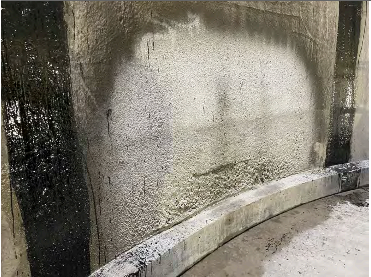
Picture 5: Patched area of the inside of the water tank where a temporary entrance was removed and sealed. Smoothing of the shotcrete surface with additional repair mortar is on the punch list of items to be finished at the water tank. View to the east.
