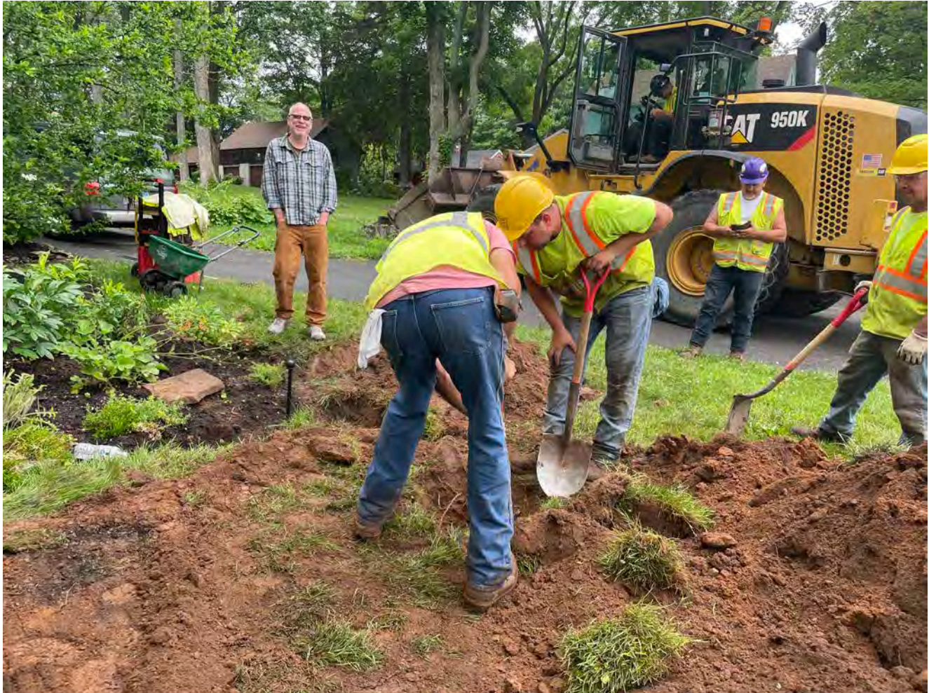
Picture 2: Ludlow hand digging on the northeast corner of the 202 Main Street residence to daylight a 4" PVC line that runs from the home's septic tank to its leach field. View to the northwest.
