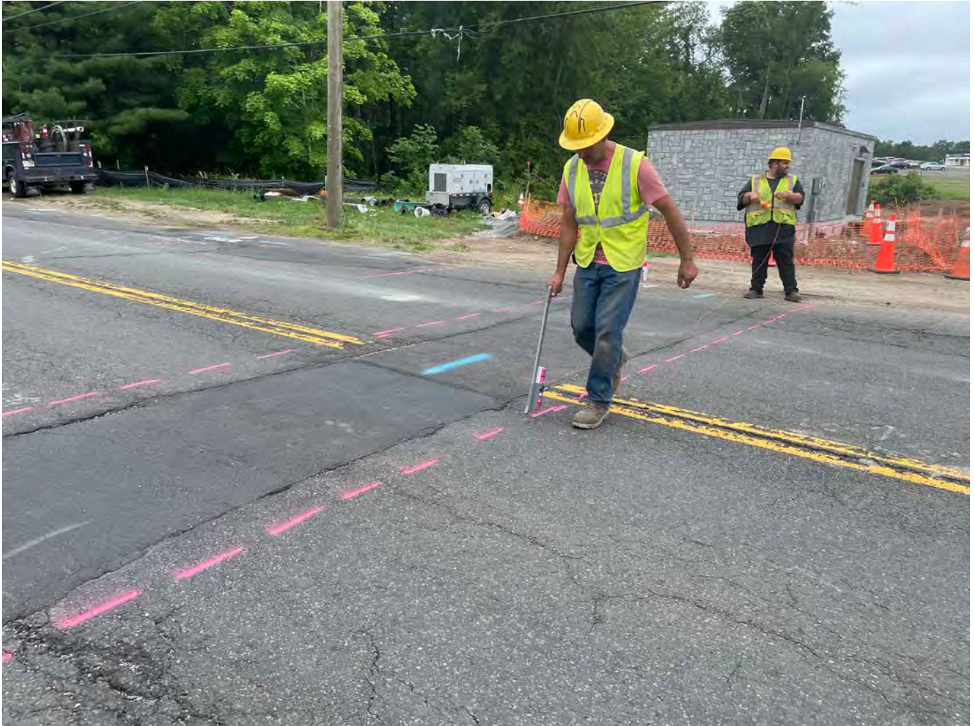
Picture 10: Ludlow marking out trench overcuts for permanent paving activities that will be performed on Monday. S. Main Street at ~Station 700+00. View to the east.
