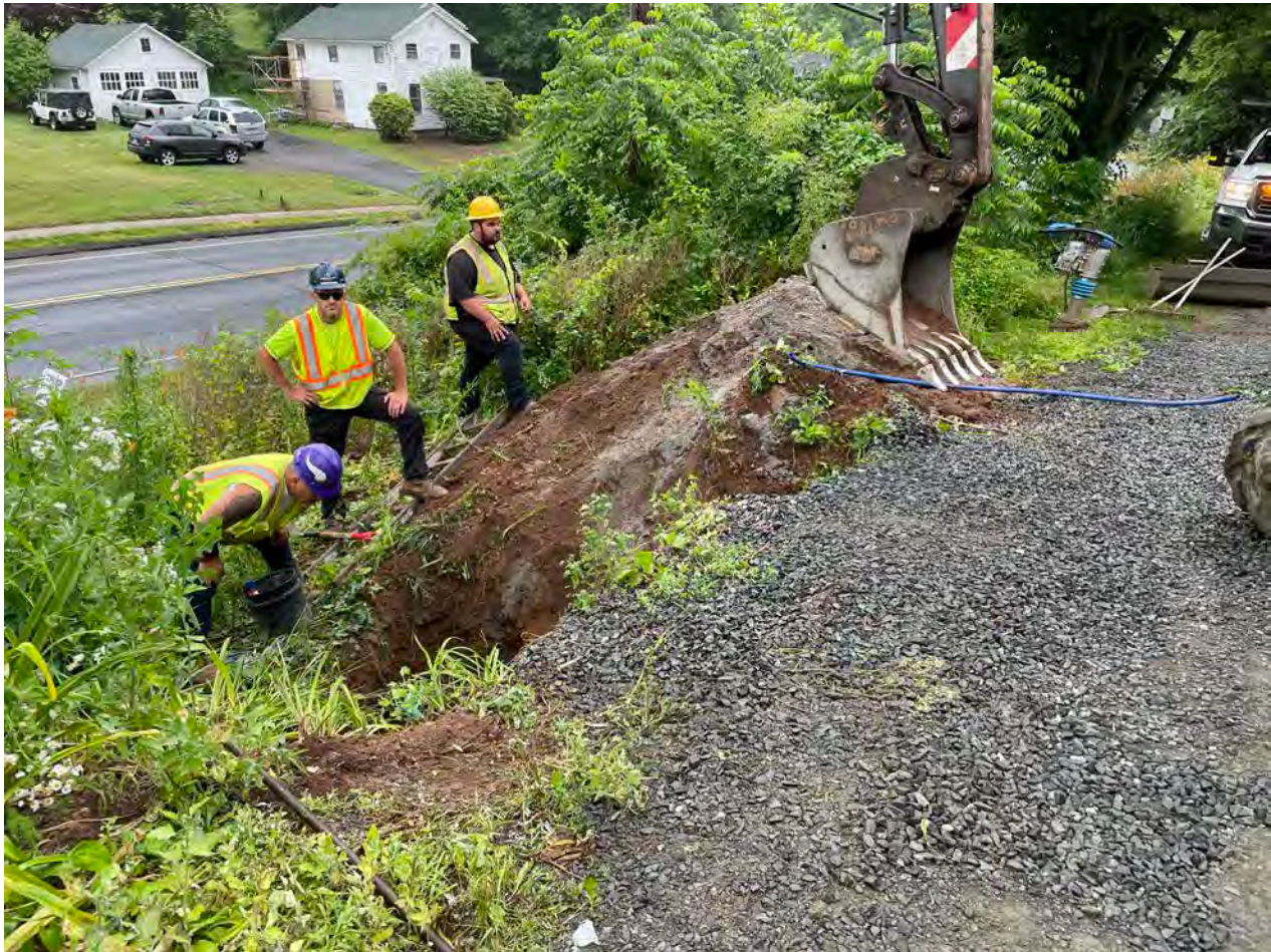
Picture 1: Ludlow excavating at the curb stop for 174 Main Street as the work to connect a section of 1" copper pipe that was previously installed at the residence to the curb stop. View to the southeast.
