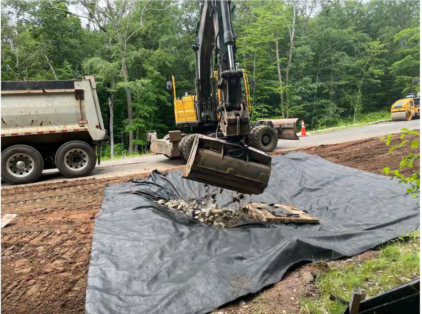
Picture 12: Ludlow placing riprap over geofabric that has been placed around a catch basin located south of the Shared Access Driveway at ~Station 13+20. View to the north.
