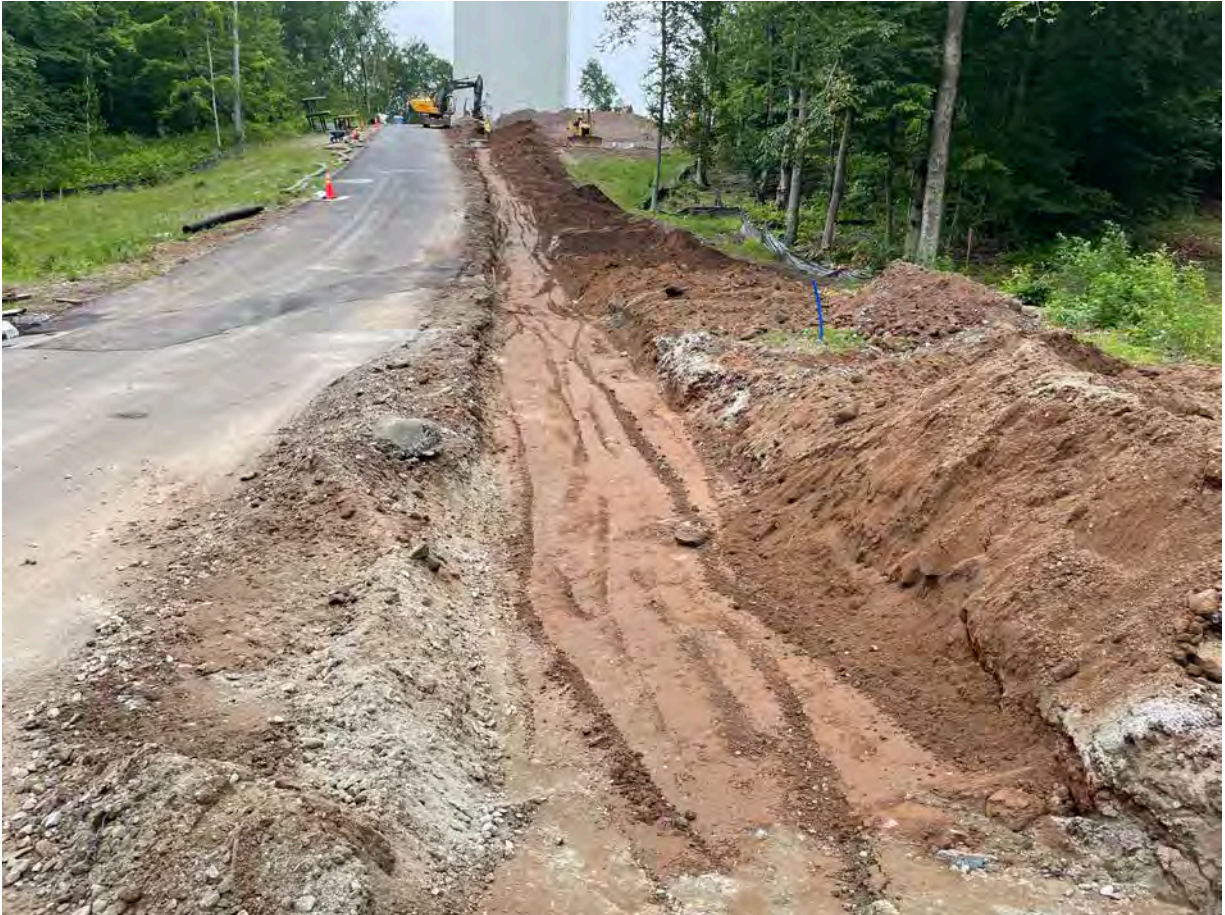
Picture 7: Backfill that Ludlow placed and compacted over electrical and communications conduits in the utility trench located south of the Shared Access Driveway in Middletown. View to the east.
