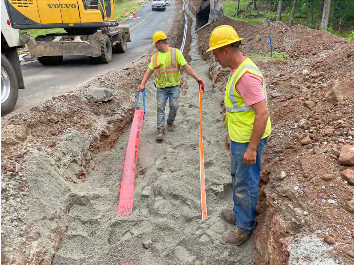
Picture 6: Ludlow placing caution tape over electrical and communications conduits in the utility trench located south of the Shared Access Road in Middletown. View to the east.
