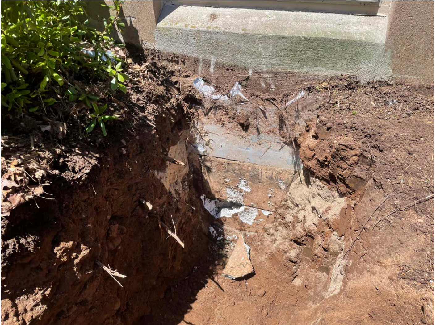
Picture 8: Penetration point on the south side of the foundation for the building at 201 Main Street for the installation of a 1" copper water service line. View to the north.
