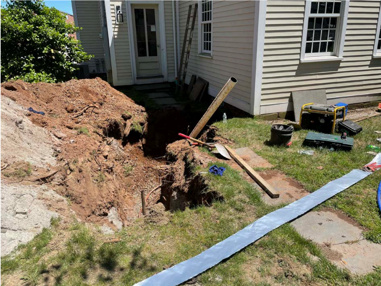
Picture 6: View of the installation of a 1" copper water service line for the building at 199 Main Street, Durham. View to the southeast.
