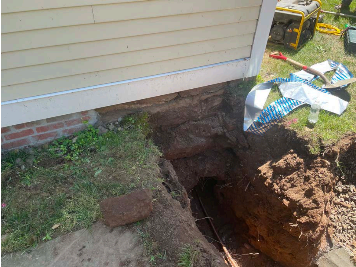
Picture 9: North-facing foundation of the building at 199 Main Street, Durham where Ludlow inserted a 1" copper water service line. View to the southwest.
