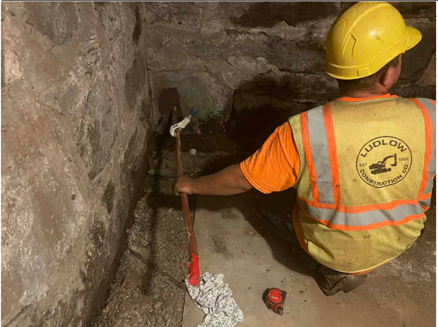
Picture 5: Ludlow pulling 1" copper water service line through the penetration that was made through the foundation of the 199 Main Street building on the north side (next to the northwest corner of the foundation). View to the north.
