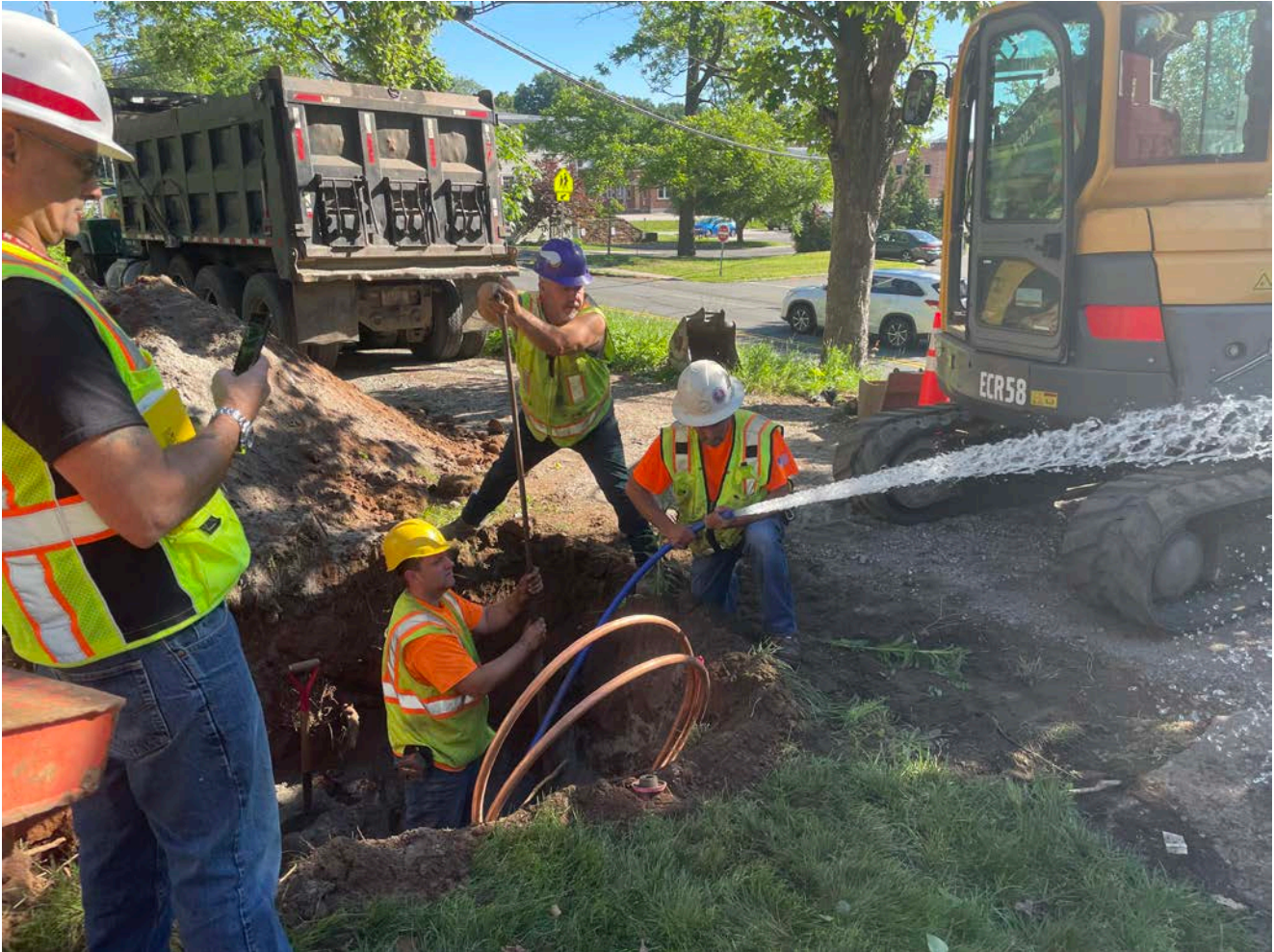
Picture 2: Ludlow purging the curb stop at 188 Main Street, Durham, before attaching a 1" copper water service line to it. View to the northeast.
