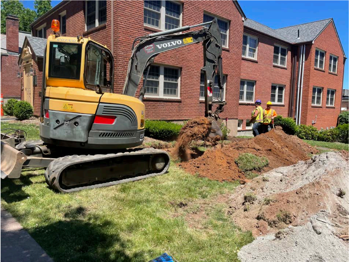
Picture 7: Ludlow excavating for the installation of a 1" copper water service line on the south side of the 201 Main Street building. View to the northeast.
