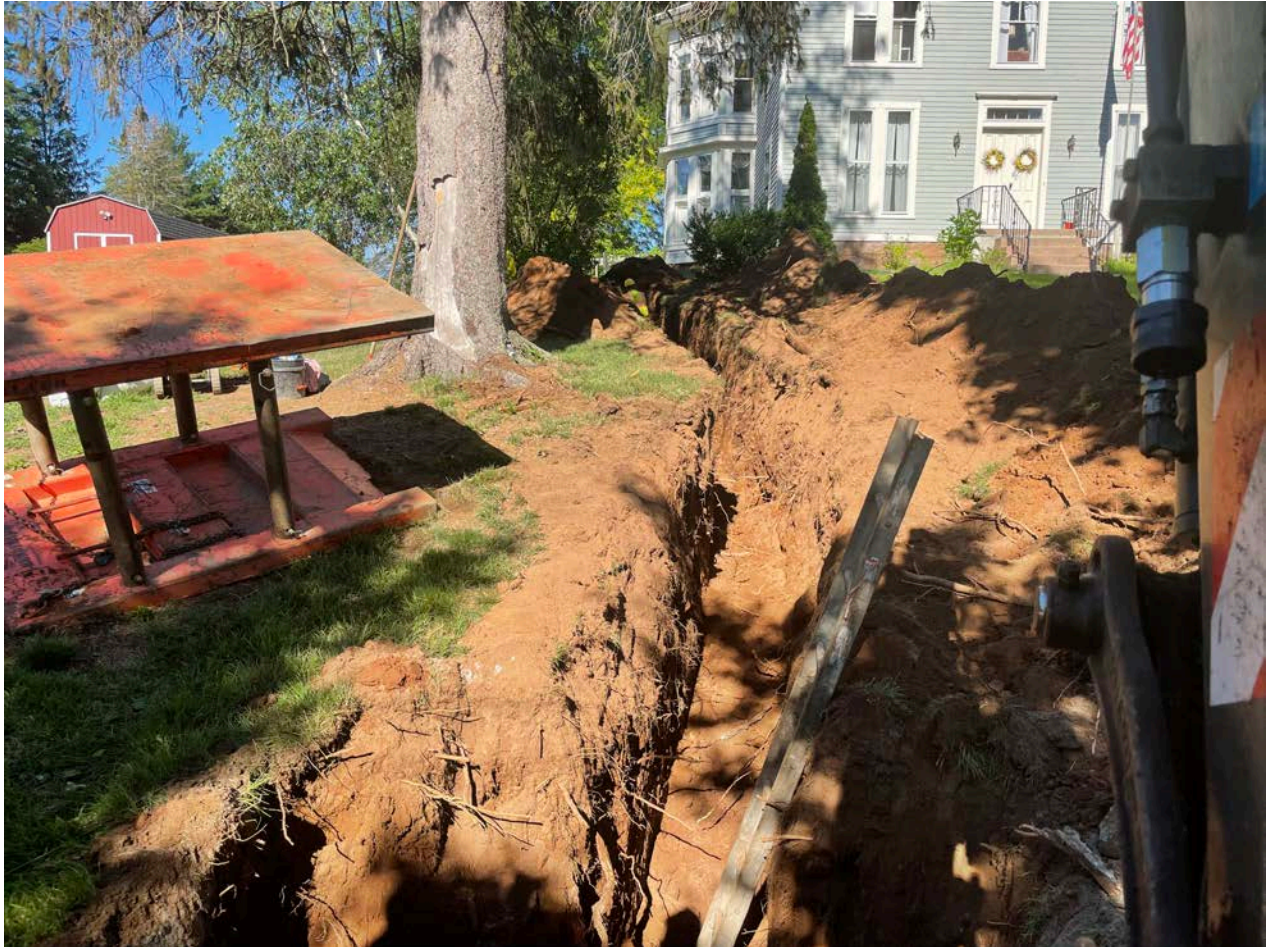
Picture 1: Trench excavated for the Installation of a 1" copper water service line at the 188 Main Street residence. View to the west.
