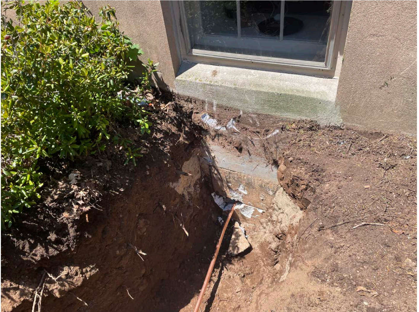
Picture 11: 1" copper water service line that has been fed through the penetration that was made on the south wall of the foundation for the 201 Main Street. View to the north.
