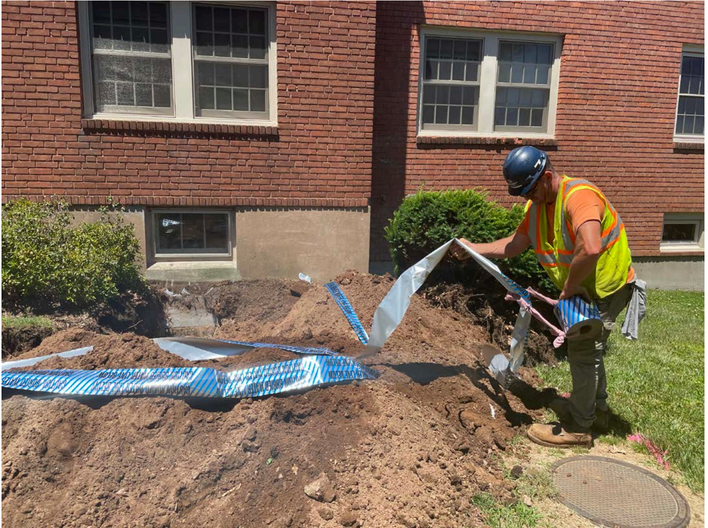
Picture 10: Ludlow laying out caution tape to place over 1" copper water service line that Ludlow installed for the building at 201 Main Street, Durham. View to the north.
