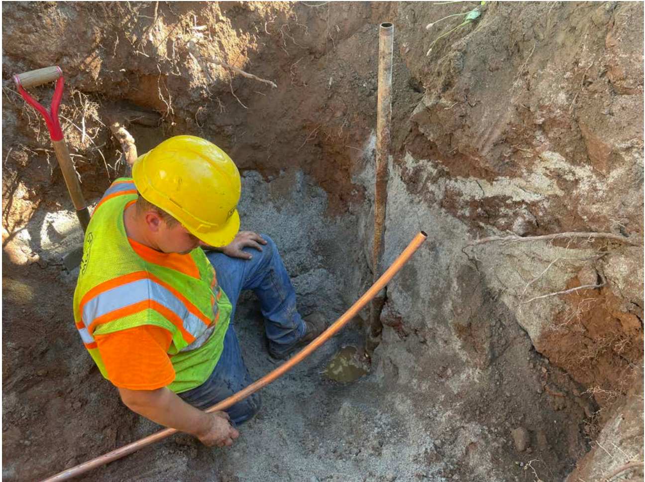
Picture 3: Ludlow preparing to connect 1" copper water service line to the curb stop for 188 Main Street, Durham. View to the northeast.
