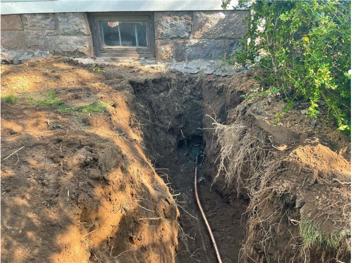
Picture 4: 1" copper water service line that has penetrated the south side of the foundation of the residence at 188 Main Street in Durham. View to the north.
