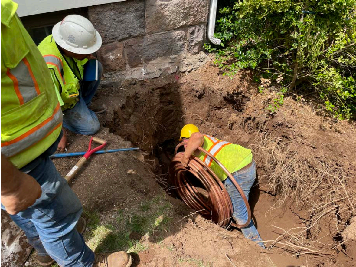
Picture 9: Ludlow inserting a 1" copper water service line through the south wall of the foundation of the 188 Main Street residence next to the southeast corner of the building. View to the northwest.
