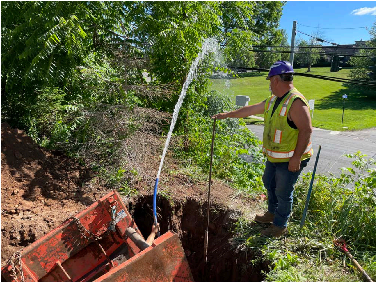
Picture 3: Ludlow purging the curb stop at 176 Main Street for the installation of a 1" copper water service line. View to the northwest.
