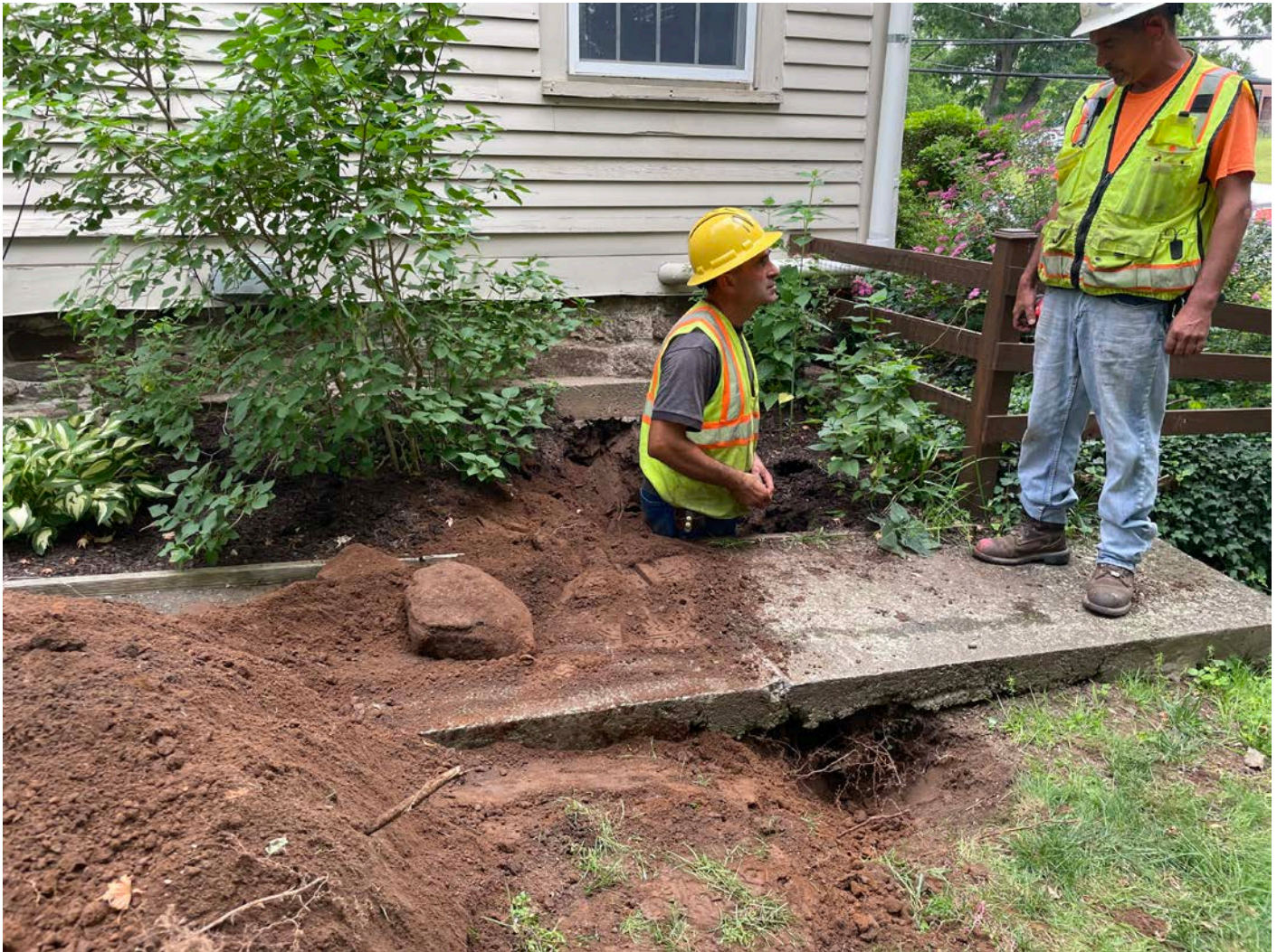
Picture 8: Ludlow in the process of hand-excavating on the south side of the foundation at the 168 Main Street residence for the installation of a 1" copper water service line. View to the northeast.
