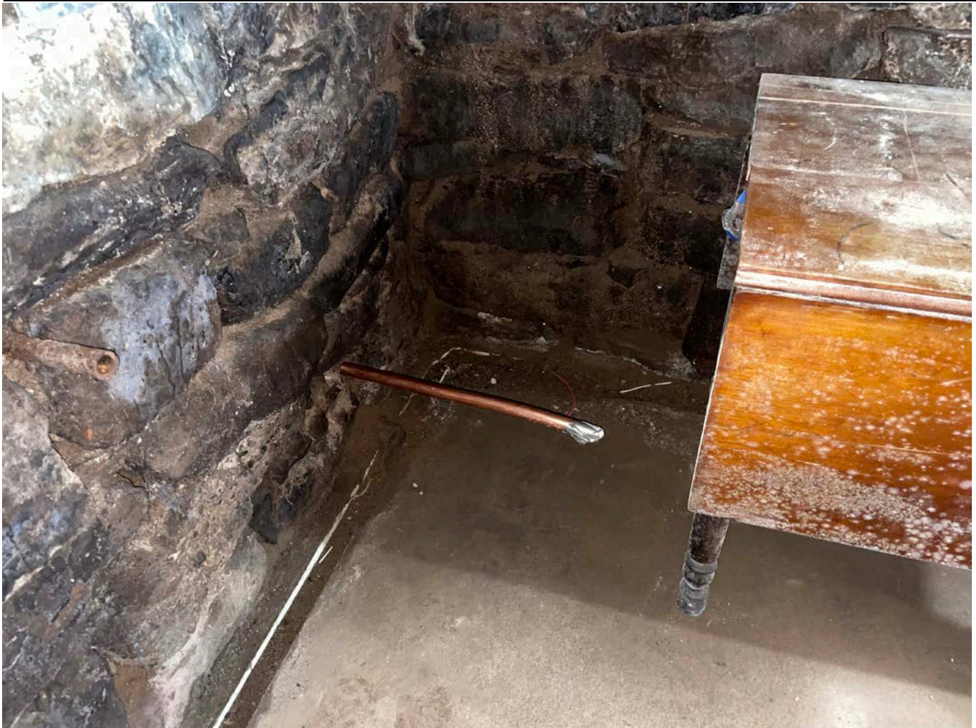
Picture 5: The west wall of the foundation for 167 Main Street and the 1" copper water service line that has penetrated the foundation. View to the north.
