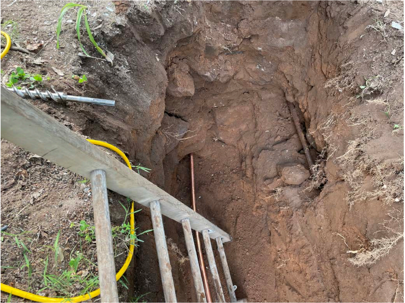
Picture 4: 1" copper water service line that has penetrated the western foundation of the residence at 167 Main Street in Durham. View to the east.
