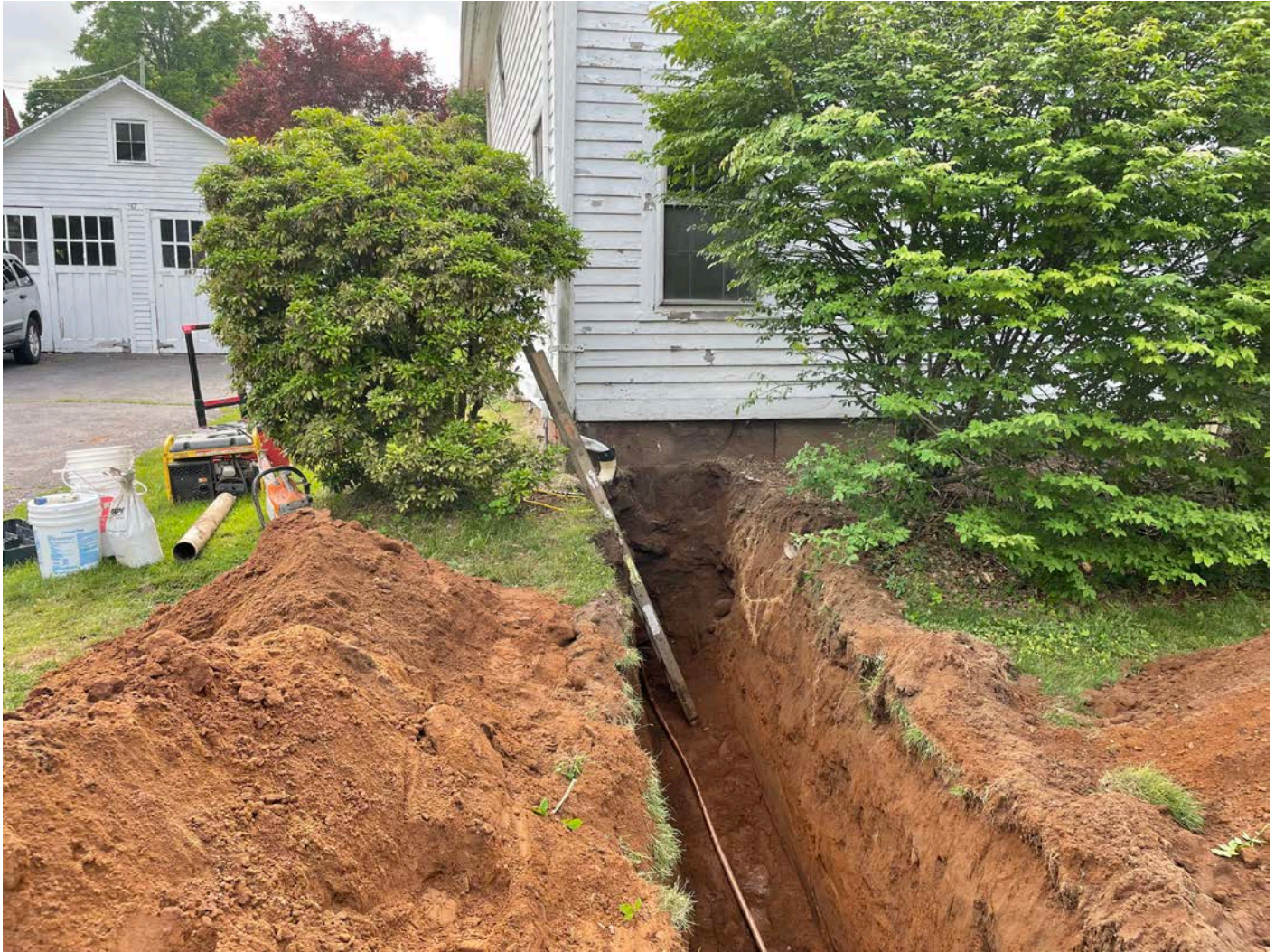
Picture 10: View of 1" copper water service line that Ludlow advanced through the west wall of the residence at 167 Main Street, Durham. View is to the east.
