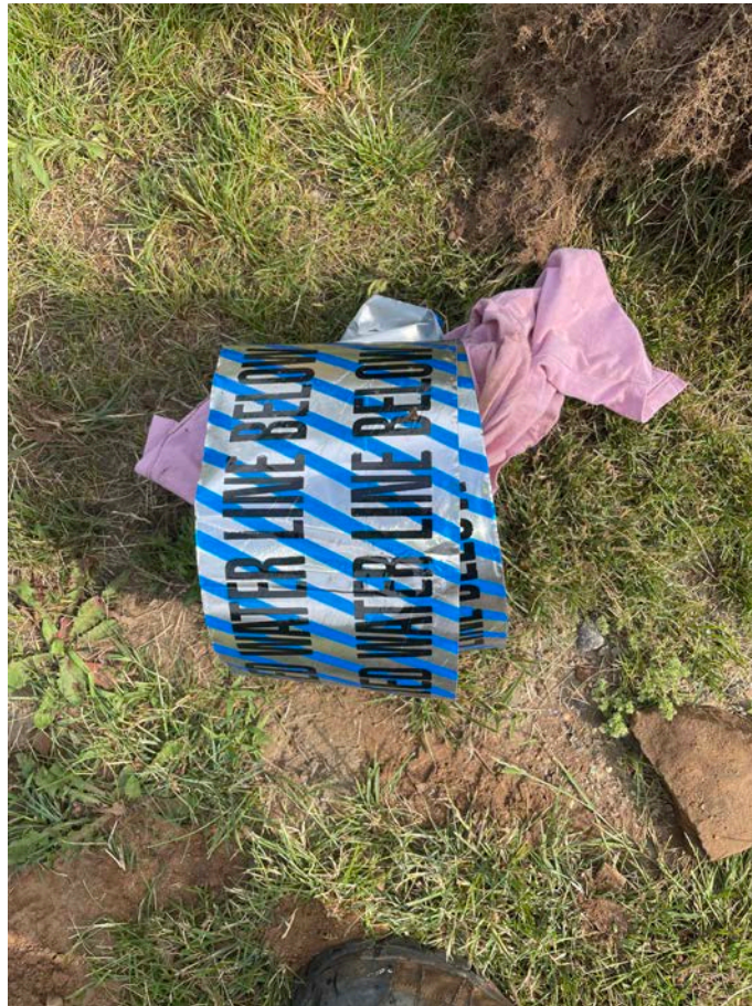
Picture 7: Caution tape that Ludlow is placing over the 1" copper water service lines they have been installing between homes and their associated curb stops.
