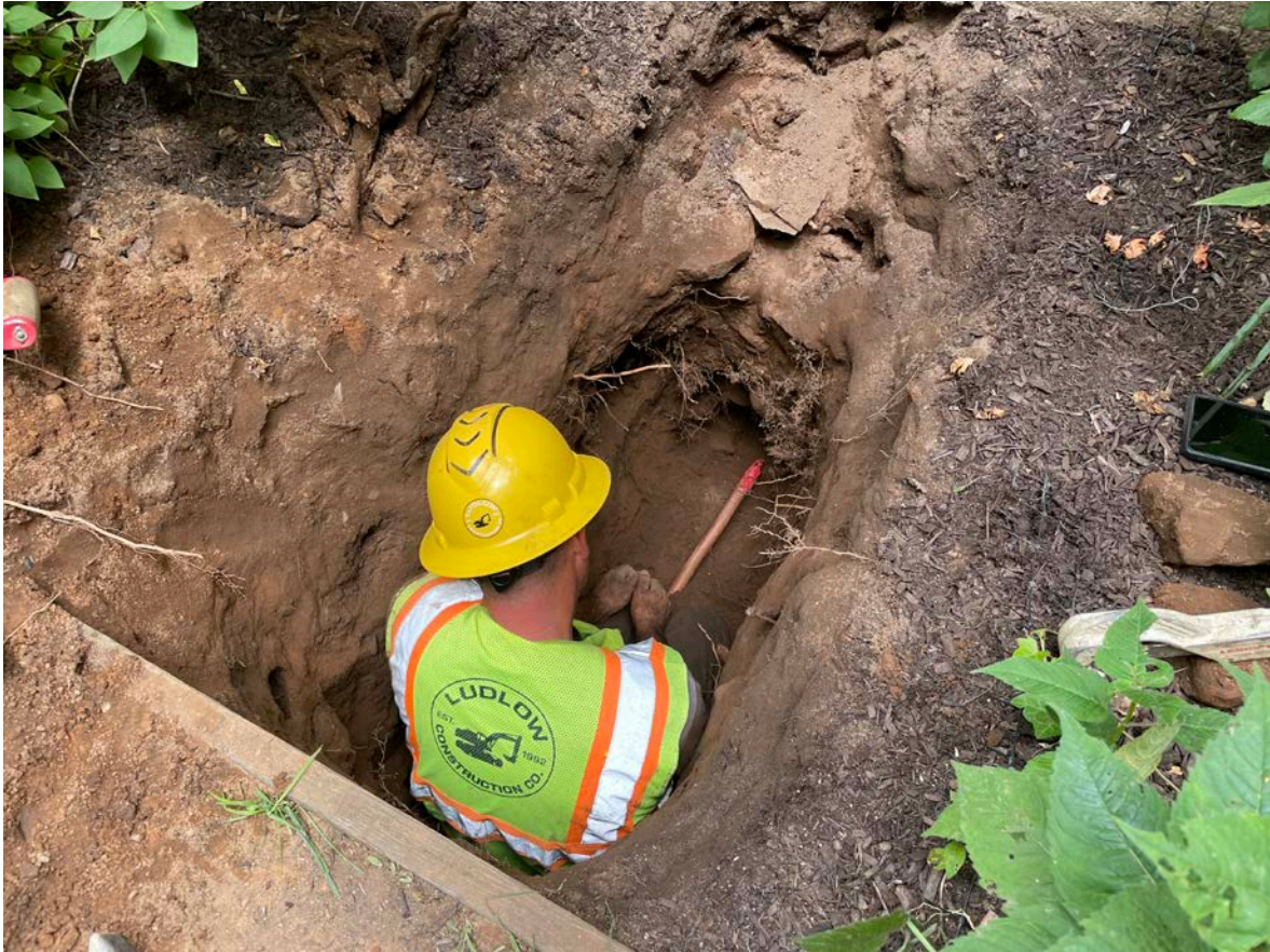
Picture 9: Ludlow inserting a 1" copper water service line through the south wall of the foundation of the 168 Main Street residence. View to the northwest.
