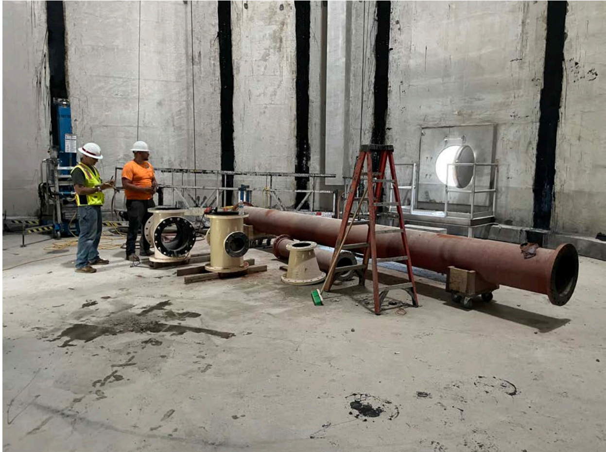
Picture 1: Materials that will be placed today by DN Tanks as they install the inlet pipe on the inside of the water tank located east of the Shared Access Driveway in Middletown. View to the southwest.
