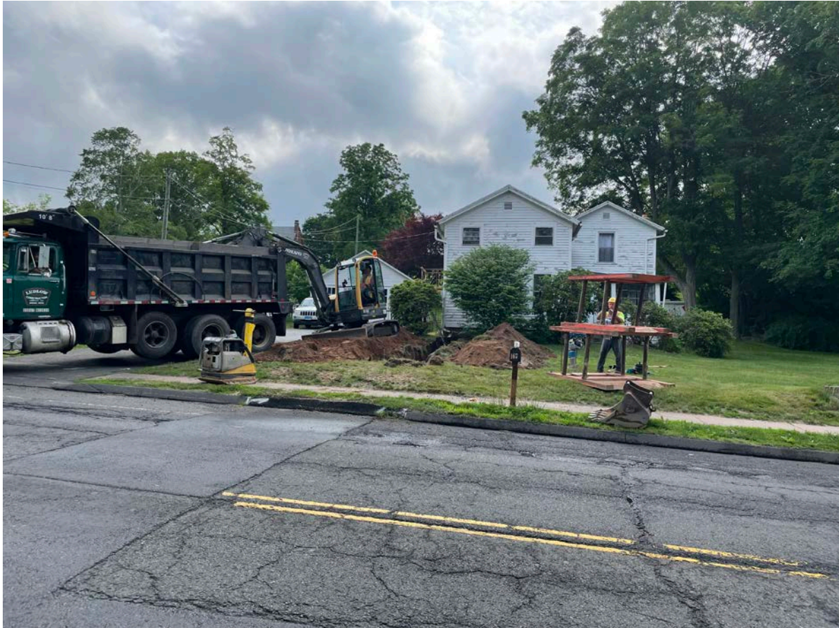
Picture 6: Overview of the installation of a 1" copper water service line at the residence of 167 Main Street in Durham. View to the east.
