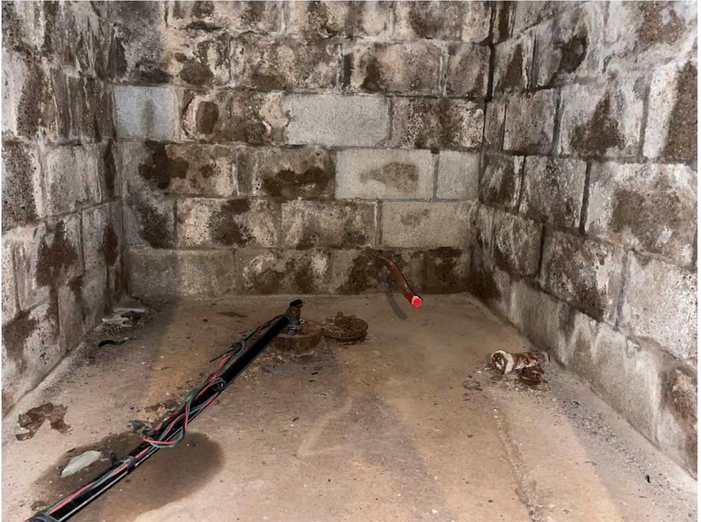
Picture 10: 1" water copper service line that Ludlow advanced through the west wall of the jog out located on the west side of the foundation of the residence at 127 Main Street, Durham. View is to the west, from the interior of the residence.
