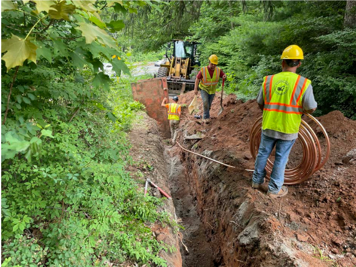
Picture 7: Ludlow placing 1” copper water service line in the trench they have excavated at 127 Main Street between the curb stop and the west side of the residence’s foundation. View to the north.
