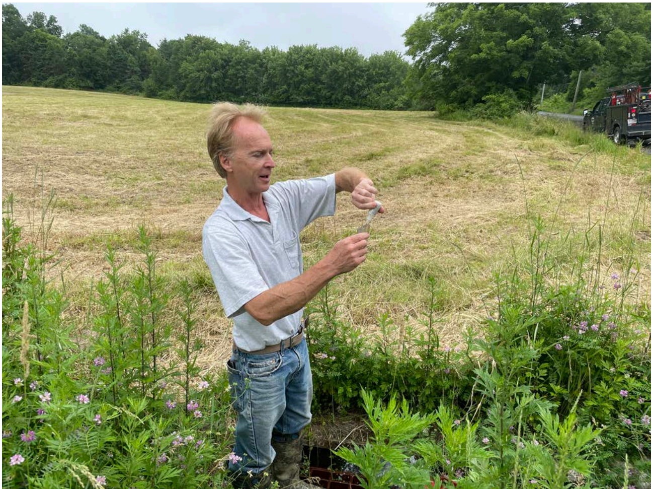
Picture 3: JMS testing for chlorine in the section of the water line they dechlorinated today on Maiden Lane. View to the north.
