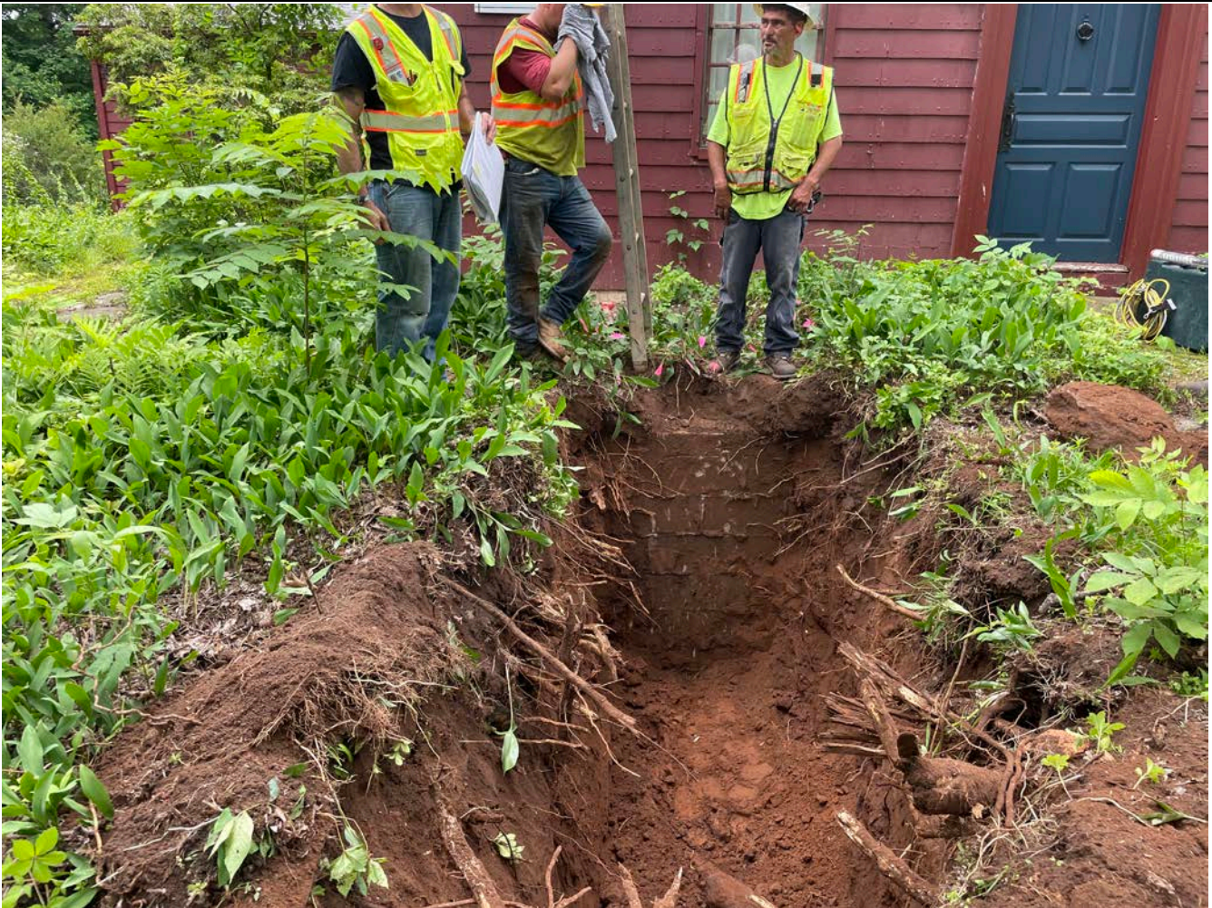
Picture 4: Ludlow has daylighted the jog out located on the west side of the residence at 127 Main Street, Durham. The west wall of the jog out was later penetrated for the insertion of a 1" copper water service line. View to the east.
