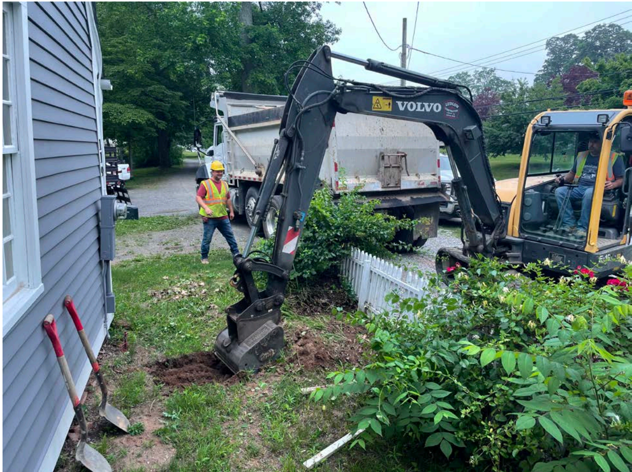
Picture 1: Ludlow begins excavating for the installation of a 1" copper water service line on the west side of the residence at 120 Main Street, Durham. View to the south.
