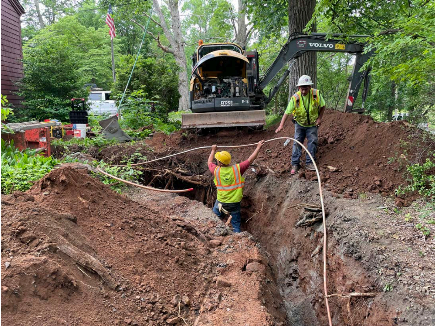
Picture 8: Ludlow placing 1” copper water service line in the trench they have excavated at 127 Main Street between the curb stop and the west side of the residence’s foundation. View to the south.
