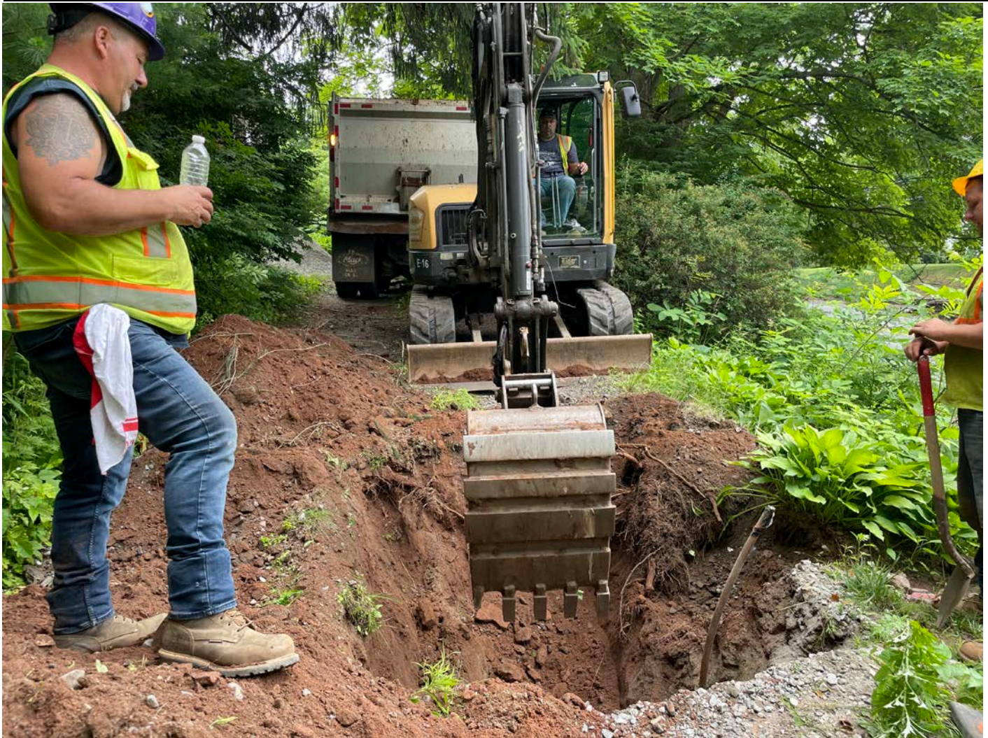
Picture 5: Ludlow excavating a trench from the curb stop at 127 Main Street, Durham, to the western foundation of the residence. View to the south.
