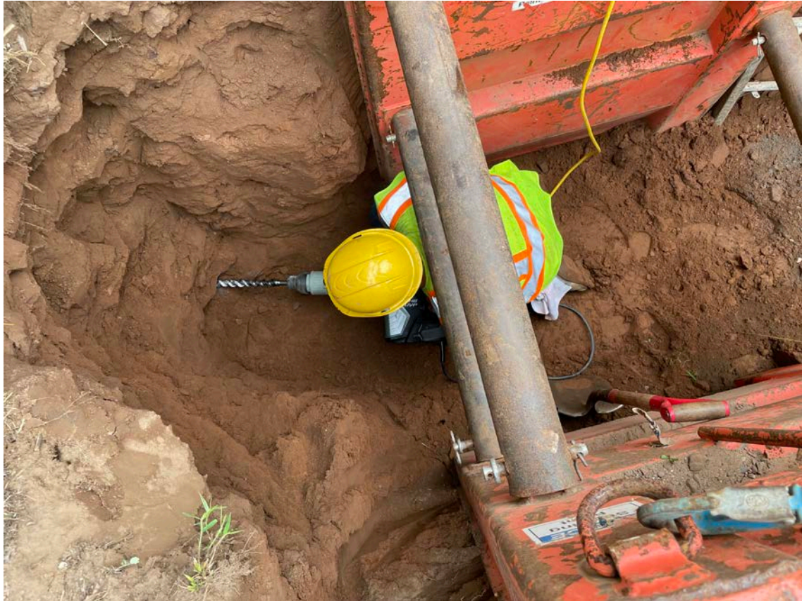
Picture 2: Ludlow begins to drill through the fieldstone foundation of the residence at 120 Main Street, Durham, for the installation of a 1" copper water service line.
