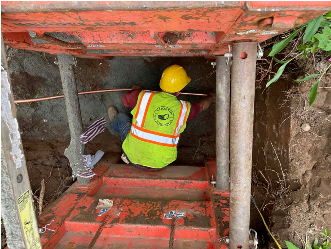
Picture 9: Ludlow inserting a 1" copper water service line through the west wall of the jog out located on the west side of the foundation of the residence at 127 Main Street, Durham.
