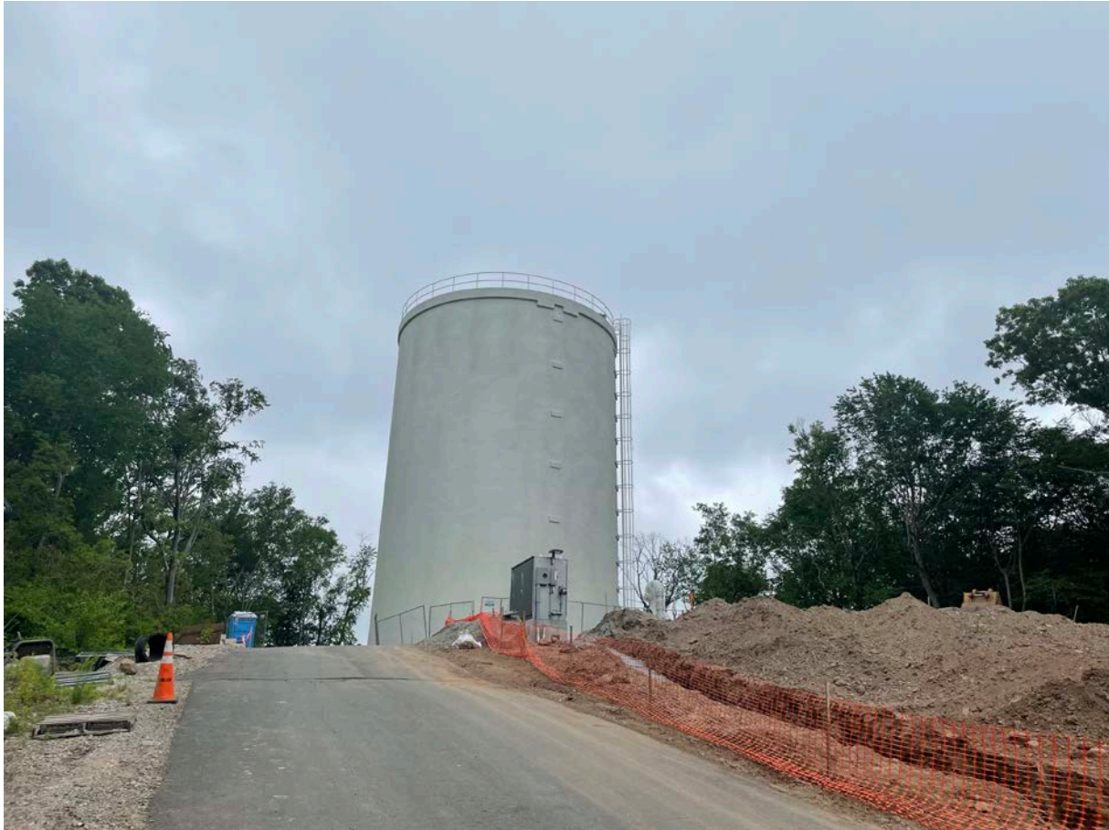
Picture 6: View of the water tank after DN Tanks installed the ladder on the west side of the water tank located east of the Shared Access Driveway in Middletown. View to the east.
