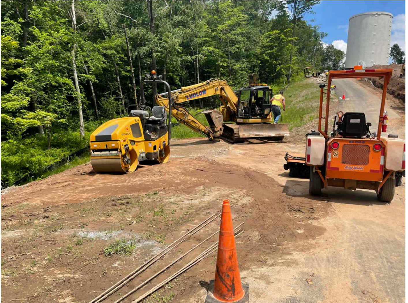
Picture 8: Vehicle turnout located on the north side of the Shared Access Driveway at Station 13+95 where Ludlow is extending it 15' to the north. View to the east.
