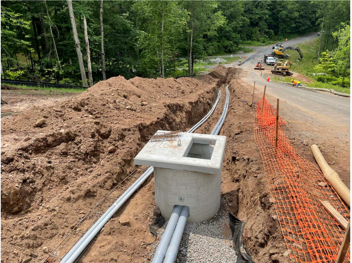
Picture 9: View of progress as A&R Electric place 2" and 4" PVC conduits in the utility trench they are excavating on the south side of the Shared Access Driveway in Middletown. View to the west.
