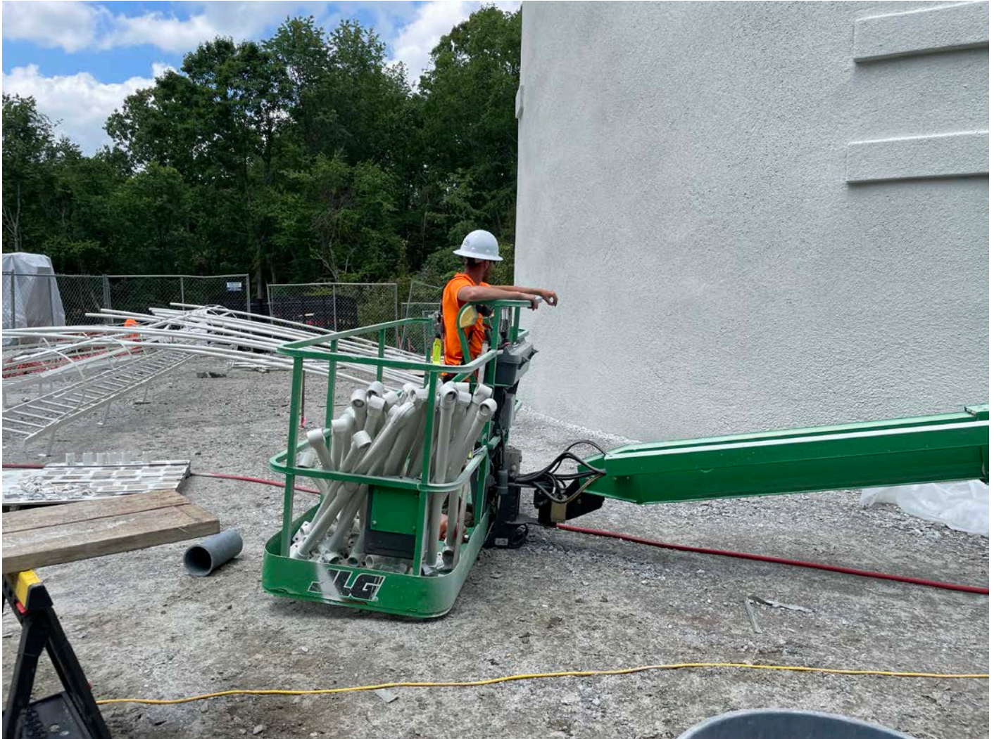
Picture 10: DN Tanks lifting railing components to the top of the water tank for installation.
