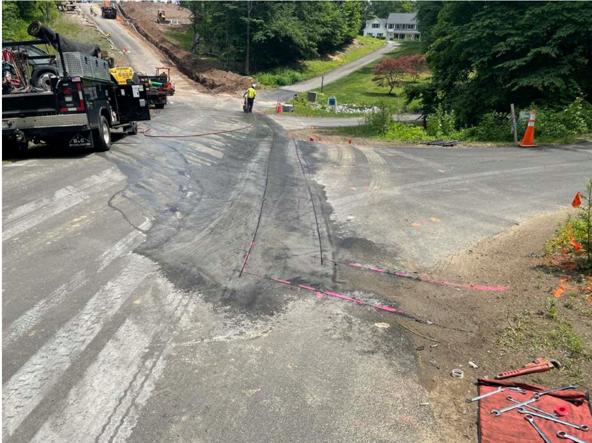
Picture 7: Ludlow saw cutting the footprint for the utility trench in front of the driveways for 214, 216, and 224 Talcott Ridge Drive in Middletown. View to the east.
