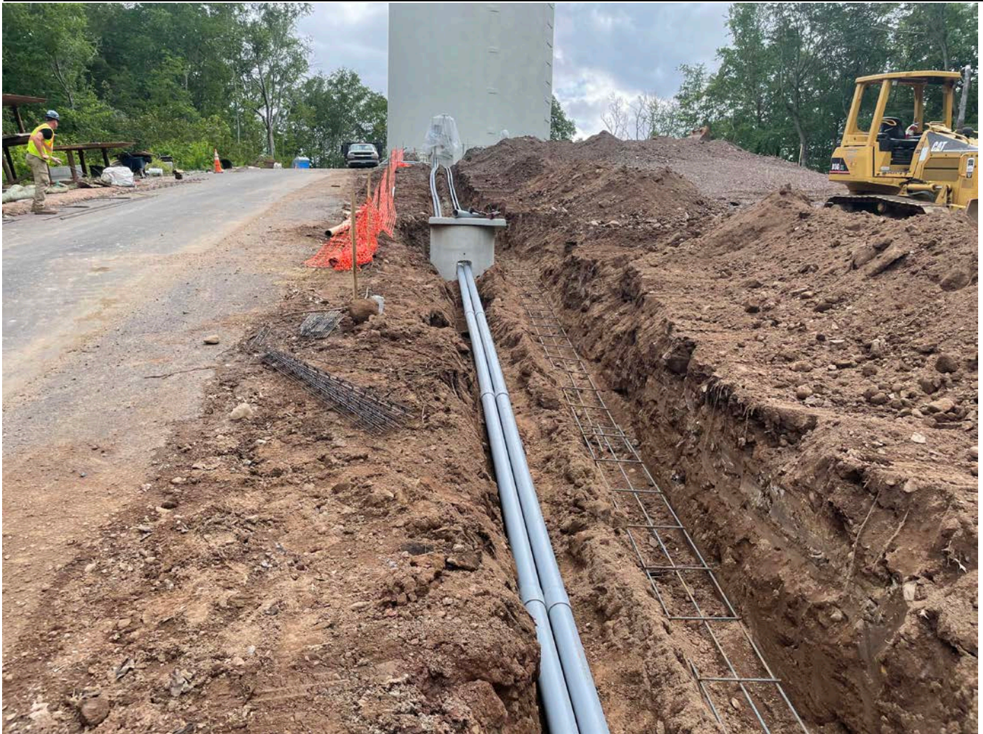
Picture 5: Another view of the PVC conduits and rebar that A&R Electric and Ludlow have placed in the utility trench on the south side of the Shared Access Driveway in Middletown. (Electric power conduits to the left, telephone conduits to the right in this photo) View to the east.
