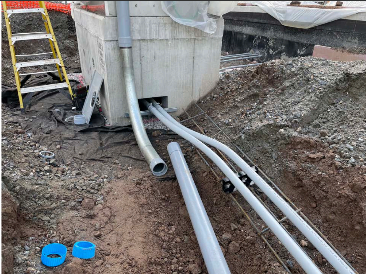
Picture 2: 2" and 4" PVC conduits and the cement vault located at ~Station 11+50 that will house a transformer; all of which are located in the utility trench on the south side of the Shared Access Driveway in Middletown. View to the east.
