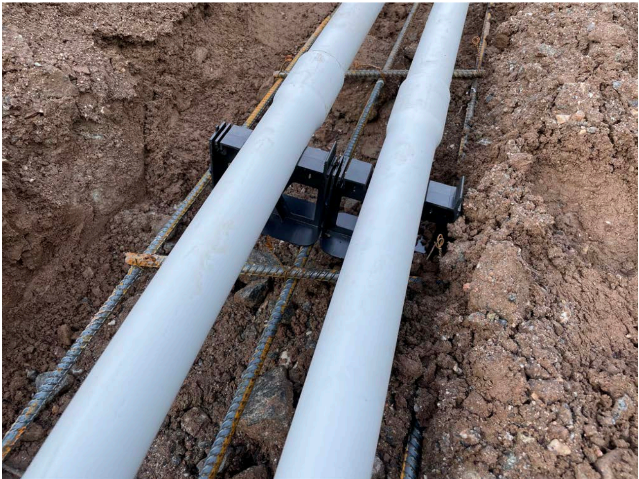
Picture 3: 2" PVC conduit for telephone placed over rebar, with black plastic chairs separating and supporting the PVC, located in the utility trench on the south side of the Shared Access Driveway in Middletown. View to the south.
