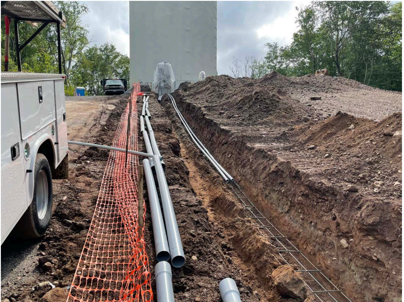
Picture 4: View of PVC conduits that A&R Electric has placed in the utility trench on the south side of the Shared Access Driveway in Middletown. View to the east.
