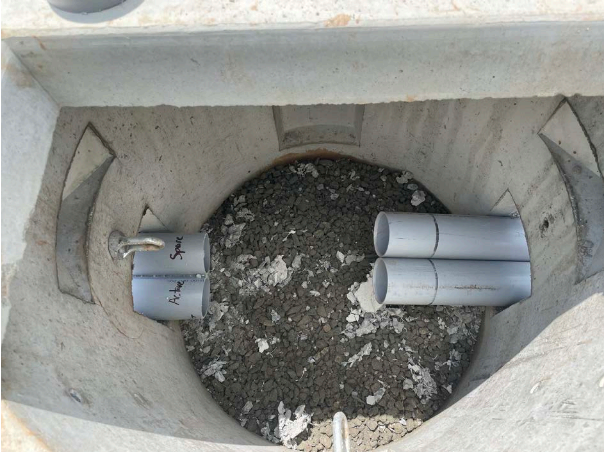
Picture 6: 4" PVC conduit entering and exiting the concrete transformer pad located at ~Station 11+50 that will house a transformer.
