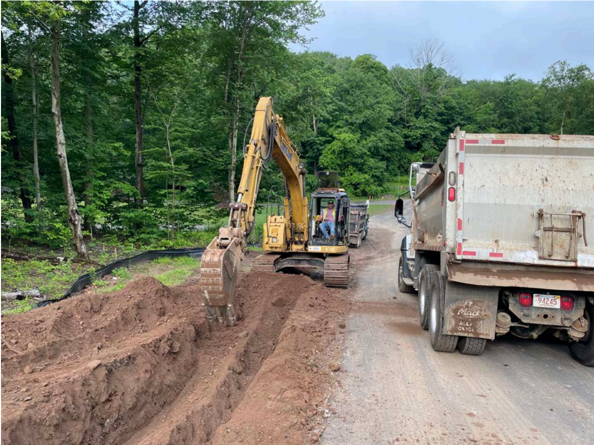
Picture 1: Ludlow excavating a utility trench on the south side of the Shared Access Driveway in Middletown. View to the southwest.
