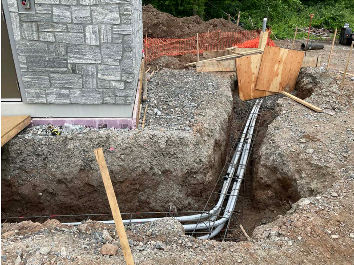
Picture 1: Bank of conduits located on the north and west side of the booster station with rebar in place, ready for the concrete placement today. View to the south.
