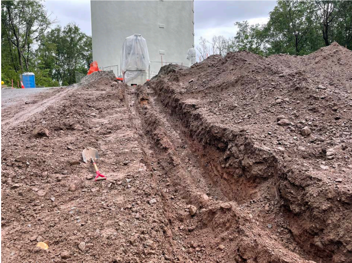
Picture 7: View of the trench that Ludlow has begun to excavate for the installation of 2” and 4” PVC utility conduits on the south side of the Shared Access Driveway. View to the east.
