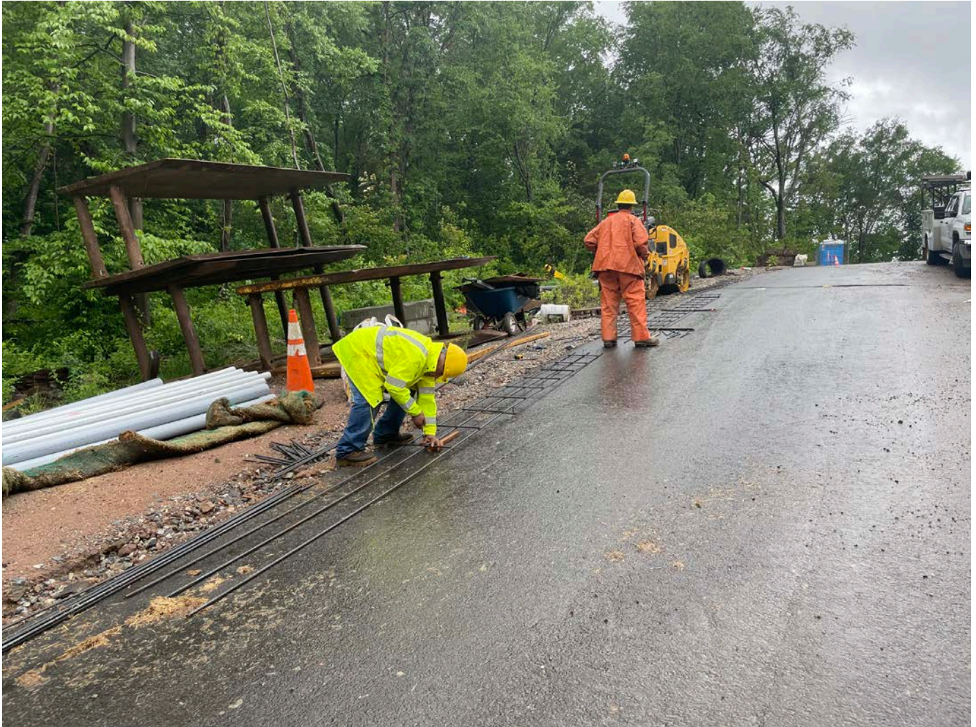
Picture 9: Ludlow connecting sections of rebar together for placement into the utility trench they are excavating on the south side of the Shared Access Driveway in Middletown. View to the east.
