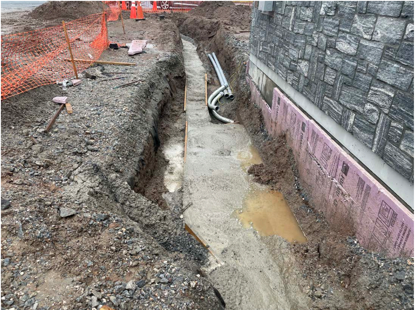
Picture 8: Concrete that Ludlow and Tilcon placed over the bank of conduits located on the north and west side of the booster station after a heavy downpour. View to the east.
