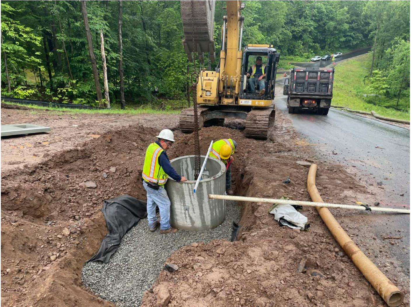
Picture 10: Concrete transformer pad that Ludlow is installing at ~Station 11+60 for the placement of a transformer to the south of the Shared Access Driveway in Middletown. (Note top slab on ground to the left in the photo) View to the west.
