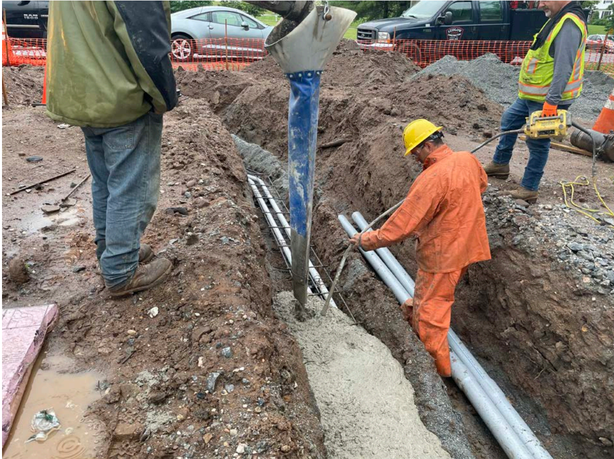
Picture 6: Ludlow and Tilcon placing concrete while Ludlow uses a vibrator to settle the concrete into place over the bank of conduits located on the north and west side of the booster station. View to the east.
