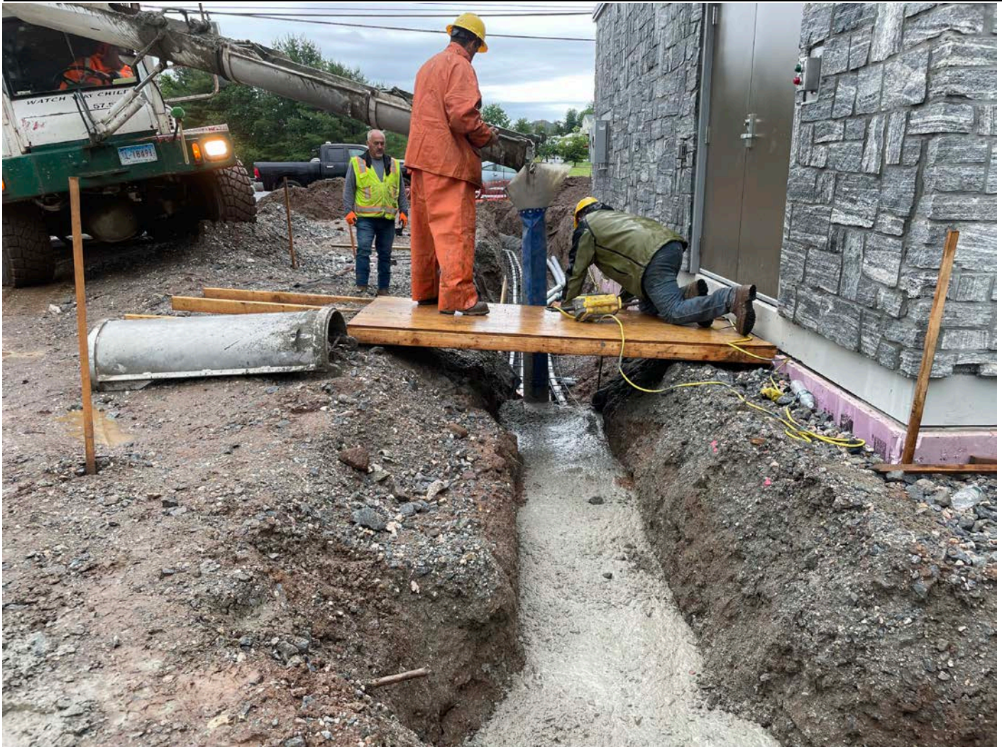
Picture 5: Ludlow and Tilcon placing concrete over the bank of conduits located on the north and west side of the booster station. View to the east.
