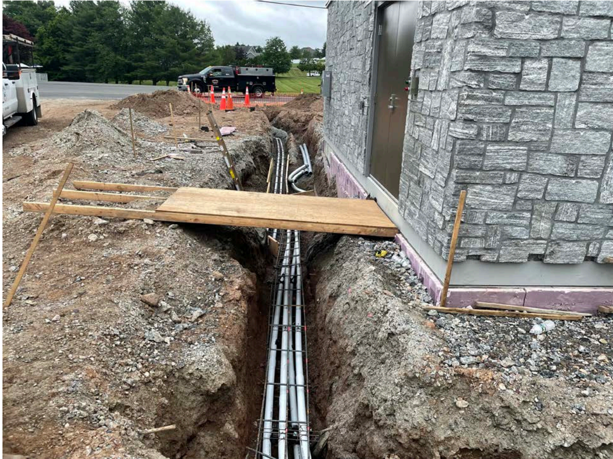
Picture 2: Bank of conduits located on the north of the booster station with rebar in place, ready for the concrete placement today. View to the east.
