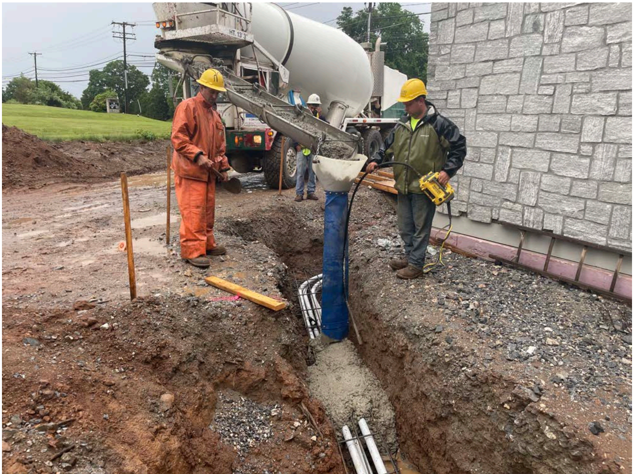
Picture 3: Ludlow and Tilcon placing concrete over the bank of conduits located on the north and west side of the booster station. View to the south.
