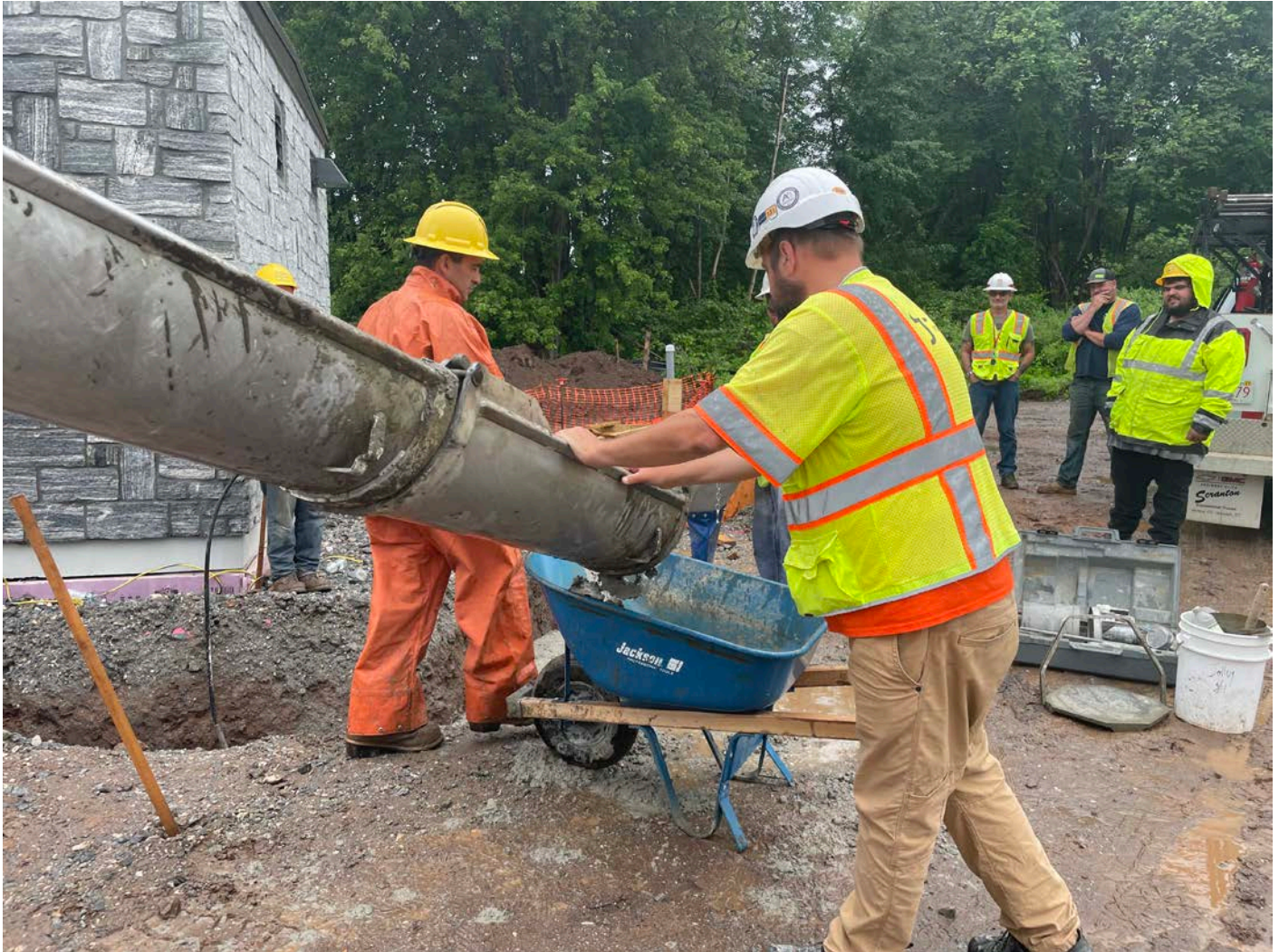
Picture 4: JTC collecting concrete for field and laboratory analysis at the booster station.
