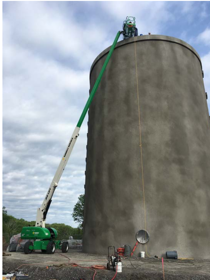
Picture 1: Facing west. Coating underway on the dome.
