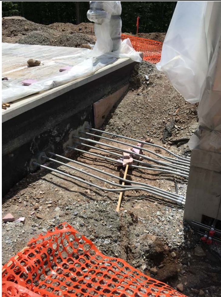
Picture 11: Facing southwest. Completed conduit between altitude valve vault and electrical enclosure up at the water tank site. Note protective plastic over vault and enclosure to protect from tank coating overspray.
