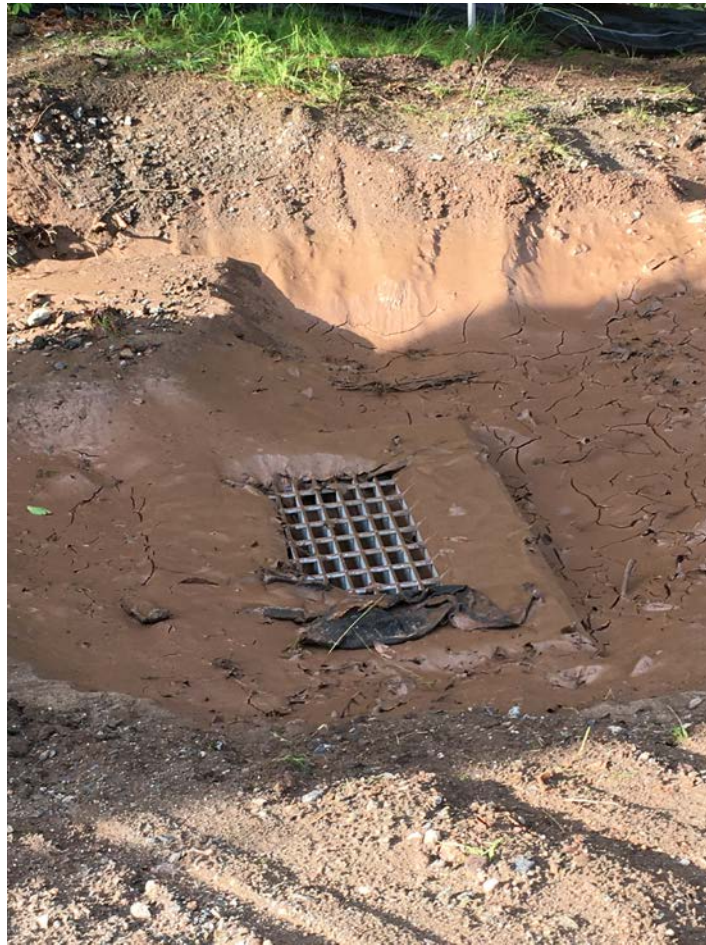
Picture 2: Facing south. View into new catch basin at tank site with silted in and flooded because silt sock plugged.
