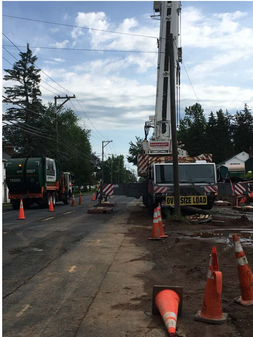
Picture 3: Facing north. Crane with outriggers extended. However back end of crane was slightly over center line hence cone placement. Traffic was able to safely pass.
