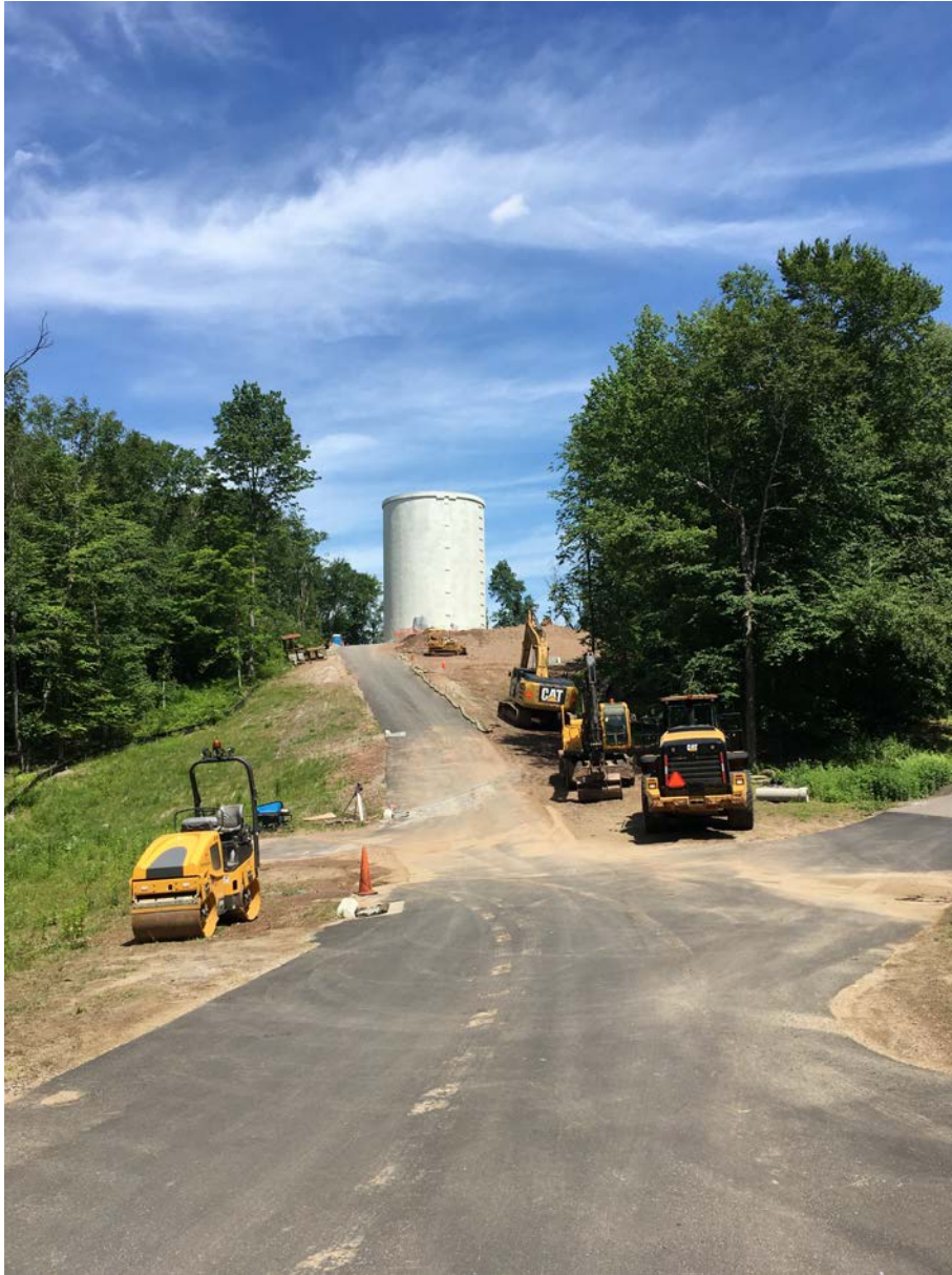
Picture 10: Facing east. View of water tank after first coat of coating. Soil on road is from overnight wash out of new catch basin.
