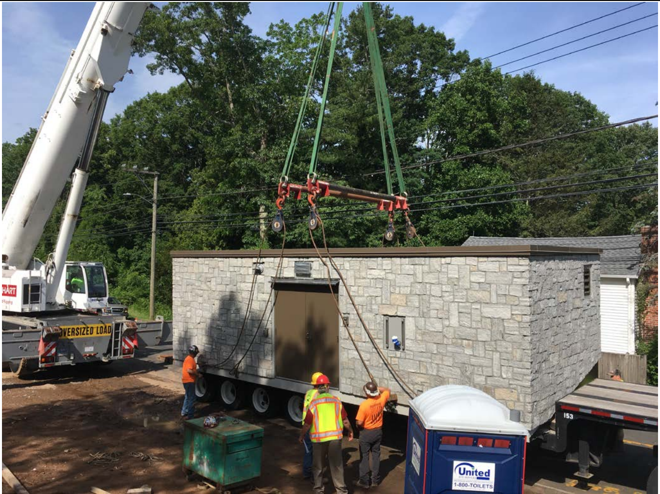
Picture 6: Facing southwest. Setting up rigging. Notice that the spreader bars are too short. Longer bars were brought in so that rigging did not damage top of meter building.
