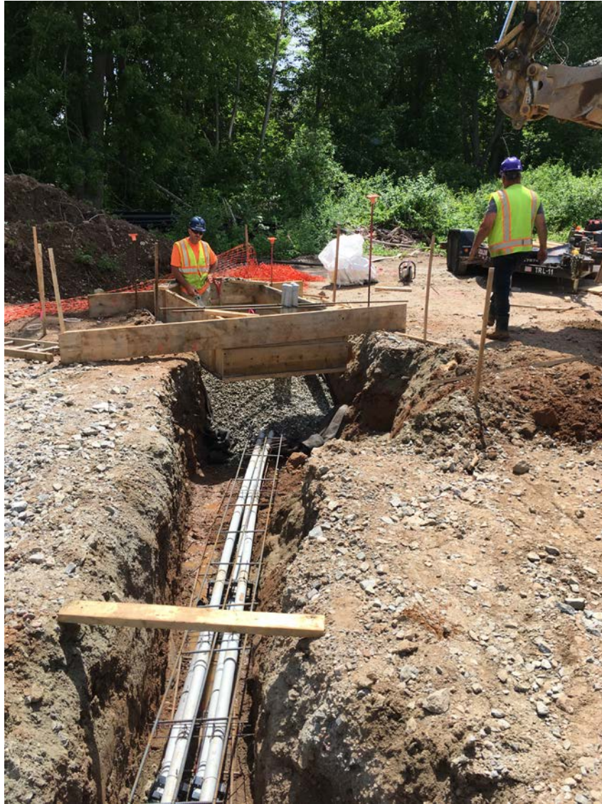
Picture 13: Facing south. Behind booster station this the form for the concrete pad for the generator. The stone base needs to be raised to the bottom of the form prior to concrete pad. Conduit leading to the generator pad in foreground.
