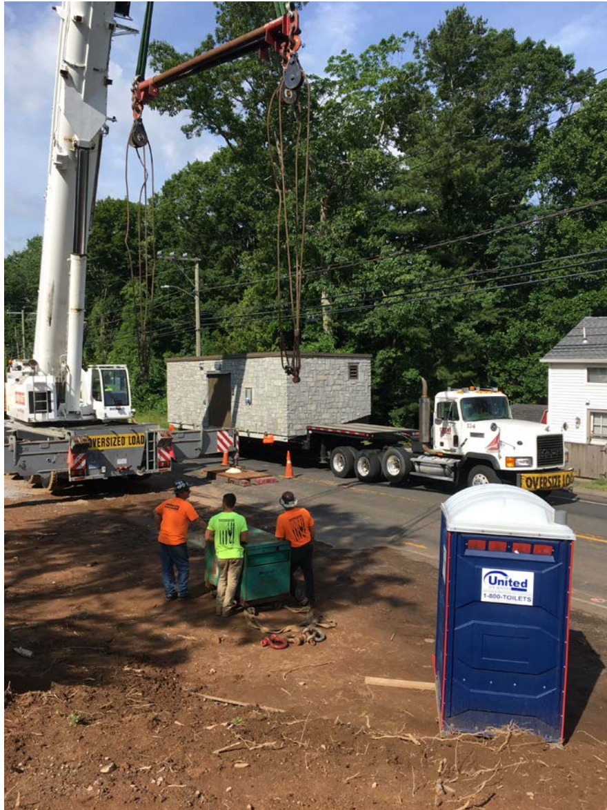
Picture 5: Facing southwest. Meter building arrives on step-deck low-boy trailer.
