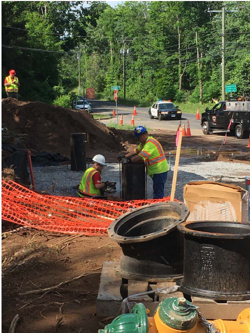
Picture 7: Facing south. United Concrete shortening piping to align with meter house piping.
