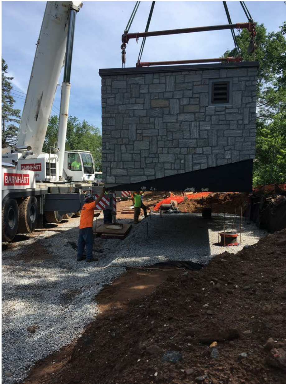
Picture 9: Facing north. Aligning the meter building with piping.
