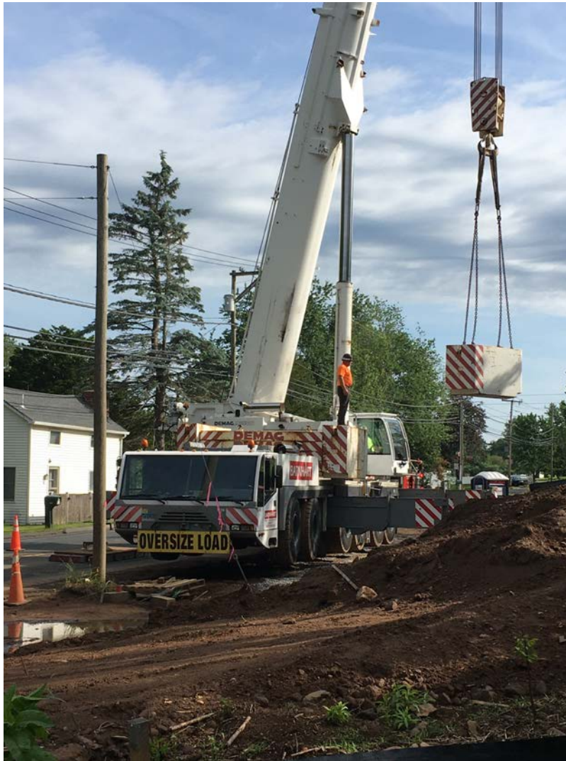
Picture 4: Facing northwest. Loading additional counterweight to crane.
