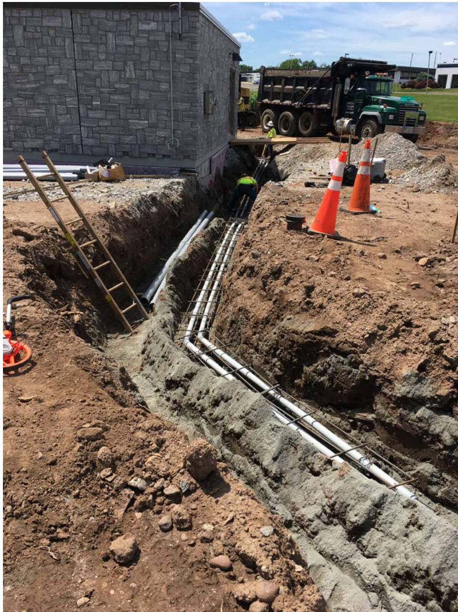
Picture 12: Facing west. Conduit from the booster station toward the street.
