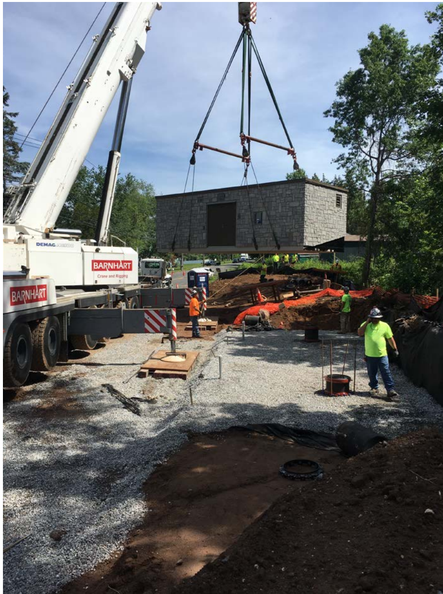
Picture 8: Facing north. Lifting the meter building off the low-boy truck
