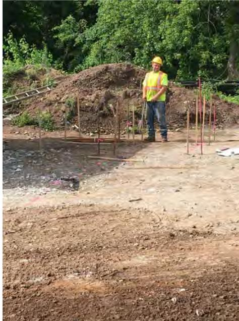
Picture 3: Facing south, behind booster station. Mark out for generator foundation.
