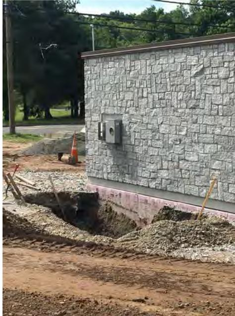
Picture 1: Facing southeast. Conduits exit through booster station wall at this location. Start of excavation
