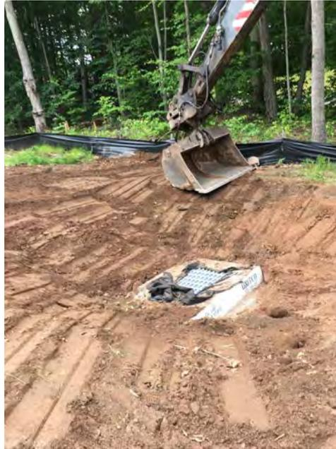
**Picture 7: View south. New catch basin installed. Finalized catchment grading around basin.**
