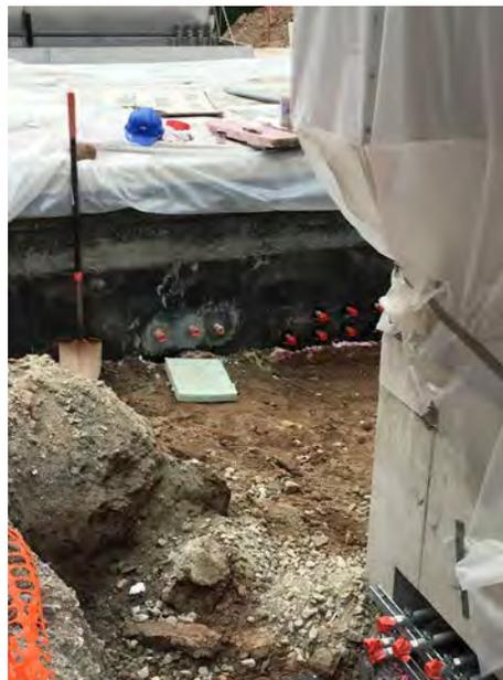
**Picture 8: Conduits sealed through vault up at water tank. Electrical enclosure to right in foreground. Two to be connected by United's electrician.**
