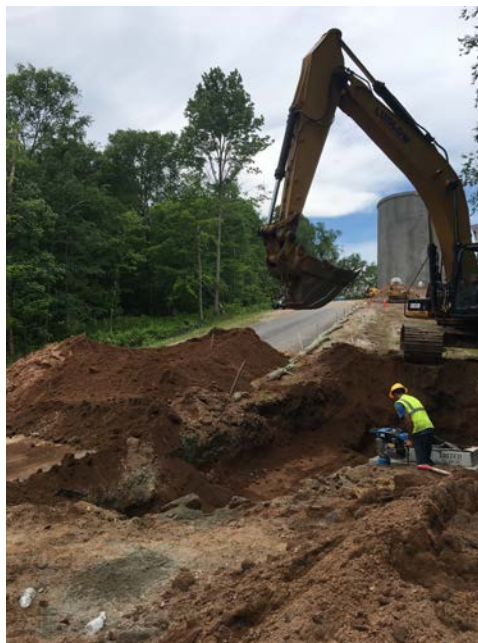
Picture 8: Compacting and grading. Note still a way to go.
