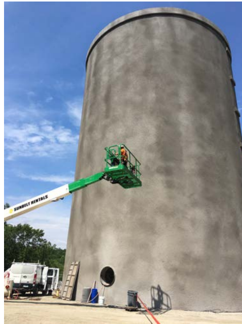
Picture 5: DN Tanks heading up to top of tank to guide crane.
