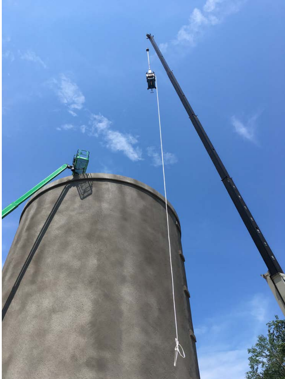
Picture 4: First lift with tether line.
