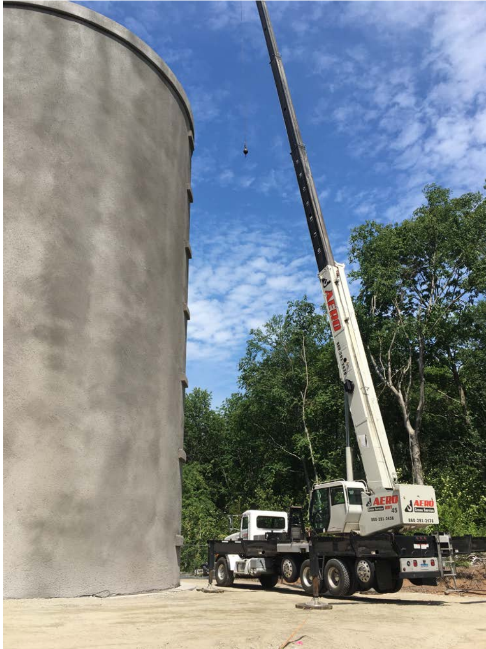
Picture 3: Crane level and extended.
