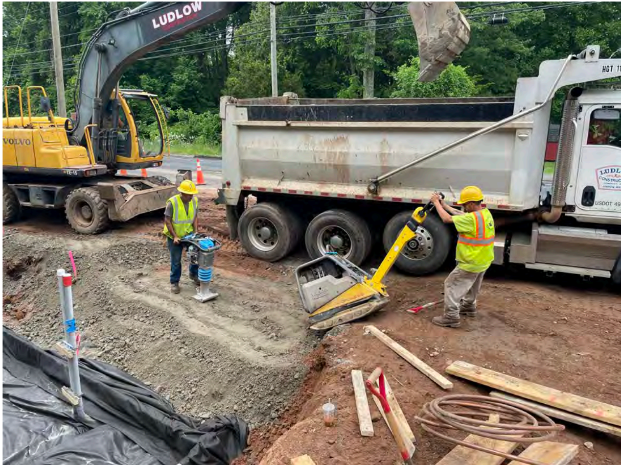
Picture 6: Ludlow compacting gravel over the 16" DIP pipe they installed on the north side of the water meter vault footprint located at ~Station 124+80. View to the southwest.
