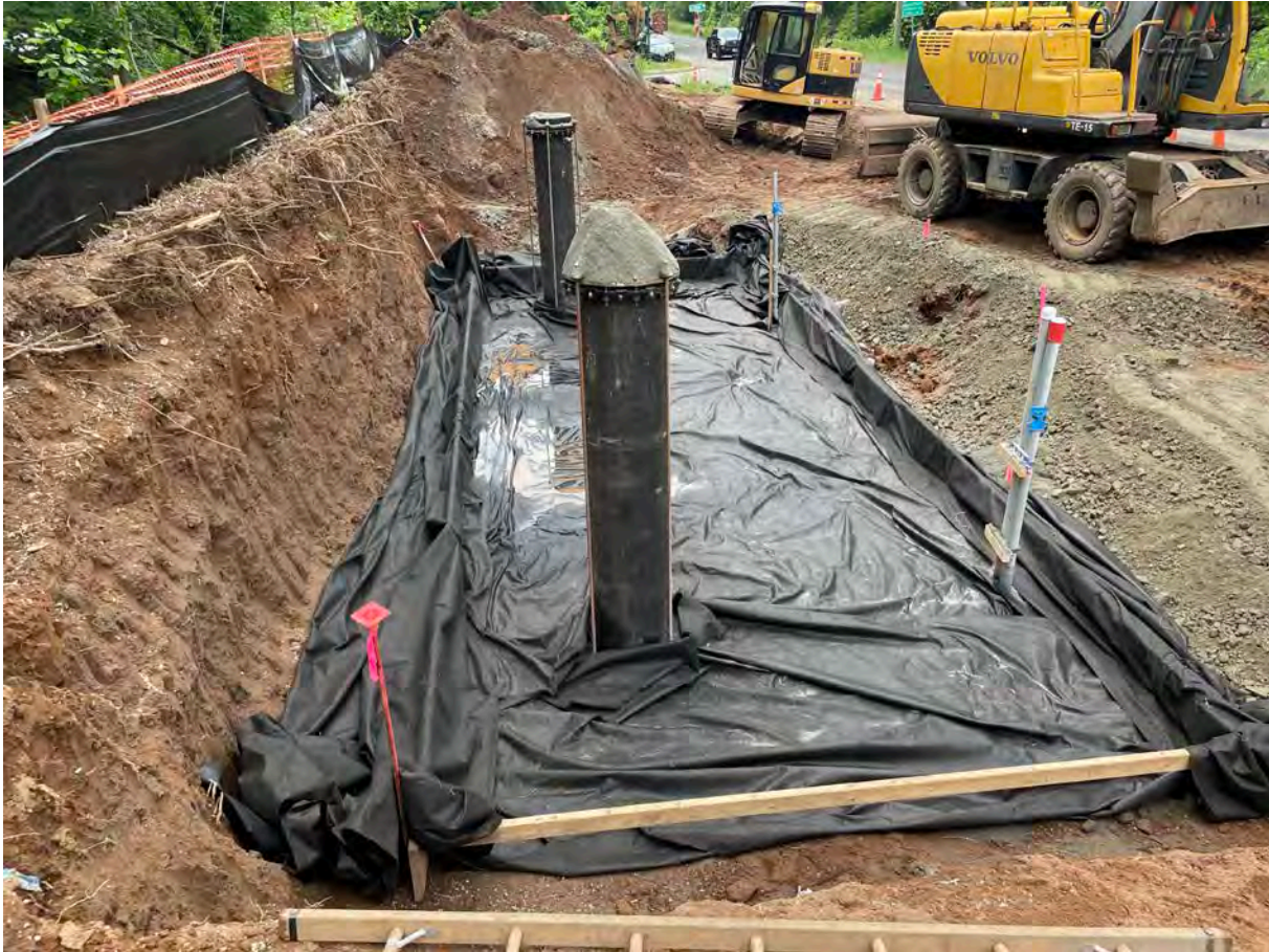
Picture 7: View of the water meter vault footprint, where Ludlow has lined it with geofabric. View to the south.
