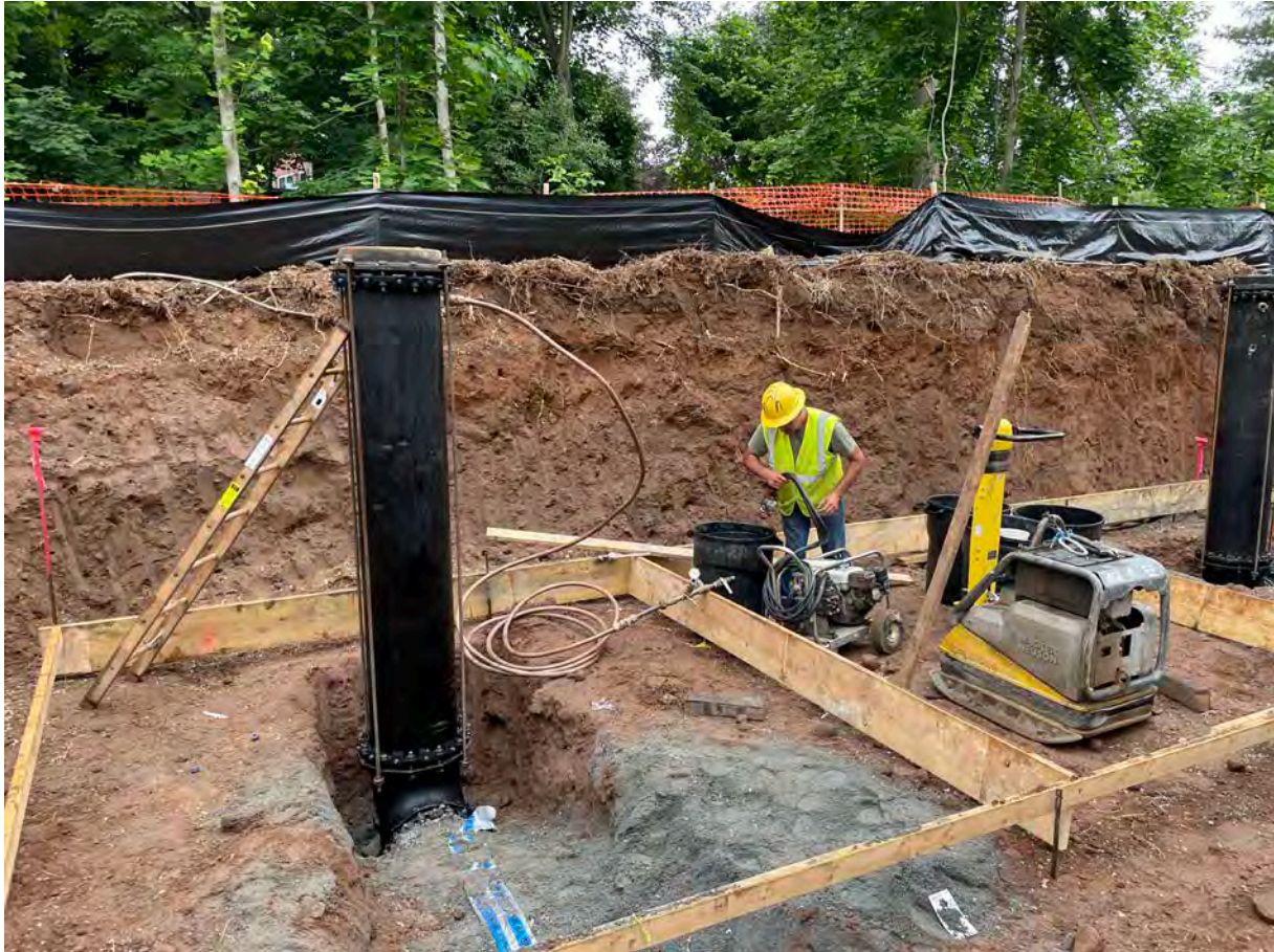
Picture 1: Section of 16" DIP that Ludlow attached to a 90° bend on the north side of the water meter vault footprint yesterday. Ludlow is starting a pressure test from this pipe to where they connected 16" DIP at Station 124+72. View to the southeast.
