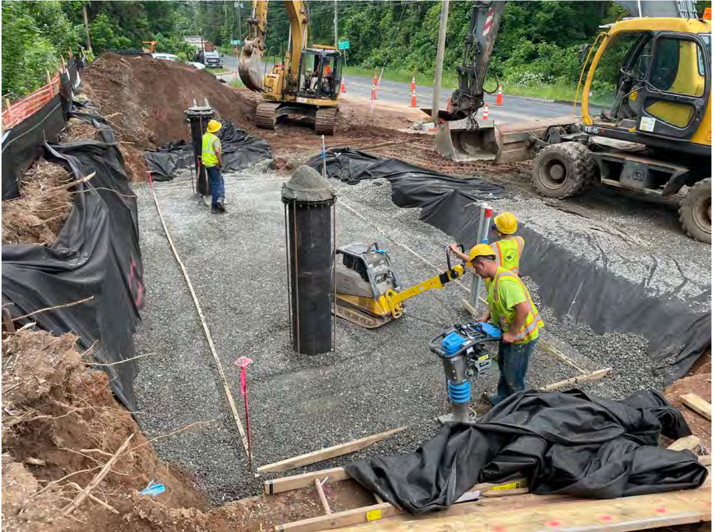
Picture 8: View of the water meter vault footprint where Ludlow placed and compacted 1' of ¾" gravel, and is placing a second 1' lift of gravel. View to the south.
