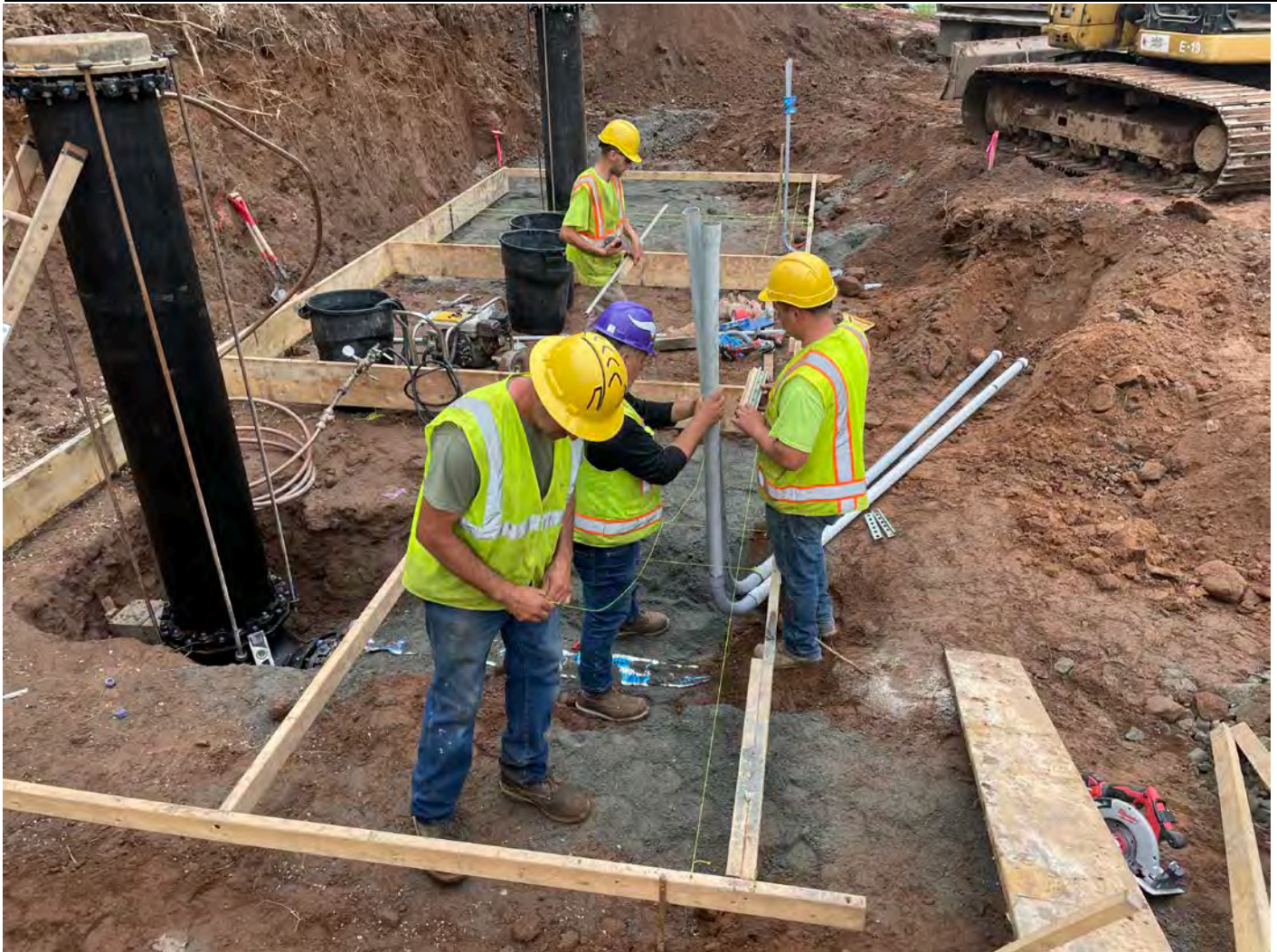
Picture 5: Ludlow installing additional PVC conduits on the west side of the water meter vault footprint. View to the south.
