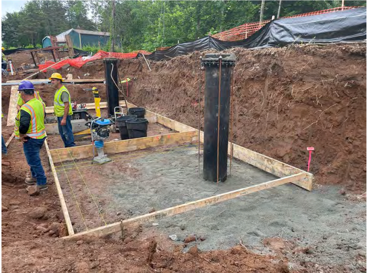
Picture 2: View of the water meter vault footprint and the pressure test that Ludlow is conducting today. View to the north.
