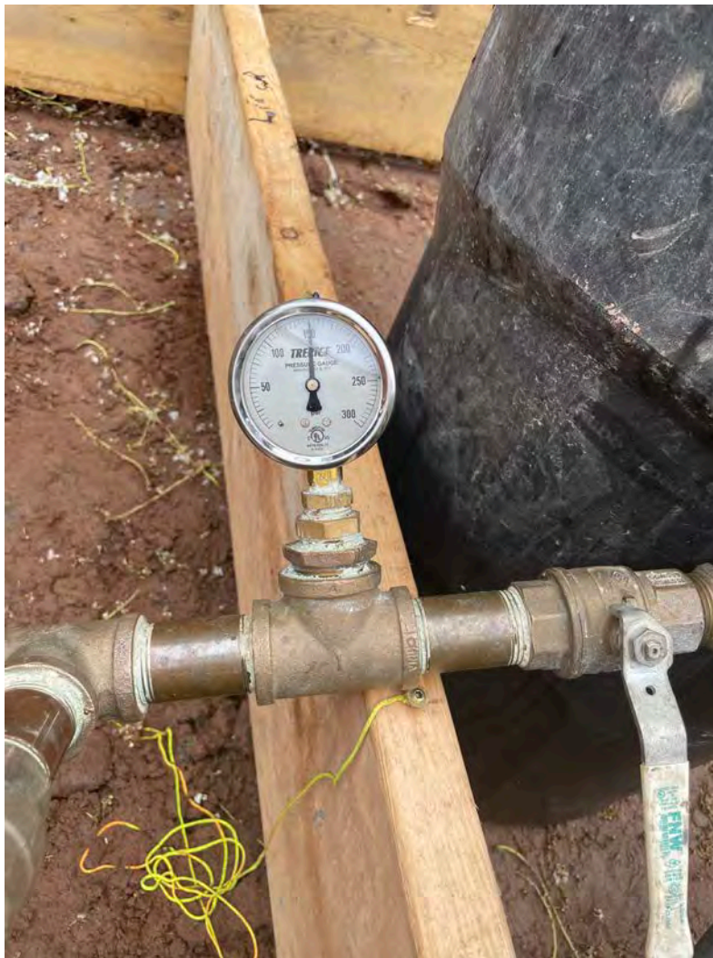
Picture 3: Starting pressure of 150 PSI on the pressure test that Ludlow is performing today at the water meter vault.
