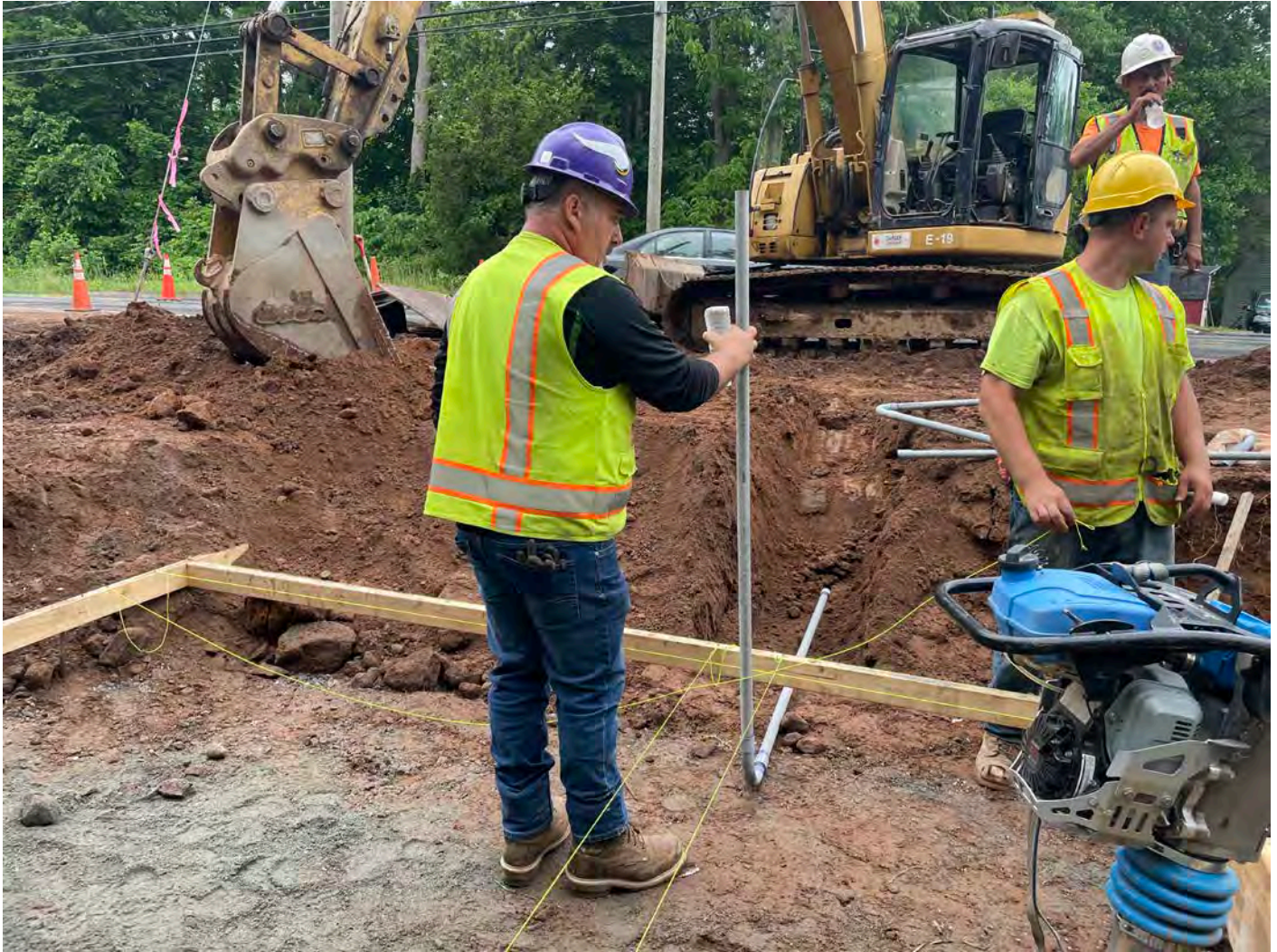
Picture 4: Ludlow installing 1" PVC electrical conduits on the west side of the water meter vault footprint. View to the west.
