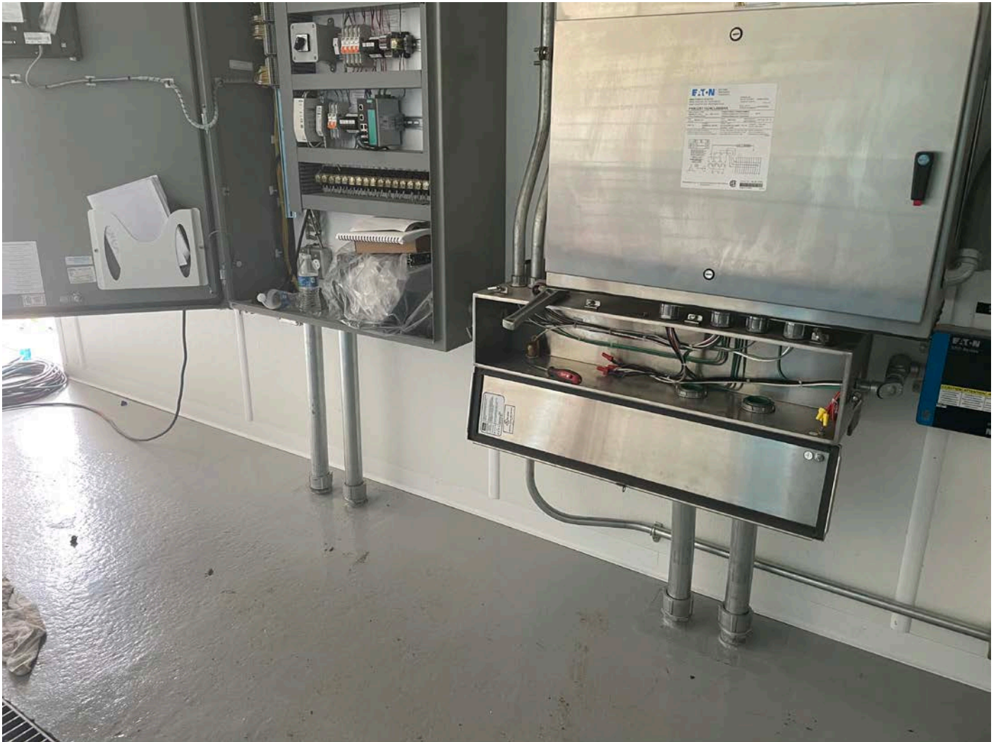
Picture 4: Cabinets on the north wall of the booster station interior where United Concrete has completed the installation of conduits on the underside of the cabinets. View to the northwest.
