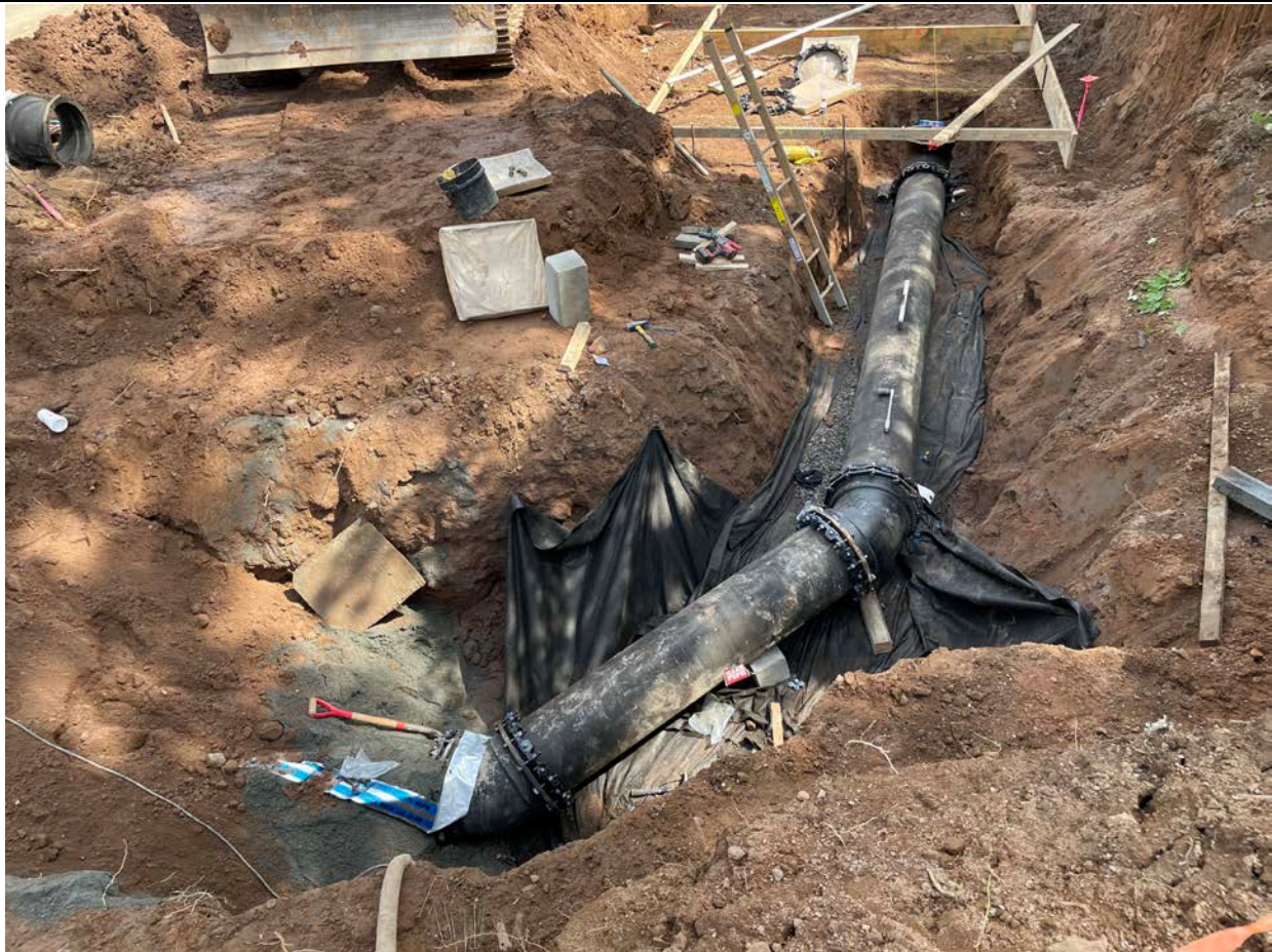
Picture 2: 16" DIP that Ludlow has installed to the south side of the water meter vault footprint. View to the north.
