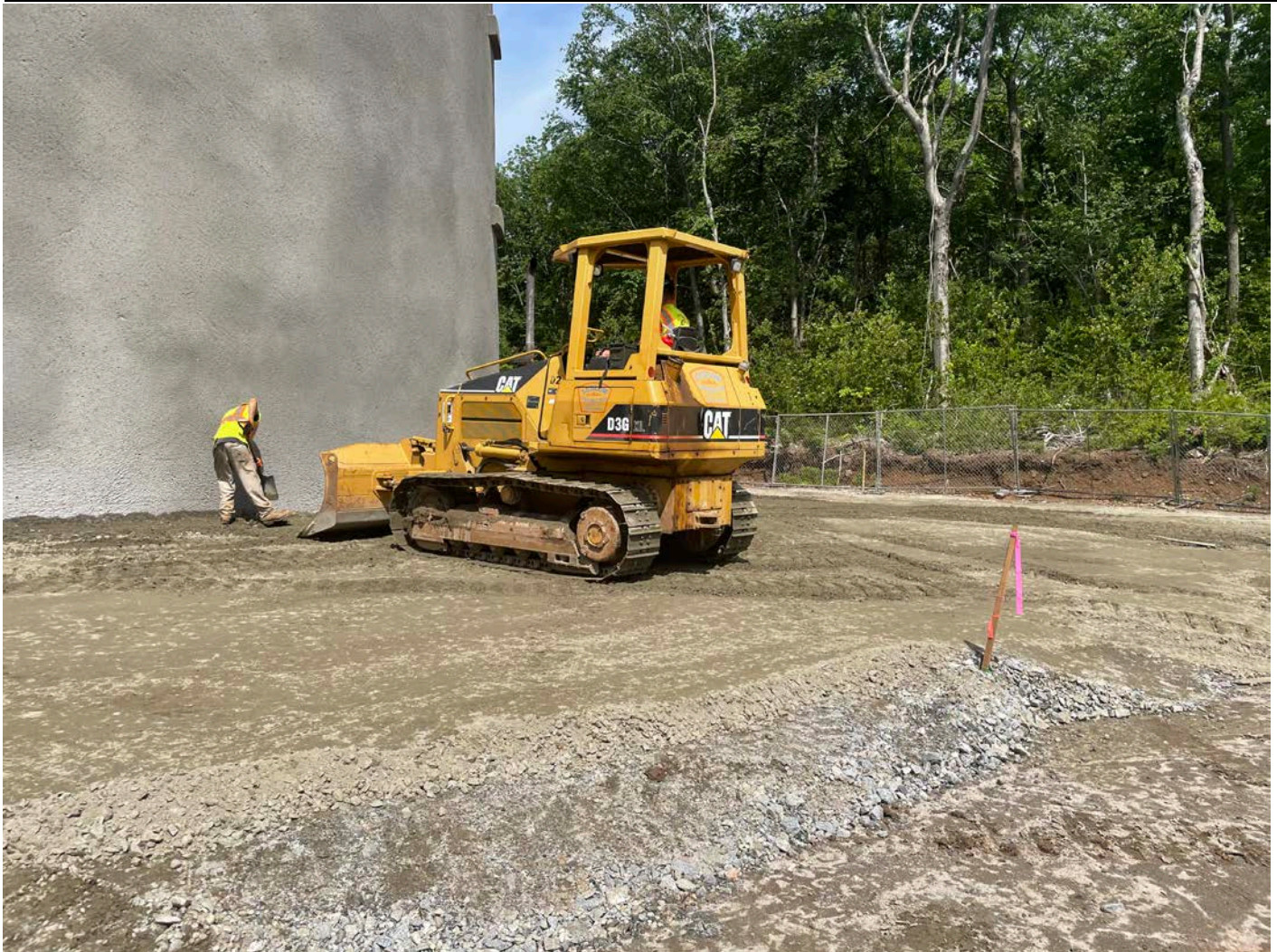
Picture 5: Ludlow grading 1.5" gravel they have been placing on the east side of the water tank located east of the Shared Access Driveway in Middletown. View to the northwest.
