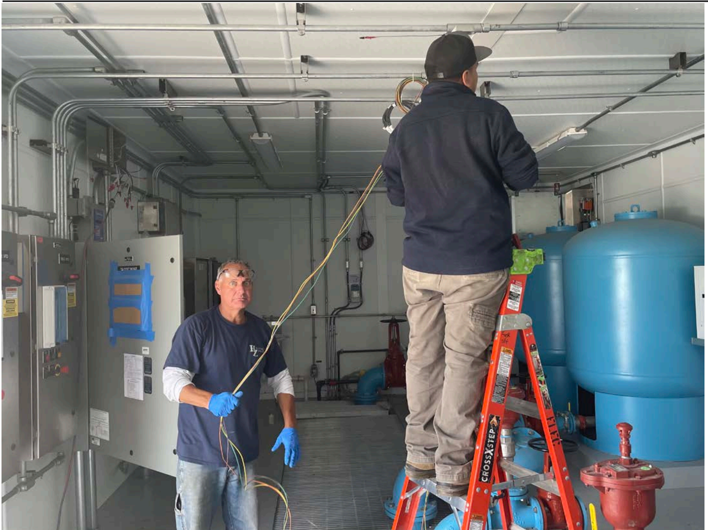
Picture 8: United Concrete installing wiring inside of the booster station located at Station 750+63 on S. Main Street, Middletown. View to the east.
