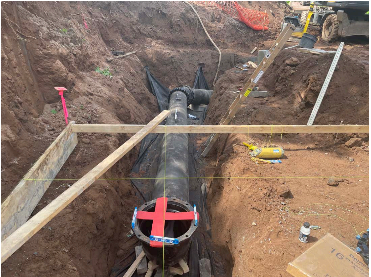
Picture 3: 16" DIP that Ludlow has installed to the south side of the water meter vault footprint. Note the 90° DIP bend that was installed on the north end of the 16" DIP. View to the south.
