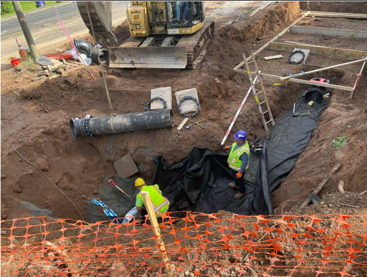
Picture 1: Ludlow in the process of installing 16" DIP close to Station 801+00 at the water meter vault located at ~Station 124+80 on S. Main Street in Middletown. View to the north.
