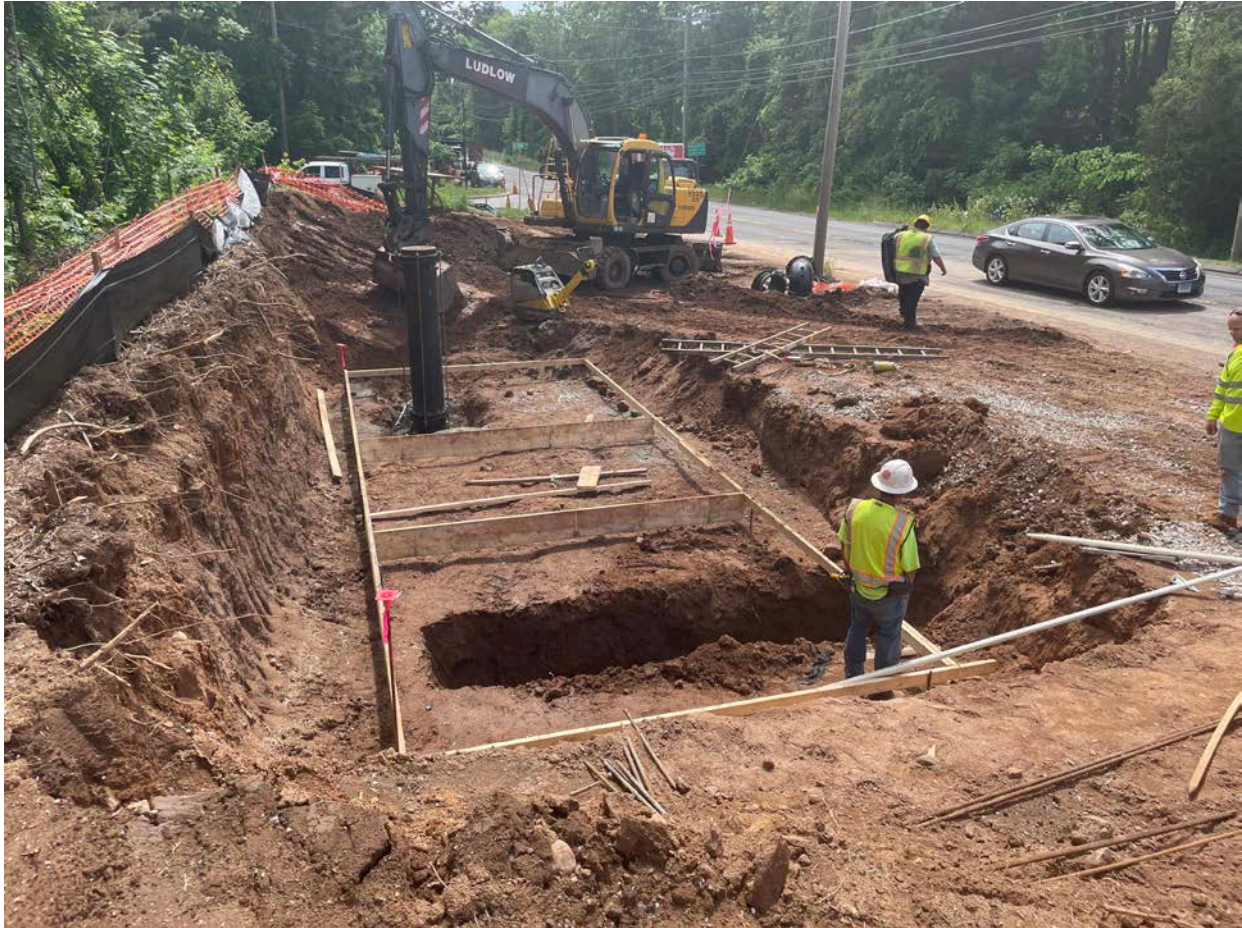
Picture 7: Overview of the water meter vault work zone located at ~Station 124+80. View to the south.
