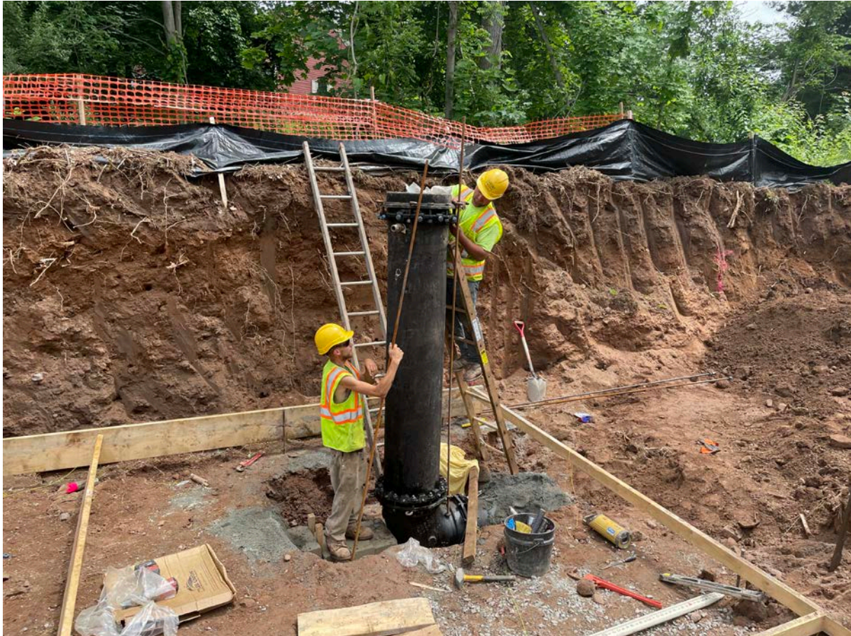
Picture 6: Ludlow securing a section of 16" DIP to the top of a 90° DIP bend on the south side of the water meter vault located at Station 124+80. View to the southeast.
