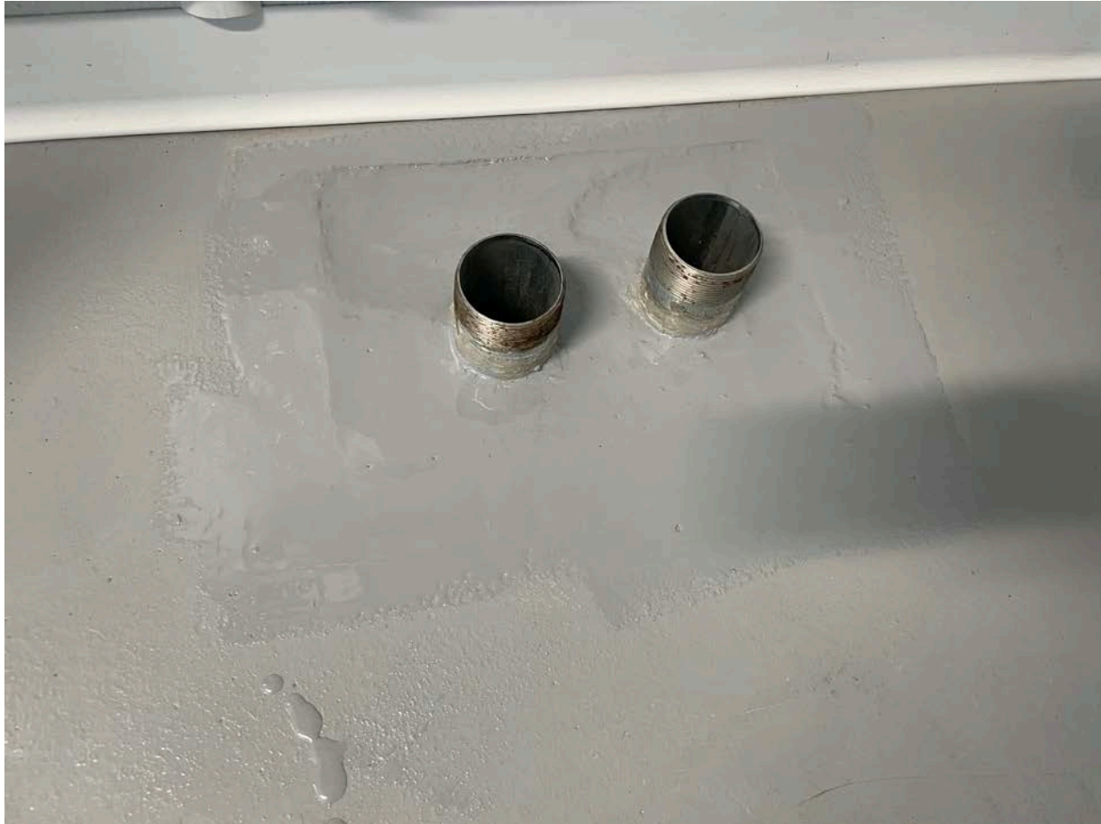
Picture 2: Concrete patch around conduits located on the floor of the booster station that were sealed off with the same epoxy-based paint that the booster station floor was coated with.
