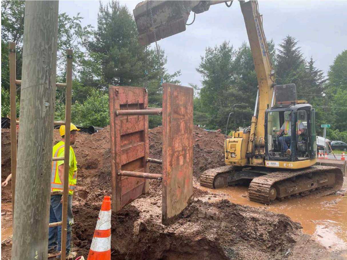
Picture 6: Ludlow placing a trench box on the east side of S. Main Street in Middletown as they excavate at Station 125+20 for the installation of 16" DIP. View to the south.
