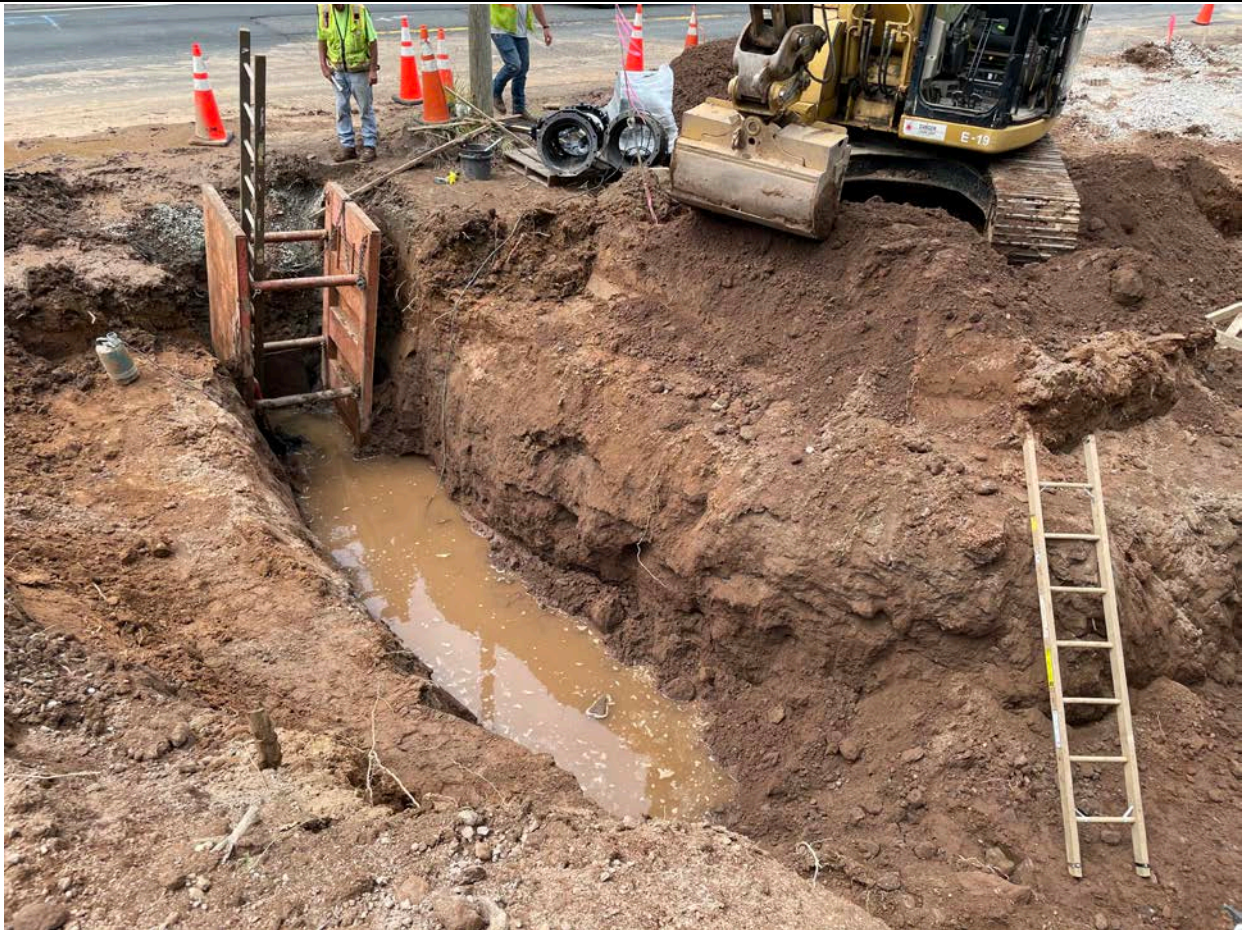
Picture 8: Water in the excavation located at the water meter vault work zone that came from beneath the 16” DIP that crosses S. Main Street at Station 125+20. View to the west.
