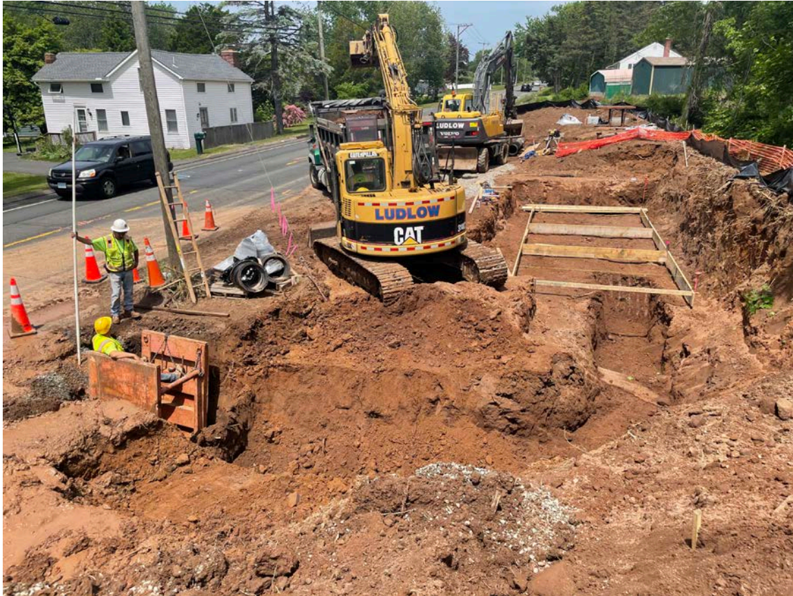
Picture 7: Overview of excavation activities at Station 125+20, and the water meter vault work zone. View to the northwest.
