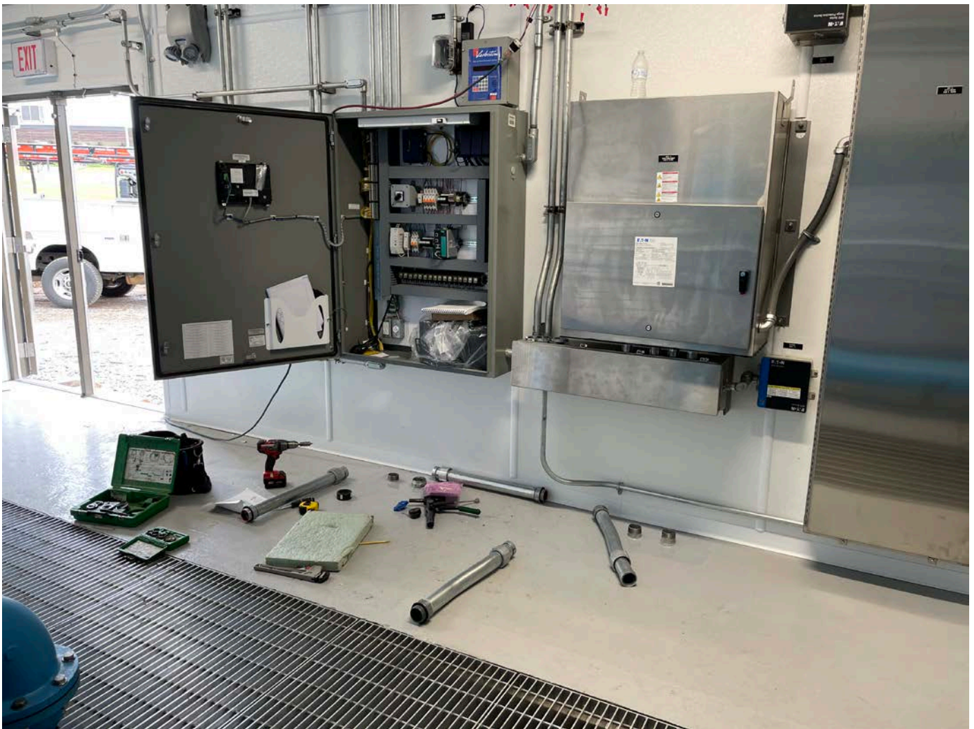
Picture 3: United Concrete installing conduits on the underside of the PLC pump cabinet located inside of the booster station at Station 750+63. View to the northwest.
