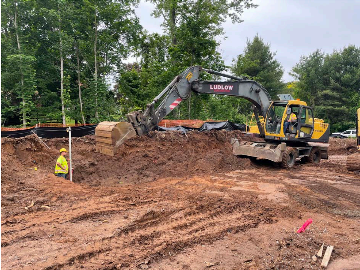
Picture 1: Ludlow continuing earthwork at the footprint of the water meter vault located at ~Station 124+80 on S. Main Street in Middletown. View to the south.
