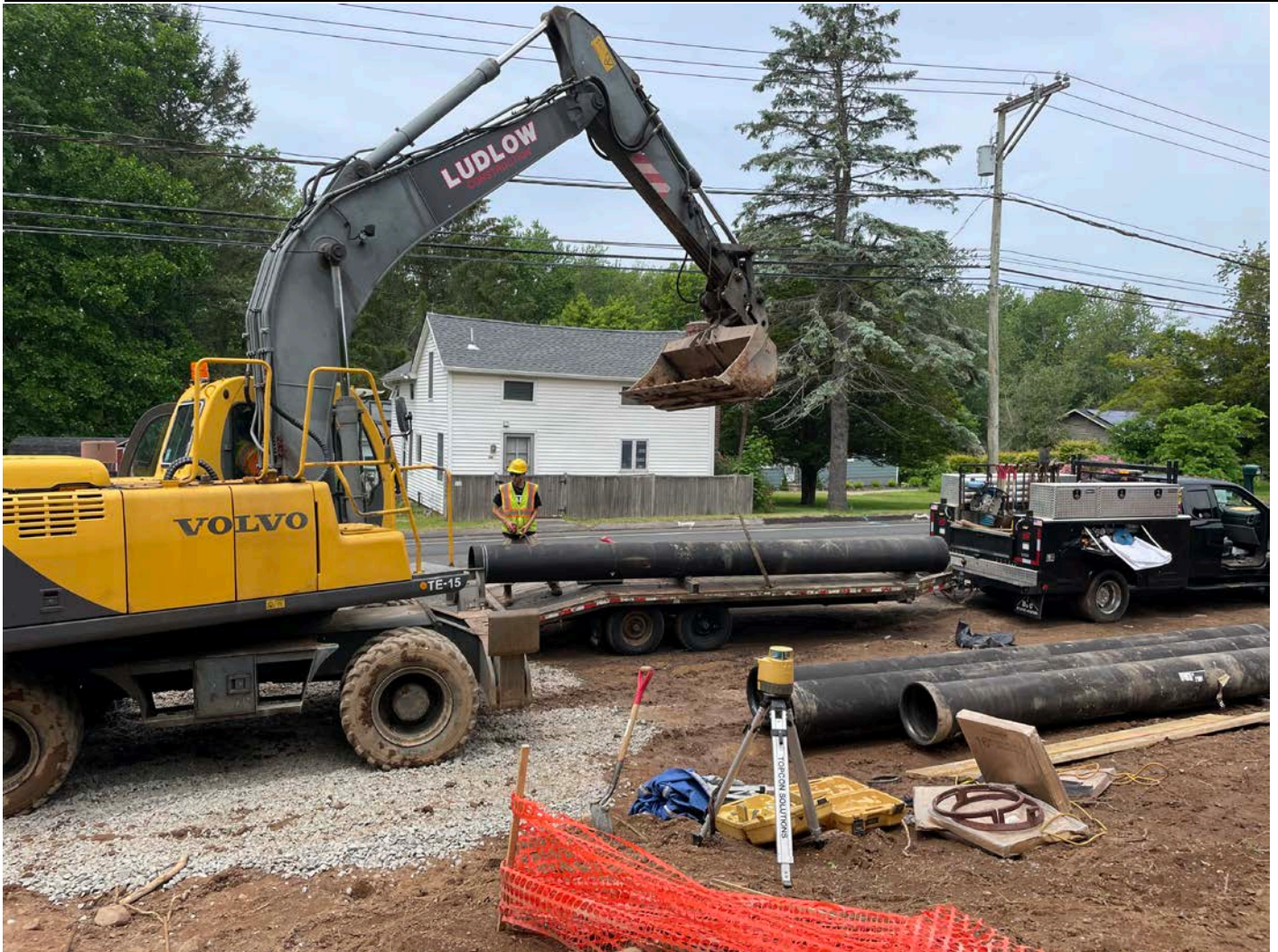
Picture 5: Ludlow offloading 16" DIP at the water meter vault work zone located at ~Station 124+80 on S. Main Street in Middletown. View to the northwest.
