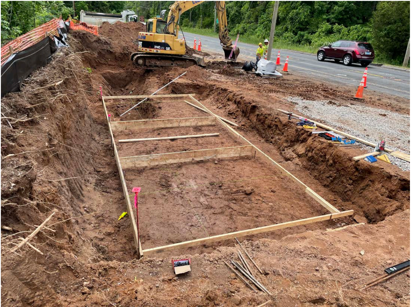
Picture 4: Ludlow in the process of laying out a wooden framework within the footprint of the water meter vault that will assist them in the accurate placement of piping going in and out of the vault. View to the southeast.
