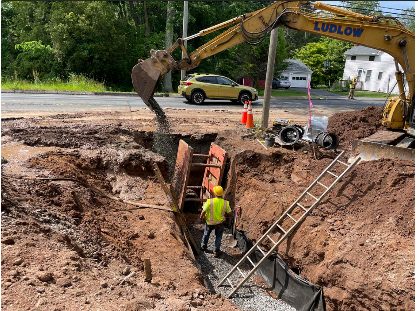
Picture 9: Ludlow placing 3/4" stone around a pump that is moving water from the excavation at Station 125+20 on S. Main Street, Middletown. View to the west.
