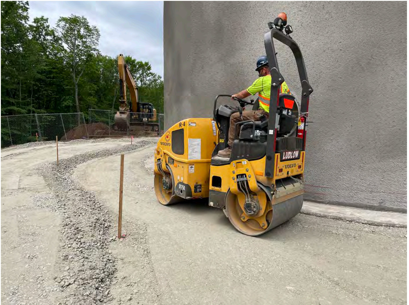
Picture 4: Ludlow compacting fill in the west side of the base of the water tank located east of the Shared Access Driveway in Middletown. View to the northeast.
