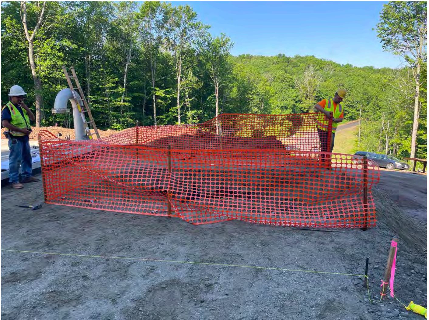
Picture 3: Ludlow placing snow fence around the footprint they prepared for the installation of an electrical enclosure tomorrow on the north side of the altitude valve vault. View to the west.
