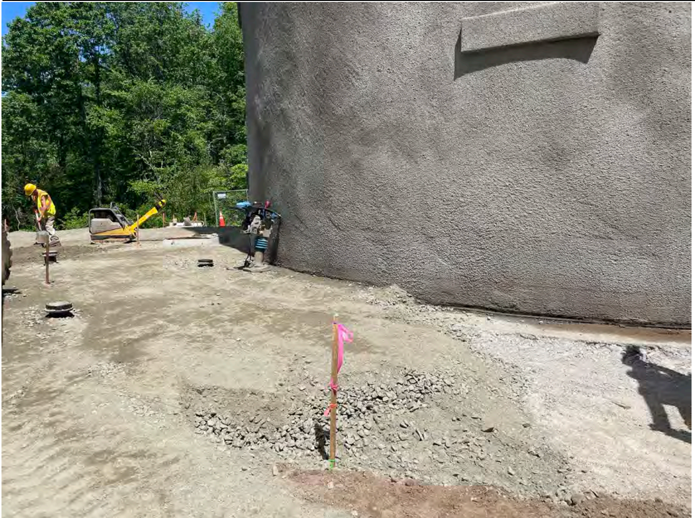
Picture 5: View of grade on the west side of the water tank as Ludlow continues to place and compact fill. View to the northeast.
