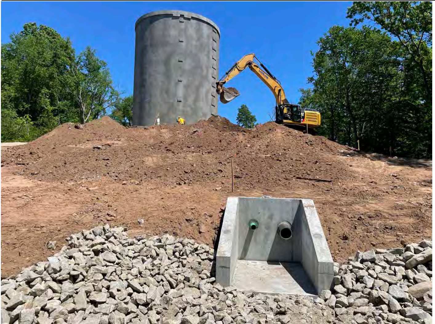
Picture 9: View of the water tank work zone located east of the Shared Access Driveway, looking east at the end of the day.
