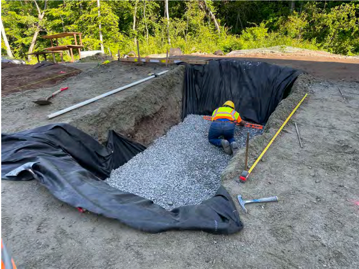
Picture 1: Ludlow leveling ¾" rock at the footprint for the electrical enclosure that United Concrete plans to install tomorrow on the north side of the altitude vault. View to the north.
