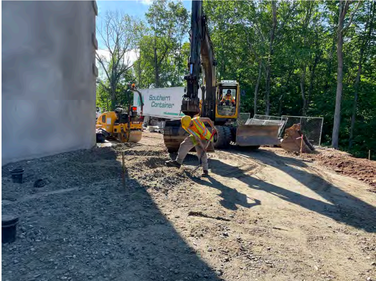
Picture 2: Ludlow bringing fill up to grade along the southwest side of the water tank located east of the Shared Access Driveway in Middletown. View to the southeast.
