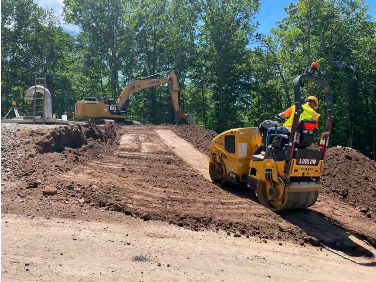
Picture 6: Ludlow compacting fill west of the altitude valve vault where they are building an earthen road. View to the south.
