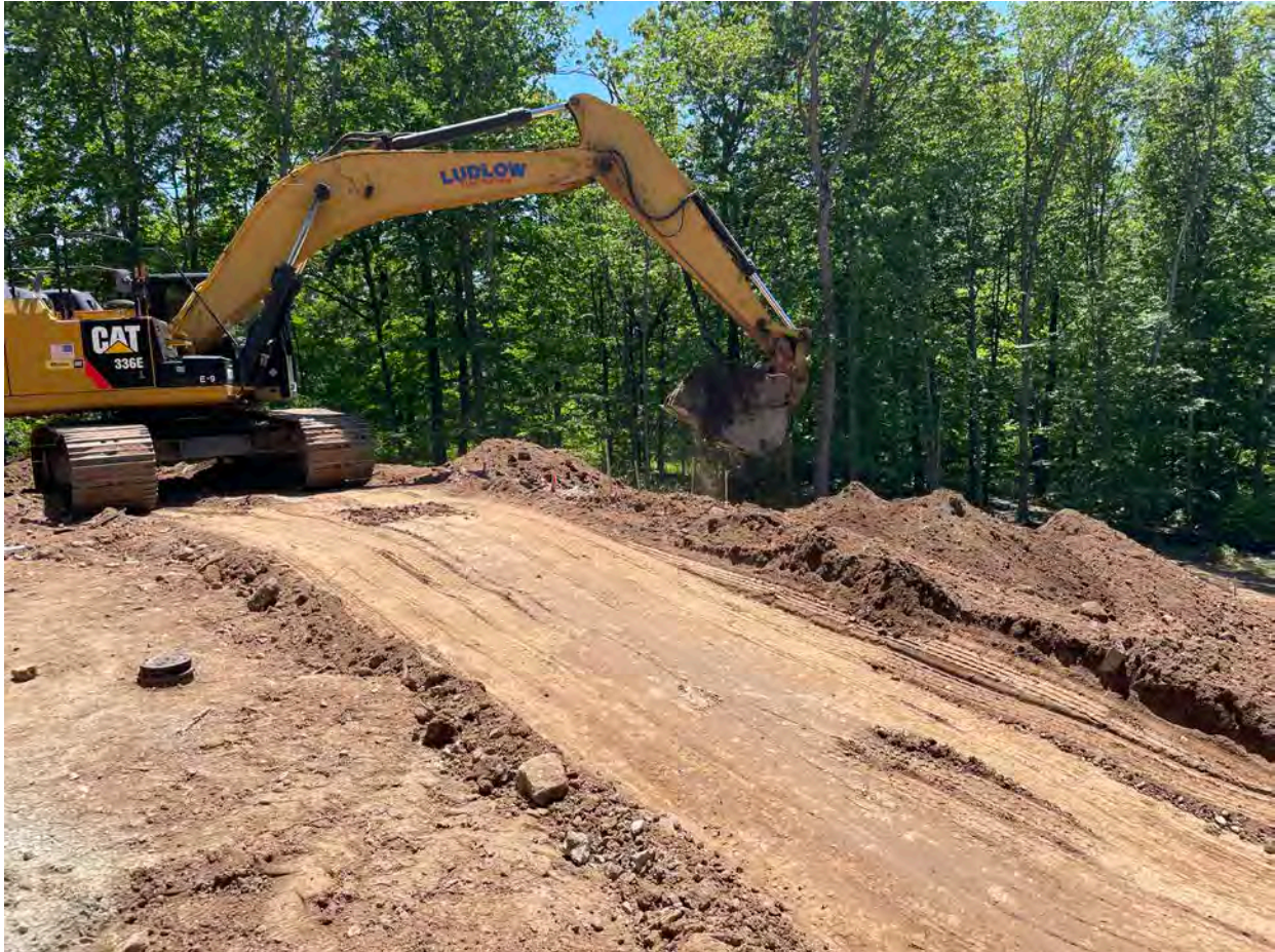
Picture 8: Ludlow performing earthwork as they build an earthen road south of the altitude valve vault. View to the south.
