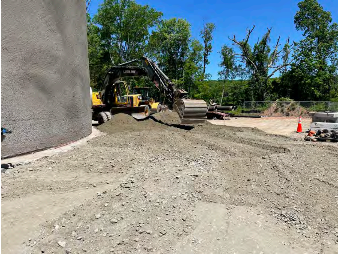
Picture 7: Ludlow bringing fill up to grade along the south side of the water tank located east of the Shared Access Driveway in Middletown. View to the east.
