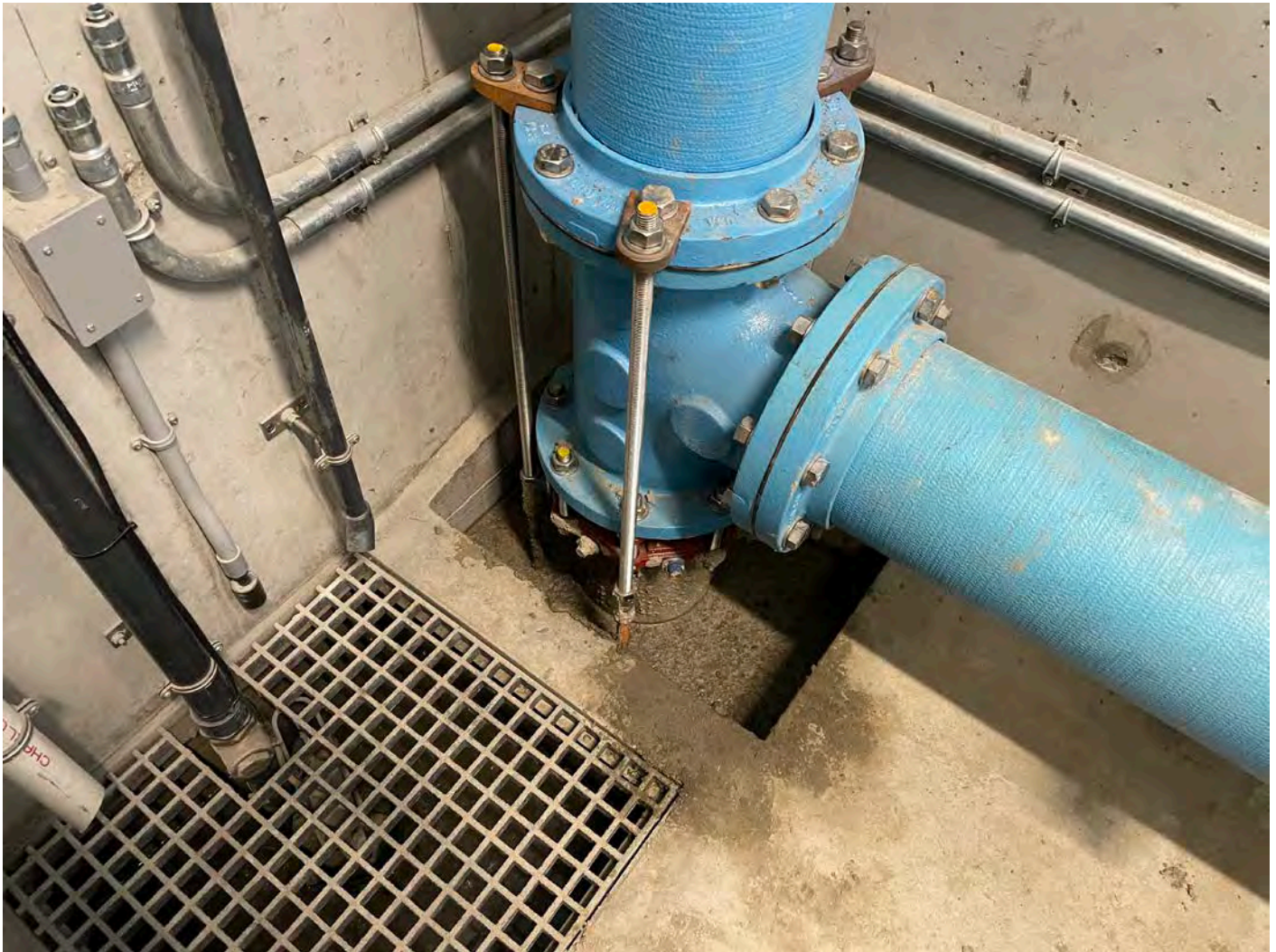
Picture 4: Penetration in the floor of the booster station trough that United Concrete filled with concrete today (photograph depicts penetration before filling). Booster station located at Station 750+63 in Middletown. View to the southeast.
