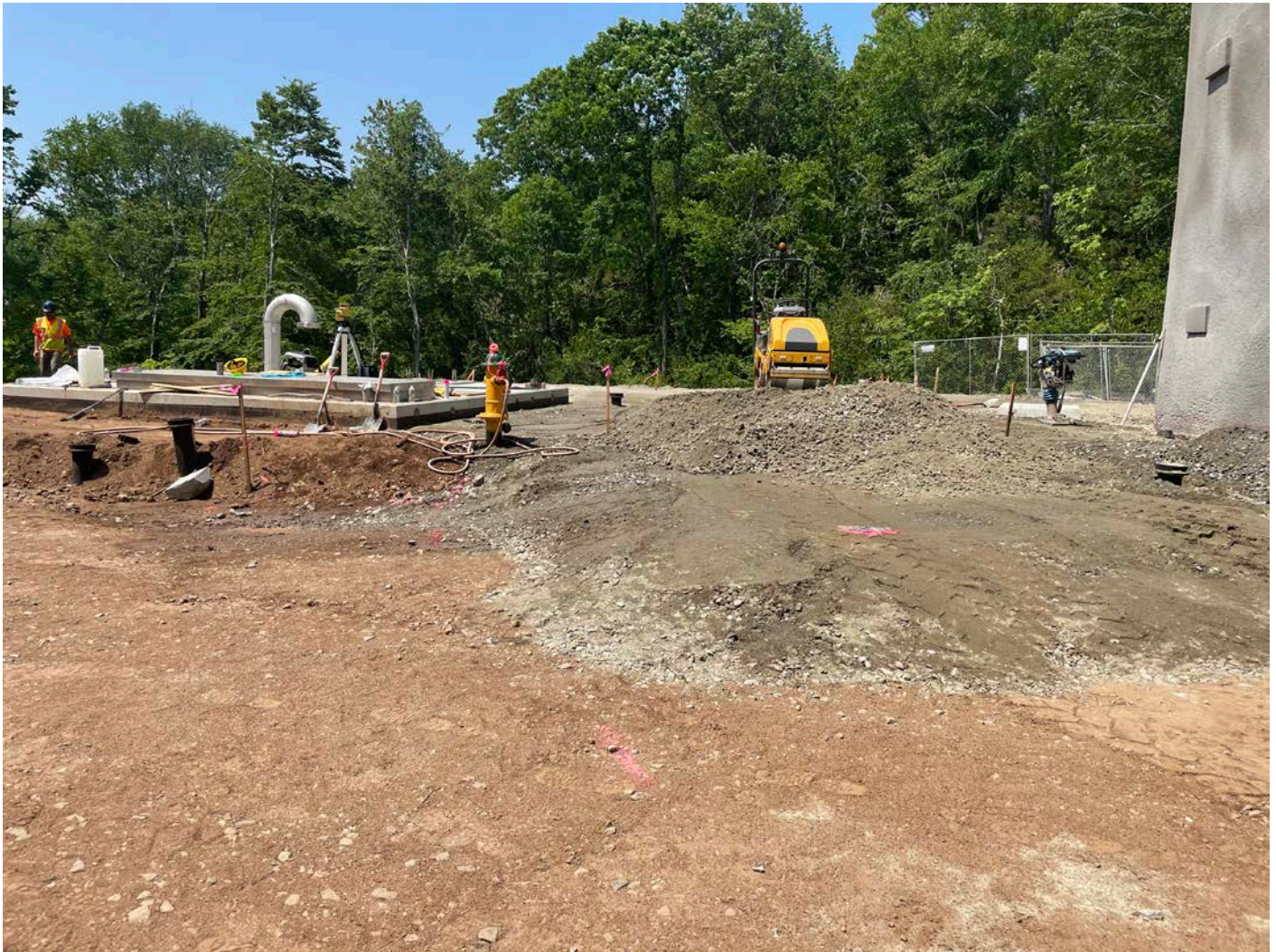
Picture 9: View of fill Ludlow has placed around the altitude valve vault on the west side of the water tank located east of the Shared Access Driveway in Middletown. View to the north.
