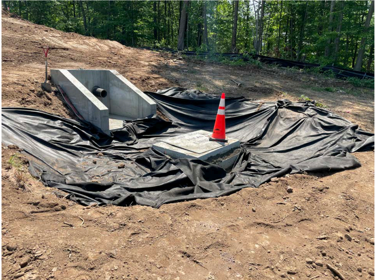
Picture 2: Headwall located at Station 11+50 catch basin under construction. View to the southeast.
