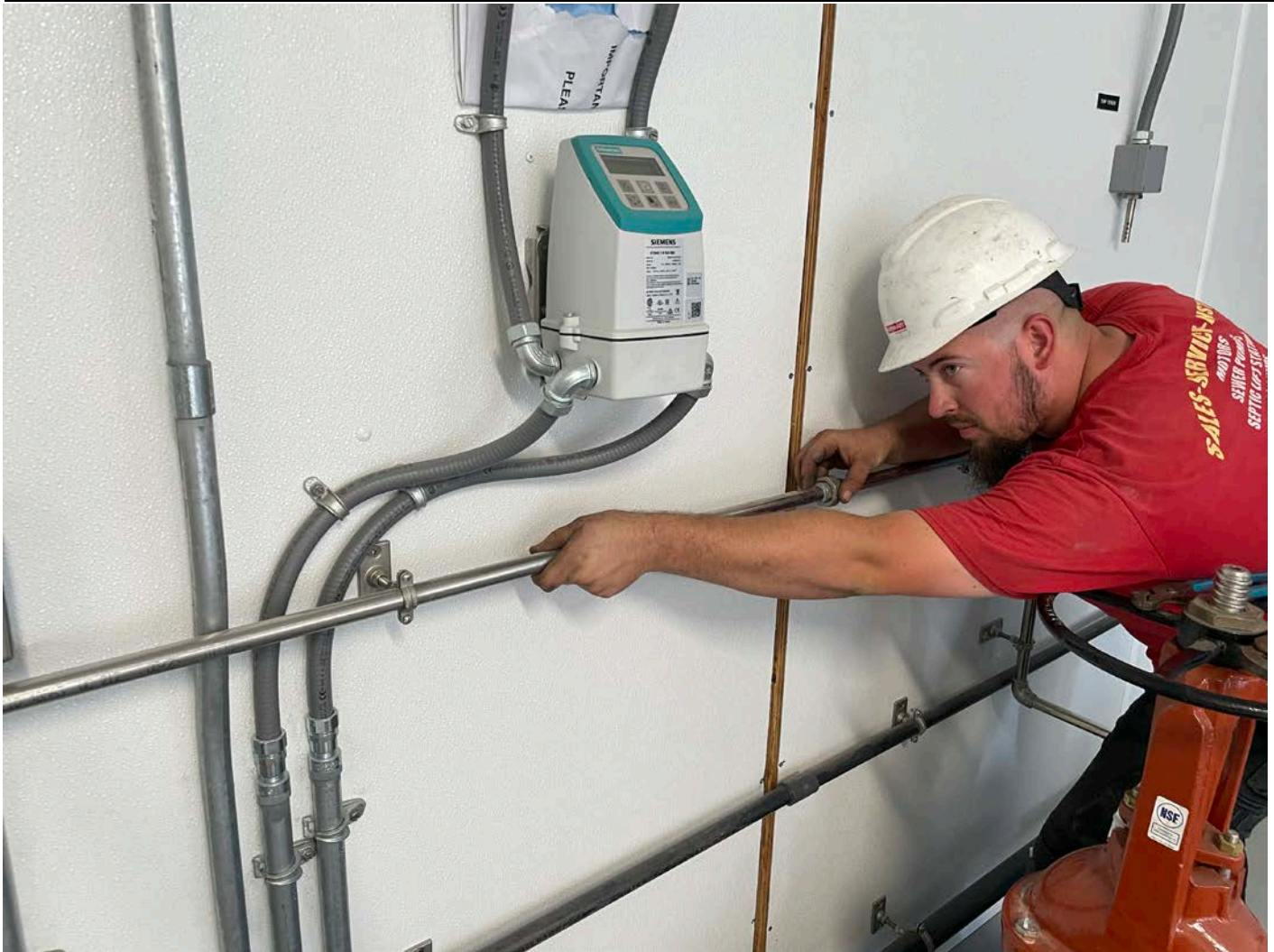
Picture 5: United Concrete installing water sampling feed line to the sink located on the east side of the booster station located at Station 750+63. View to the southeast.
