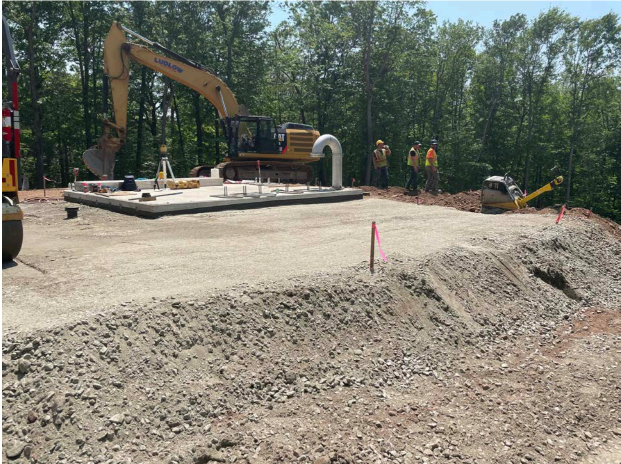
Picture 8: View of fill Ludlow has placed around the altitude valve vault on the west side of the water tank located east of the Shared Access Driveway in Middletown. View to the southwest.
