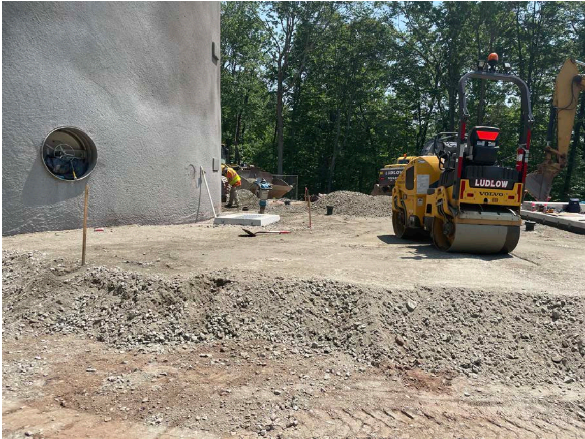
Picture 7: View of fill Ludlow has placed around the altitude valve vault on the west side of the water tank located east of the Shared Access Driveway in Middletown. View to the south.
