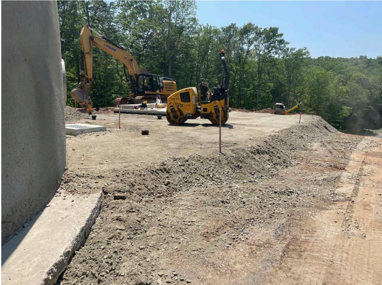
Picture 6: View of fill Ludlow has placed around the altitude valve vault on the west side of the water tank located east of the Shared Access Driveway in Middletown. View to the southwest.
