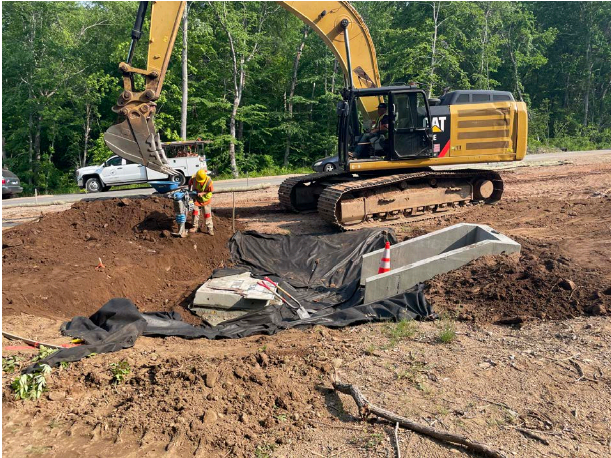
Picture 1: Ludlow compacting fill with a jumping jack on the northwest side of the plunge pool located at ~Station 11+60. View to the north.
