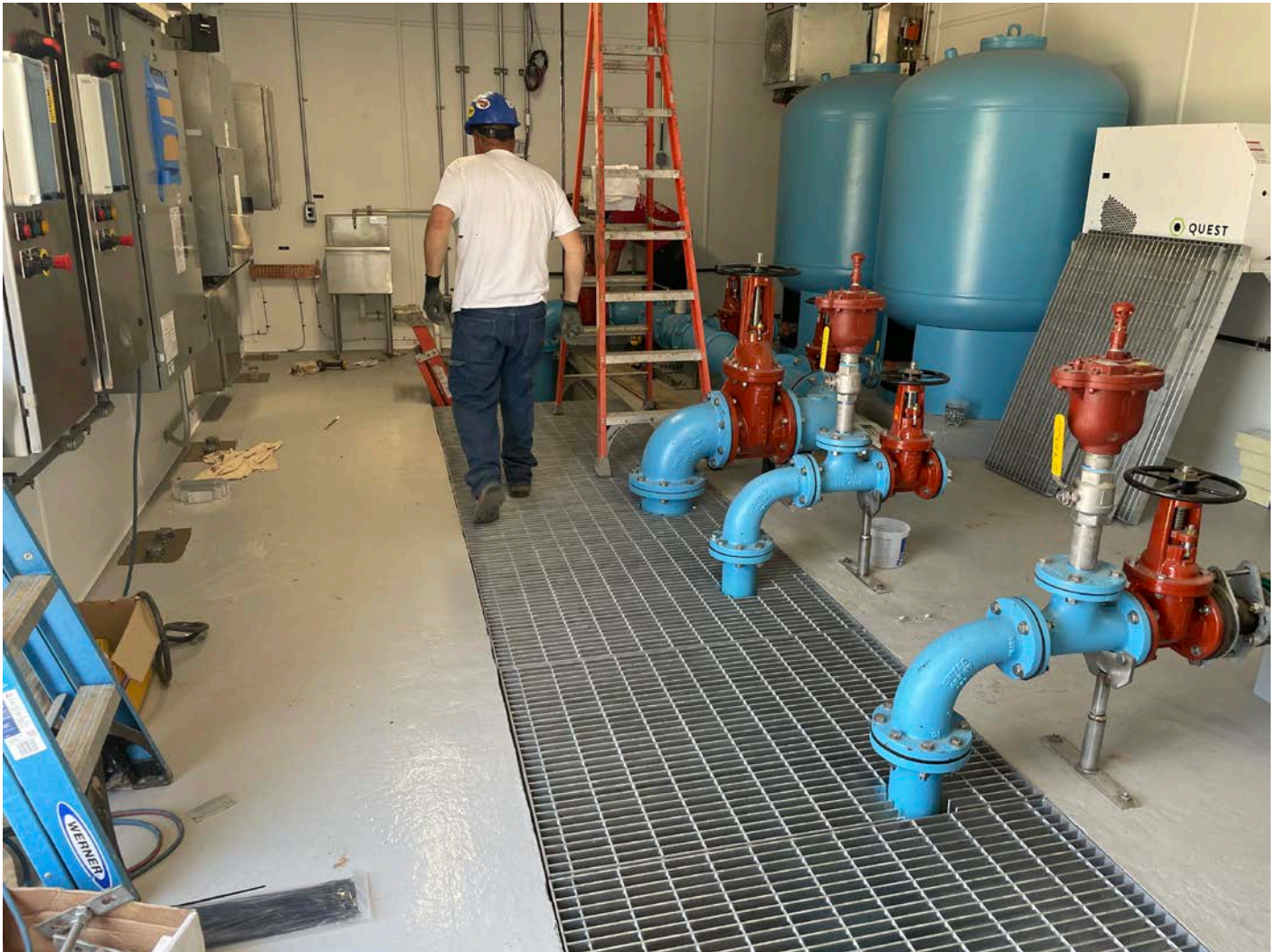
Picture 4: United Concrete has placed grating over the pipe trough in the booster station located at Station 750+63 in Middletown. View to the east.
