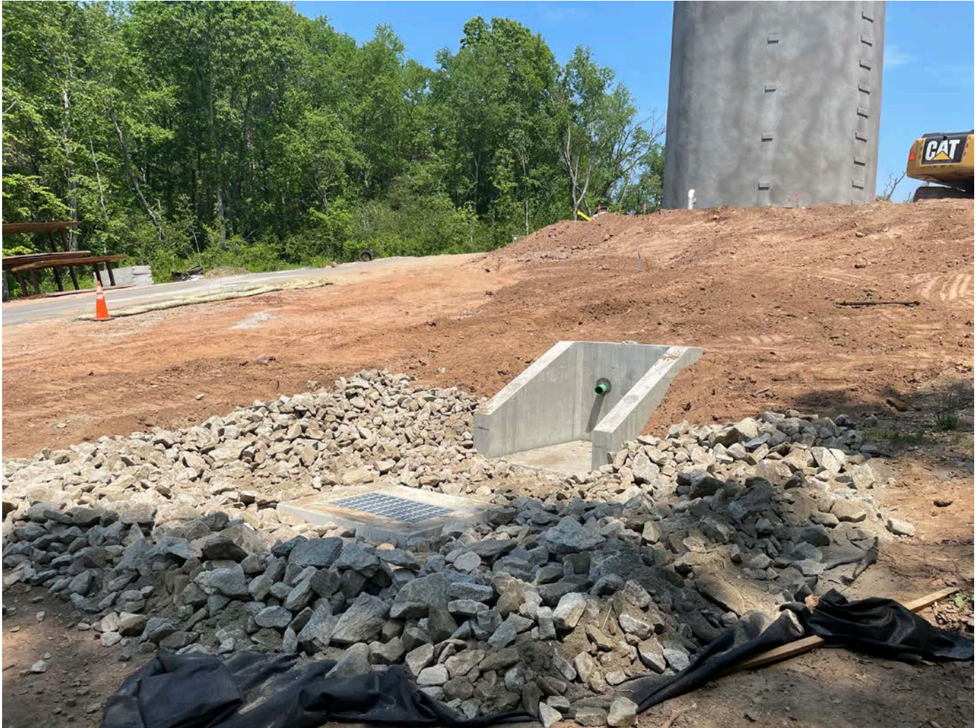
Picture 10: View of the headwall, catch basin, and plunge pool located west of the water tank. View to the northeast.
