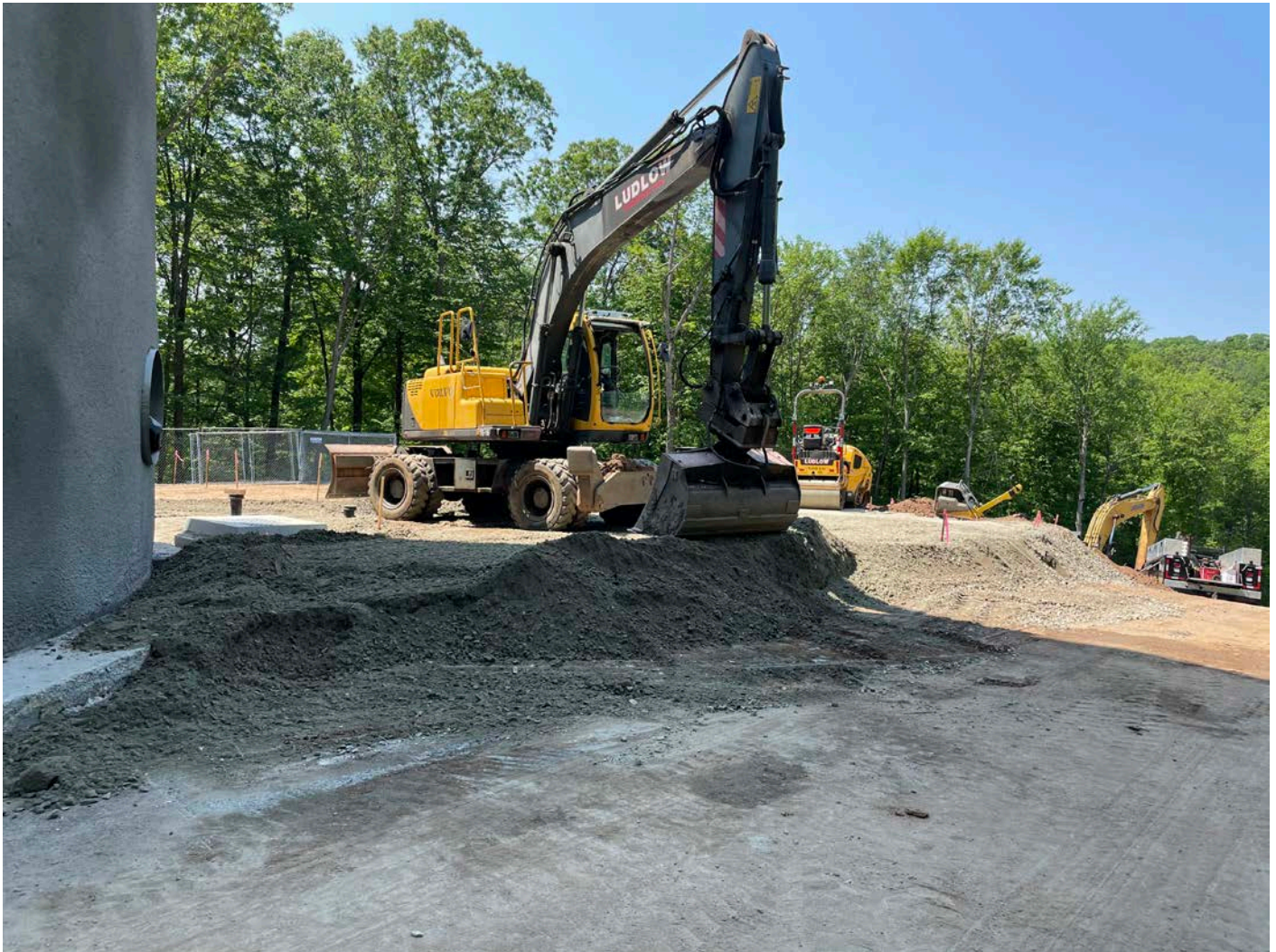
Picture 3: Ludlow placing fill in 1' lifts to raise the grade around the altitude vault on the west side of the water tank located east of the Shared Access Driveway in Middletown. View to the southwest.
