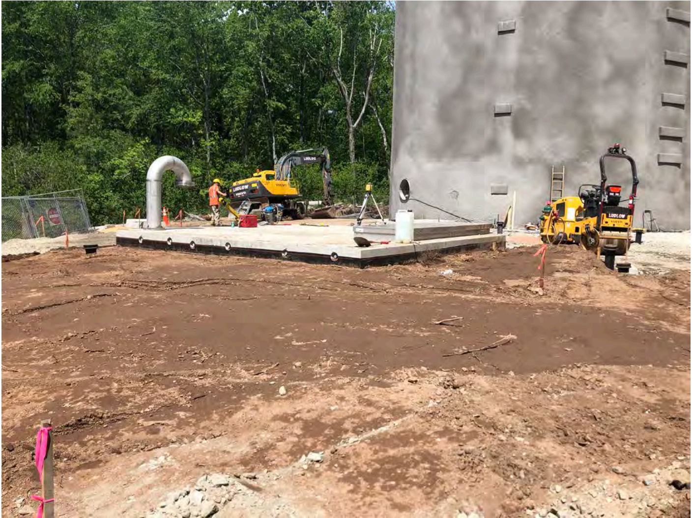
Picture 11: Ludlow backfilling, grading and compacting around the altitude valve vault west of the water tank. View to the east.
