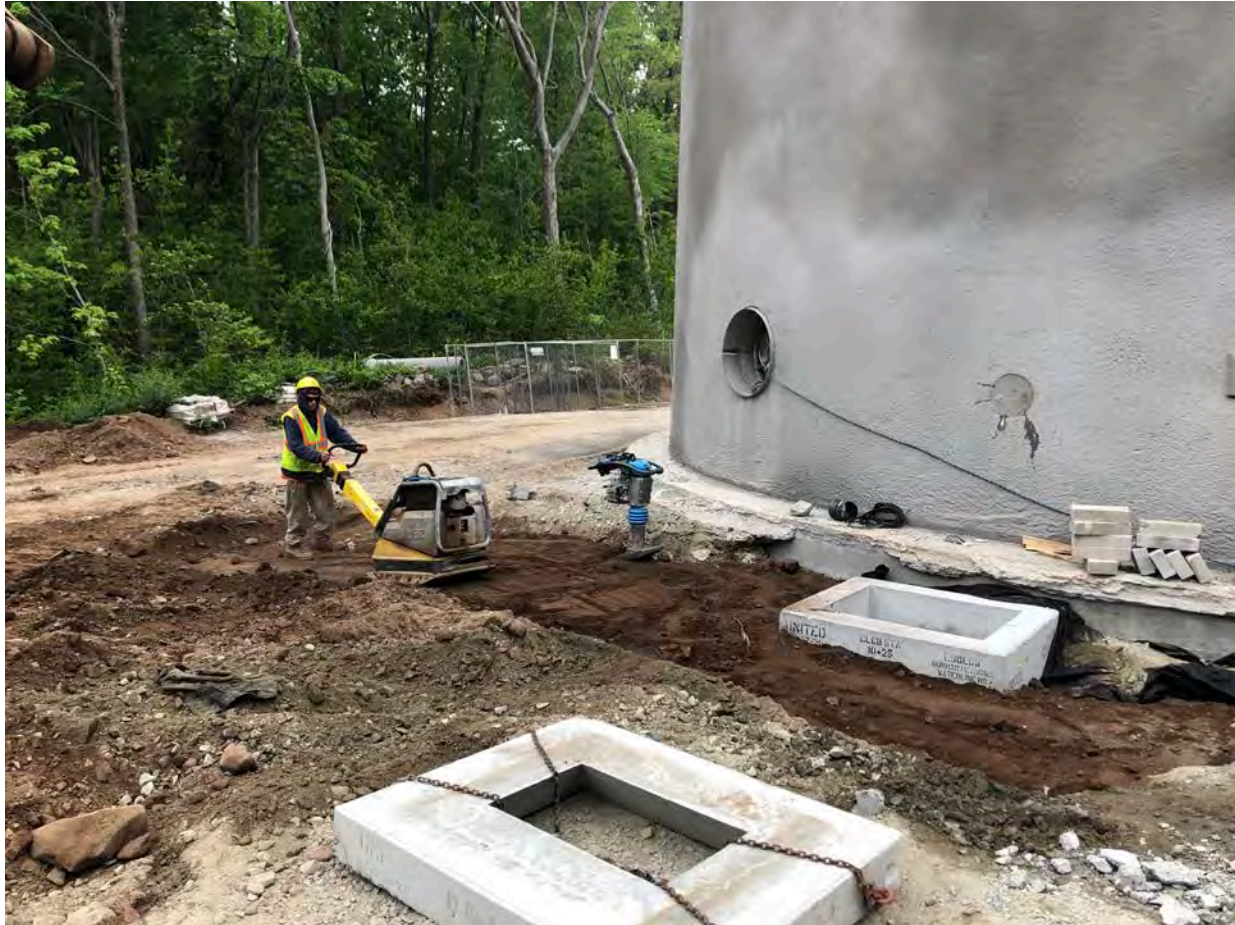
Picture 2: Ludlow compacting fill with a plate compactor on the west side of the water tank in Middletown. View to the northeast.
