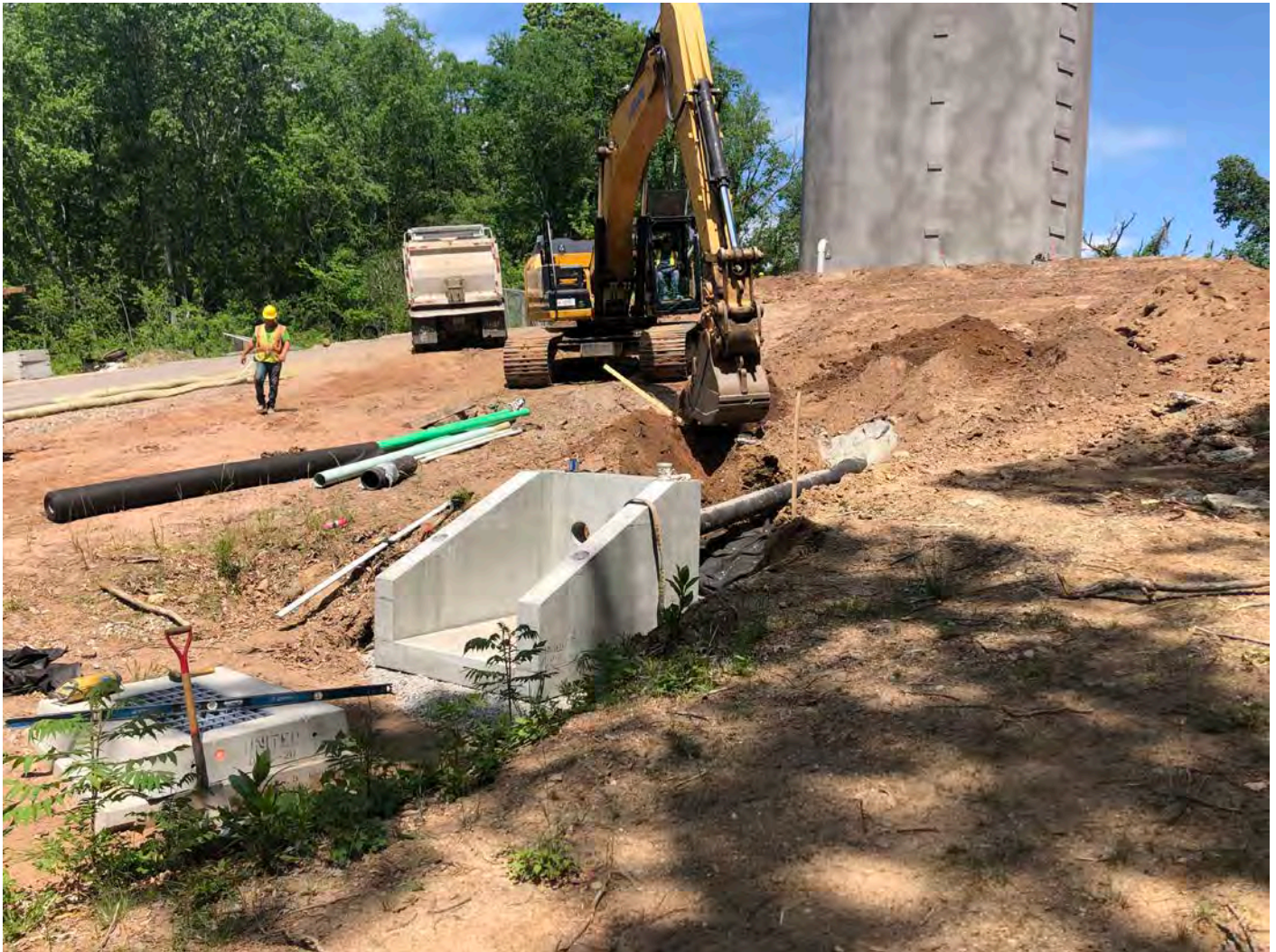
Picture 10: Ludlow excavating to install tank drain pipe to headwall at the water tank site. View to the east.
