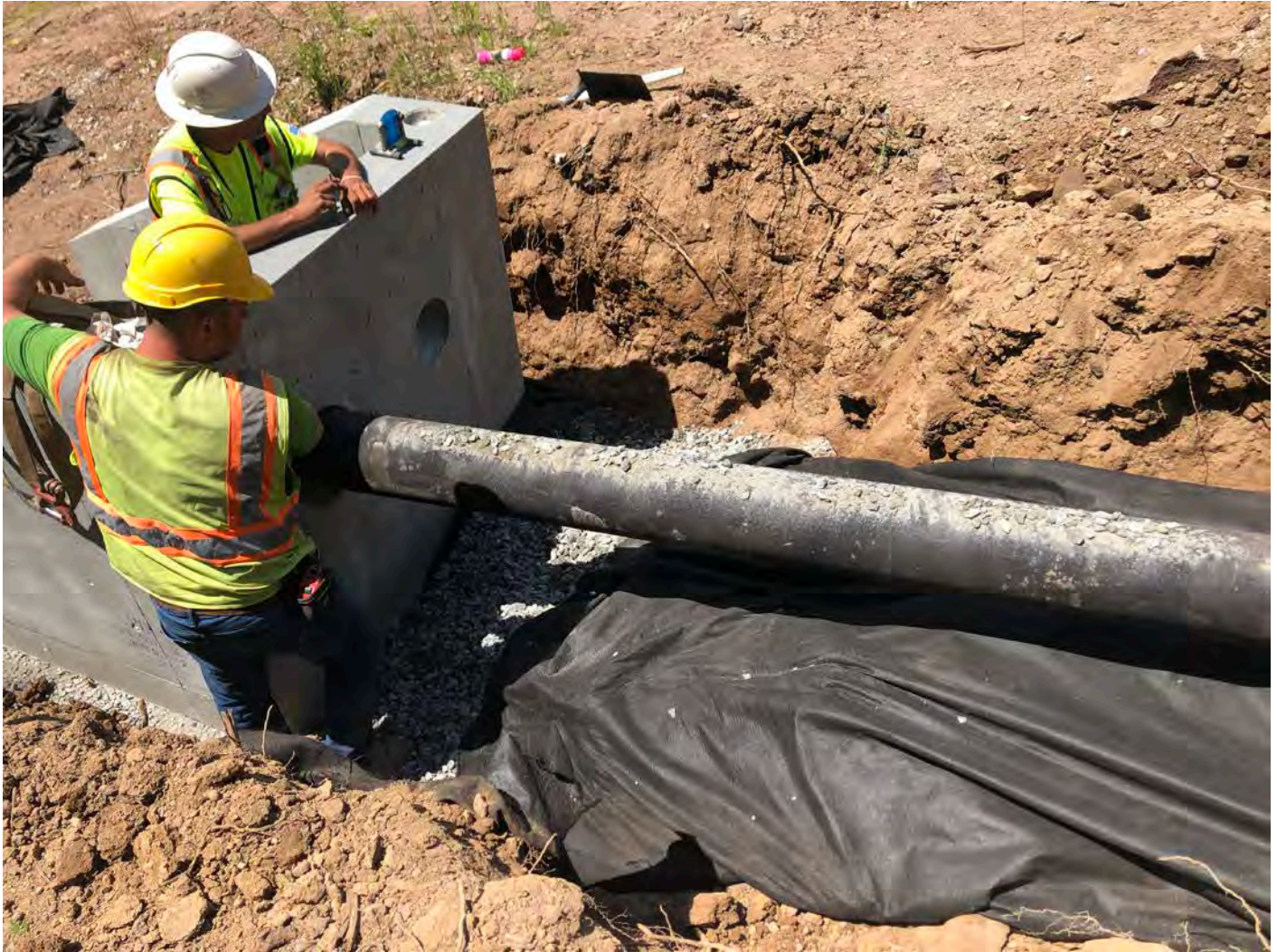
Picture 9: Ludlow in the process of installing 8" DIP to connect to the headwall they just installed at Station 11+50. View to the north.
