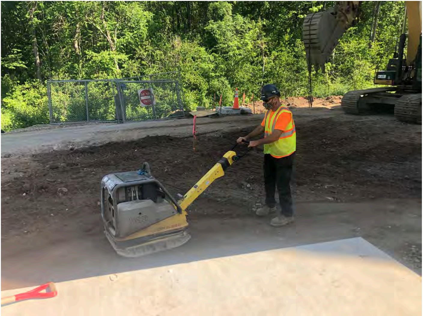
Picture 4: Ludlow compacting fill with a plate compactor on the northwest side of the water tank in Middletown. View to the north.
