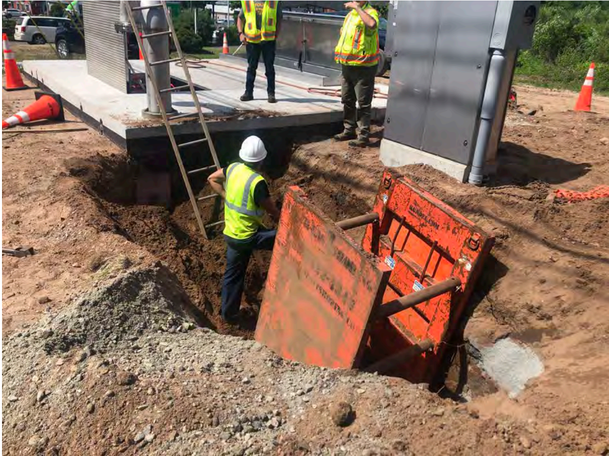
Picture 6: Ludlow excavating on the northeast corner of the pressure reducing valve vault as they attempt to troubleshoot difficulties in conducting a pressure test on the piping associated with the vault. ~Station 161+40, Durham. View to the south.
