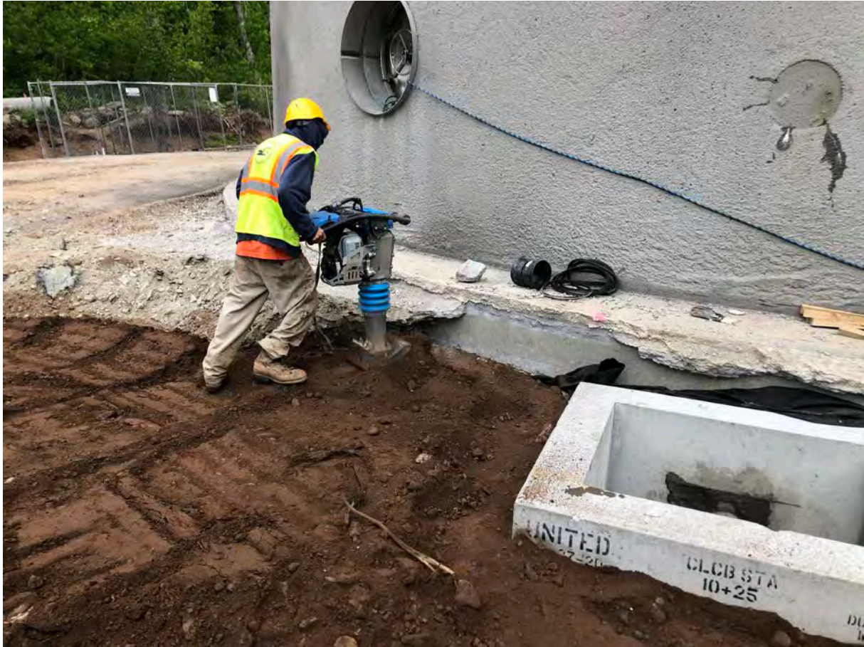
Picture 1: Ludlow compacting fill with a jumping jack on the west side of the water tank in Middletown. View to the northeast.
