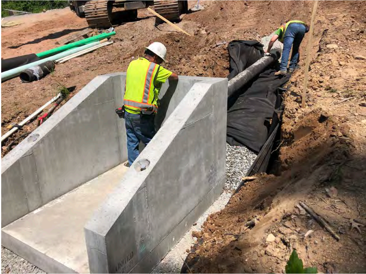
Picture 8: Ludlow in the process of installing 8" DIP to connect to the headwall they just installed at Station 11+50. View to the northeast.
