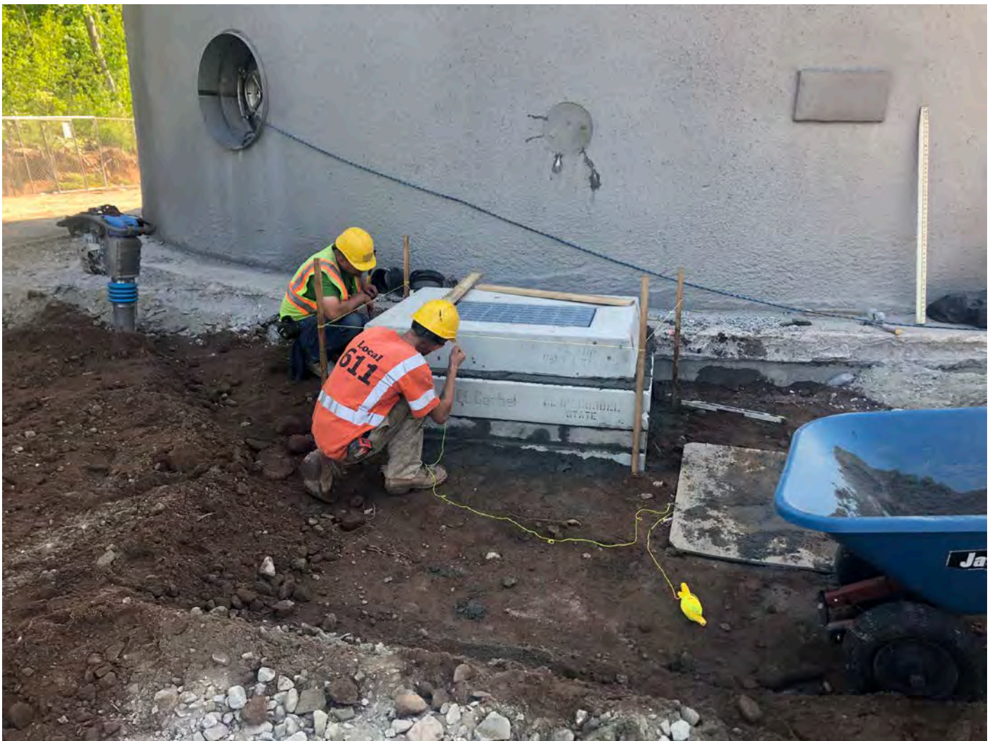
Picture 3: Ludlow applying mortar to the top sections of the catch basin located at Station 10+25 on the west side of the water tank located east of the Shared Access Driveway in Middletown. View to the east.
