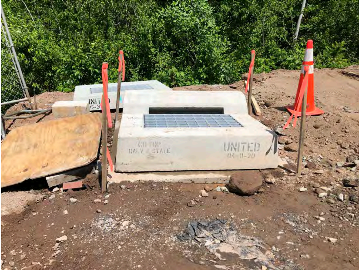
Picture 7: Ludlow changed the top to the catch basin located ~70' northwest of the water tank located east of the Shared Access Driveway in Middletown. View to the north.
