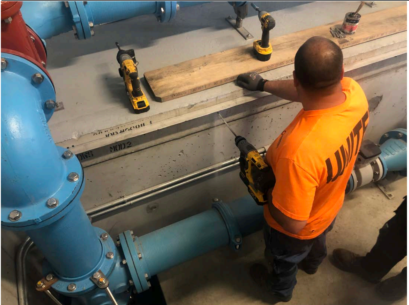
Picture 5: United Concrete installing support bracket for the grating that will sit over the trough in the booster station located at Station 750+63.
