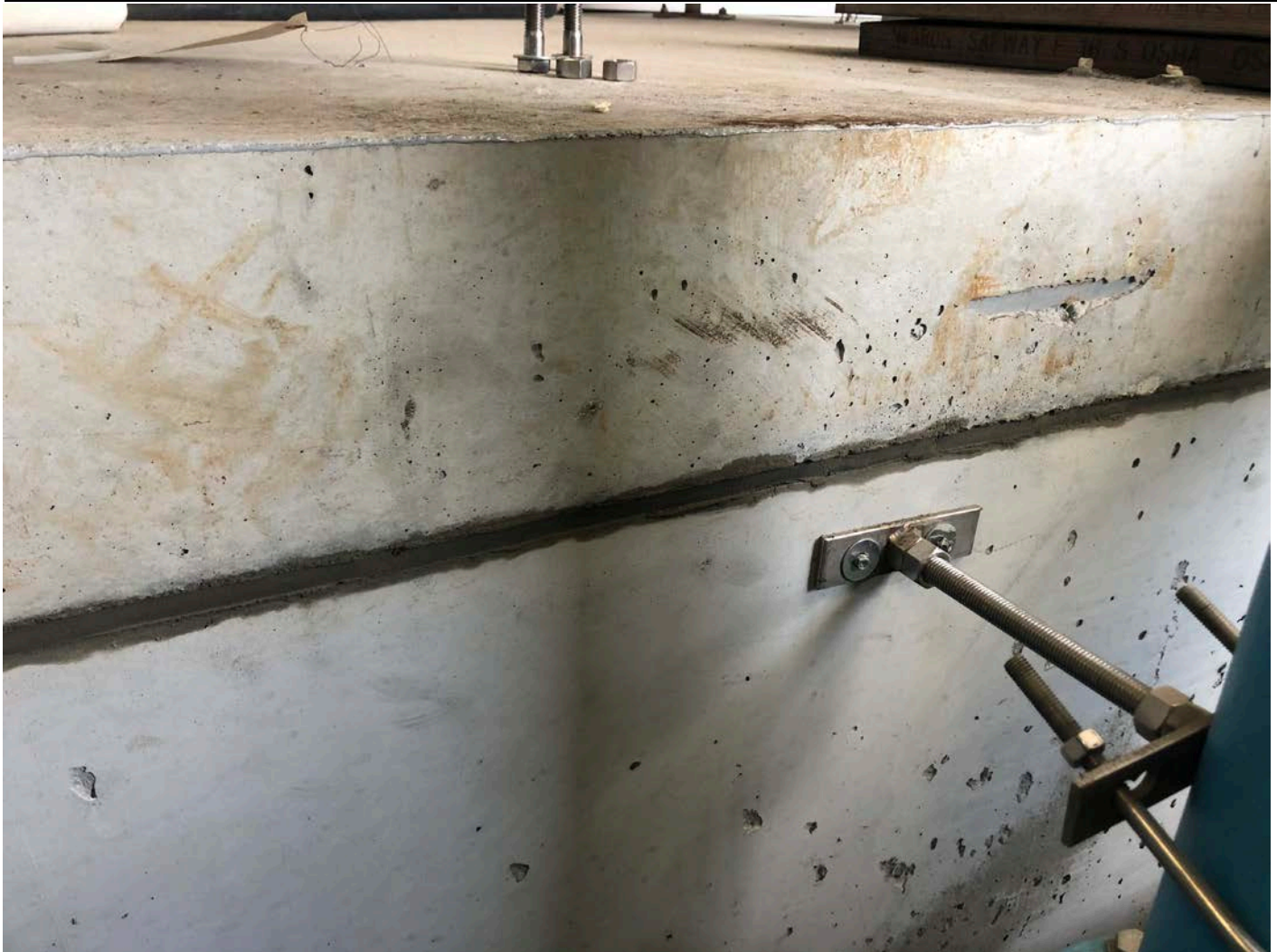
Picture 5: The gap between the top of the trough and the underside of the booster station. United Concrete used Harris Construction grout with some Euclid Chemical Speed plug (rapid-setting hydraulic water stop) to fill the gap.
