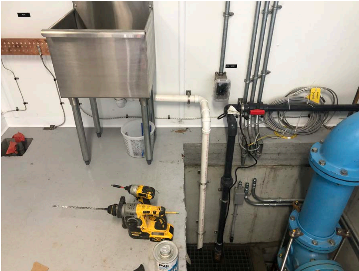
Picture 7: The east side of the booster station interior where United Concrete has installed PVC for the sink drain, and has completed the PVC discharge connection to the sump pump. View to the east.
