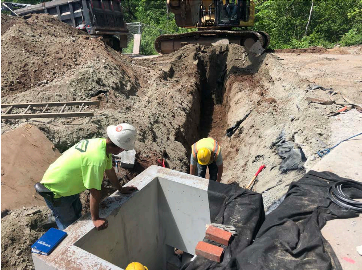
Picture 8: Ludlow beginning to place 12" RCP from the catch basin located at Station 10+25 to another catch basin located approximately 75' northwest of the water tank (on the north side of the Shared Access Driveway). View to the north.
