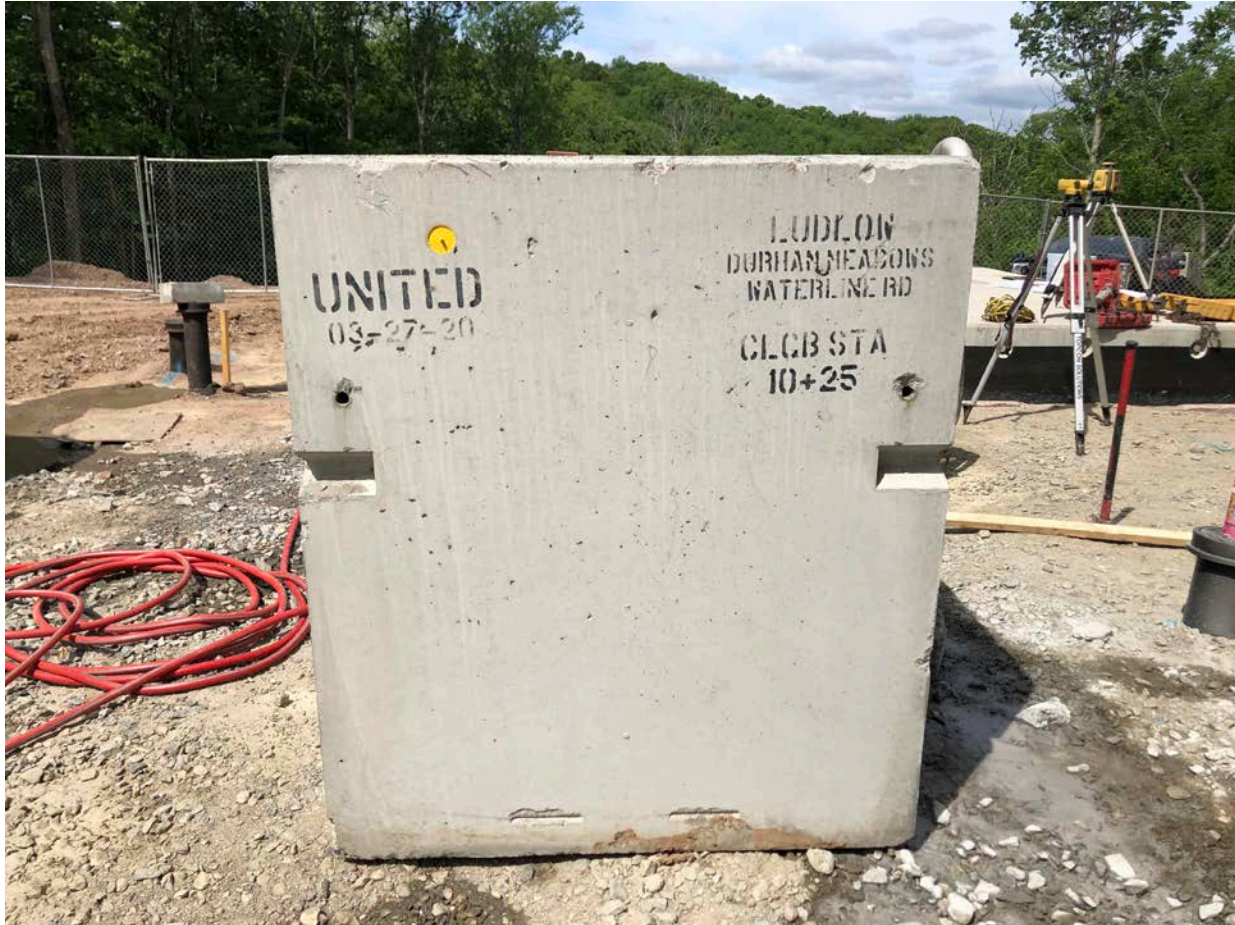
Picture 2: Catch basin that Ludlow is preparing to install Station 10+25 into the excavation located on the west side of the water tank in Middletown.
