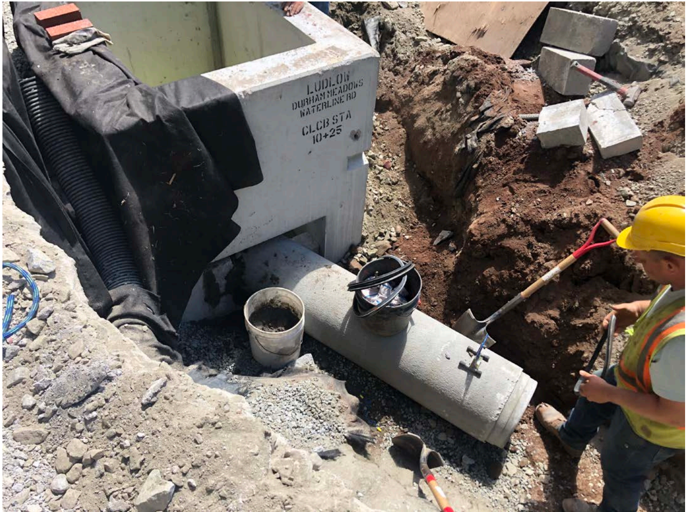
Picture 9: Ludlow placing 12" RCP from the catch basin located at Station 10+25 to another catch basin located approximately 75' northwest of the water tank (on the north side of the Shared Access Driveway). View to the west.
