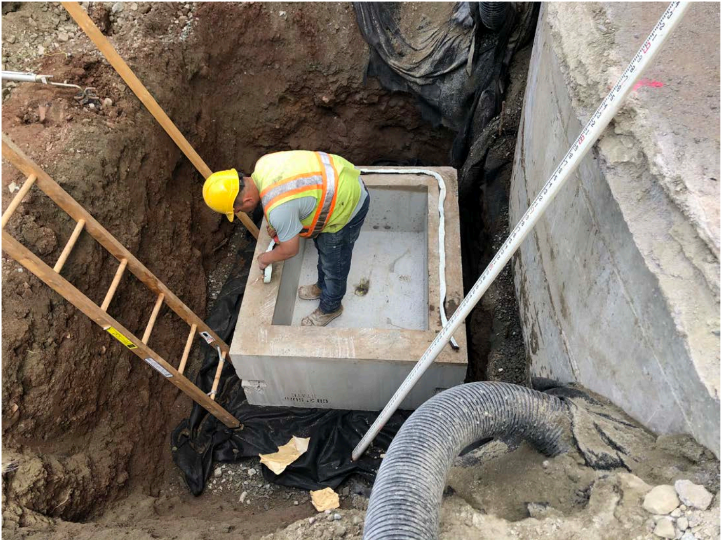
Picture 3: Ludlow applying ConSeal tape on the top rim of the catch basin sump located at Station 10+25 on the west side of the water tank located east of the Shared Access Driveway in Middletown. View to the north.
