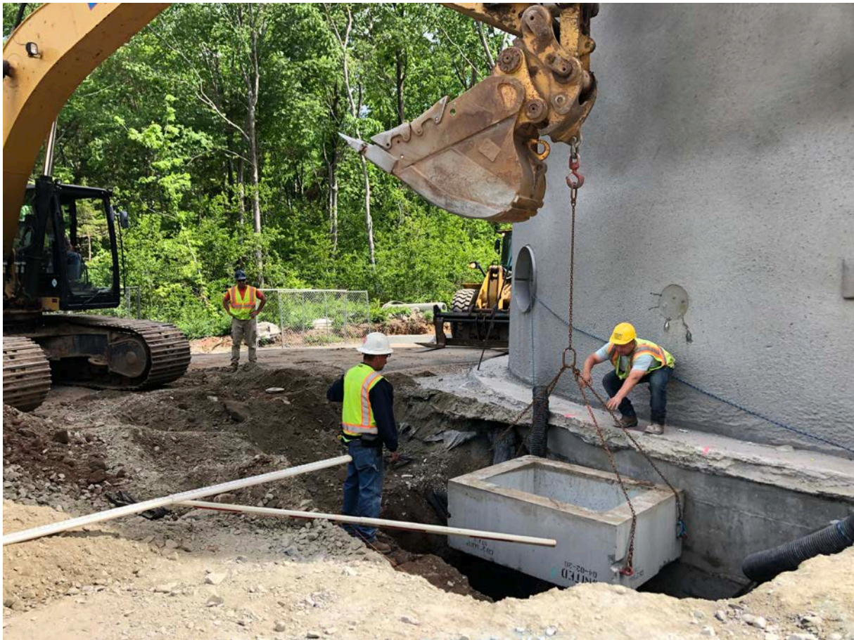
Picture 1: Ludlow placing a catch basin sump at Station 10+25 into the excavation located on the west side of the water tank in Middletown. View to the northeast.
