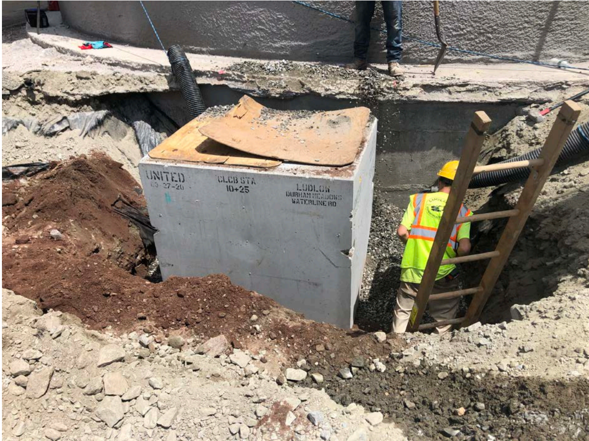
Picture 6: Catch basin that has just been placed at Station 10+25 on the west side of the water tank located east of the Shared Access Driveway in Middletown. View to the east.
