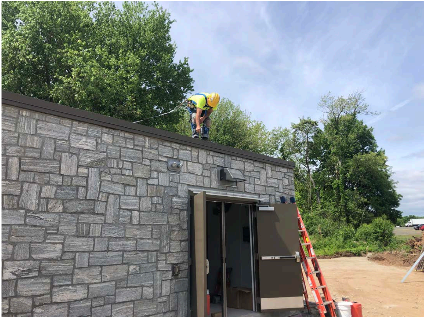
Picture 4: United Concrete installing flashing on the booster station roof. Station 750+63 in Middletown.
