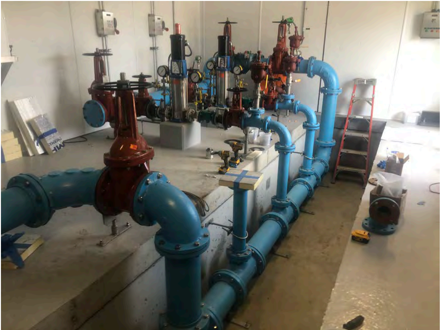
Picture 3: View of the interior of the booster station as United Concrete installs elbows on piping within the trough. View to the east.
