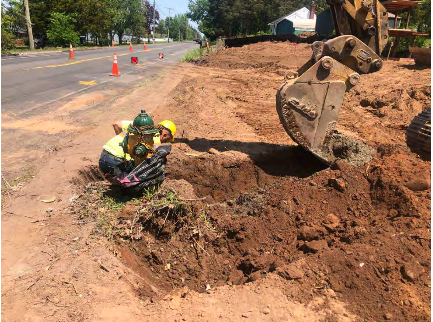
Picture 9: Ludlow temporarily removing a hydrant at the water meter building work zone located at ~Station 124+80 in Middletown. View to the north.
