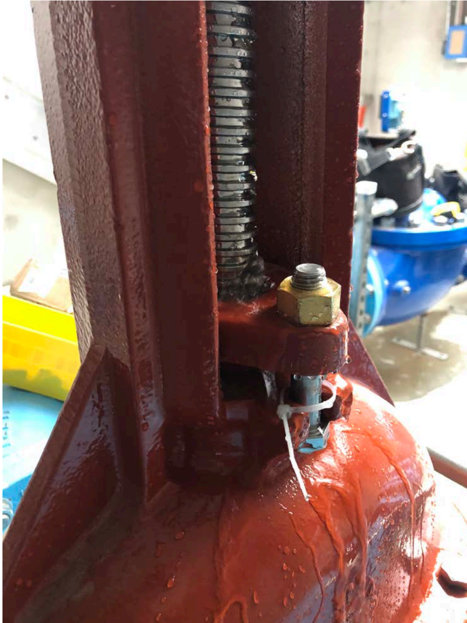
Picture 1: 12" gate valve located inside of the altitude valve vault that began to leak when Ludlow was setting up to perform a pressure test.
