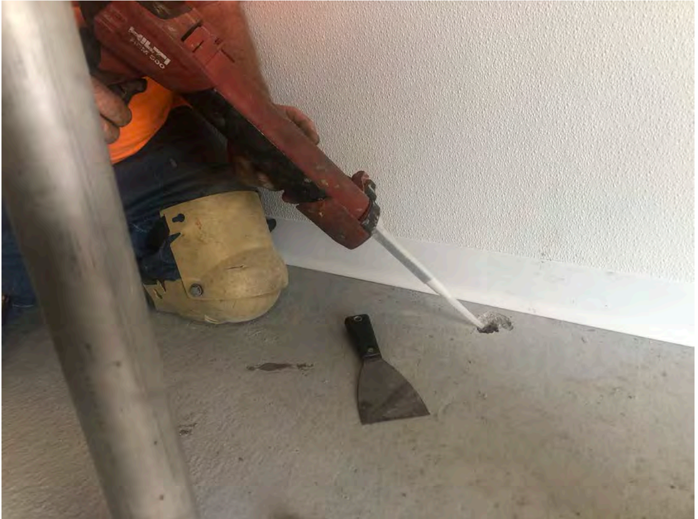
Picture 4: United Concrete filling holes in the booster station floor with Hilti – HIT HY 200-A (injectable hybrid mortar) where segments of rebar penetrate the floor and go into the top of the frost wall.
