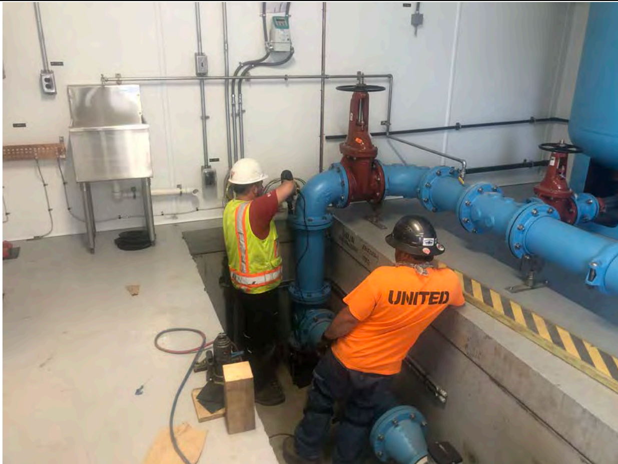
Picture 2: United Concrete installing an elbow at the booster station located at Station 750+63.
