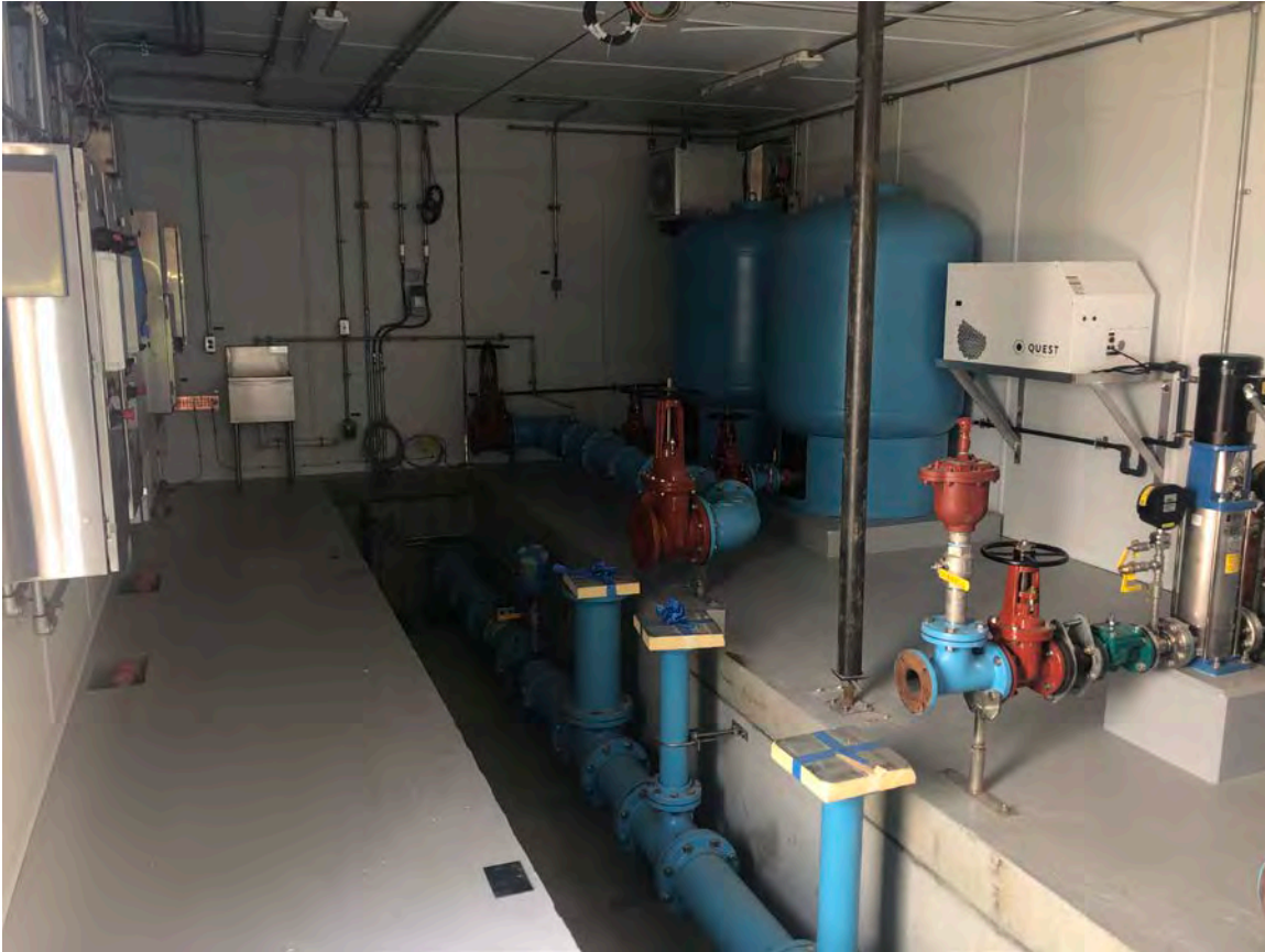
Picture 7: View of the interior of the booster station, looking to the east. Station 750+63, Middletown.
