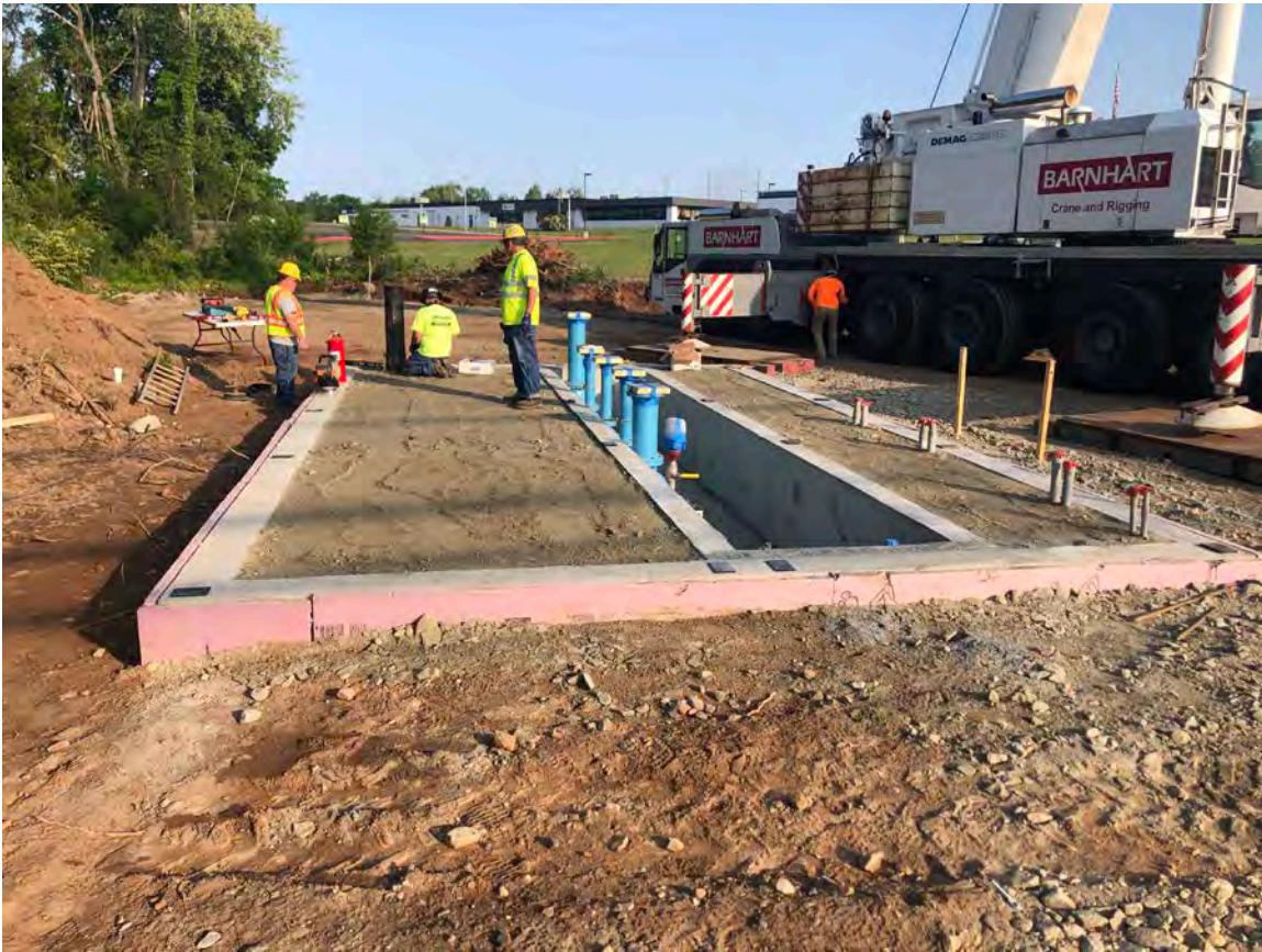
Picture 1: View of the booster station after fill was placed and compacted on either side of the trough. Station 750+63, Middletown. View to the west.
