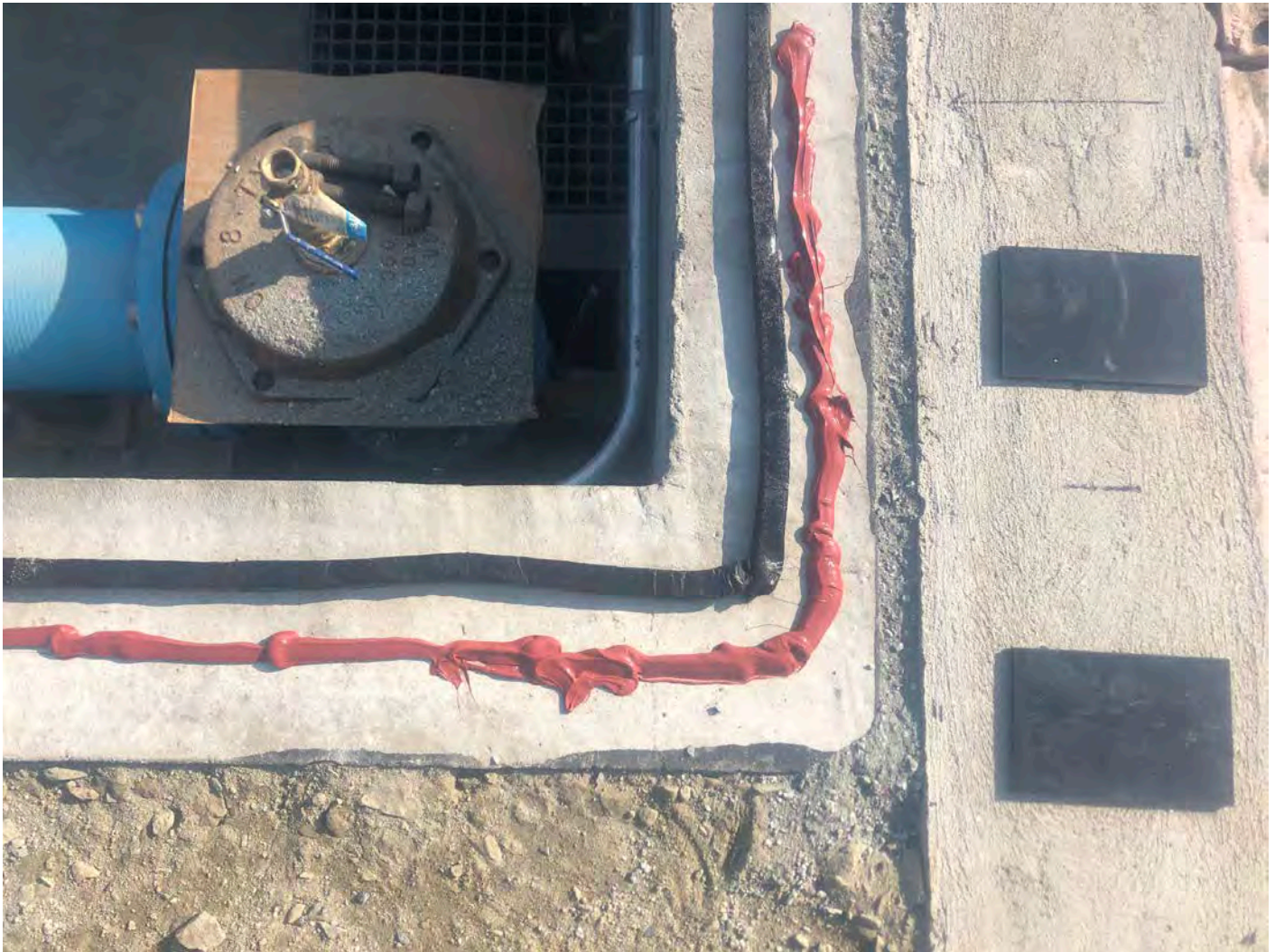
Picture 3: SikaSwell S-2 (polyurethane-based waterstop) that United Concrete applied to the top of the frost wall ahead of the placement of the booster station section placed today (view of southeast corner of the frost wall).
