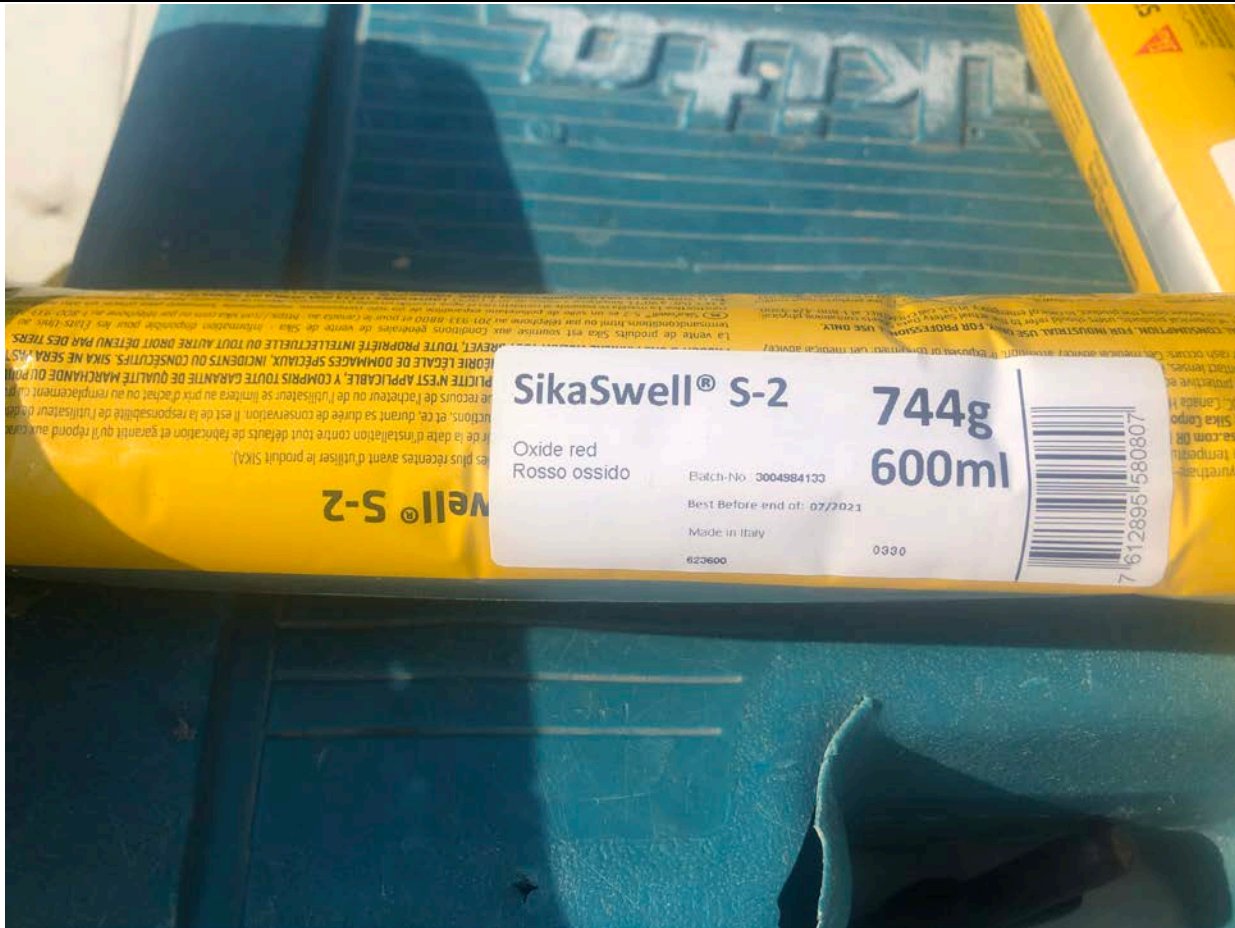
Picture 2: SikaSwell S-2 (polyurethane-based waterstop) that United Concrete applied to the top of the frost wall ahead of the placement of the booster station section placed today.
