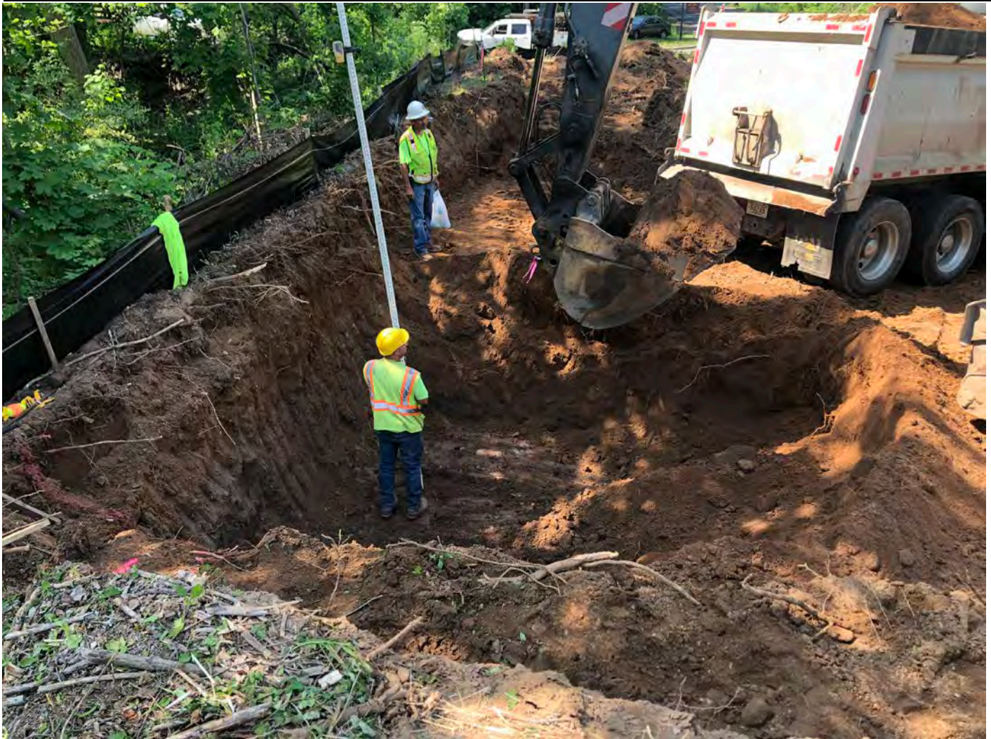
Picture 5: View of the earthwork being performed by Ludlow at the water meter building located at ~Station 124+80 in Middletown. View to the south.
