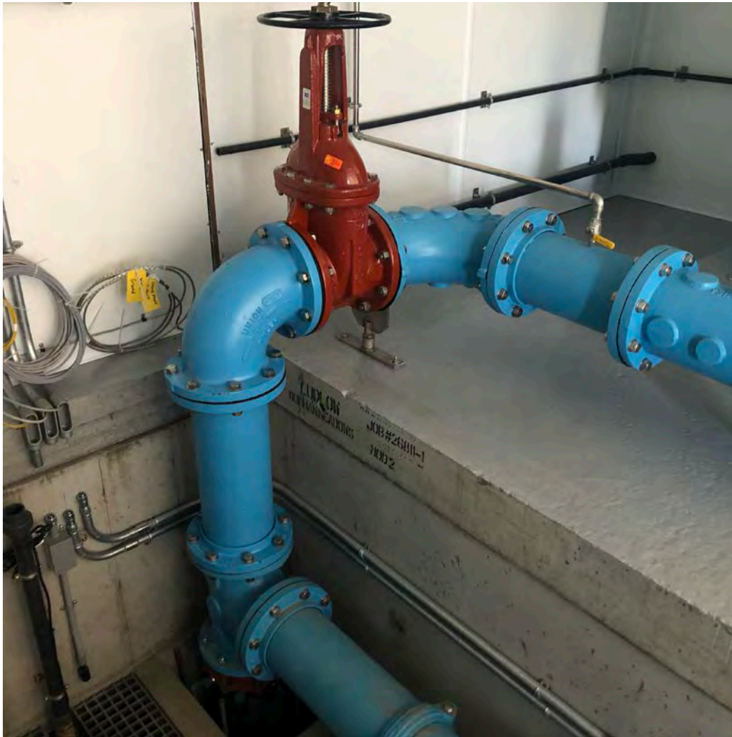
Picture 13: DIP elbow that United Concrete has installed on the east side of the booster station building. View to the east/southeast.
