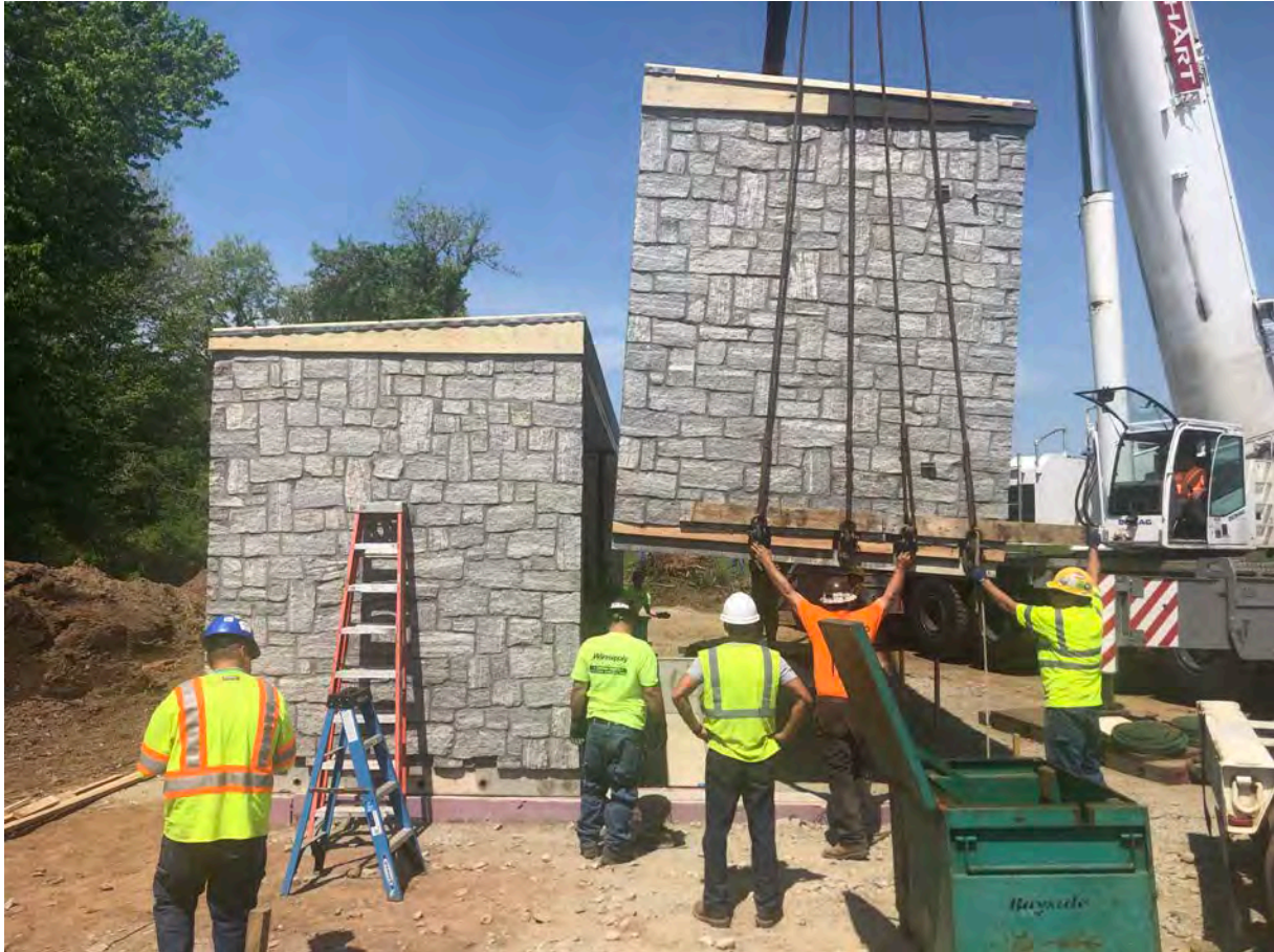
Picture 6: United Concrete positioning the second half of the booster station building as Barnhart performs the lift at the booster station work zone. View to the west.
