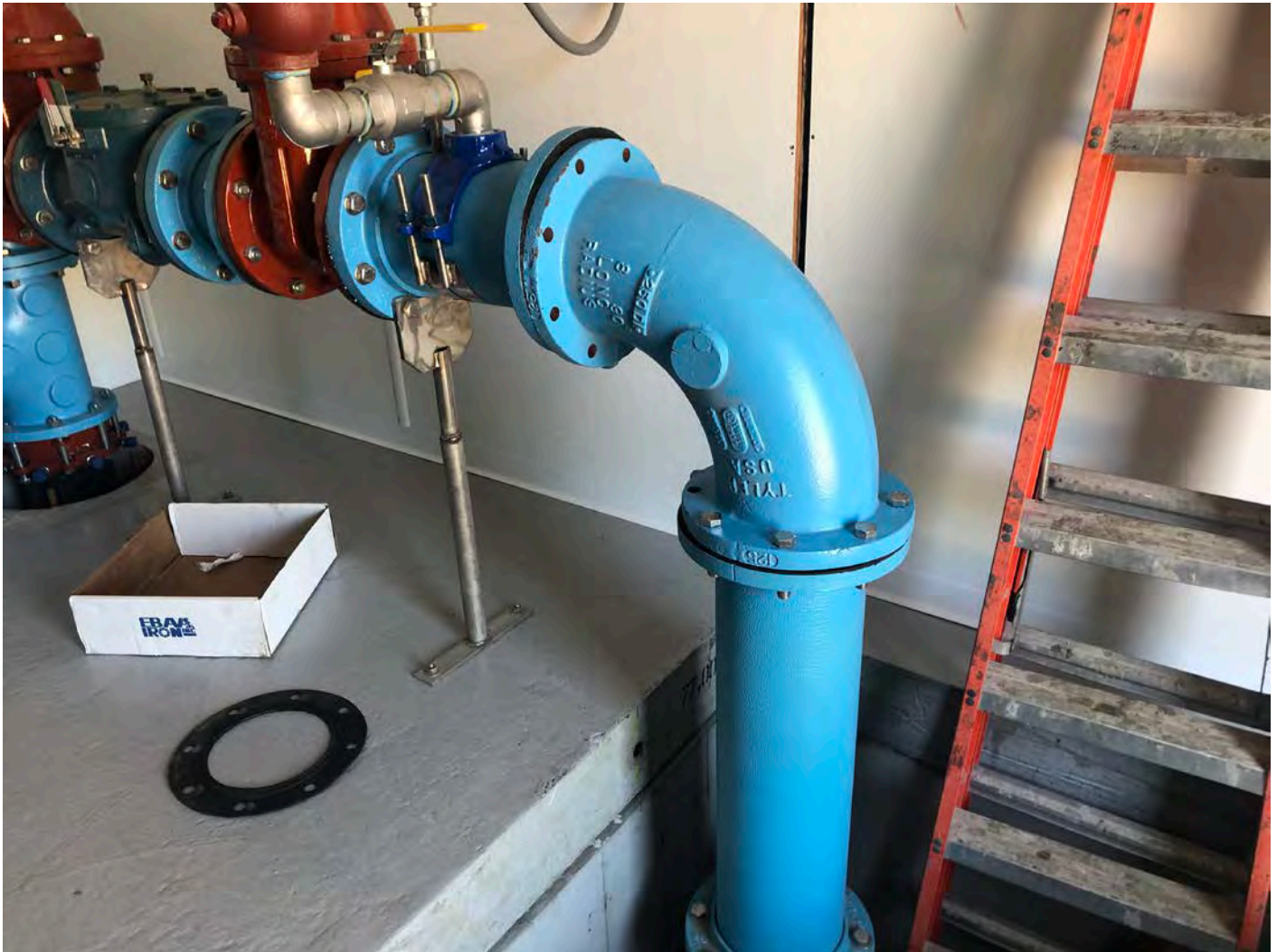
Picture 12: DIP elbow that United Concrete has installed on the west side of the booster station building. View to the west/southwest.
