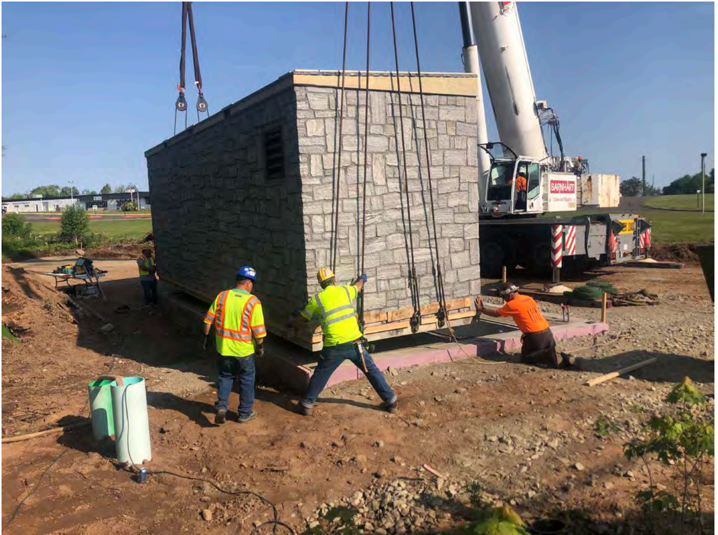
Picture 4: United Concrete positioning the first half of the booster station building as Barnhart performs the lift at the booster station work zone. View to the northwest.
