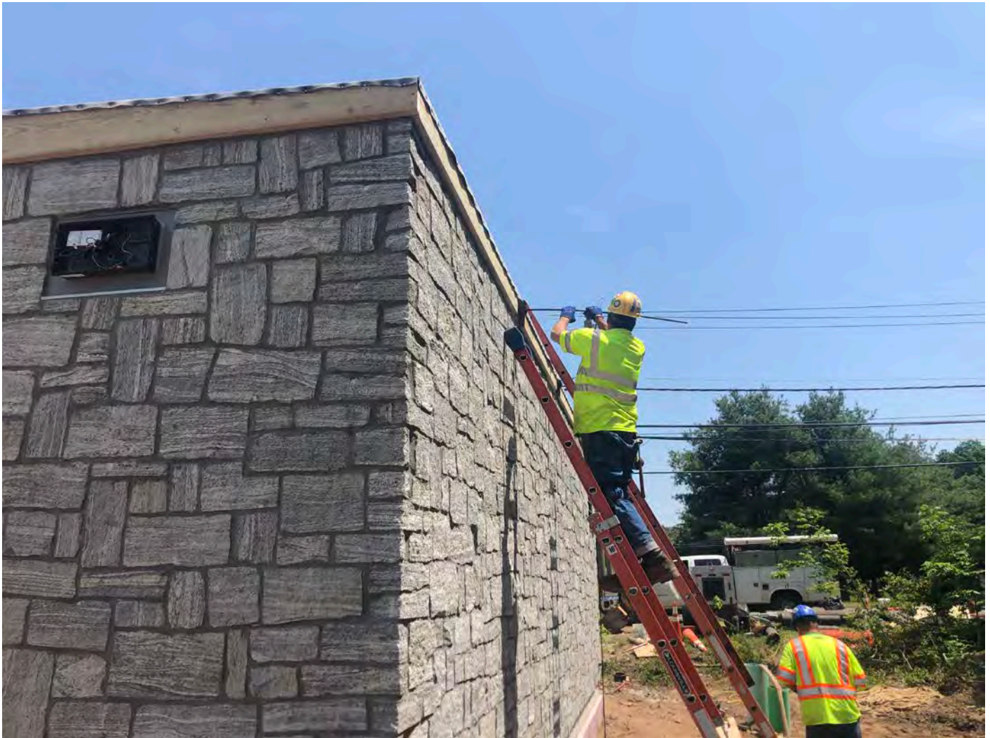
Picture 10: United Concrete running cable through the two sections of the booster station building. View to the east.
