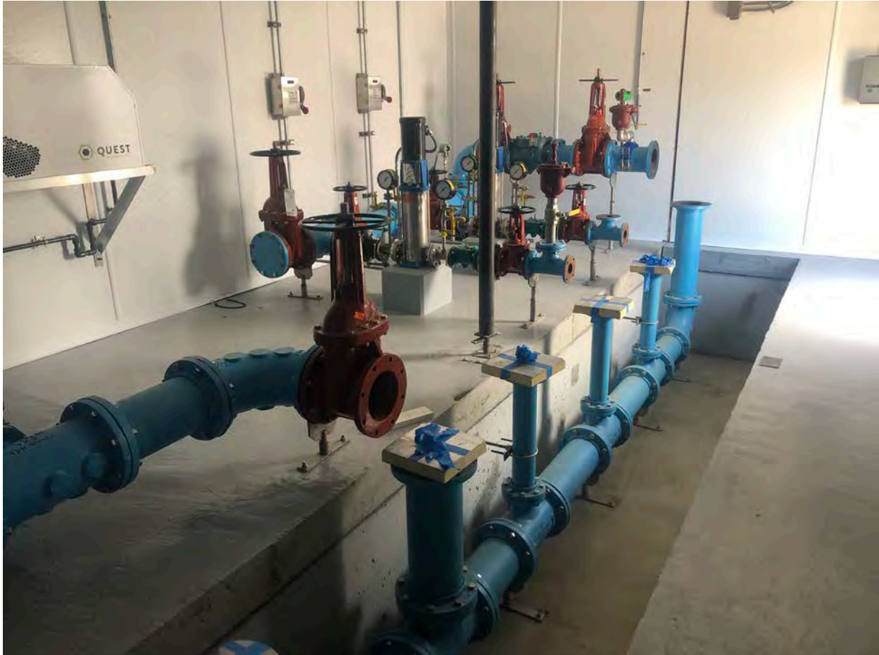
Picture 8: View of the interior of the booster station, looking to the west. Station 750+63, Middletown.
