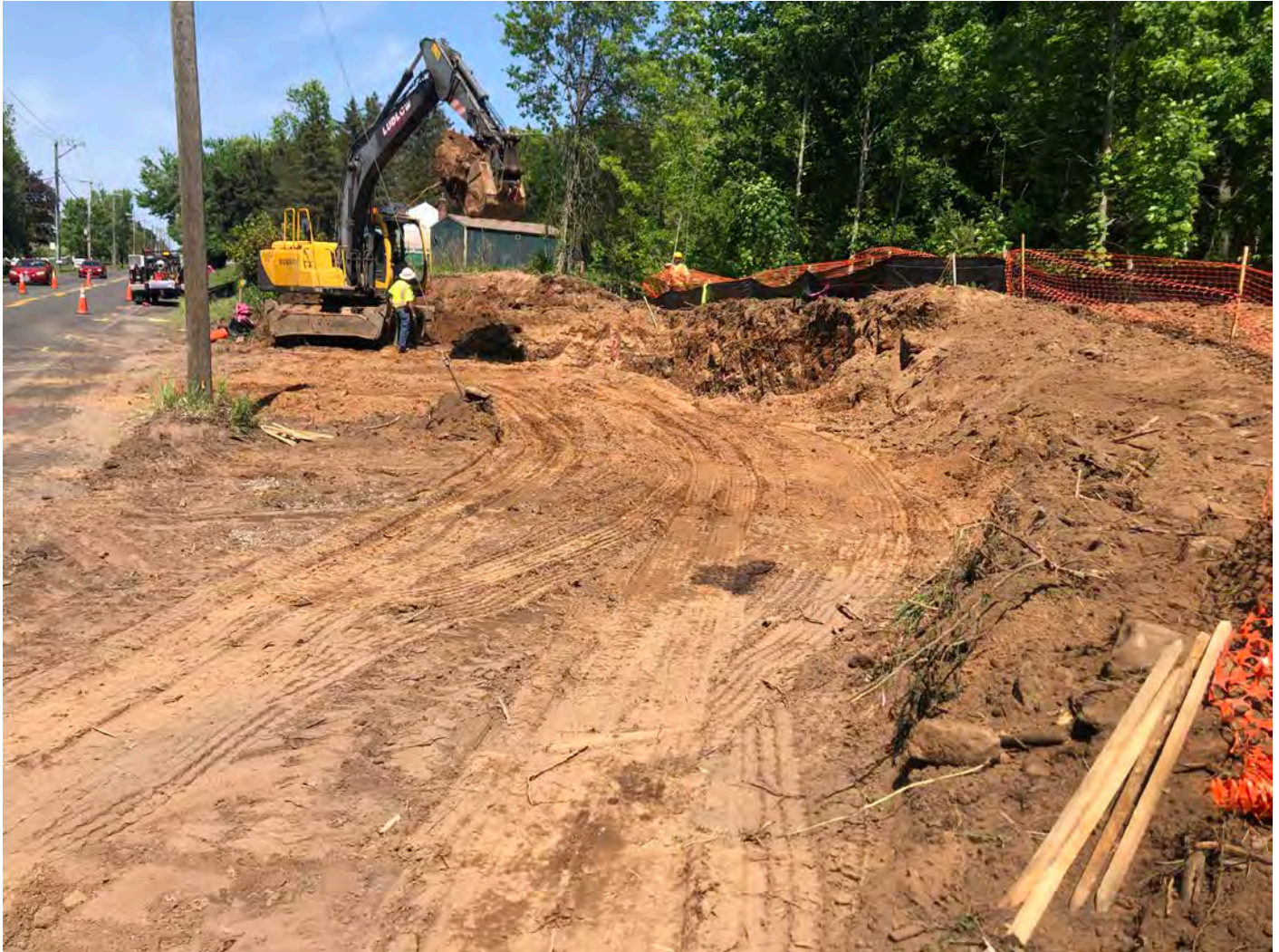
Picture 11: View of progress at the water meter building work zone located at ~Station 124+80 in Middletown. View to the north.
