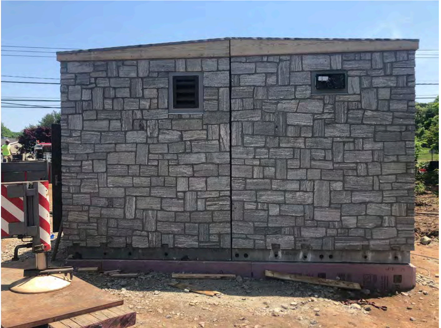
Picture 9: View of the booster station building, looking to the east. Station 750+63, Middletown.
