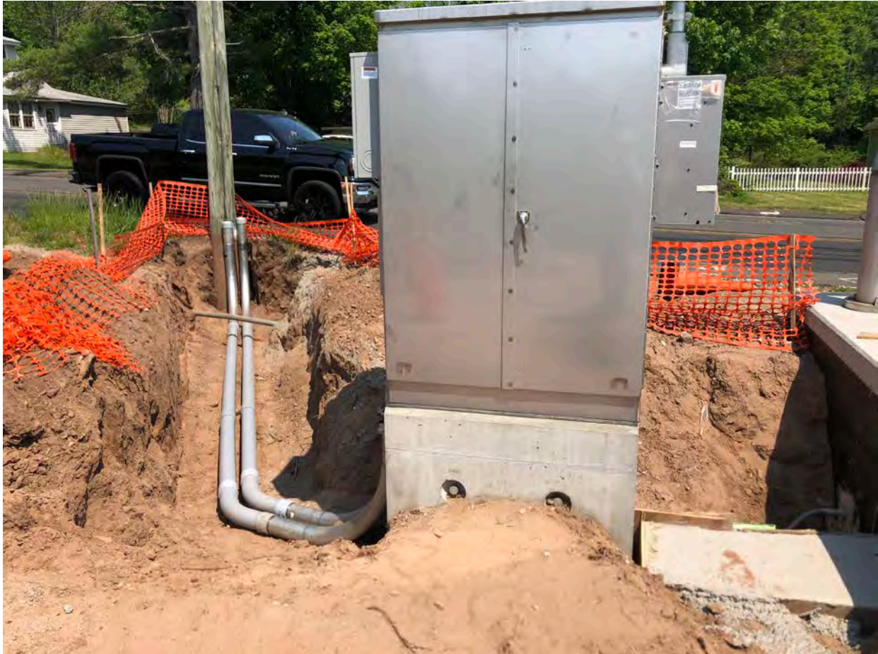
Picture 8: Overview of progress at the pressure reducing vault, where A&R Electric installed PVC conduits with steel sweeps. ~Station 161+40, Main Street, Durham. View to the east.
