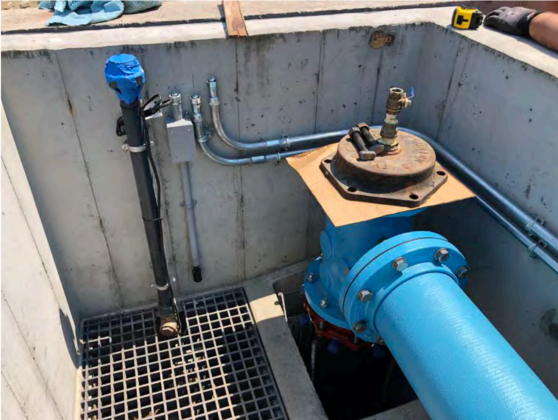
Picture 7: View of where piping that arrived within the trough is connected to the vertical section of 8" DIP located on the interior of the eastern frost wall of the booster station. Station 750+63, Middletown. View to east/southeast.
