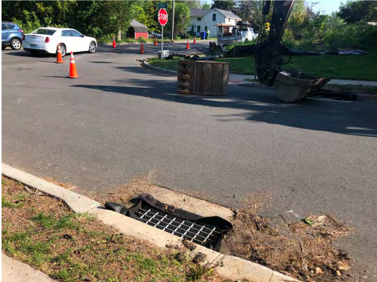
Picture 2: Geofabric placed under a catch basin grate next to the water meter building work zone located at ~Station 124+80. S. Main Street, Middletown. View to the northwest.
