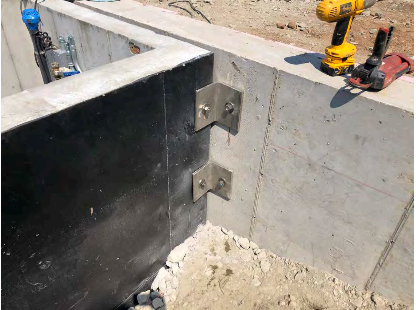
Picture 9: Metal brackets that United Concrete installed that connect the booster station frost wall to the trough they placed today.
