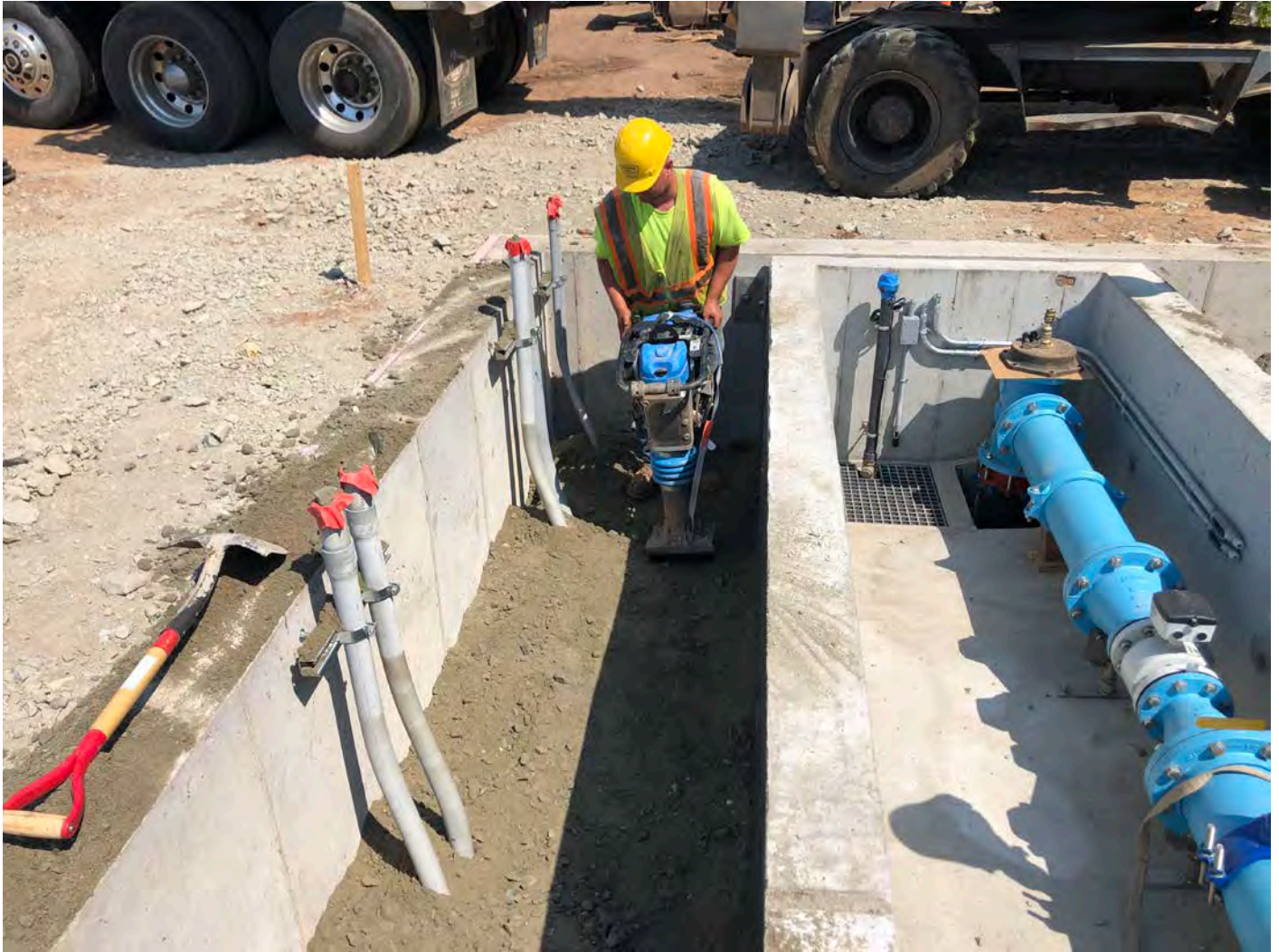
Picture 10: Ludlow compacting fill on the north side of the trough at the booster station footprint. View to the east.
