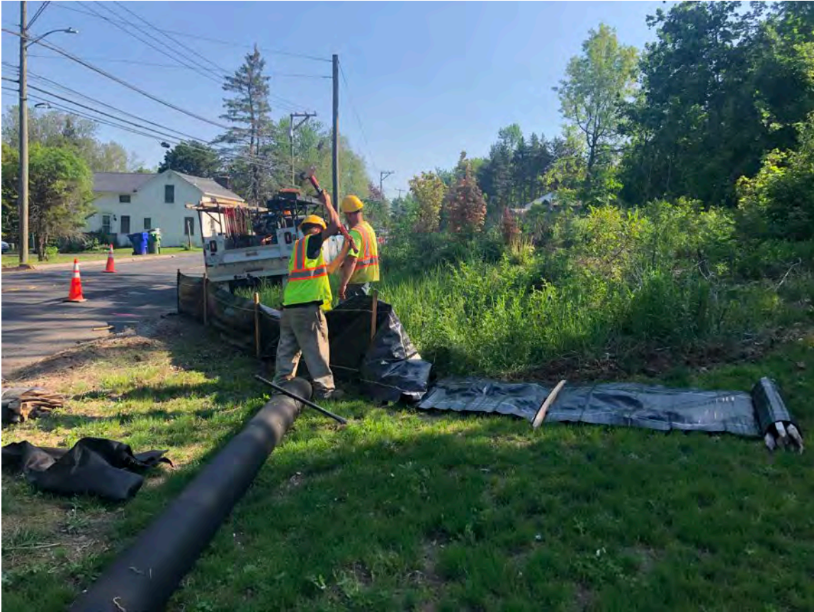
Picture 1: Ludlow installing silt fence at the water meter building work zone located at ~Station 124+80. S. Main Street, Middletown. View to the north.
