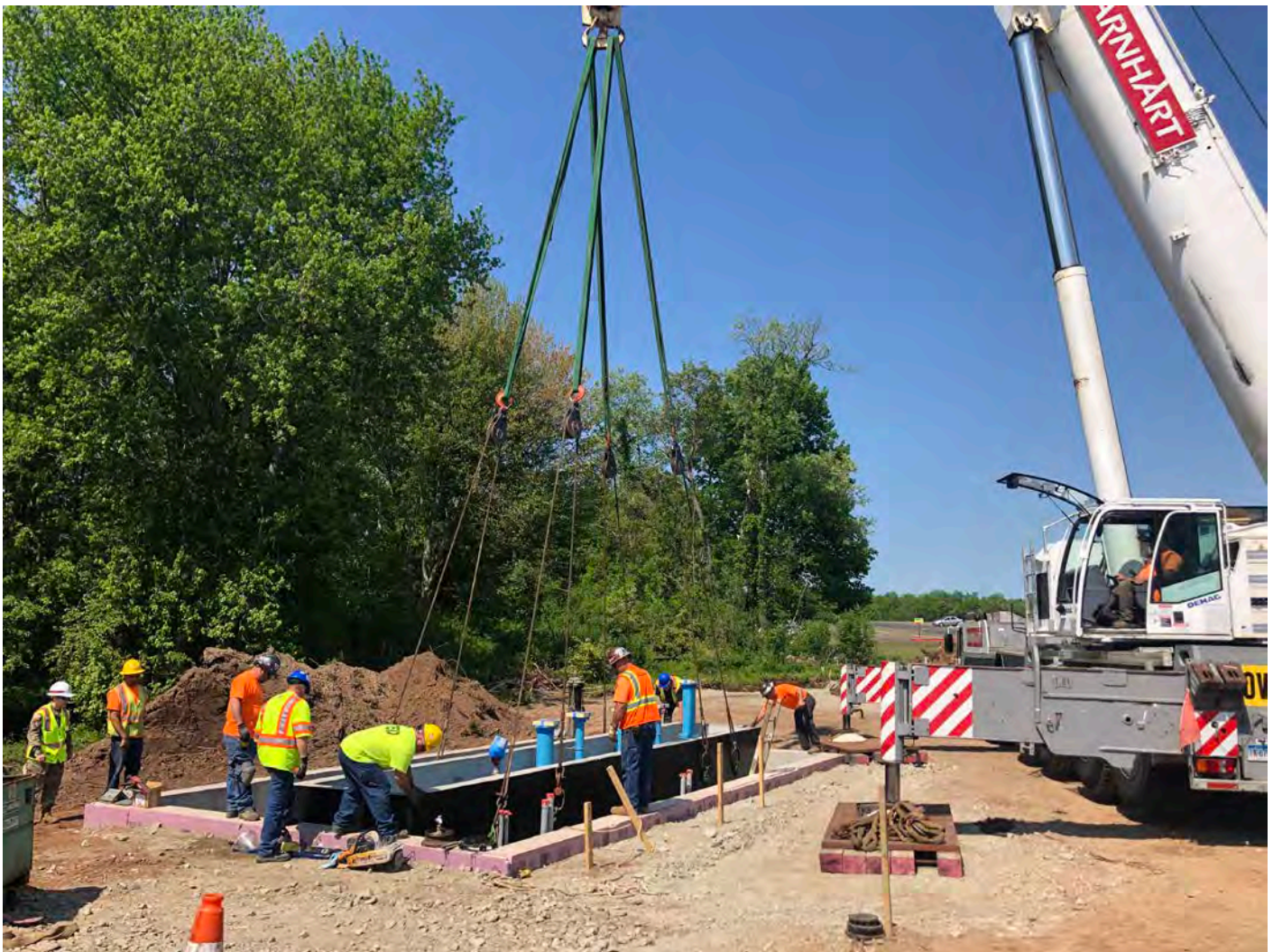
Picture 3: Barnhart lowering the trough into the booster station footprint at Station 750+63 in Middletown. View to the west/southwest.
