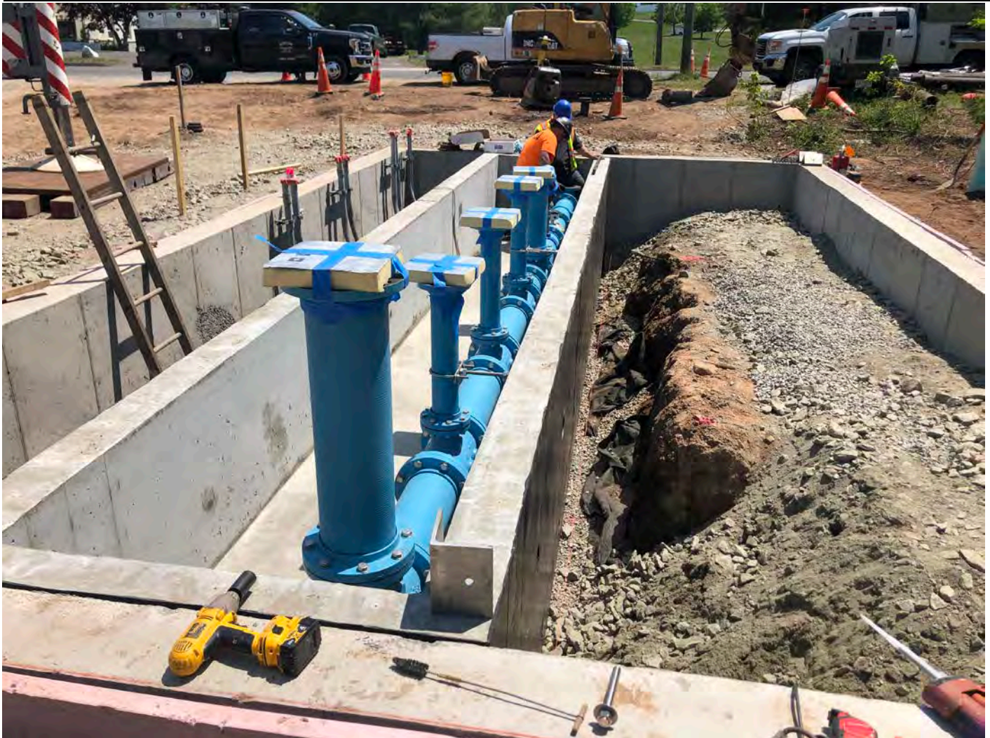
Picture 5: View of the trough after it was placed inside the booster station footprint. Station 750+63, Middletown. View to the east/northeast.
