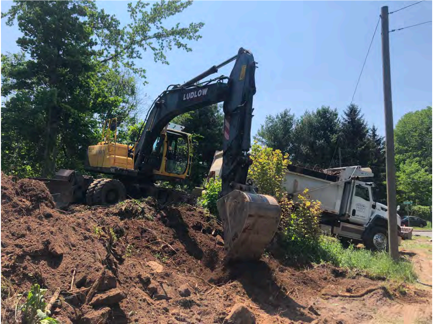
Picture 4: Ludlow clearing and grading at the water meter building work zone located at ~Station 124+80. S. Main Street, Middletown. View to the southeast.
