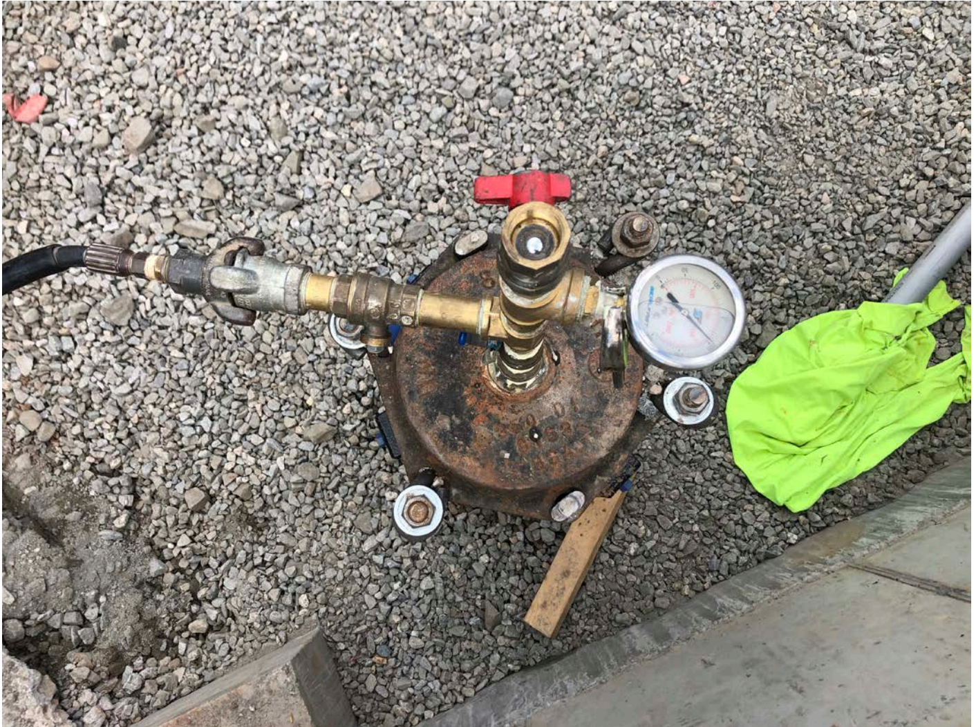
Picture 4: Pressure test setup at the booster station footprint located at Station 750+63 in Middletown, looking down at the pressure gauge. View to the northeast.
