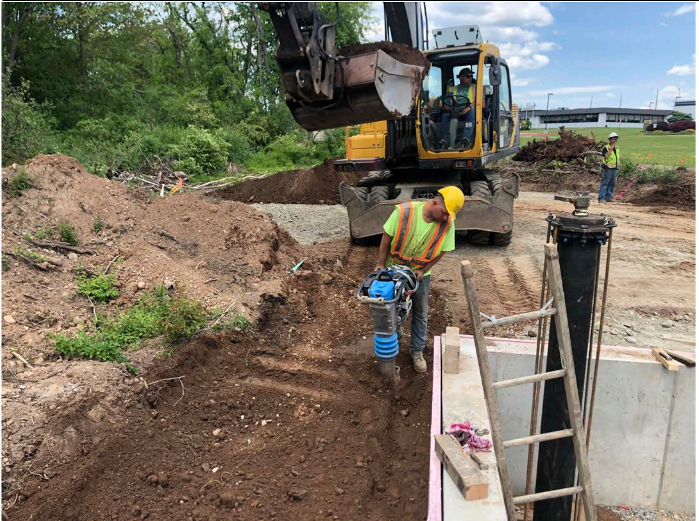
Picture 5: Ludlow compacting fill with a jumping jack along the south side of the booster station frost wall. Station 750+63, Middletown. View to the west.
