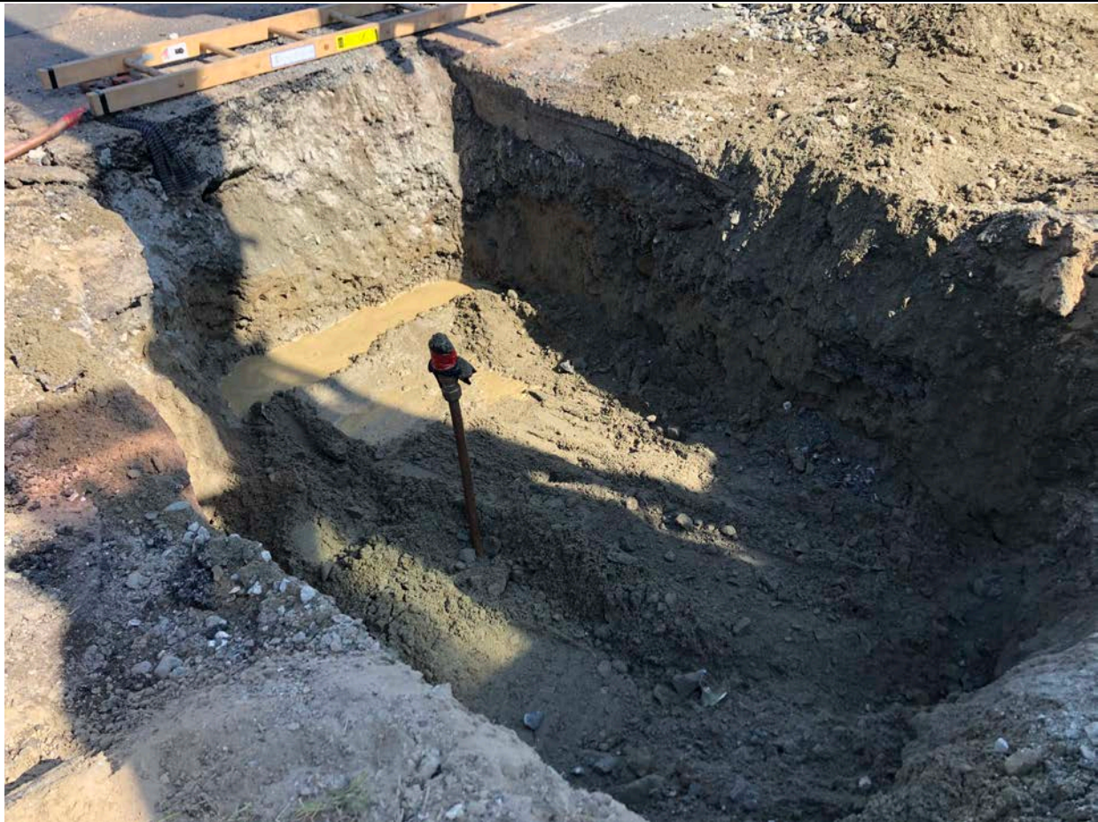
Picture 2: 1" copper blowoff that is attached to a 1" corporation stop that Ludlow installed on 8" DIP at Station 700+00 today. View to the northeast.
