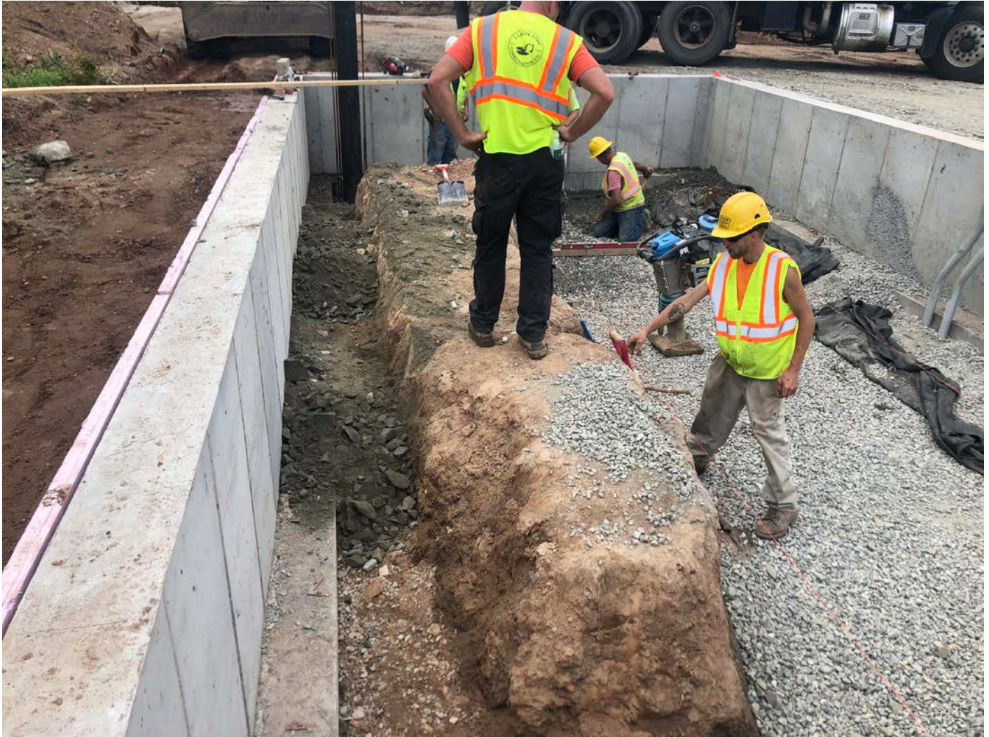
Picture 9: Ludlow in the process of placing backfill on the north side of the southern frost wall at the booster station work zone. View to the west.
