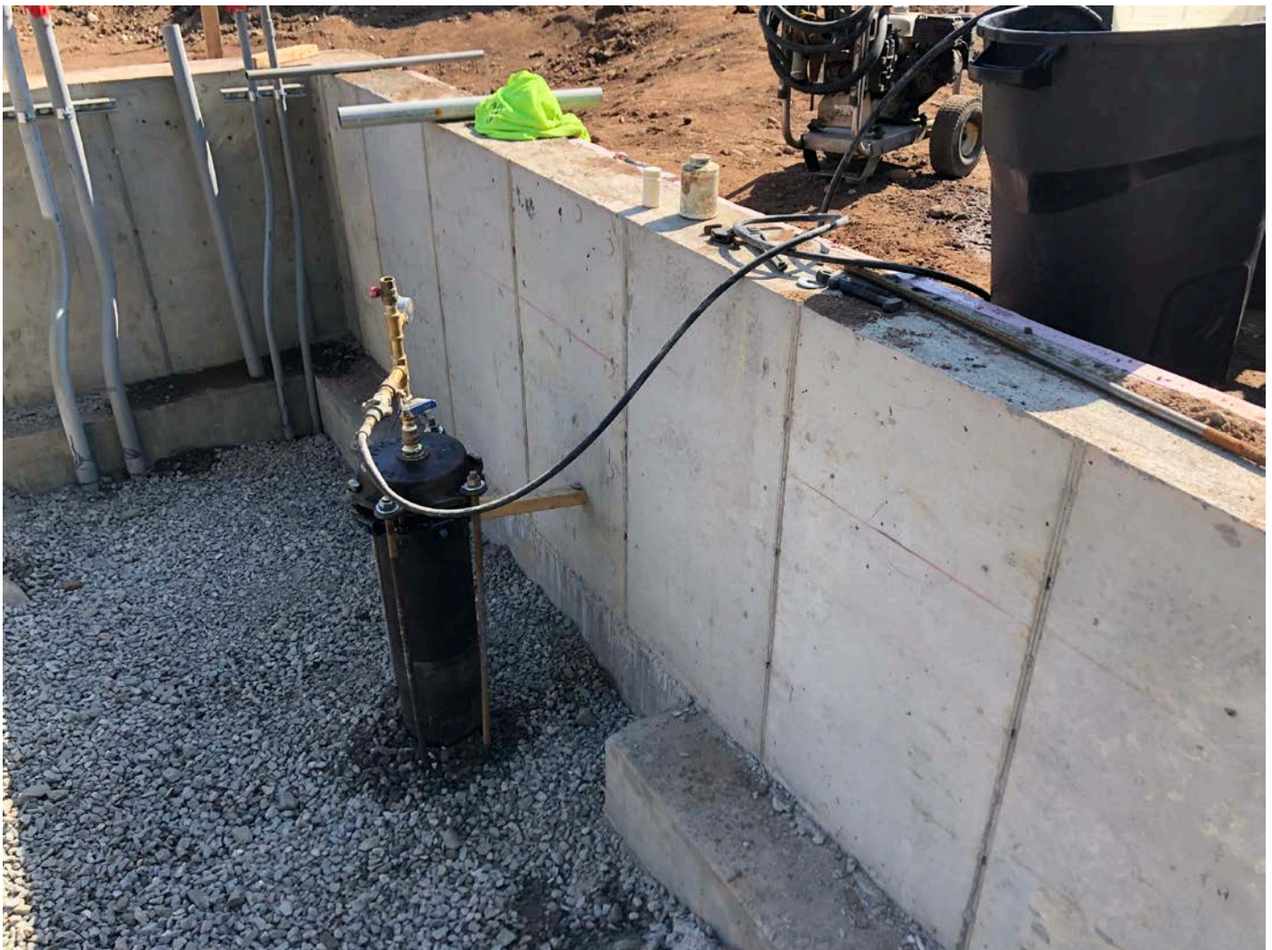
Picture 3: Pressure test setup at the booster station footprint at Station 750+63 in Middletown. View to the northeast.
