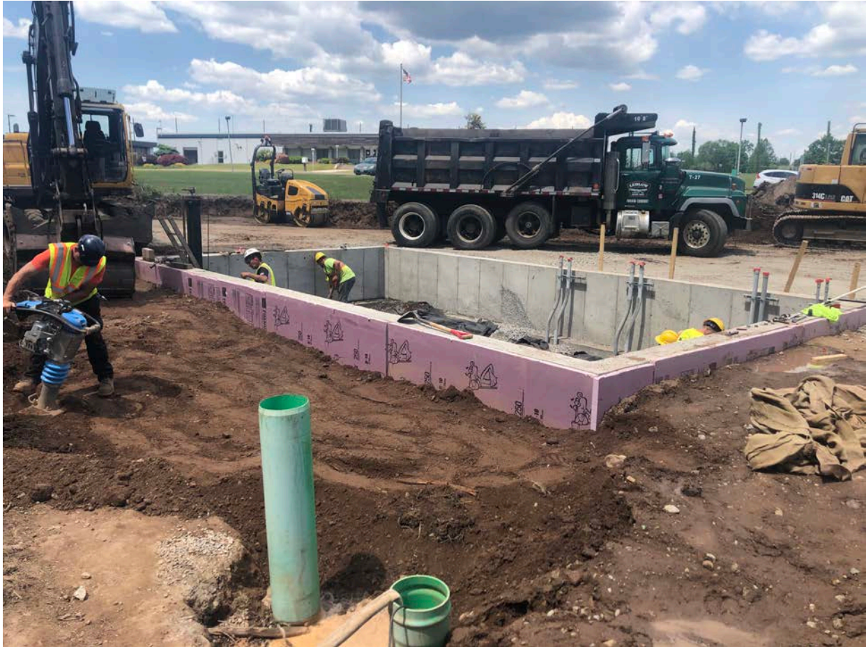
Picture 8: Overview of progress at the booster station footprint located at Station 750+63 in Middletown. View to the north.
