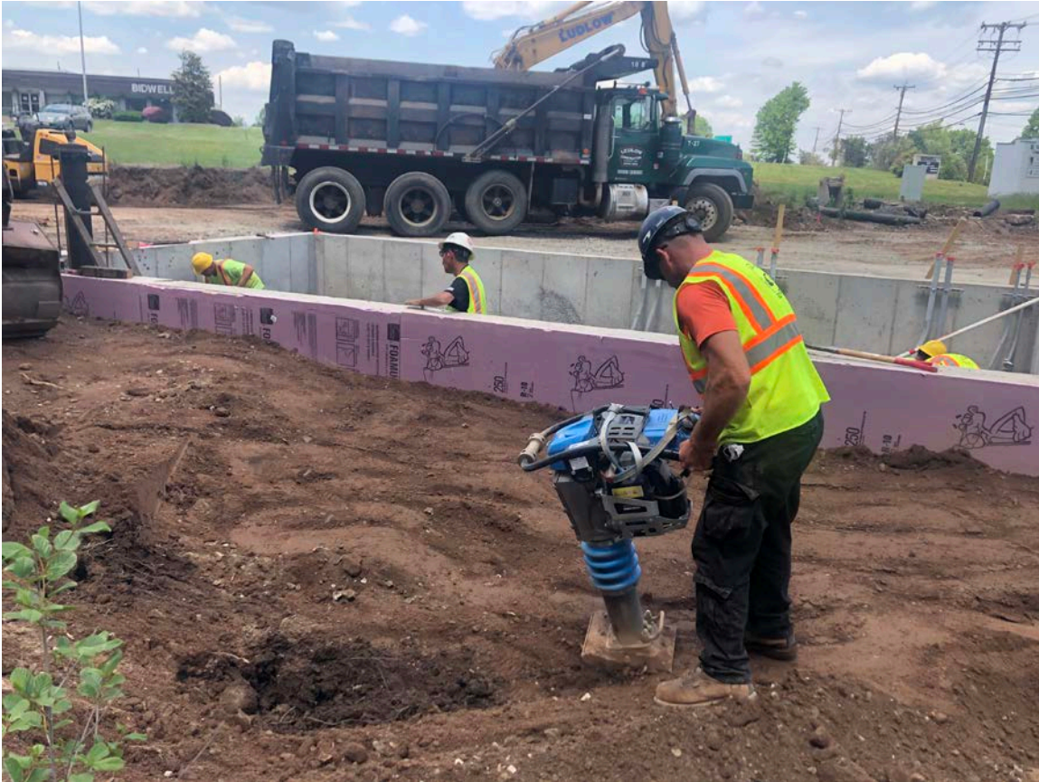
Picture 7: Ludlow compacting fill with a jumping jack south of the booster station footprint. Station 750+63, Middletown. View to the north.
