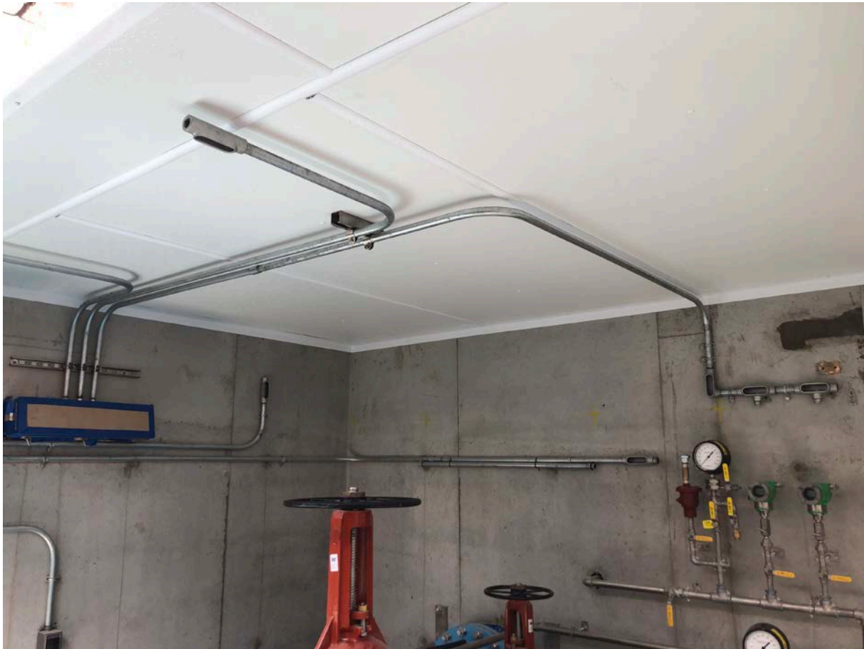
Picture 6: Rigid galvanized steel electrical conduit in the process of being installed by United Concrete at the altitude valve vault located east of the Shared Access Driveway in Middletown.
