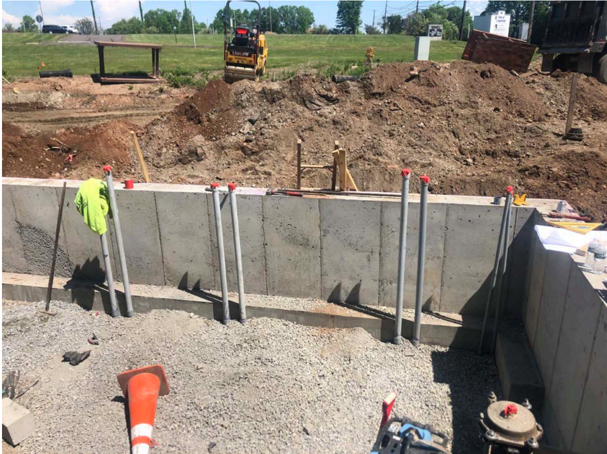
Picture 6: View of progress on PVC conduit installation on the north side of the booster station footprint. Booster station work zone, Station 750+63, S. Main St., Middletown. View to the north.
