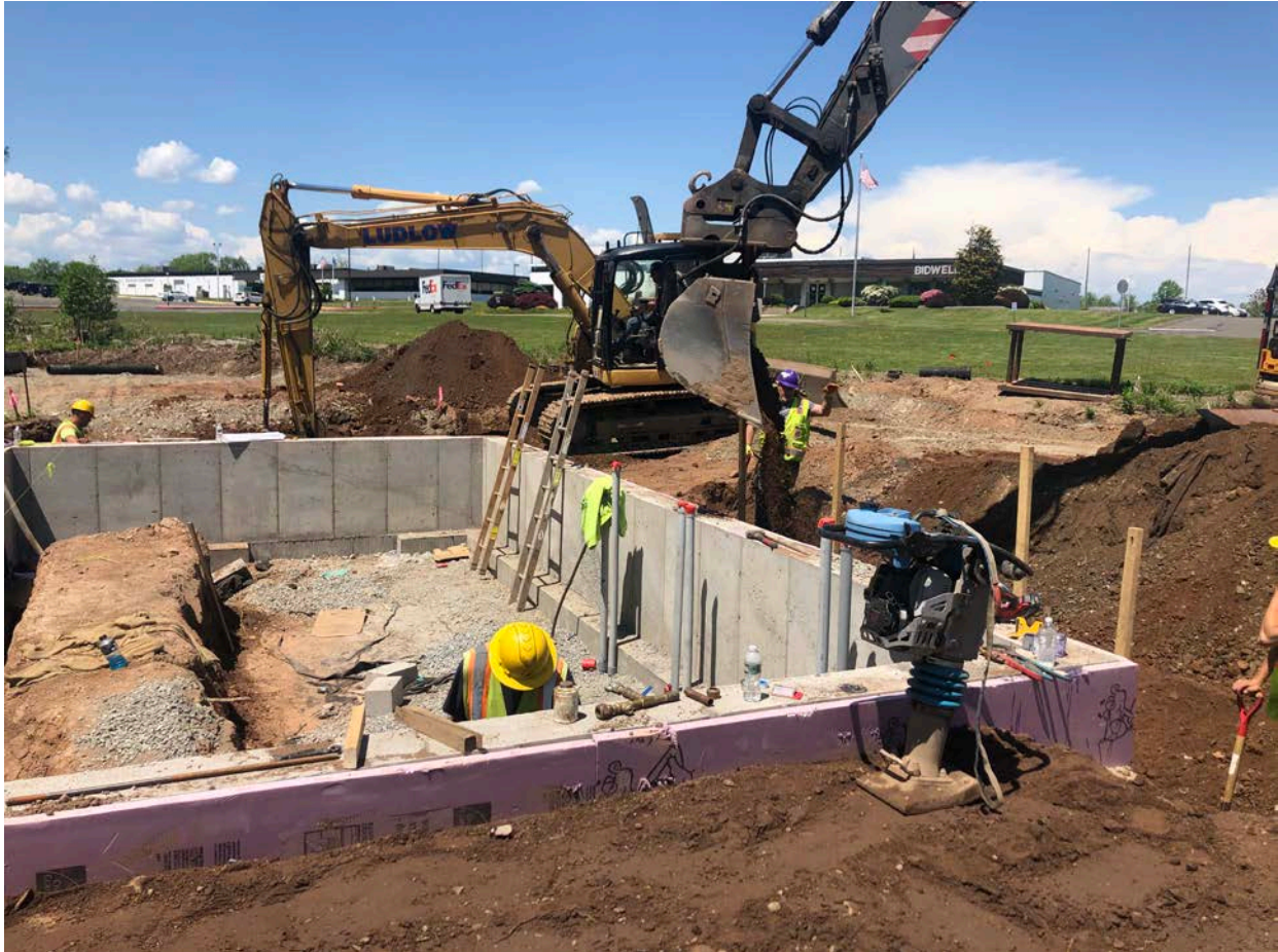
Picture 8: Ludlow in the process of backfilling on the north side of the booster station after PVC conduits were installed. Booster station work zone, Station 750+63, Middletown. View to the northwest.
