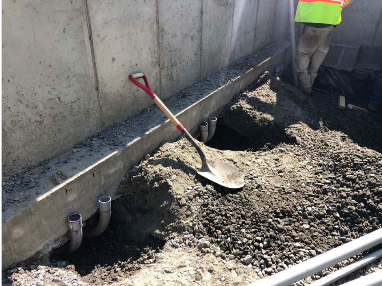
Picture 2: Same conduits as depicted in Picture 1; view of where they daylight inside of the booster station footing. View to the northeast.
