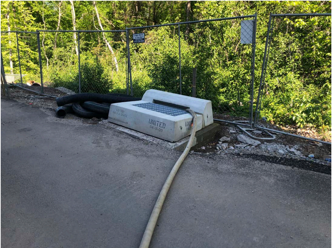
Picture 3: Catch basin that Ludlow is pumping water into from the water tank located east of the Shared Access Driveway in Middletown. View to the northwest.
