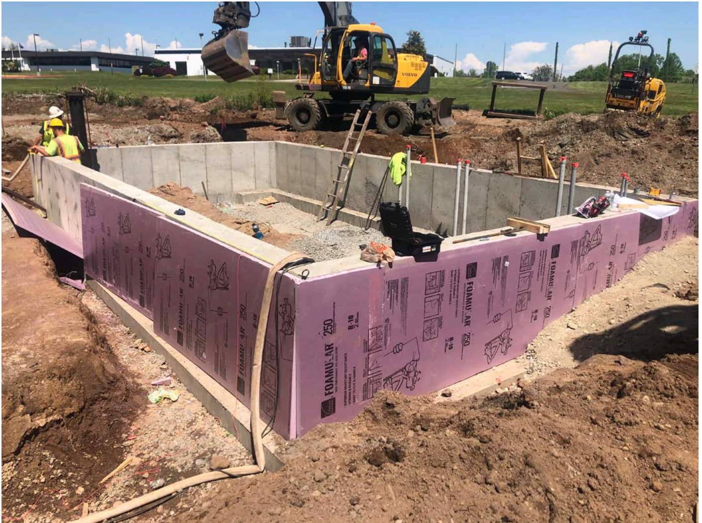
Picture 4: View of progress at the booster station footprint, looking to the northwest. A dewatering hose is visible at the southeast corner of the footprint and is directing water from inside of the frost wall into the adjoining woods to the south.
