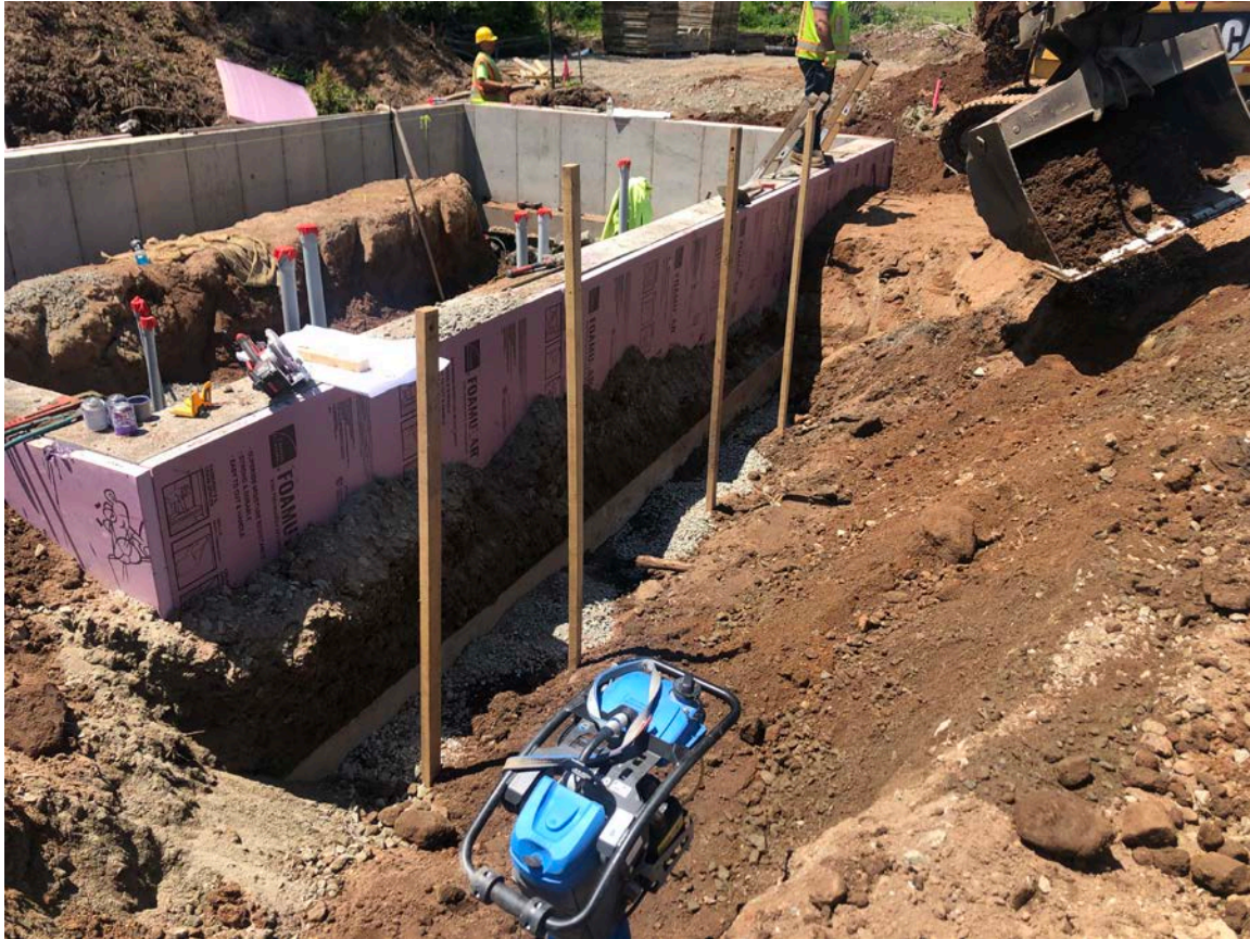
Picture 7: Ludlow in the process of backfilling on the north side of the booster station after PVC conduits were installed. Booster station work zone, Station 750+63, Middletown. View to the southwest.
