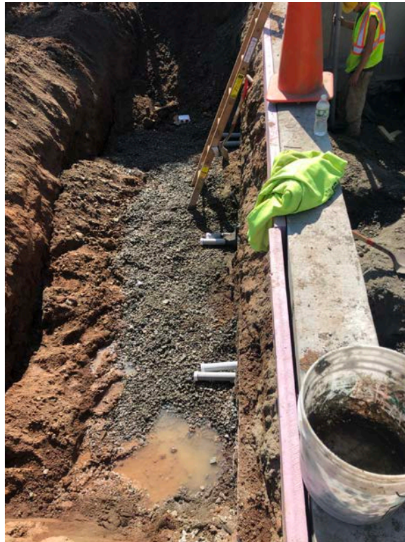
Picture 1: PVC conduits that Ludlow is installing today, protruding beneath the north side, and exterior of, the booster station footing. View to the east.
