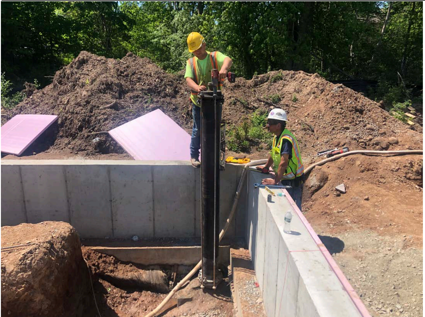
Picture 5: Ludlow reinstalling vertical section of 8" DIP at the southwest corner of the booster station footprint in Middletown. View to the west.
