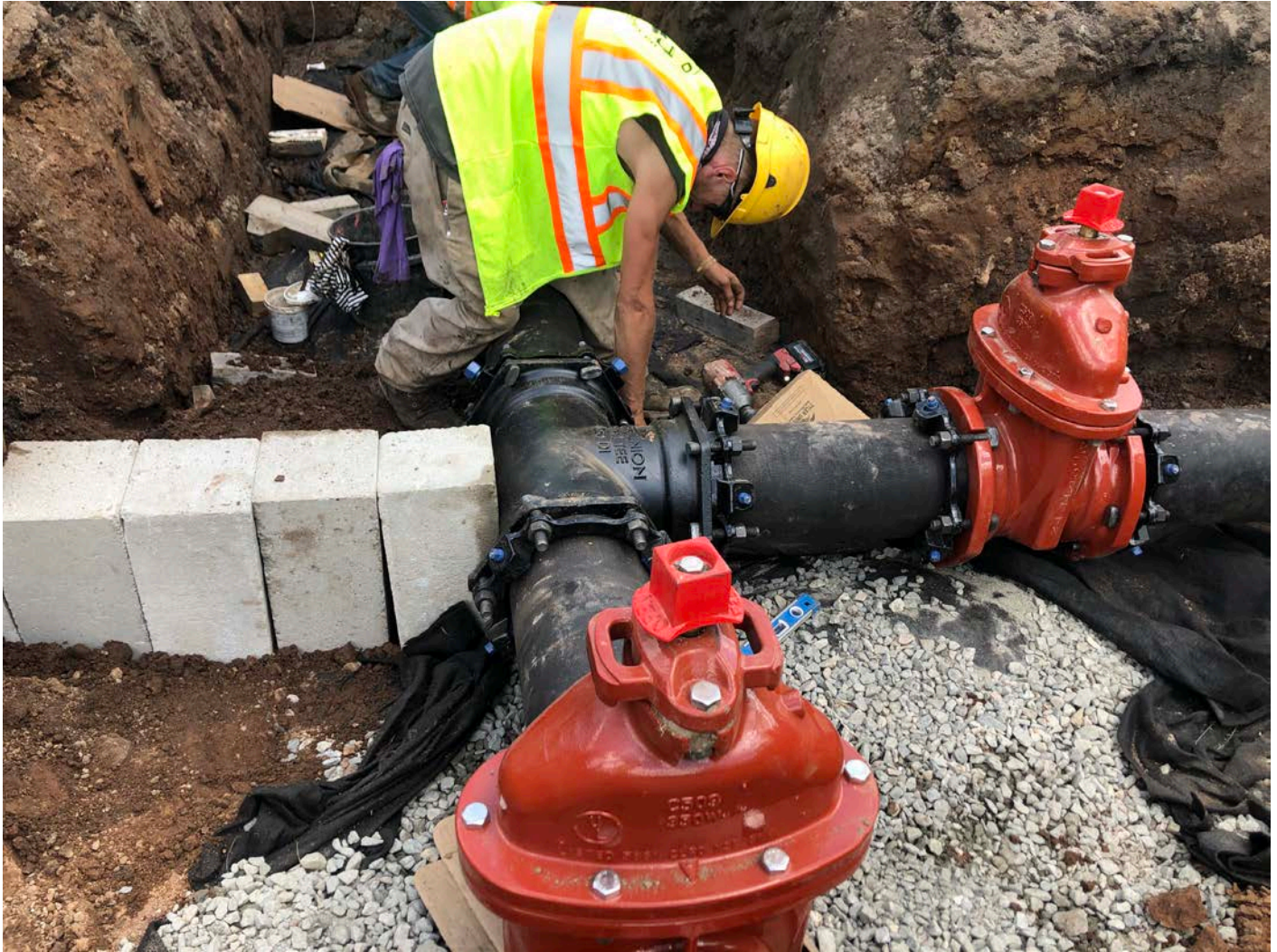
Picture 10: Thrust block placed on the north side of the 8"x8"x8" M.J. C.L.D.I. TEE at Station 700+73. View to the east.
