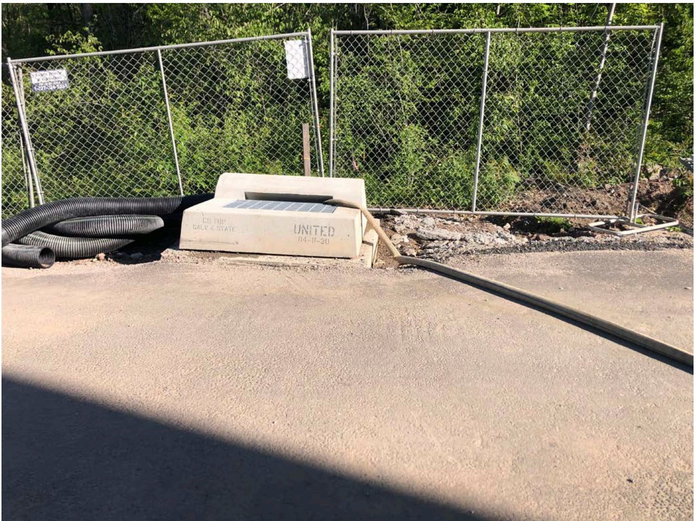
Picture 3: Catch basin that Ludlow is pumping water into from the water tank located east of the Shared Access Driveway in Middletown. View to the north.
