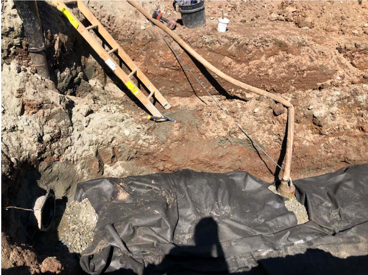
Picture 6: Ludlow pumping water from the trench located due east of the booster station footprint located at Station 750+63 in Middletown. View to the west.
