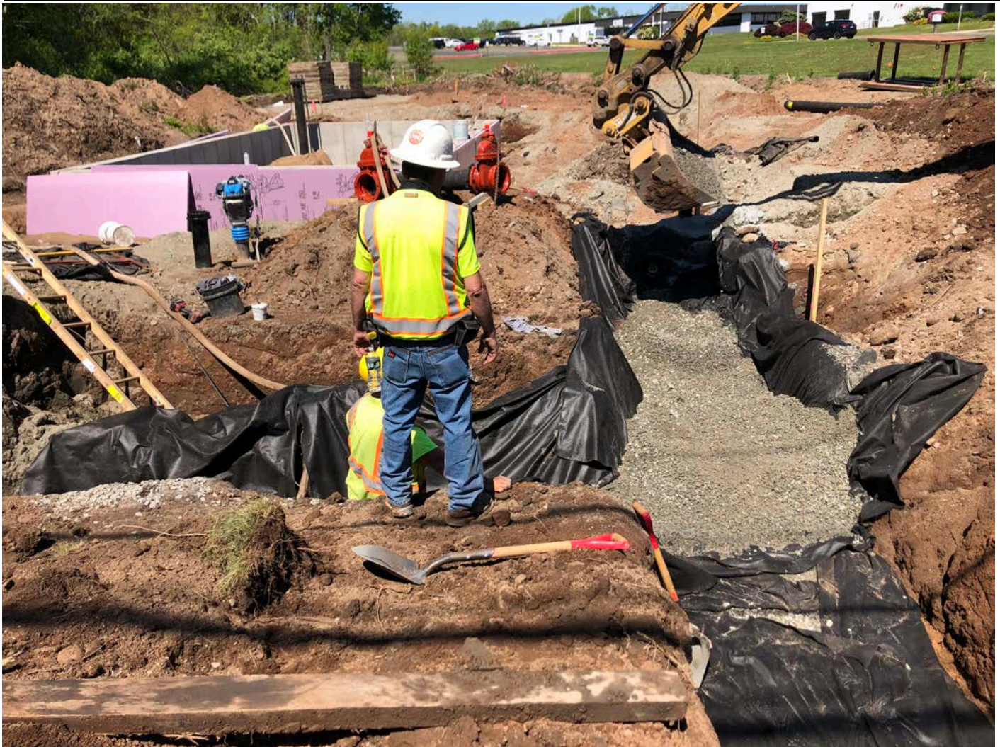
Picture 5: Ludlow placing ¾" gravel on top of geofabric in the trench located just north of the booster station footprint in Middletown. View to the west.
