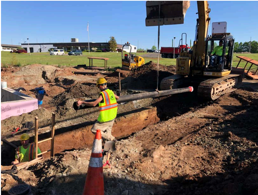
Picture 1: Ludlow preparing to install 6" DIP that is part of a hydrant assembly at Station 700+93, Station 750+10. View to the northwest.
