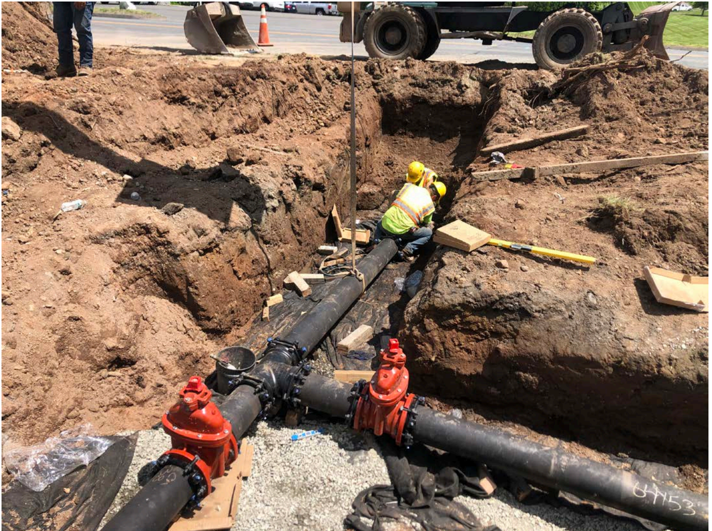
Picture 9: Ludlow installing 8" DIP from north of the booster station to previously-installed 8" DIP located at Station 750+00. View to the east.
