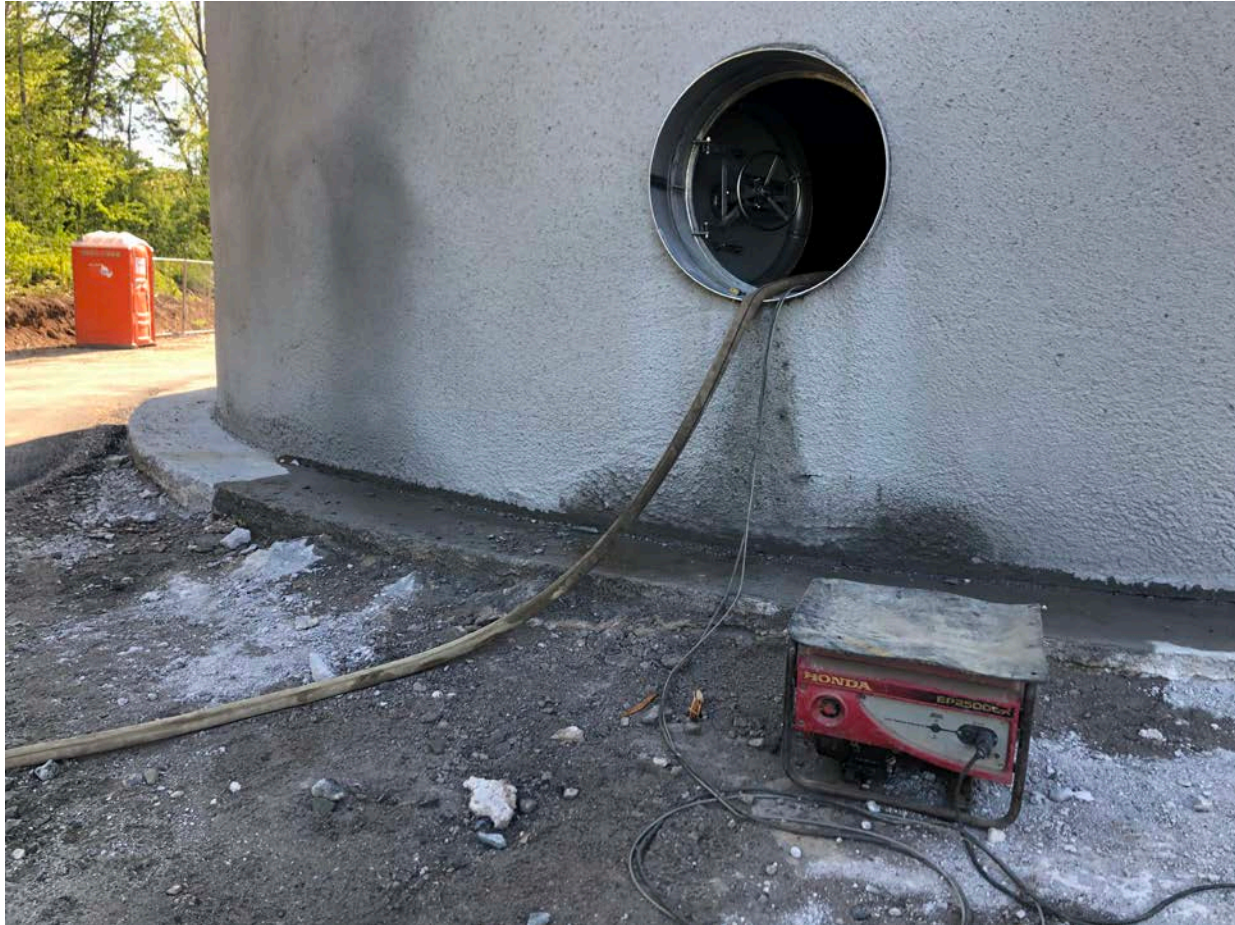
Picture 2: Ludlow pumping water out of the water tank located east of the Shared Access Driveway in Middletown. View to the northeast.
