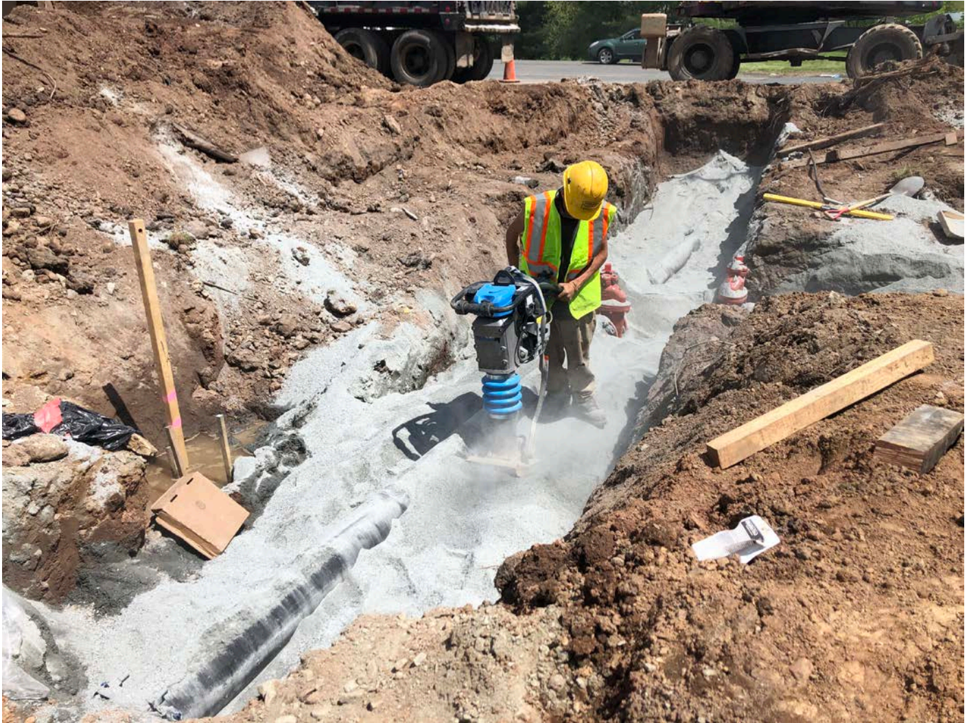
Picture 11: Ludlow compacting sand with a jumping jack next to the 8" DIP they installed from north of the booster station to previously-installed 8" DIP located at Station 750+00. View to the east.
