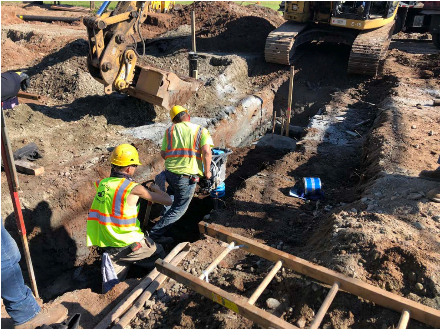
Picture 4: Ludlow compacting sand with a jumping jack at the 6" DIP they just installed east of the booster station footprint. View to the northwest.
