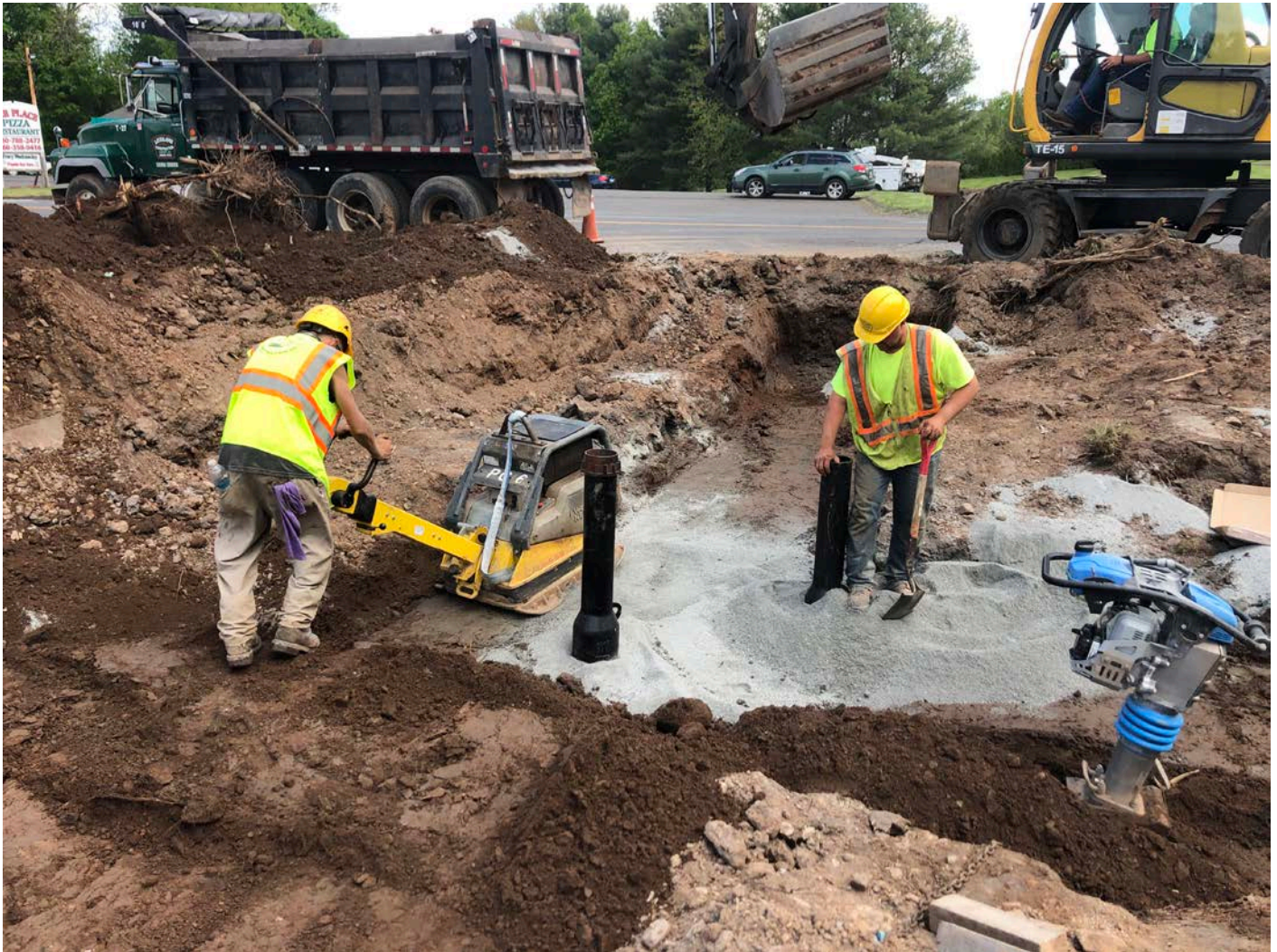
Picture 12: Ludlow compacting sand with a plate compactor next to the 8" DIP they installed from north of the booster station to previously-installed 8" DIP located at Station 750+00. View to the east/northeast.
