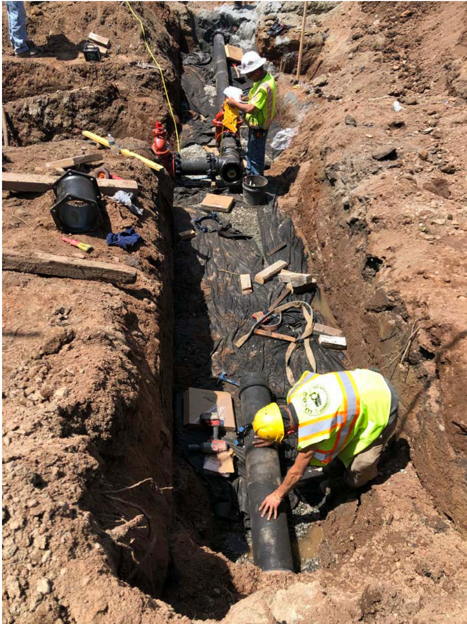
Picture 8: Ludlow installing 8" DIP from north of the booster station to previously-installed 8" DIP located at Station 750+00. View to the west.
