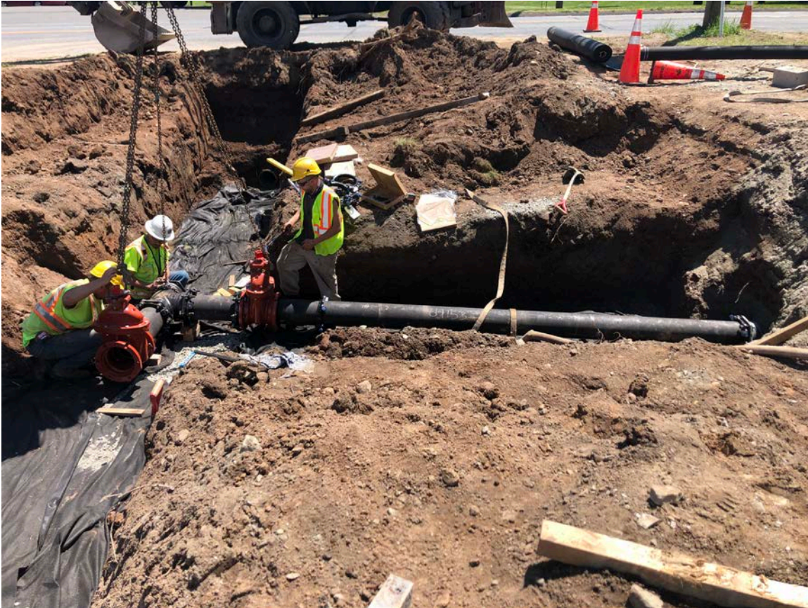
Picture 7: Ludlow in the process of installing 8" DIP on the east side of the booster station located at Station 750+63. This pipe is part of the bypass line from Station 750+25 to Station 700+73. View to the east.
