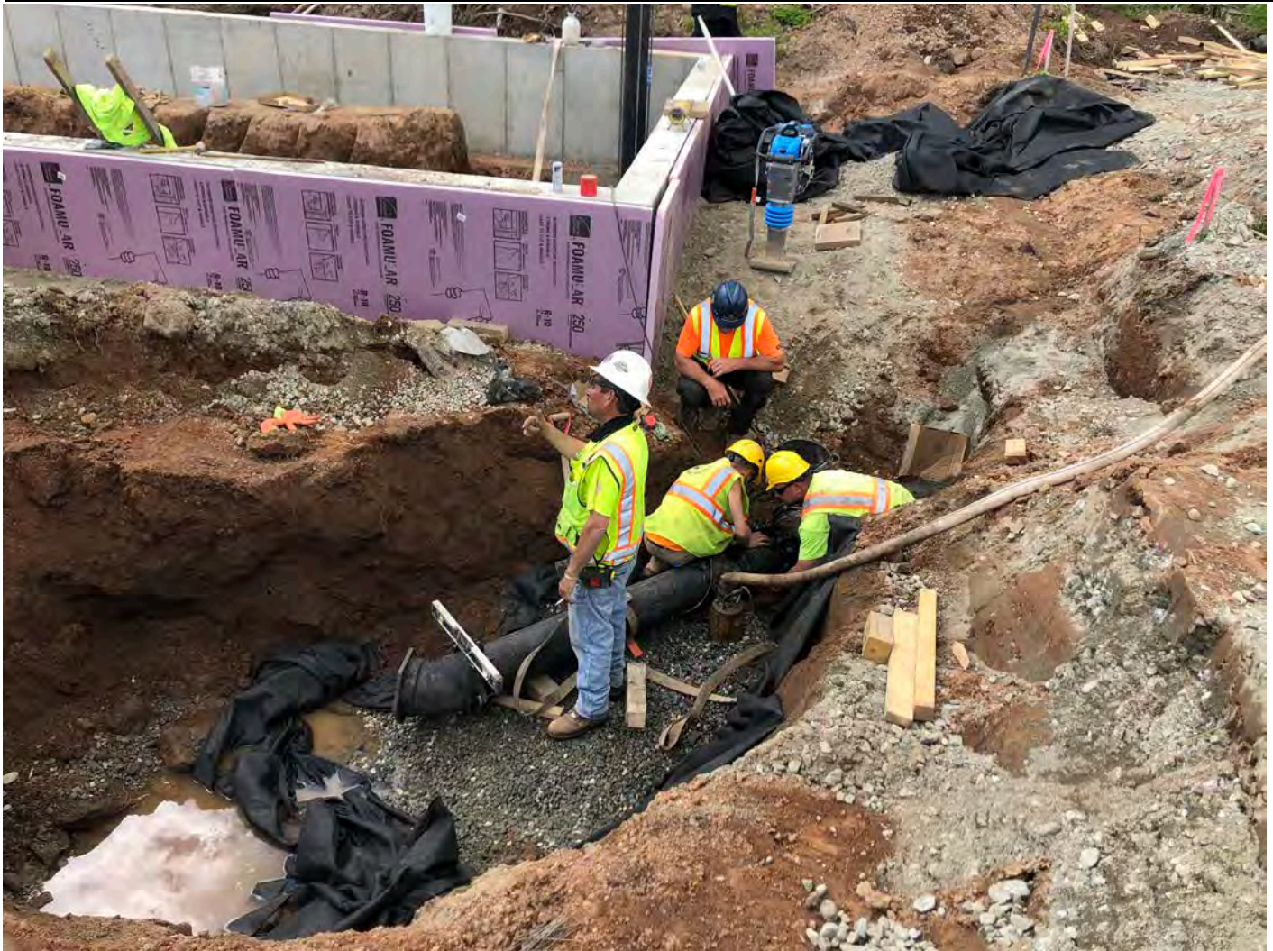
Picture 5: Ludlow installing 8" DIP with a 45° bend at the northwest corner of the booster station footprint. View to the southeast; Station 750+59 in Middletown.
