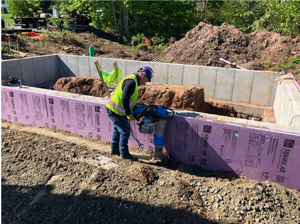
Picture 2: Ludlow compacting fill along the north side of the booster station with a jumping jack. Booster station work zone located at Station 750+63 South Main St. Middletown. View to the south.
