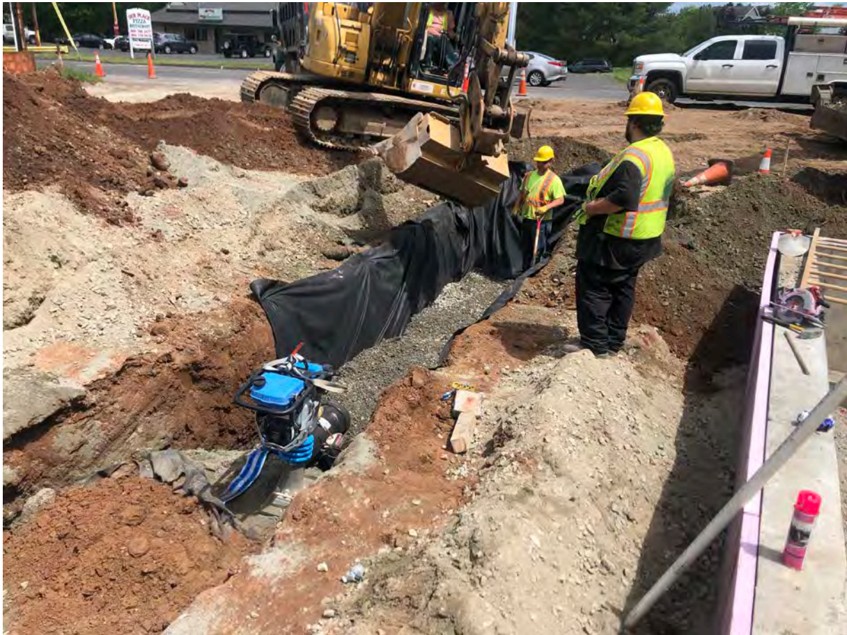
Picture 6: Ludlow placing geofabric and ¾" gravel as they prepare the bedding for the 8" DIP suction they are installing on the north side of the booster station located at Station 750+63. View to the east.
