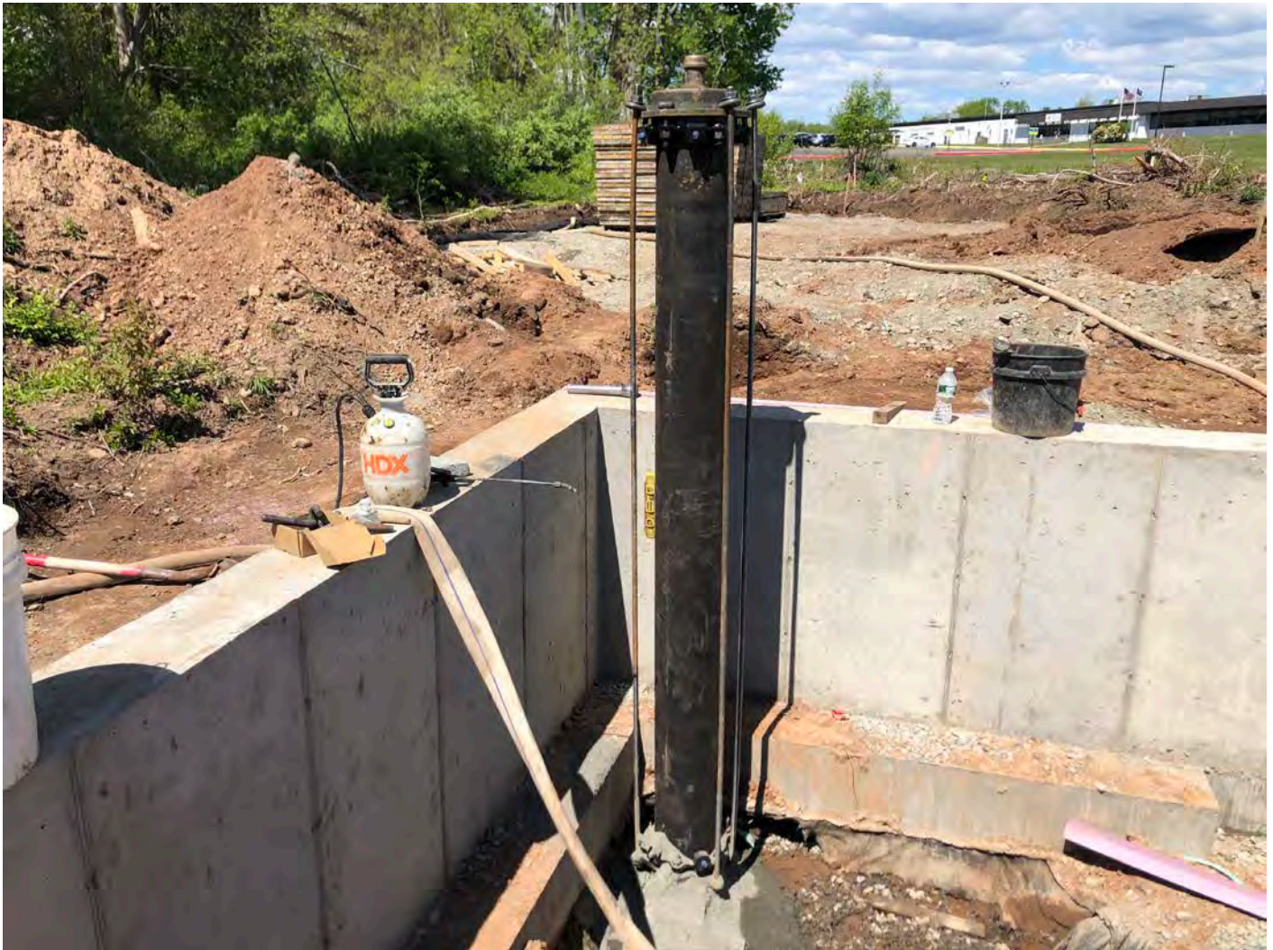
Picture 3: Section of 8" DIP that Ludlow installed on top of an 8" DIP 90° bend that is restrained with 1" threaded rods per United Concrete drawing A-3. Booster station work zone, Station 750+63, Middletown. View to the west.
