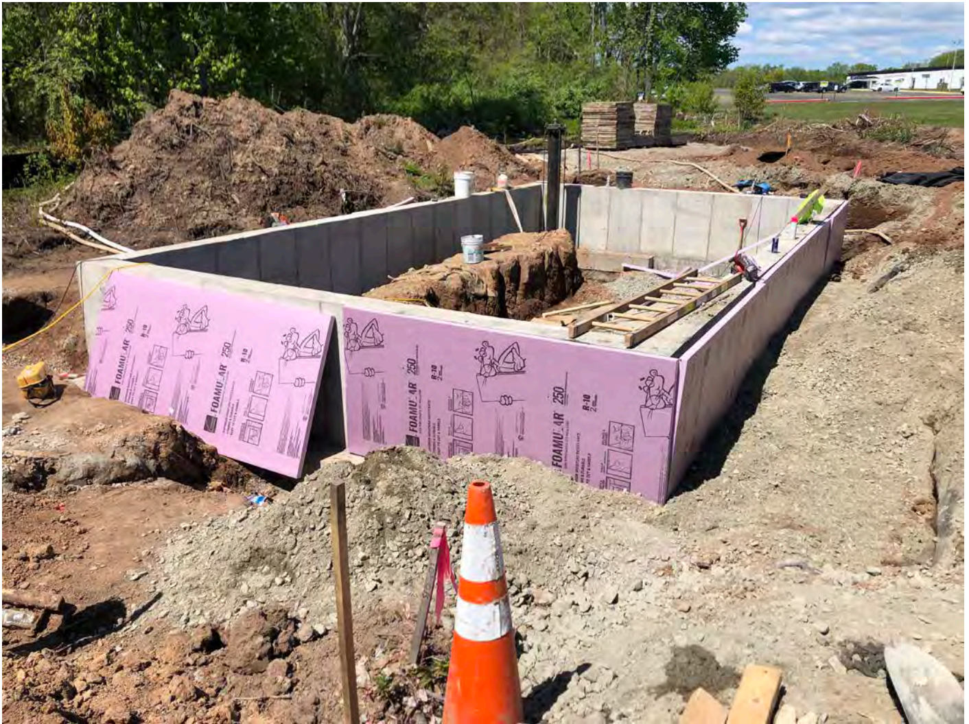
Picture 4: Booster station frost wall with 2" foam insulation panels being placed on the exterior. View to the west; booster station work zone located at Station 750+59 in Middletown.
