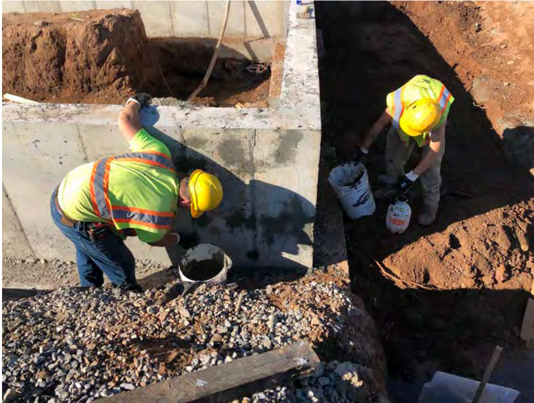
Picture 1: Ludlow filling minor imperfections on the exterior of the frost wall with grout.
