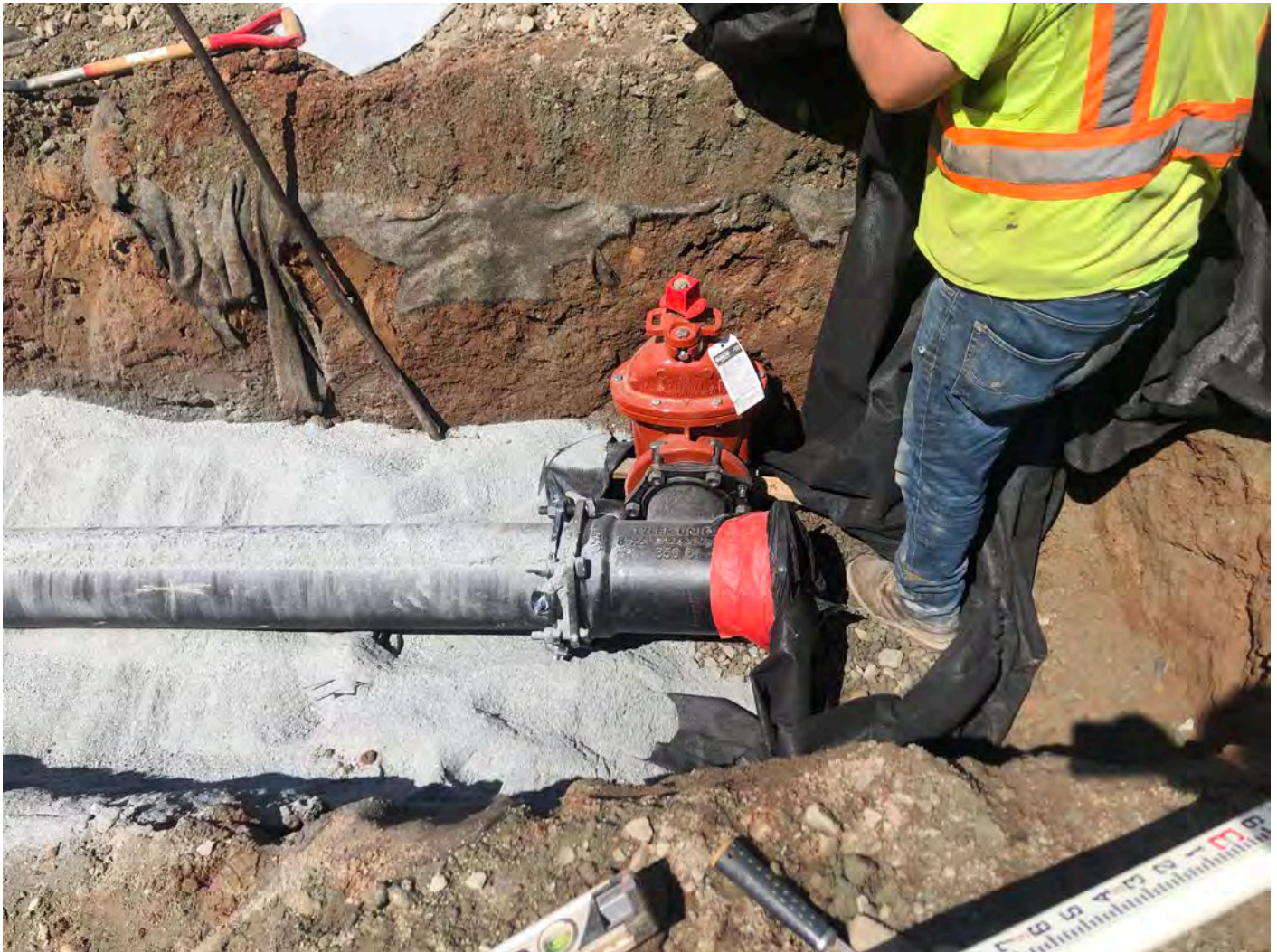
Picture 8: An 8"x8"x6" M.J. C.D.L.I. TEE with a 6" M.J gate valve that Ludlow installed on the 8" DIP line they are running along the north side of the booster station footprint. View to the north.
