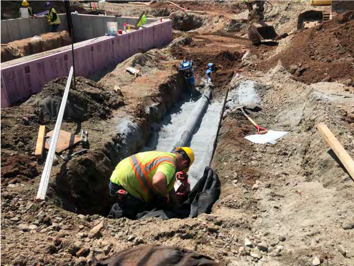
Picture 7: Ludlow in the process of installing 8" DIP on the north side of the booster station located at Station 750+63. View to the west.
