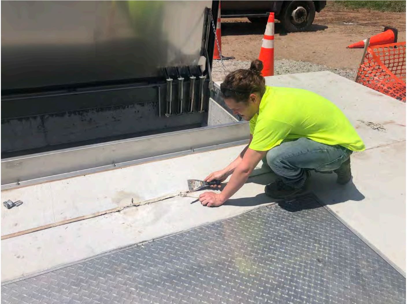
Picture 9: United Concrete removing damaged caulking from the seam between the two sections of the pressure reducing valve vault located at ~Station 161+40 Main Street Durham. View to the west.
