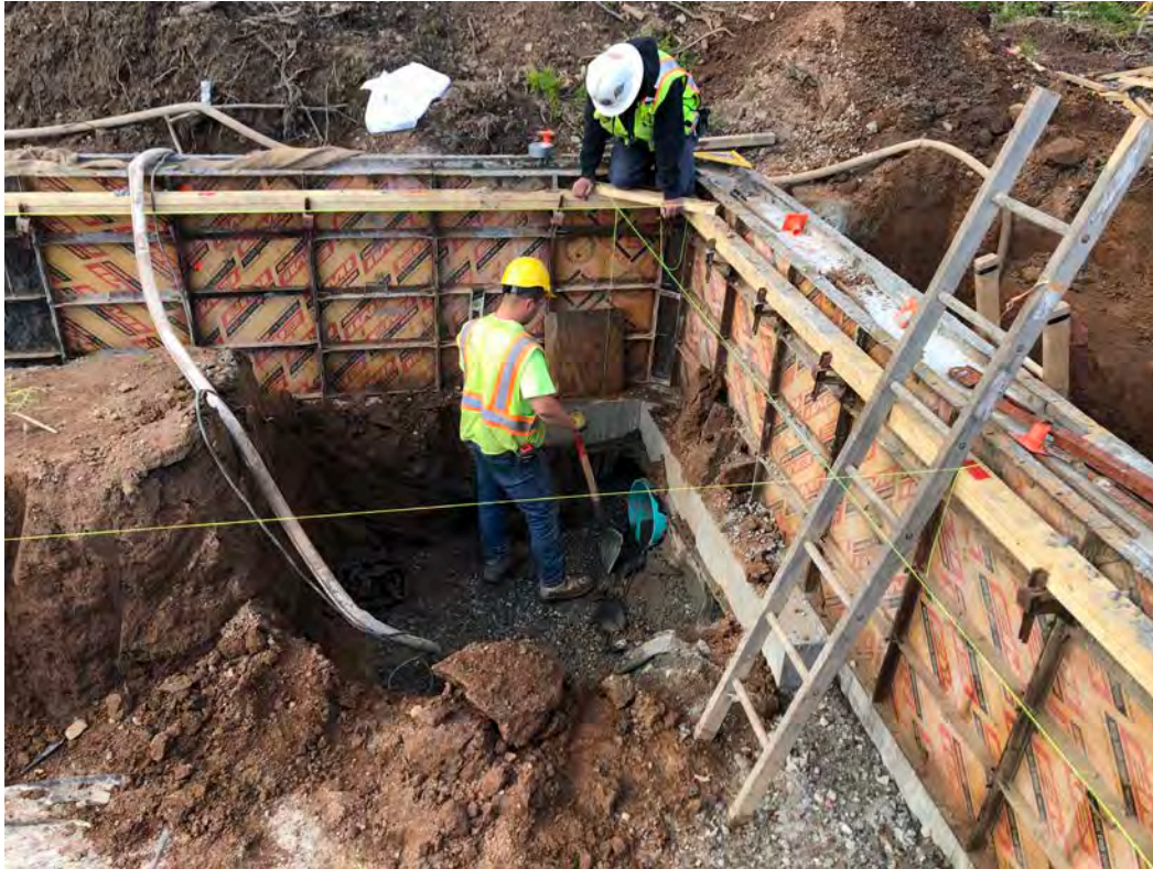
Picture 1: View of the southwest interior corner of the booster station footprint that was excavated to daylight the previously-installed PVC conduit for the installation of 8" DI booster station suction pipe. View to the southwest.
