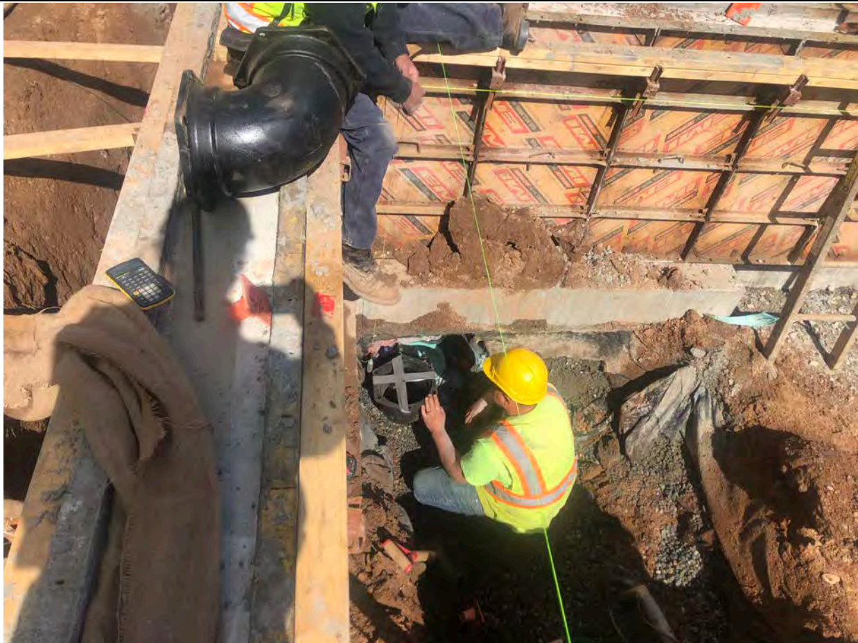
Picture 2: View of the southwest interior corner of the booster station footprint, where Ludlow has installed 8" DIP through the 16" PVC conduit that runs beneath the western footing of the booster station. Also visible is the 90° bend that Ludlow attached to the east side of the 8" DIP (the bend is facing upwards in the photograph). Booster station work zone located at Station 750+63 South Main St. Middletown. View to the west.
