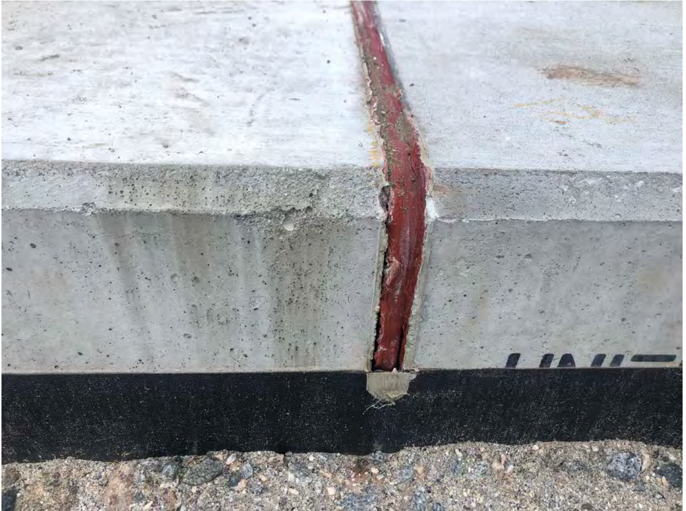
Picture 10: View of the seam located between the two sections of the pressure reducing vault located at ~Station 161+40 with some of the caulking removed.
