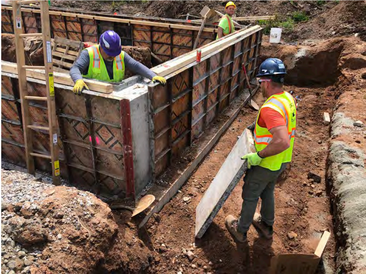
Picture 6: Ludlow beginning to remove concrete forms from the northwest corner of the booster station frost wall. View to the southeast.
