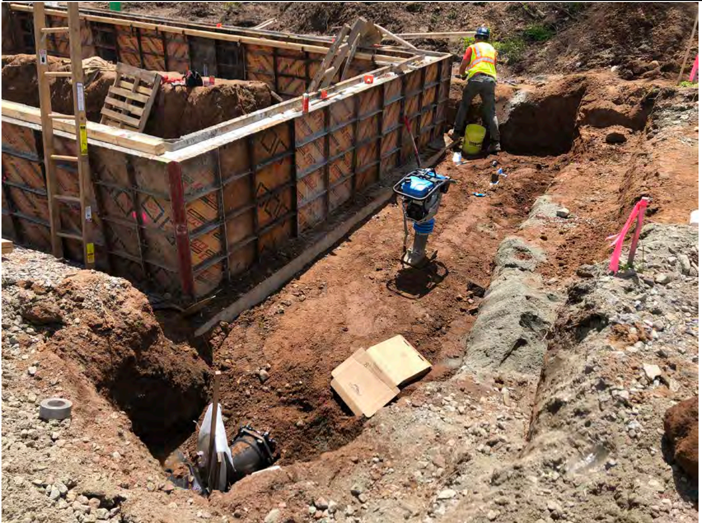
Picture 5: Ludlow used a jumping jack to compact fill that was placed over the 8" DIP that they just installed to the west of the booster station footprint. View to the southeast; booster station work zone located at Station 750+59 in Middletown.
