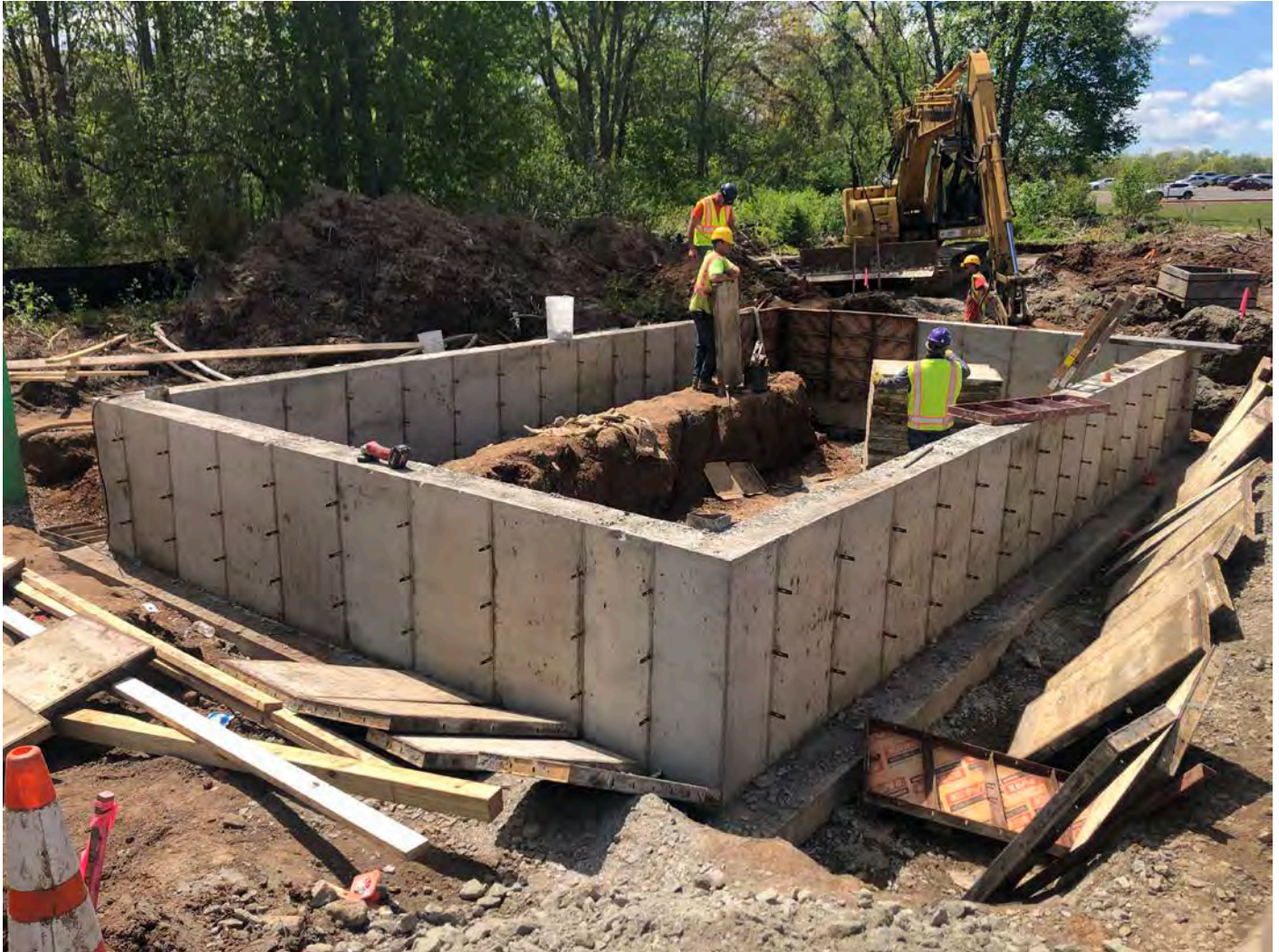
Picture 7: View of booster station frost wall with most of the concrete forms removed. View to the southwest.
