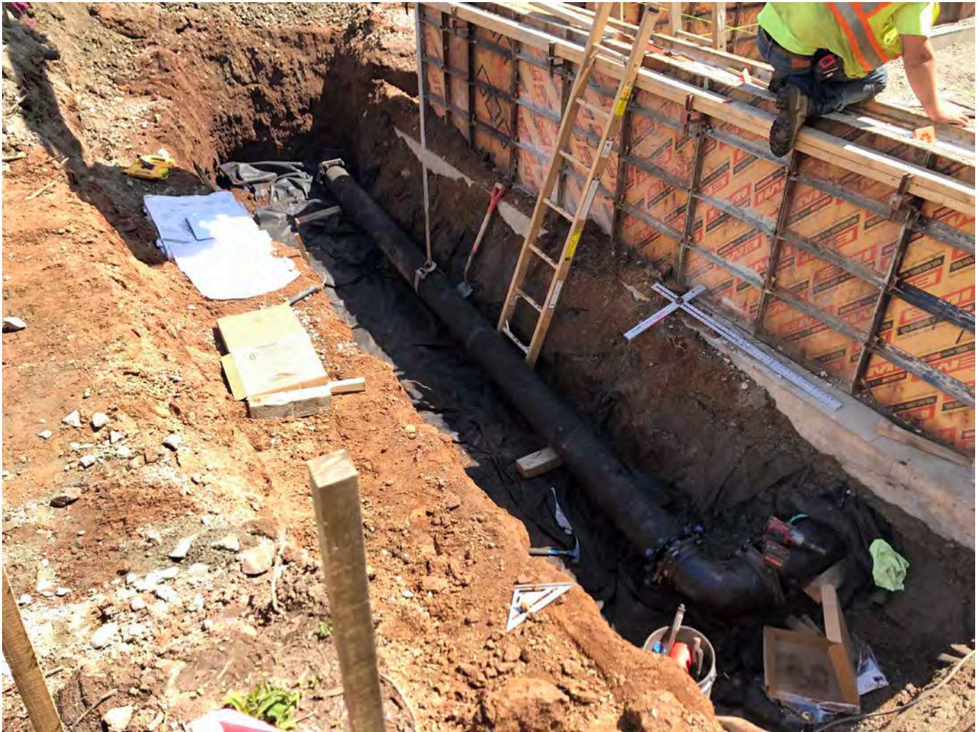
Picture 4: Ludlow in the process of installing a section of 8" DIP to the 8" DIP 90° bend that they just installed at the southwest exterior corner of the booster station footprint. View to the northeast; booster station work zone located at Station 750+59 South Main Street in Middletown.
