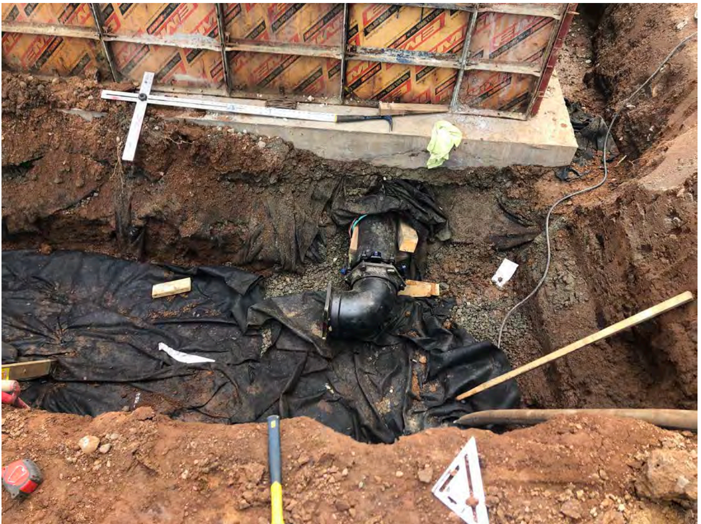
Picture 3: View of 8" DIP installation beneath the western footing of the booster station, with an 8" DIP 90° bend attached to it. View to the east; booster station work zone located at Station 750+63 South Main Street in Middletown.
