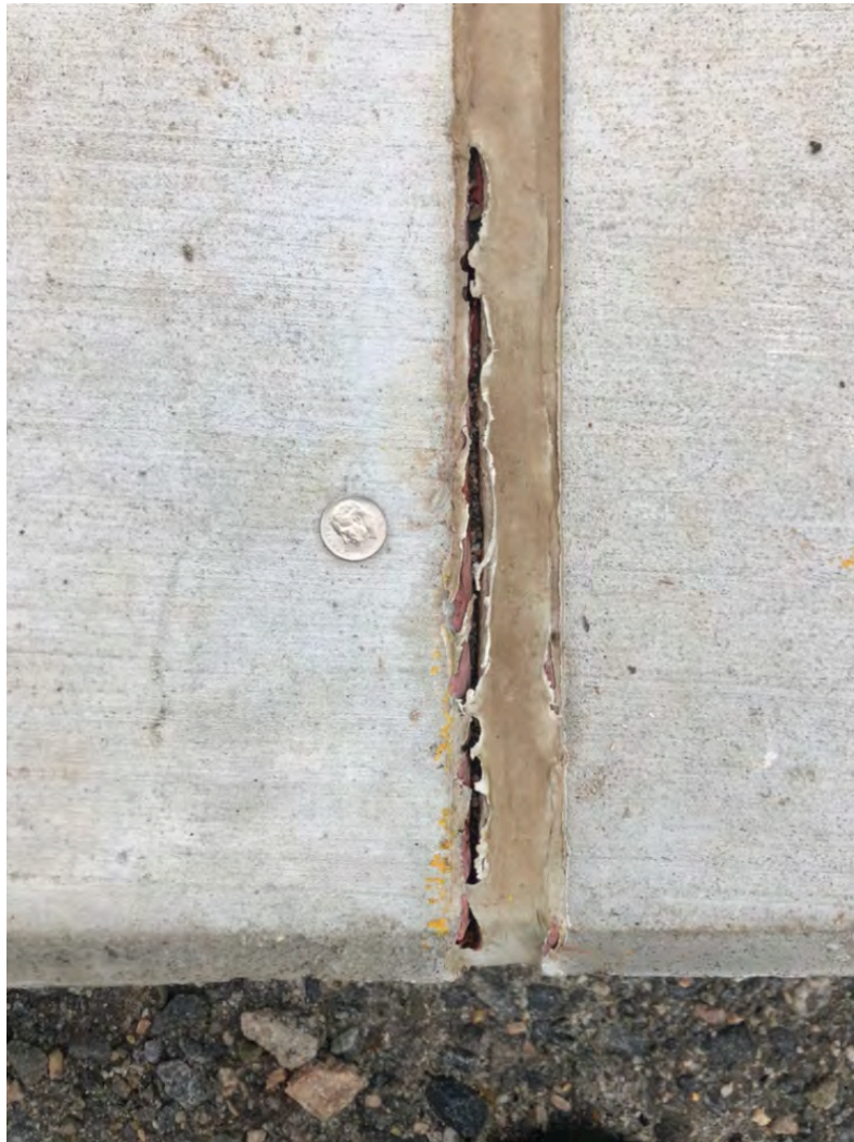
Picture 8: Caulking on the seam between the two sections of the pressure reducing valve vault located at ~Station 161+40 Main Street Durham.
