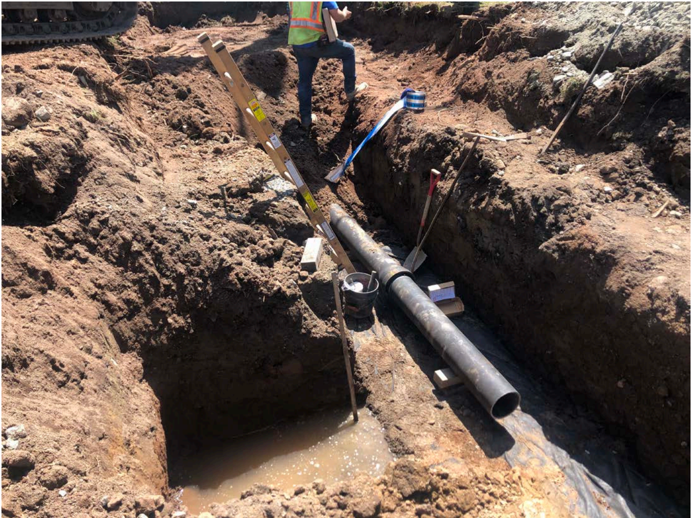
Picture 3: View of 8" DIP installation located east of the booster station footprint, depicting progress. View to the east; booster station work zone located at Station 750+63 in Middletown.
