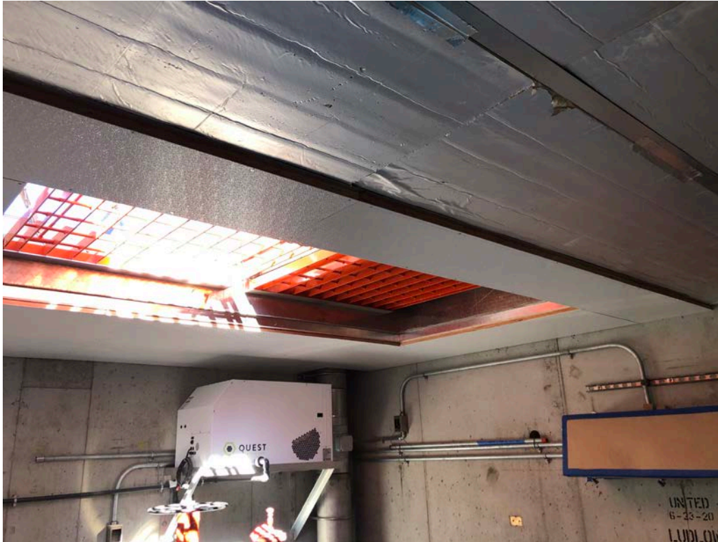
Picture 1: Fire retardant panels that have been installed over 2" insulation at the interior of the altitude valve vault located east of the Shared Access Driveway in Middletown. View to the northeast.
