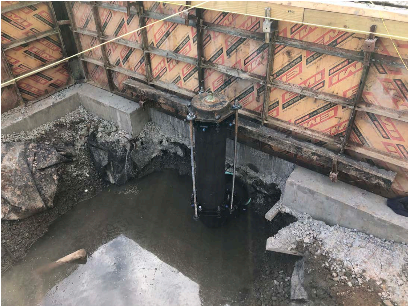
Picture 10: Section of 8" DIP booster station discharge that Ludlow installed on top of an 8" DIP 90° that is restrained with 1" threaded rods per United Concrete drawing A-3. Booster station work zone in Middletown. View to the east.
