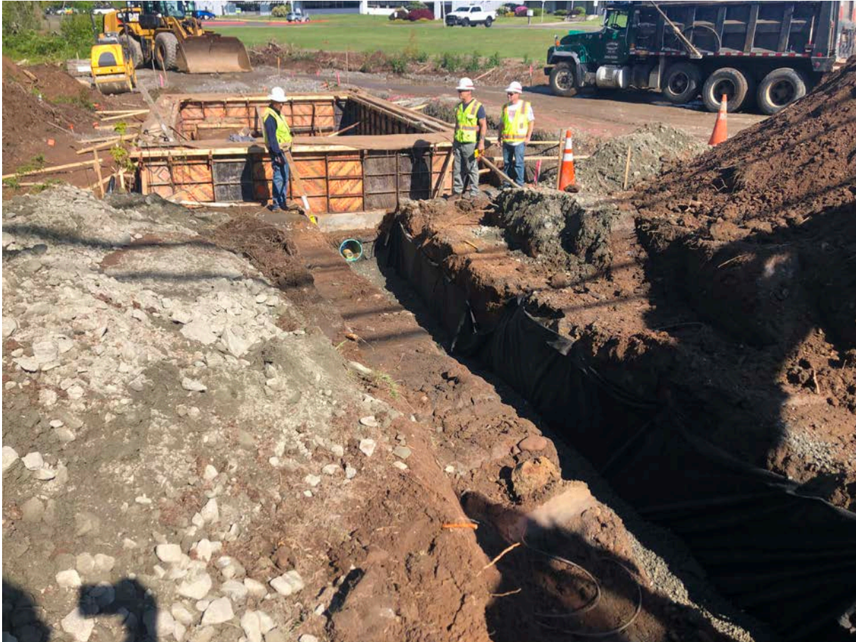
Picture 2: Trench that Ludlow excavated as they prepare to install 8" DIP booster station discharge between the previously-installed 8" DIP on South Main Street in Middletown at Station 750+59 to the interior of the booster station footprint. Station 750+63 in Middletown. View to the east.
