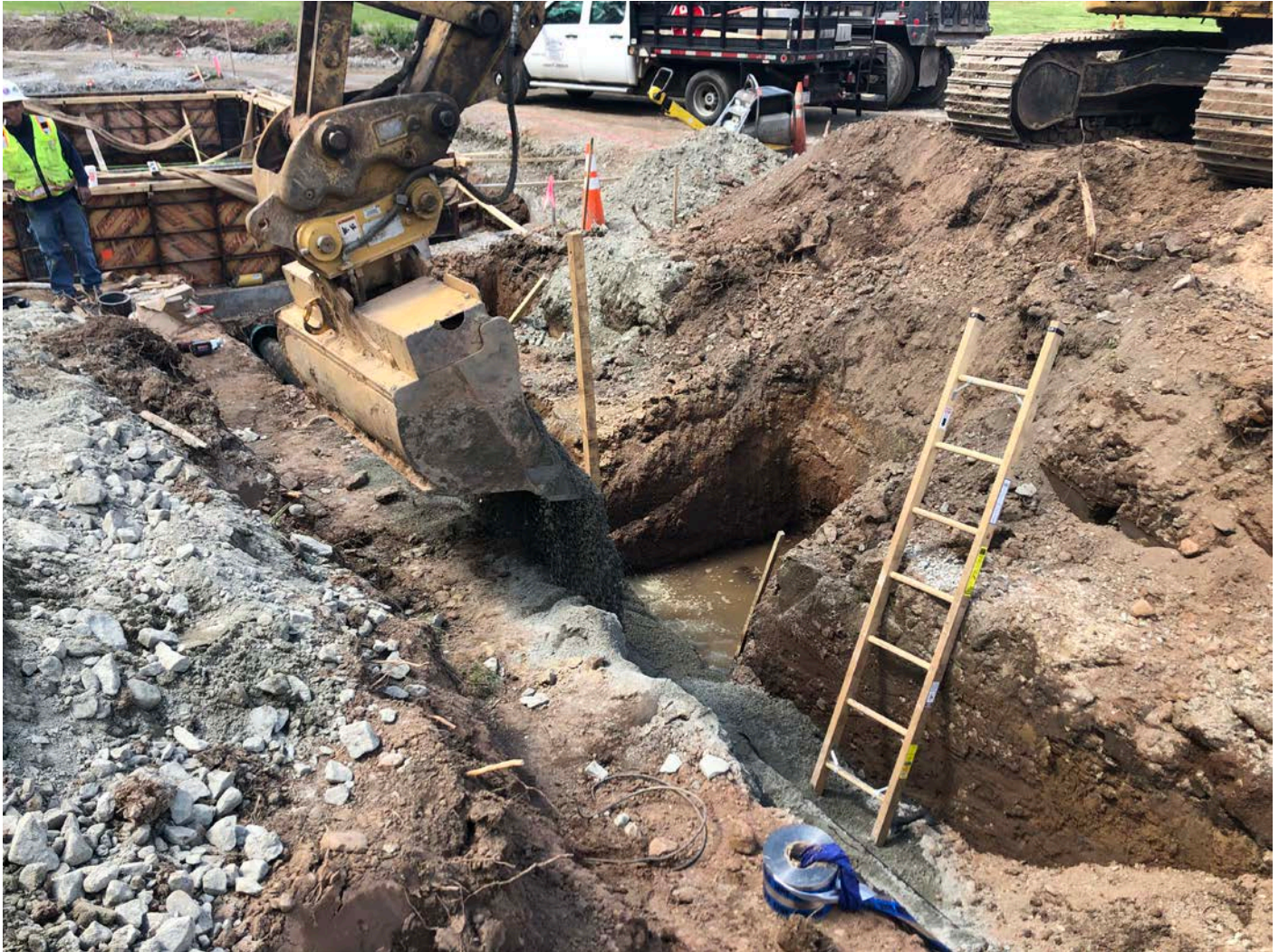
Picture 9: Ludlow placing sand on top of 8" DIP that they installed today at the booster station work zone in Middletown. View to the west.
