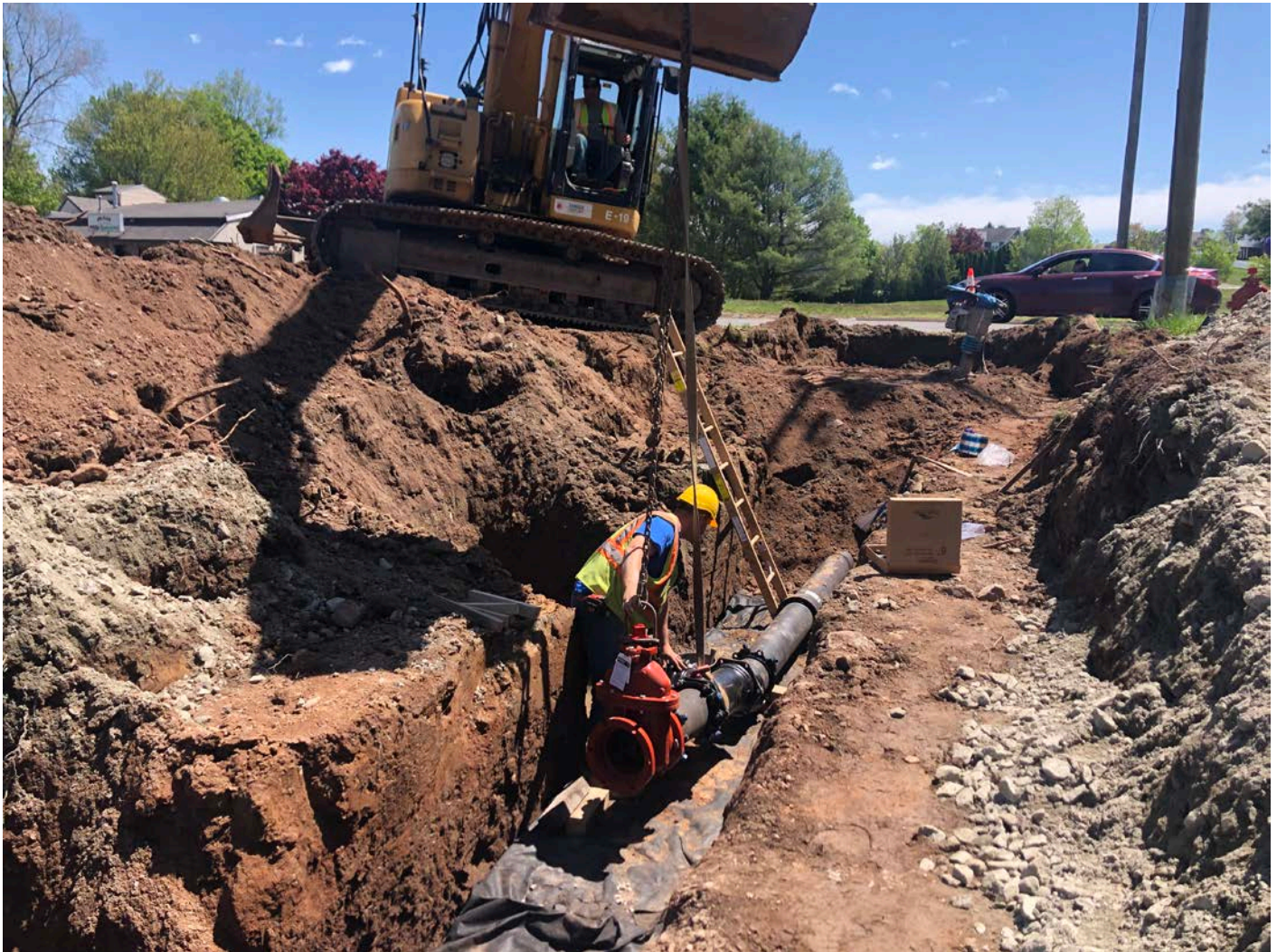
Picture 4: Ludlow in the process of installing an 8"x8"x6" M.J. C.L.D.I. TEE and a 6" M.J. gate valve between the booster station footprint and previously-installed 8" DIP located at Station 750+59 in Middletown. View to the east.
