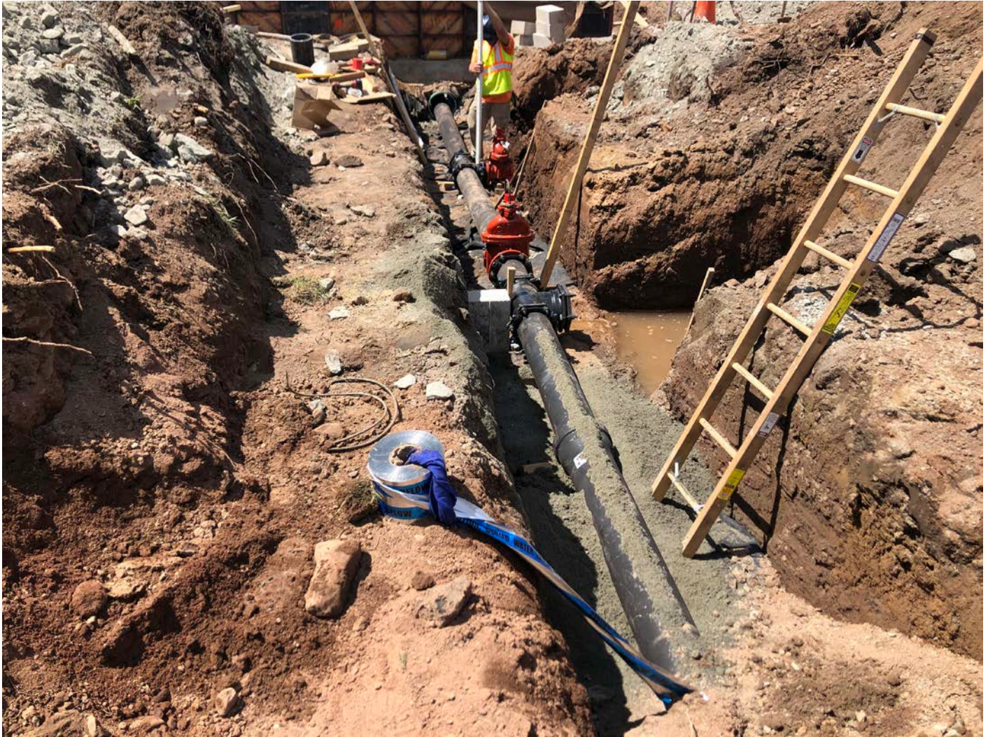
Picture 7: View of 8" DIP that Ludlow installed today between the booster station footprint and previously-installed 8" DIP at Station 750+59 in Middletown, including an 8"x8"x8" M.J. C.L.D.I. TEE and an 8" M.J. gate valve and a fire hydrant assembly (8"x8"x6" M.J. C.L.D.I. hydrant TEE and a 6" M.J. gate valve). View to the west.
