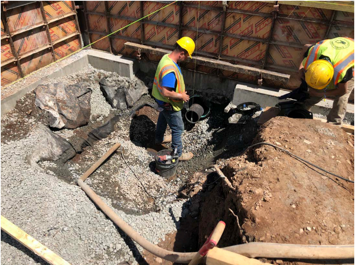
Picture 8: Ludlow preparing to install an 8" DIP 90° bend on the 8" DIP booster station discharge that now protrudes into the booster station footprint on the east side. View to the east/northeast.
