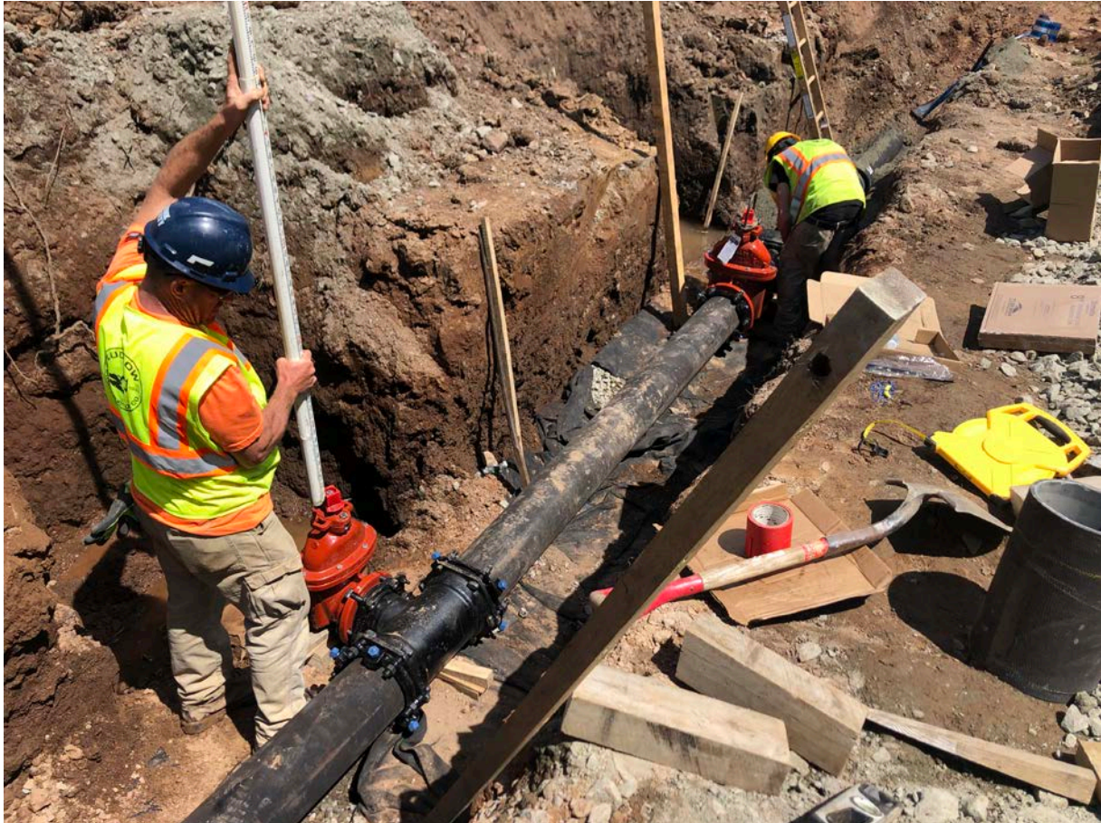
Picture 6: View of 8" DIP that Ludlow installed today between the booster station and previously-installed 8" DIP at Station 750+59 in Middletown, including an 8"x8"x8" M.J. C.L.D.I. TEE and an 8" M.J. gate valve and a fire hydrant assembly (8"x8"x6" M.J. C.L.D.I. hydrant TEE and a 6" M.J. gate valve). View to the east/northeast.
