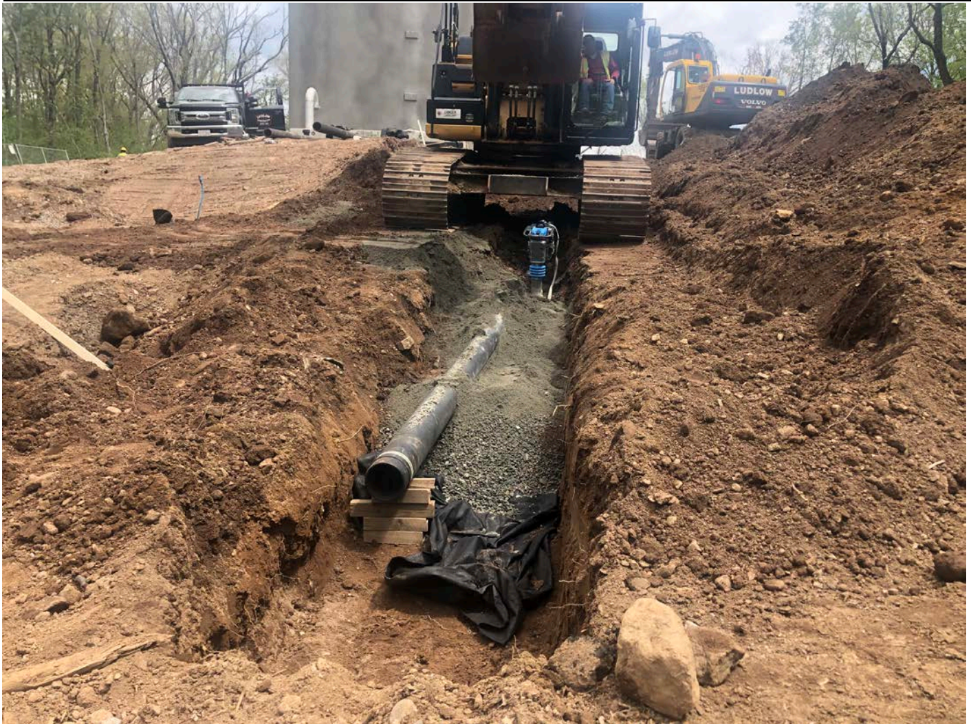
Picture 5: 8" DIP drain line that Ludlow is installing between the water tank and the headwall located at ~Station 11+70 in Middletown. View to the east.
