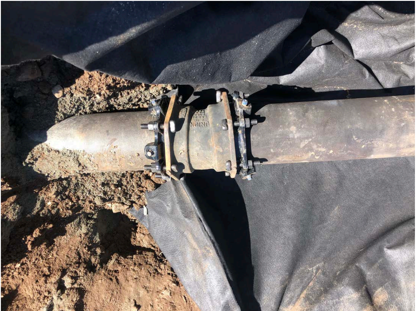
Picture 3: 11.25° DIP bend placed in line with the 8" DIP drain line that Ludlow is installing between the water tank and the headwall located at ~Station 11+70 in Middletown. View to the east.
