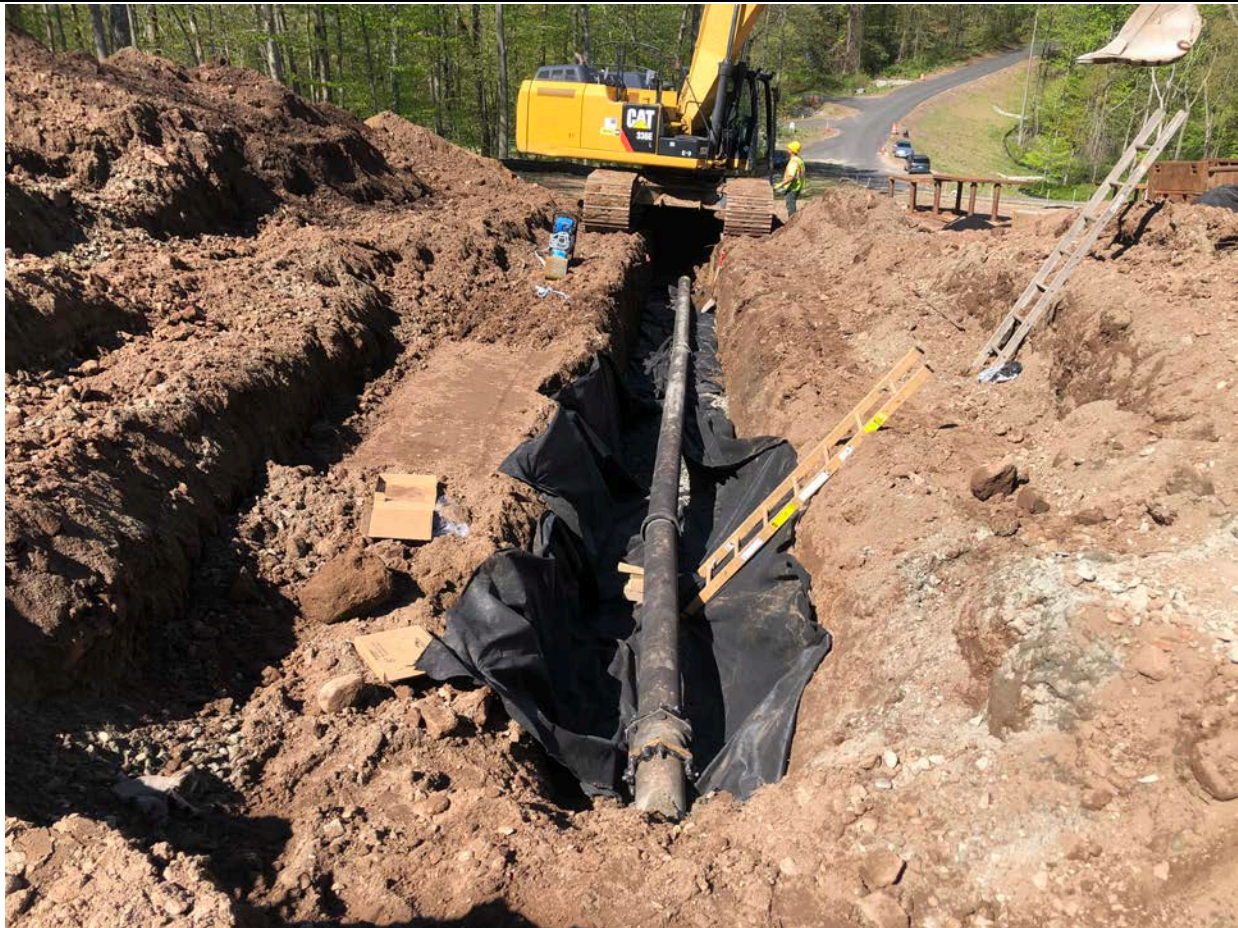
Picture 2: Geofabric placed over \frac{3}{4} " gravel and another layer of geofabric beneath the 8" DIP that is being installed for the drain between the southwest side of the water tank and the headwall located at ~Station 11+70 in Middletown. View to the west.
