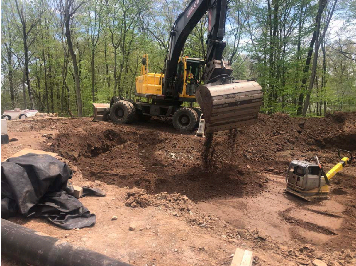
Picture 6: Ludlow placing native fill over the 8" DIP drain line between the southwest side of the water tank and the headwall located at Station 11+70. Water tank work zone located east of the Shared Access Driveway in Middletown. View to the south.
