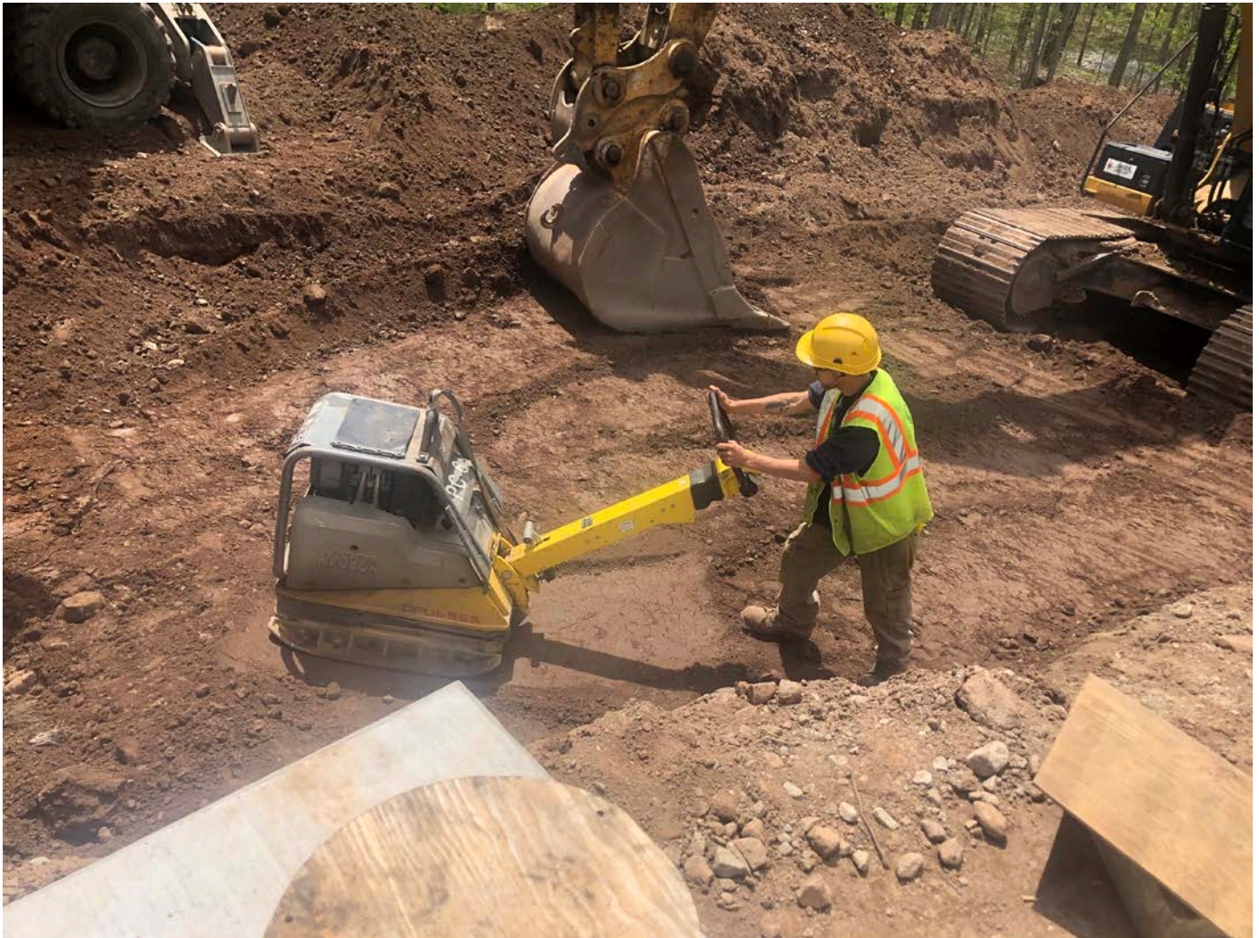
Picture 7: Ludlow compacting native fill over the 8" DIP drain line that runs between the southwest side of the water tank and the catch basin located at Station 11+70. Water tank work zone located east of the Shared Access Driveway in Middletown. View to the southwest.
