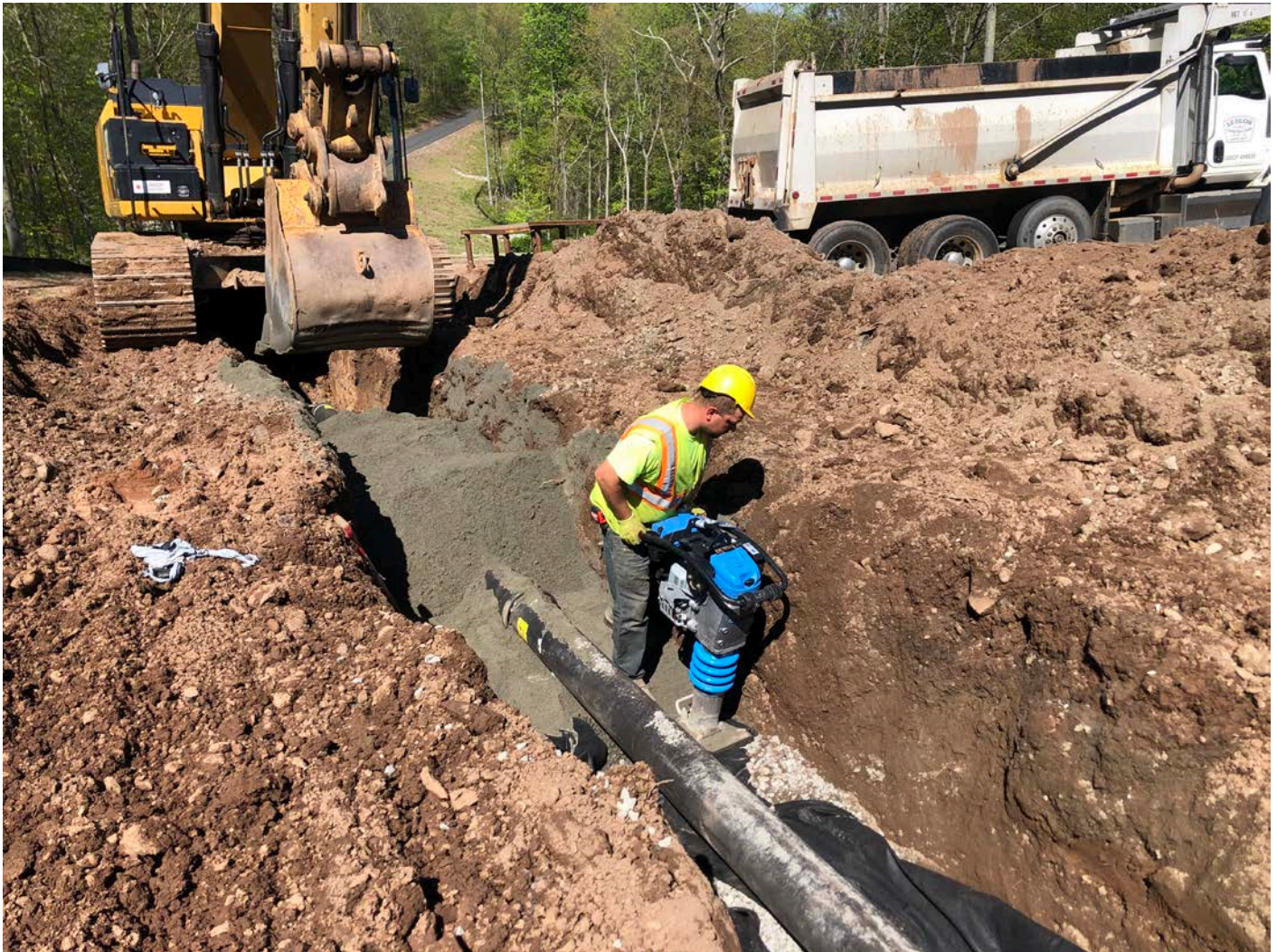
Picture 4: Ludlow placing and compacting sand on and around the 8” DIP drain line that Ludlow is installing between the water tank and the headwall located at ~Station 11+70 in Middletown. View to the northwest.
