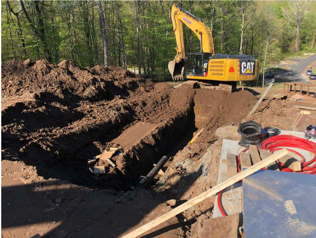
Picture 1: Ludlow in the process of installing 8" DIP for the tank drain between the southwest side of the water tank and the headwall located at ~Station 11+70 in Middletown. View to the west.
