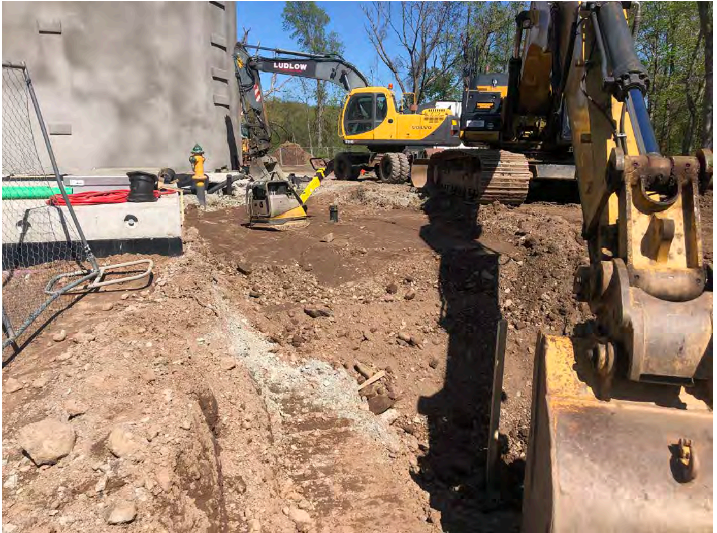
Picture 7: Final progress of placement of backfill over the 8" DIP drain line that runs from the southwest side of the water tank towards a headwall located at Station 11+70. Water tank work zone located east of the Shared Access Driveway in Middletown. View to the east.
