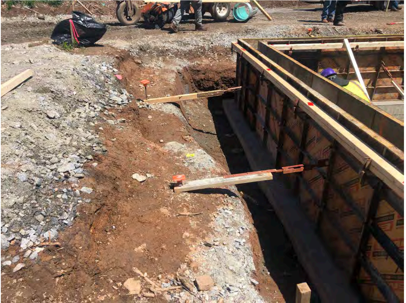
Picture 4: Bracing that Ludlow has placed on the exterior of the west side of the concrete form for the booster station frost wall. Station 750+63, South Main Street in Middletown. View to the north.
