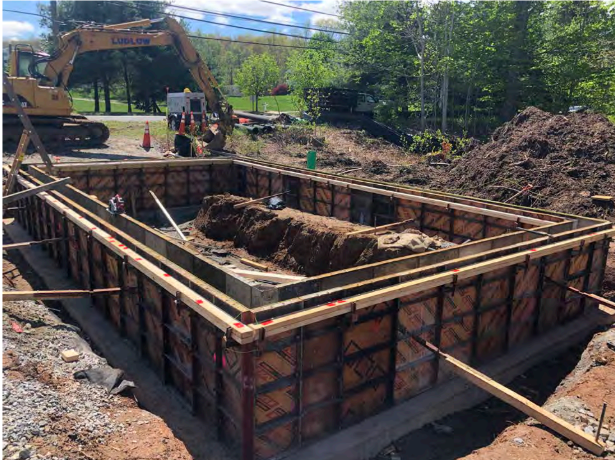
Picture 2: Bracing that Ludlow has placed on the exterior of the north and west side of the concrete forms and the interior of the east and south wall of the concrete form for the booster station frost wall. Station 750+63 South Main Street, Middletown. View to the southeast.
