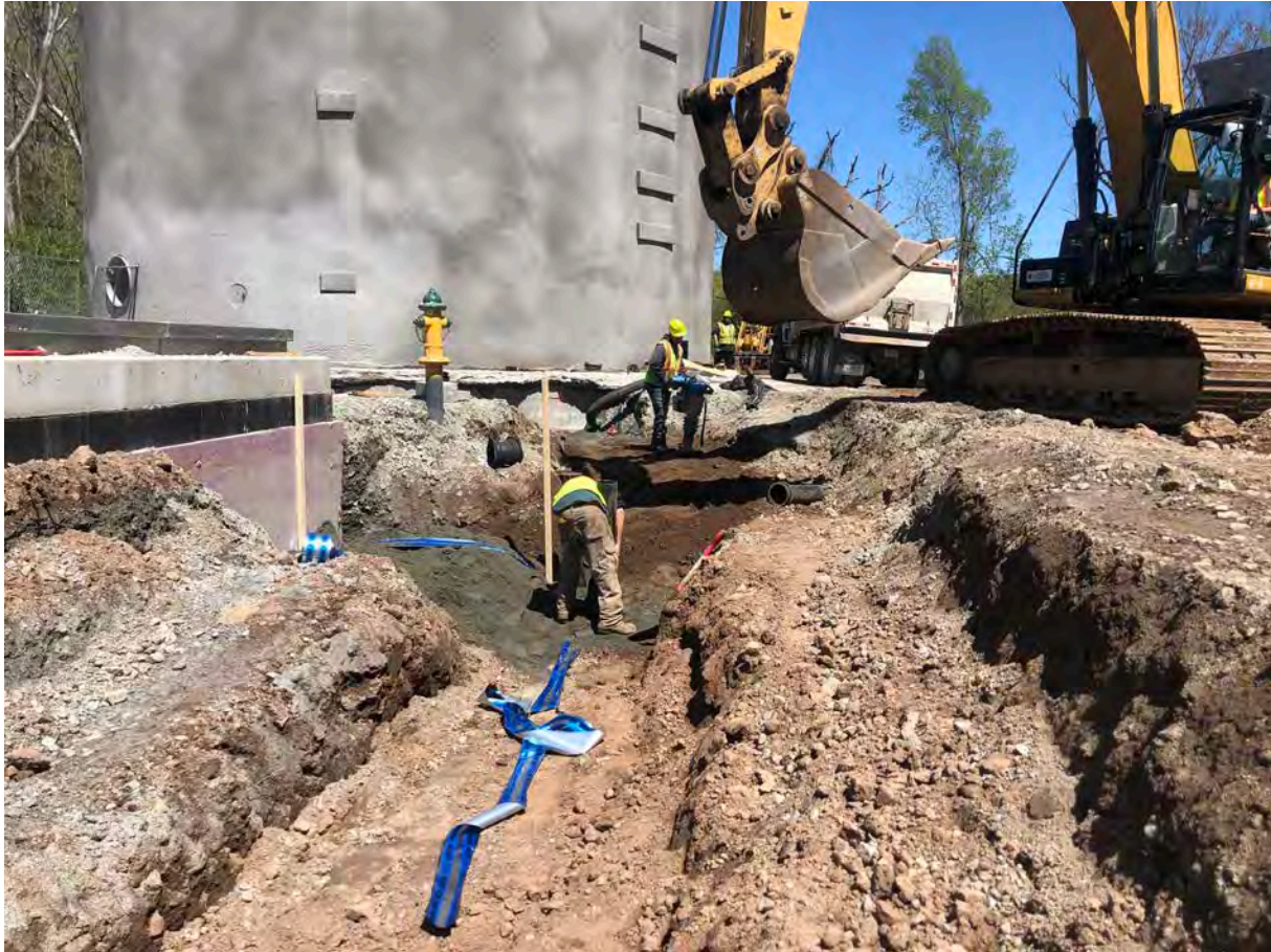
Picture 6: Ludlow placing backfill over the 8" DIP drain line that runs from the southwest side of the water tank towards a headwall located at Station 11+70. Water tank work zone located east of the Shared Access Driveway in Middletown. View to the east.
