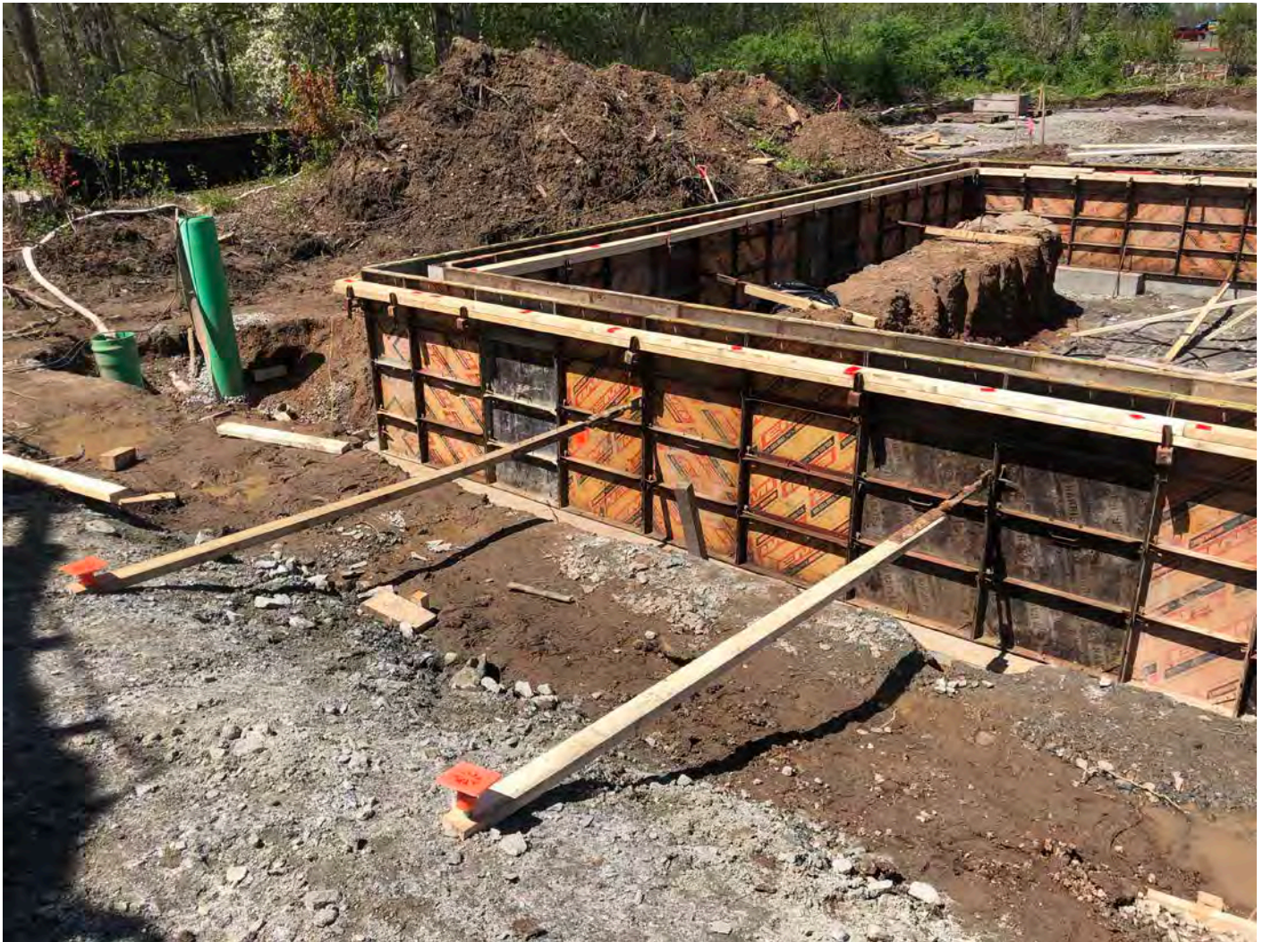
Picture 3: Bracing that Ludlow has placed on the exterior of the east side of the concrete form for the booster station frost wall. Station 750+63 South Main Street in Middletown. View to the southwest.
