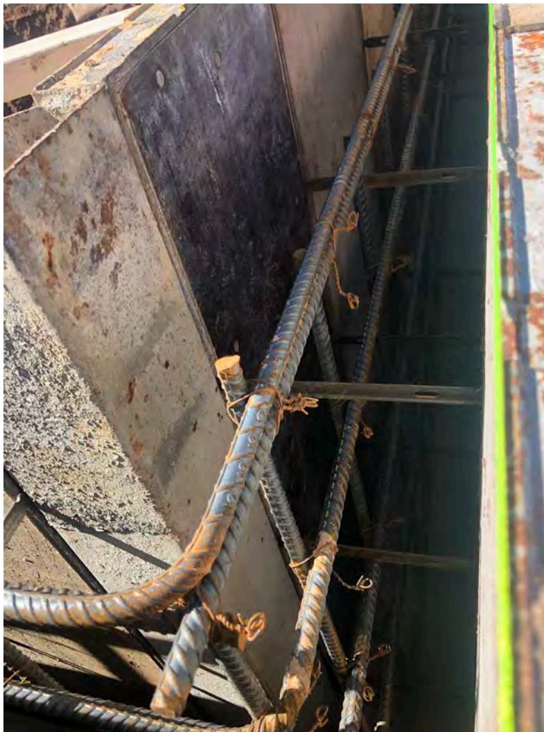
Picture 1: Overlapping rebar on a corner of the concrete form for the booster station frost wall located at Station 750+63 in Middletown. The corner overlaps meet or exceed the minimum overlap required.
