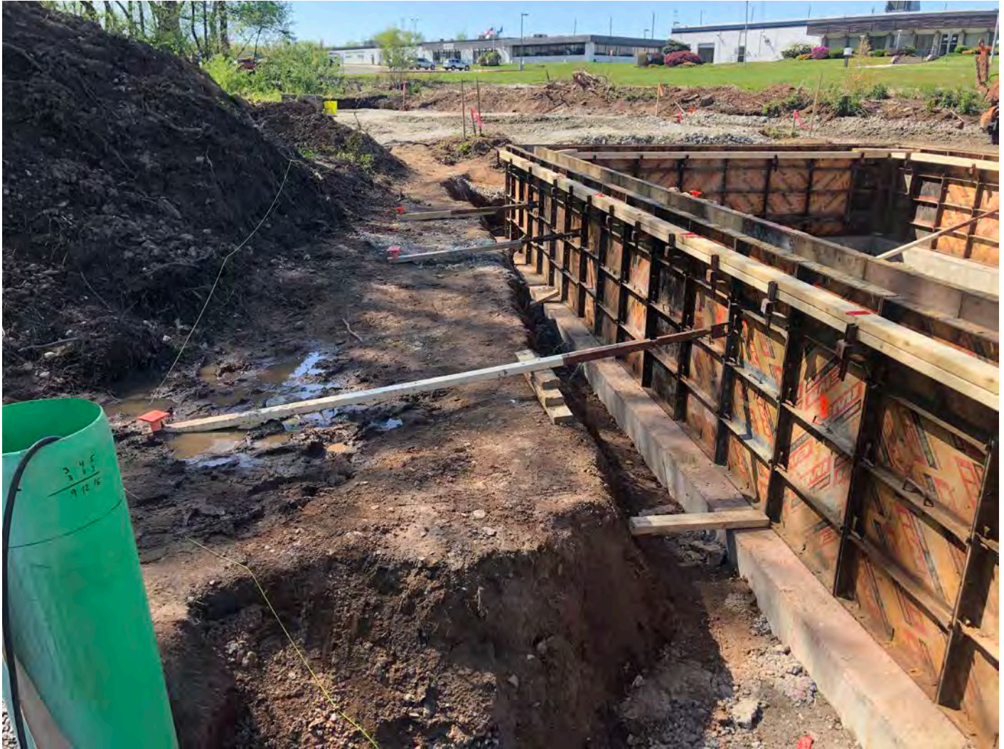
Picture 8: Bracing that Ludlow has placed on the exterior of the southern side of the concrete forms for the booster station frost wall. Station 750+63, South Main Street, Middletown. View to the east.
