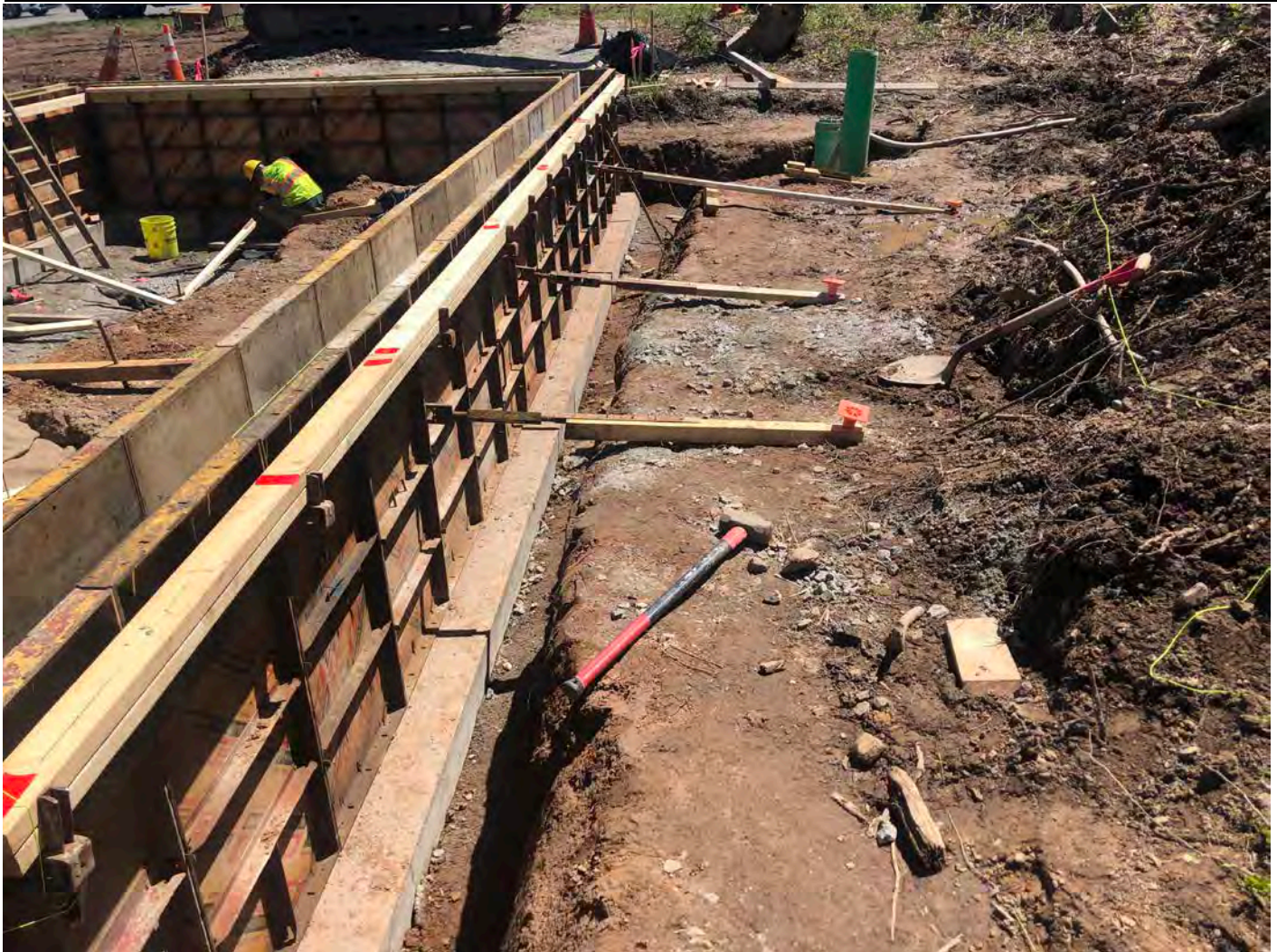
Picture 5: Bracing that Ludlow has placed on the exterior of the north side of the concrete form for the booster station frost wall. Station 750+63, South Main Street in Middletown. View to the east.
